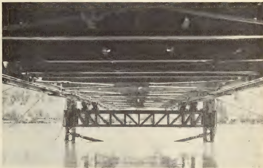
Fig. 8—The underside of the bridge supported on the trestle and rolling through on the rocking rollers.
