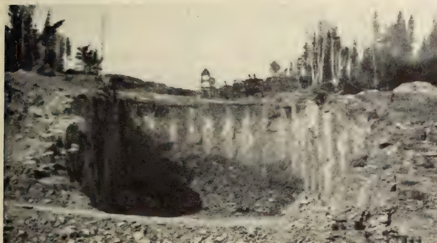
Fig. 11.—Face of west cut immediately after a blast.
