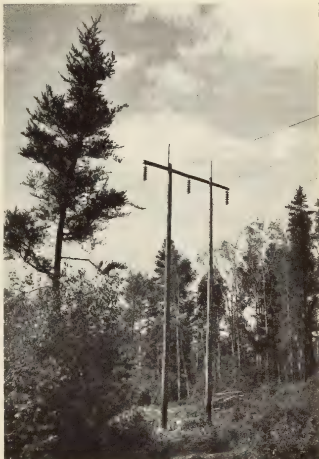
Fig. 3—Typical suspension structure—Steep Rock Line.
