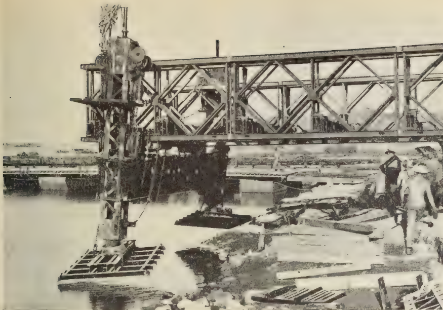
Fig. 7—Launching has begun with one trestle suspended from the end of the barge, and rolling forward is under way.
