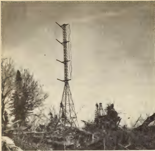
Fig. 12—The robust form in which directional antennas at high frequencies can be designed as exemplified by this 50 megacycle antenna. The total height is about 60 ft., and the construction is entirely of galvanized steel angle.
