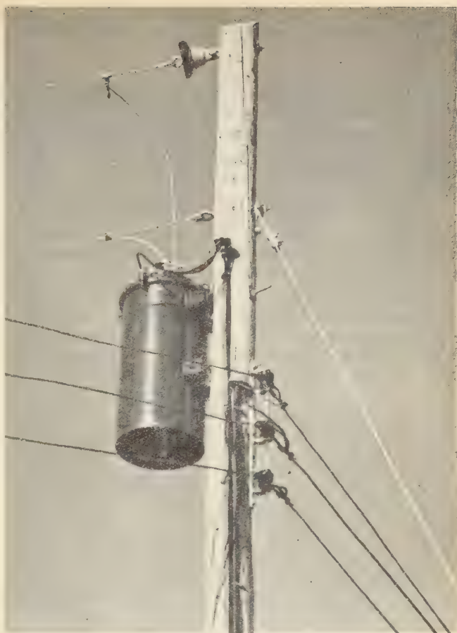
3 kva. transformer installation—6900V farm lines.
