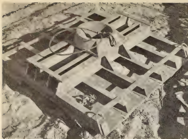
Fig. 4—The trestle footing complete with footing cables.
