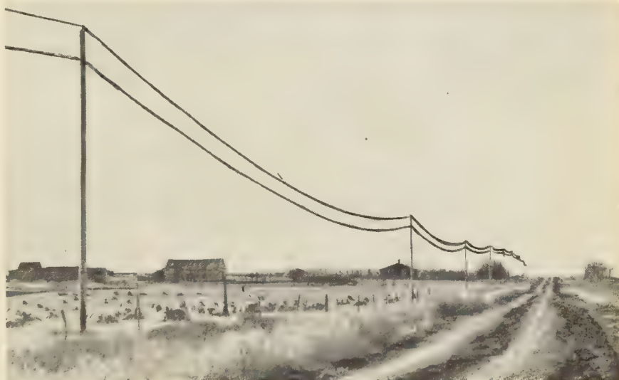
Section 6900 volt farm lines experimental area No. 1
