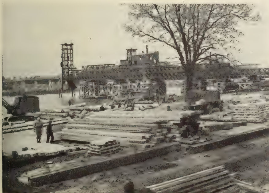
View of part of timber and pile yard at Zutphen. Note batter piles being driven by pile driving rig.
