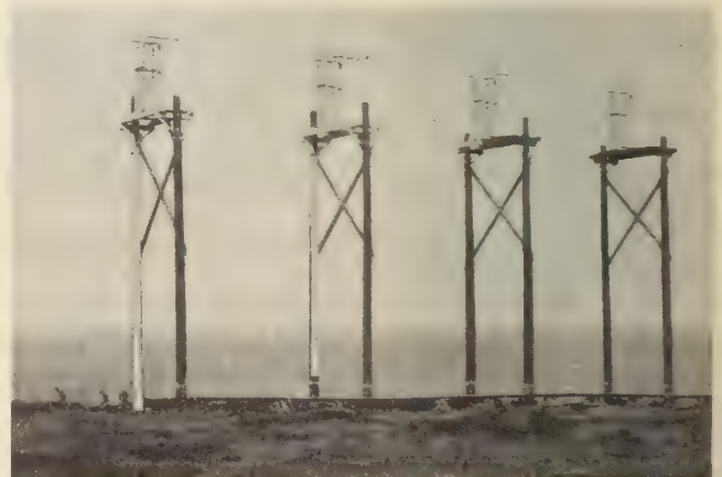
Fig. 13—At frequencies of the order of 100 megacycles simplified directional antennas become possible, and the cost and amount of land required for a site are both reduced.
