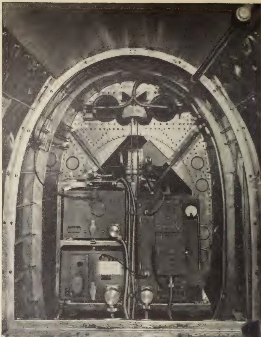
Fig. 3—Typical T.C.A. installation in tail of Lockheed aircraft.
