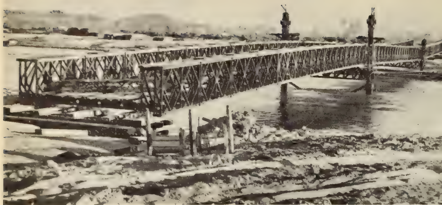
Fig. 9—The bridge is shown completely launched and supported on two trestles; the transoms are not adjusted to level up the bridge,
