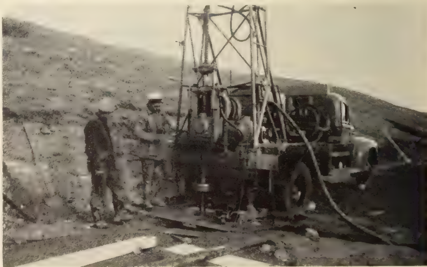
Fig. 1—Truck-mounted drilling unit in operation.
