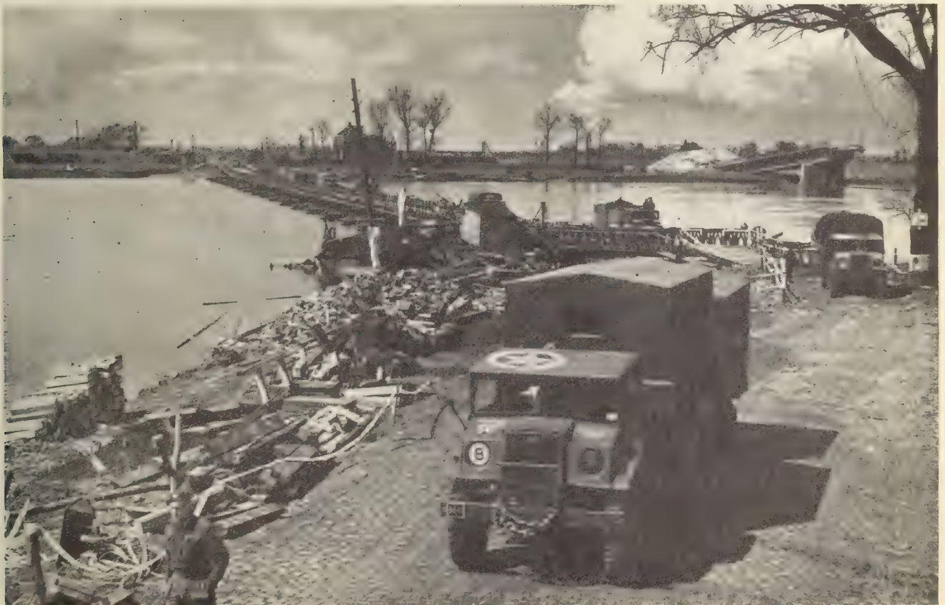
This is the "Gales" bridge, a thousand foot floating Bailey over the river Eems near Leer. The Eems is a tidal river which had to be crossed by the Canadians before Leer could be taken. (Canadian Army Overseas Photo)
