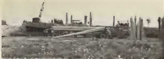
Unloading 50 ft. and 60 ft. timber piles—note transporter built specially for this task.
