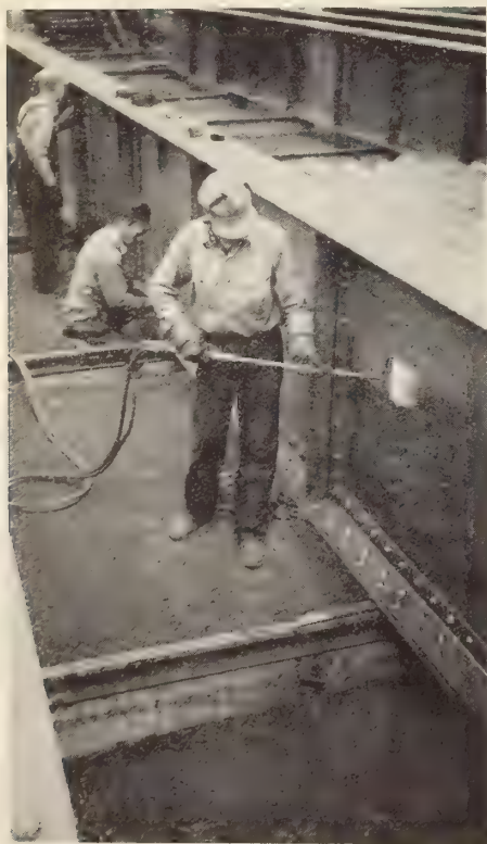
Fig. 4—These operators are flame-priming, sweeping and painting part of an order for 4,000 tons of structural steel members used in the construction of an overhead parkway system.
