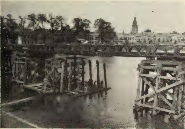
Class 70 navigation span 100 ft. long at Zutphen. (Temporary pile bent is being dismantled.)
