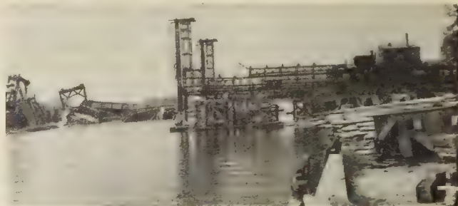
The two pile driving rigs at Zutphen viewed from up stream.
