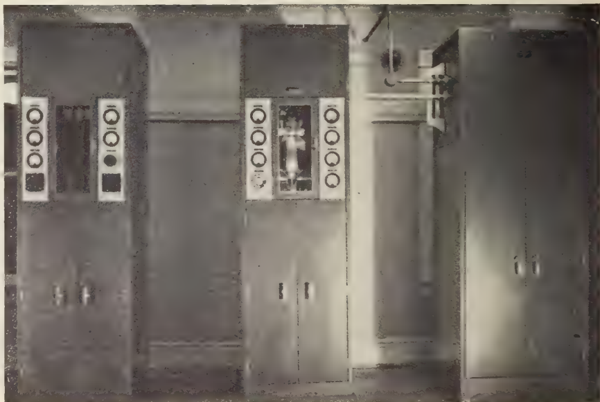
Fig. 1—Northern Electric Model 14C, 10 channel, crystal controlled transmitter used at majority of Trans-Canada Air Lines ground stations.
