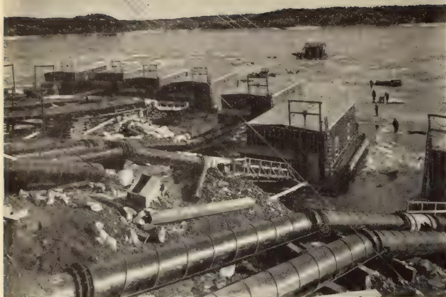
Pumping installation, showing connection to shore and flexible couplings. Lake down 15 ft. when picture taken; now down 135 ft.
