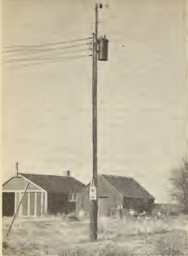
Transformer pole showing transformer and meter box—6900V farm lines.
