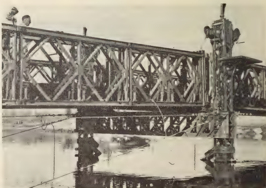
Fig. 10—The bridge has been split and the ends of the two simple spans lowered onto the trestle bearings.
