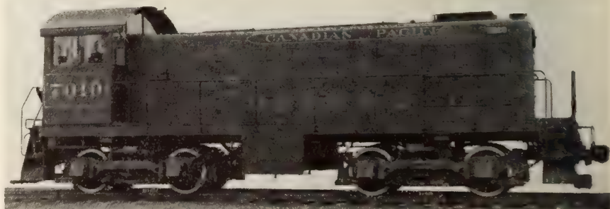
1,000 hp. Alco-G.E. Diesel-electric switching locomotive, 115 tons weight on drivers, 69,000 lbs. starting tractive effort.
