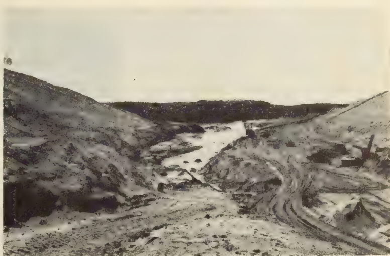
Fig. 10—Earth excavation in progress at the esker cut.
