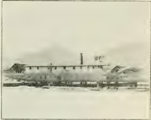
THE UPPER CABINS WERE TRANSFERRED TO THE NEW HULL WHICH WAS SUNK INTO POSITION THROUGH A HOLE IN THE ICE.
