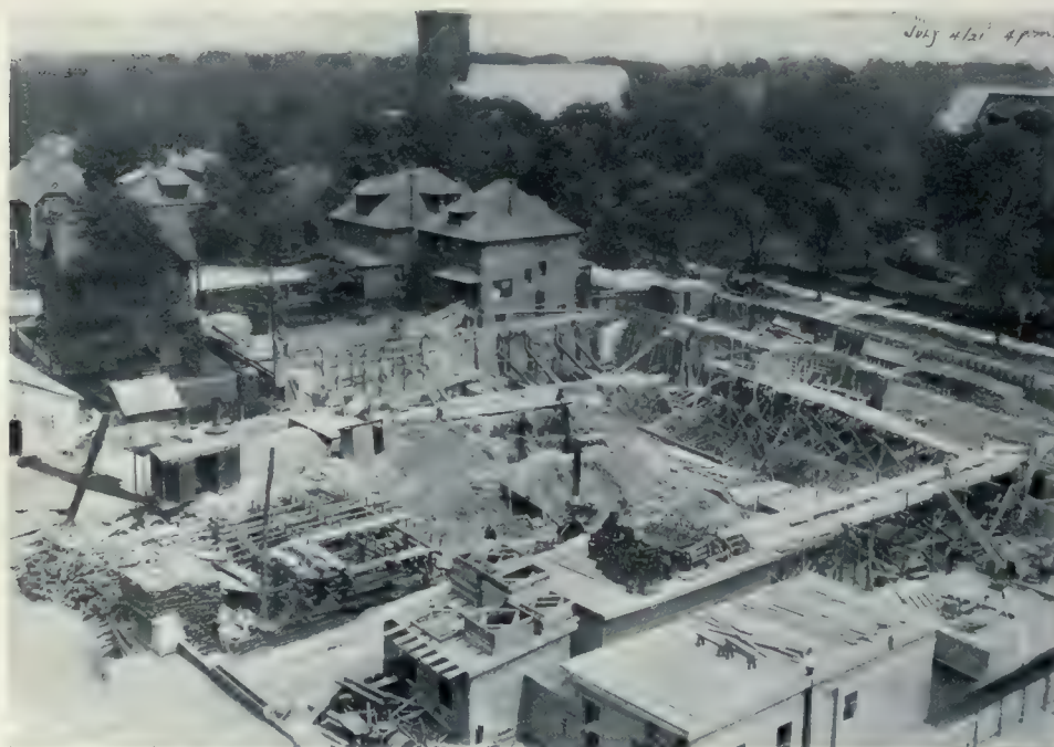
POURING OF FOUNDATION WALLS PRIOR TO ERECTION OF STEEL WORK.
