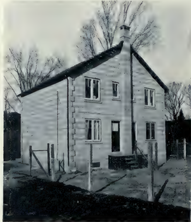
FRONT AND REAR VIEWS OF PAIR OF HOUSES AT TORONTO, BUILT OF MACHINE-MADE CONCRETE PARTS.
