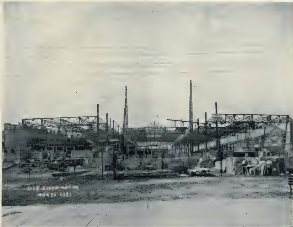
ROOF TRUSS IN PROCESS OF ERECTION
