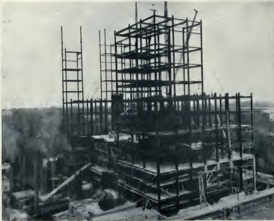
ERECTING FOUR FLOORS OF STEEL AT ONE LIFT
