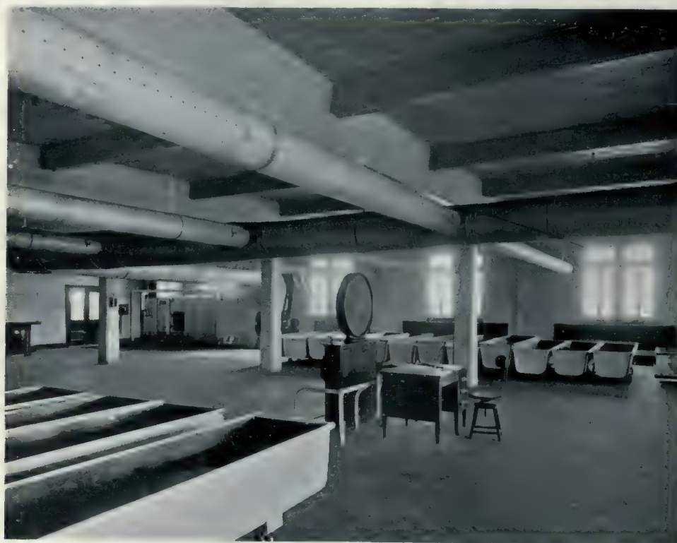
DOUGH ROOM, THIRD FLOOR, SHOWING HUMIDIFIER AND DISTRIBUTION FROM SAME. CANADA BREAD COMPANY'S BAKERY, DANFORTH AVENUE, TORONTO. MCCORMICK COMPANY AND CHARLES S. COBB, ASSOCIATE ARCHITECTS AND ENGINEERS.
