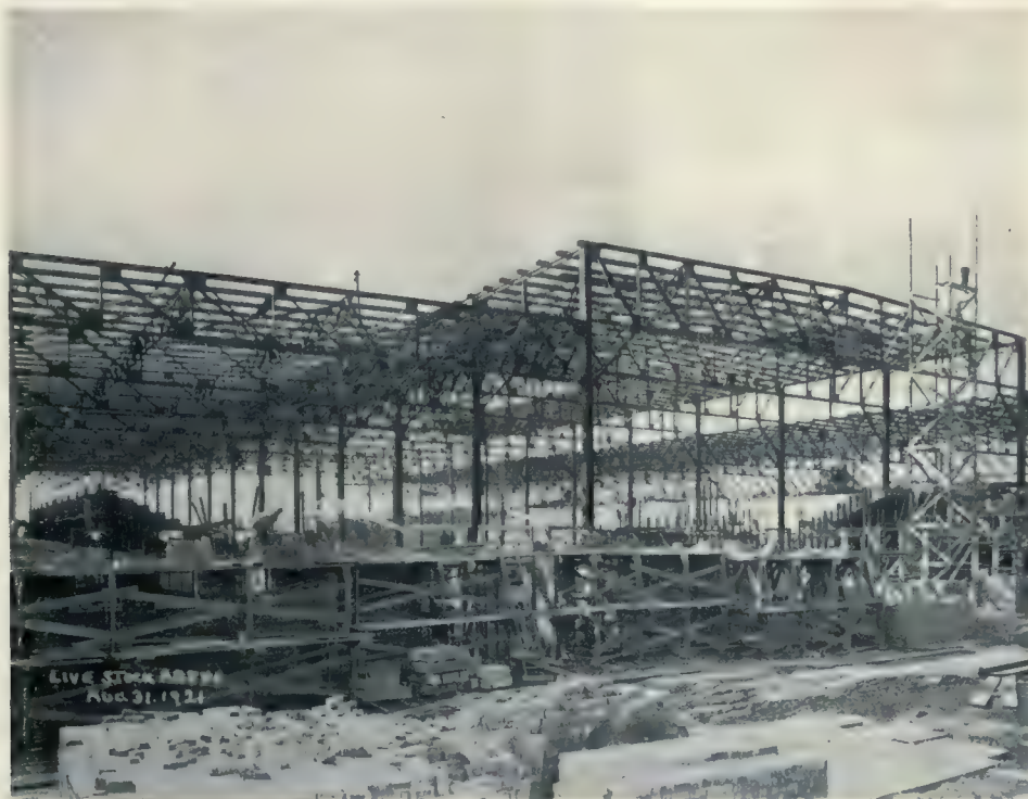
NEW LIVE STOCK BUILDING, CANADIAN NATIONAL EXHIBITION, TORONTO, SHOWING STEEL TRUSS WORK OVER ARENA COMPLETED
