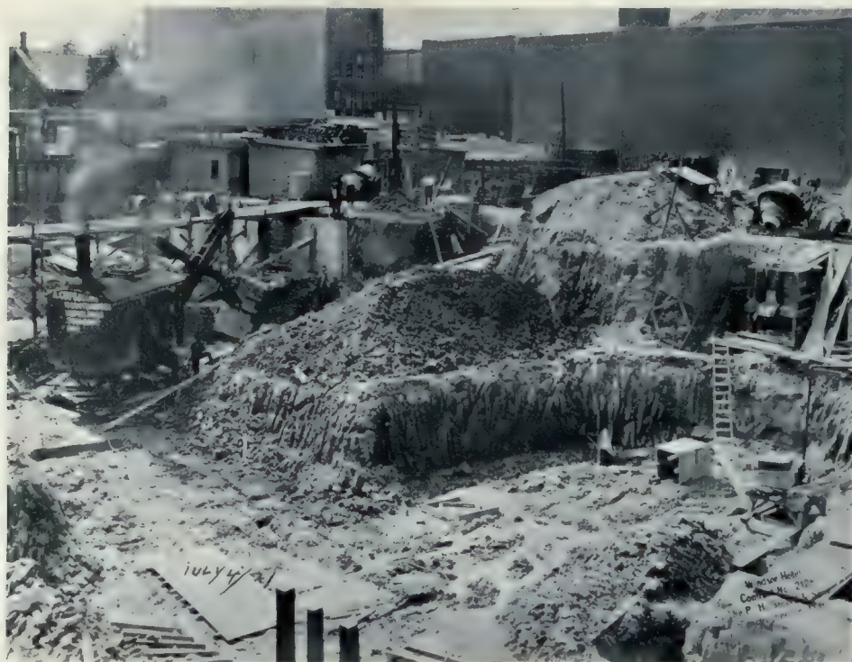
VIEW SHOWING TEETH MARKS OF STEAM SHOVEL INDICATING TOUGH NATURE OF FOUNDATION CLAY.
