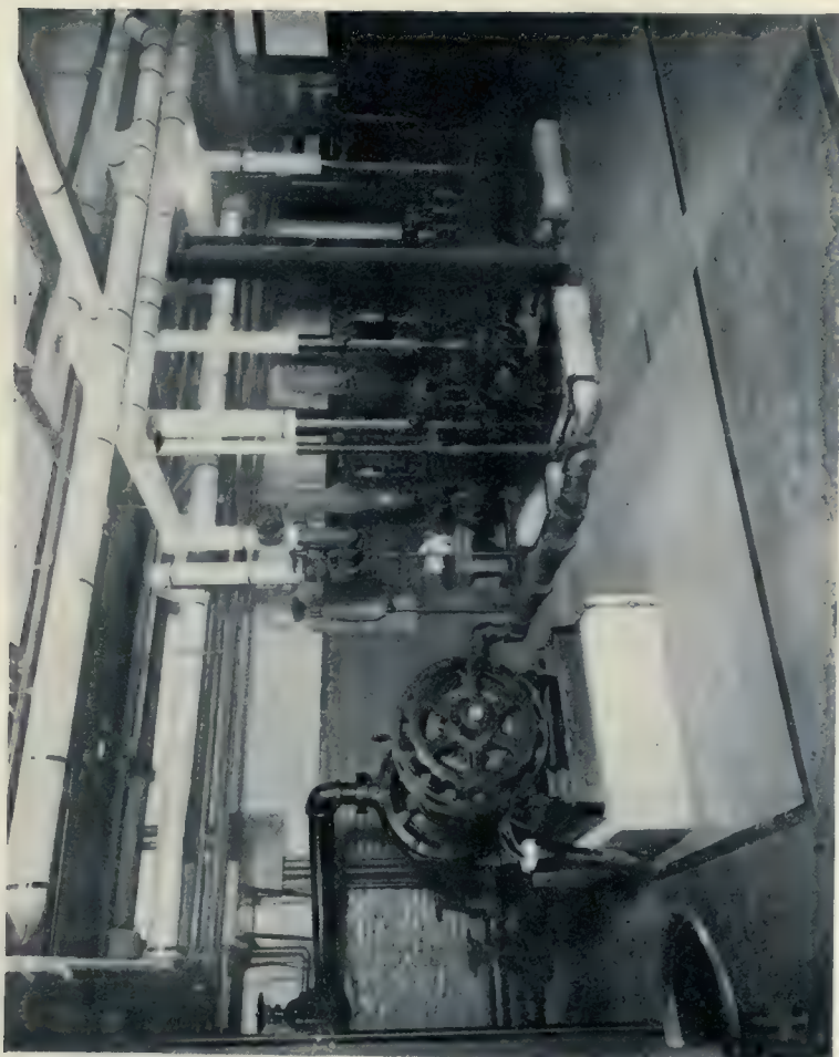
PUMP ROOM, SHOWING FIRE PUMP AND BOILER FEED PUMPS.
