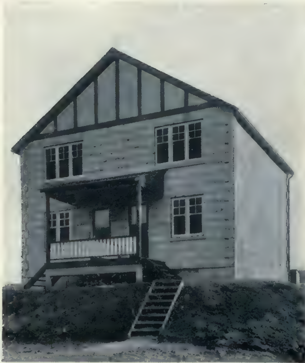
FRONT AND REAR VIEWS OF PAIR OF HOUSES AT TORONTO, BUILT OF MACHINE-MADE CONCRETE PARTS.
