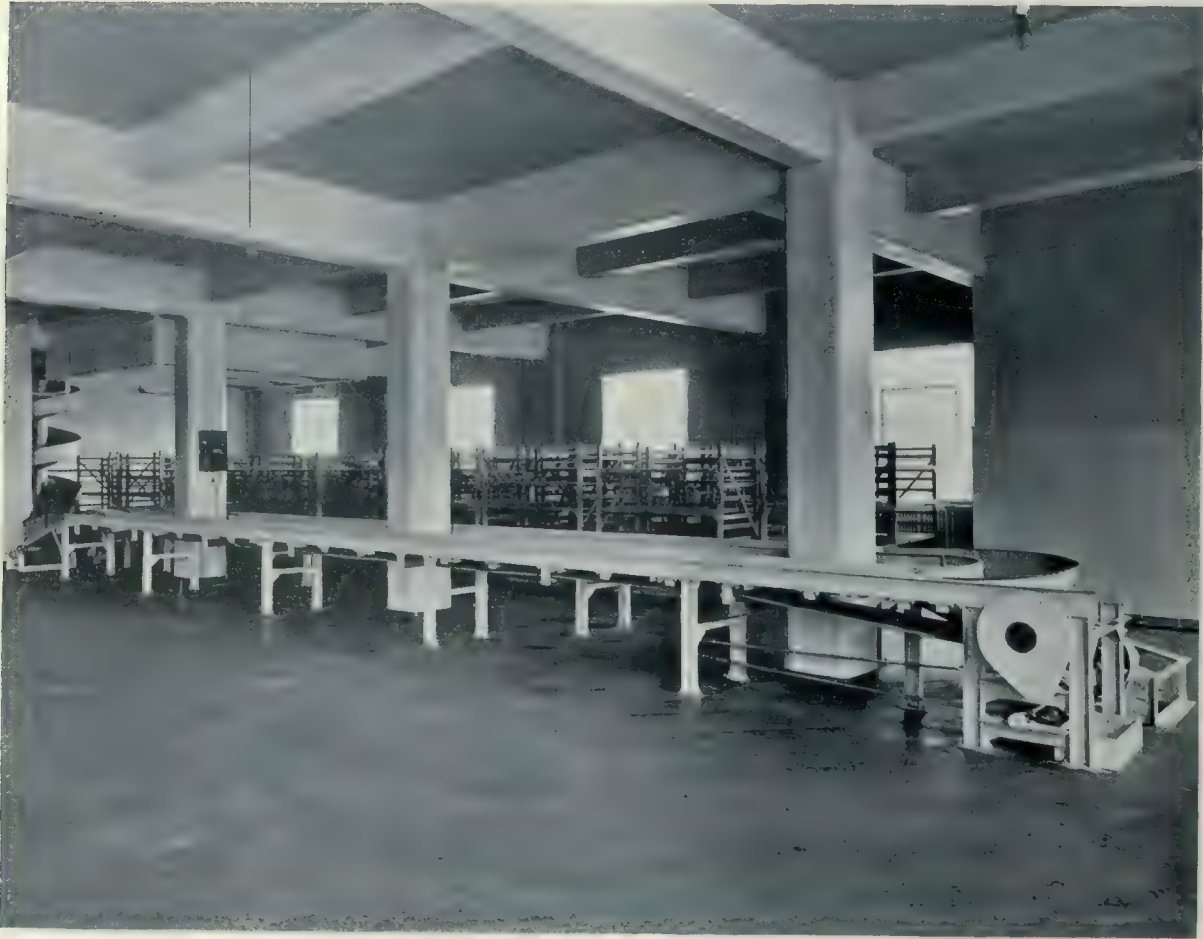
BREAD ROOM, FIRST FLOOR, SHOWING DELIVERY END OF BREAD CONVEYOR.
