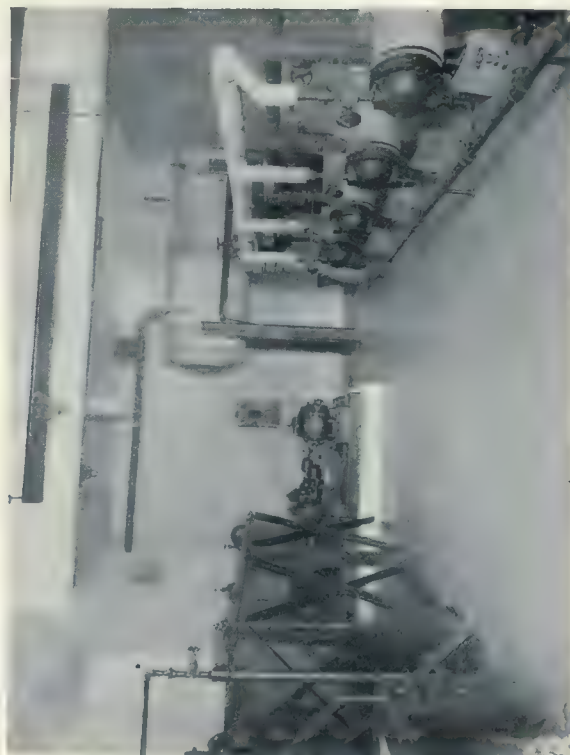
HOT WATER HEATERS AND DRINKING WATER TANK AND PUMP
