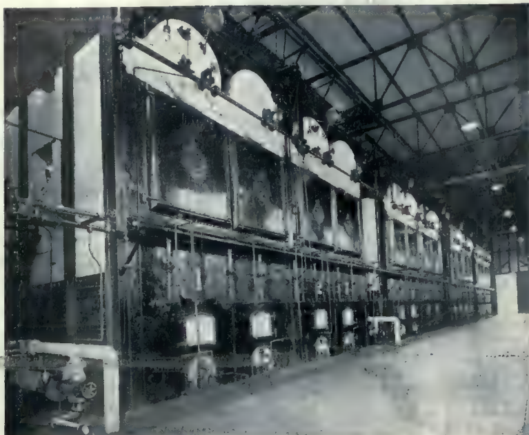
Showing the Boiler Room of The Imperial Oil Co. at Dartmouth, N.S. equipped with 8-G. & McC. Sectional Water-Tube Boilers
