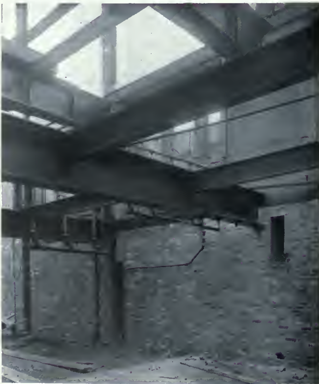
STEEL FRAMING SHOWING ADVANCED PIPING.
