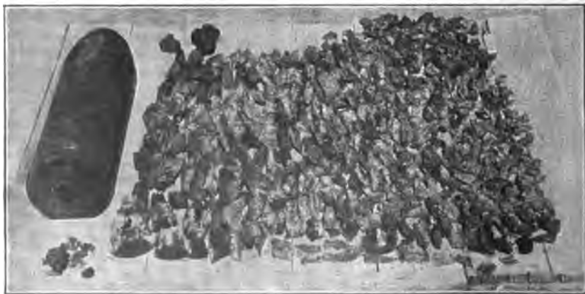
Fragmentation with 70 lbs. of Maximite of another 12-inch forged steel A. P. shell, which beautifully illustrates, by the regularity in size and the ragged character of the fragments, the terrific violence of the detonation.
