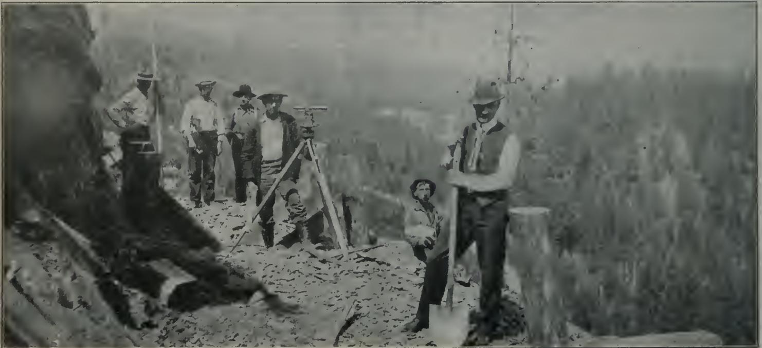
THE RAILWAY'S SURVEYORS CONSTRUCTING A BED FOR STEEL FLUME AT HORSE THIEF CREEK
