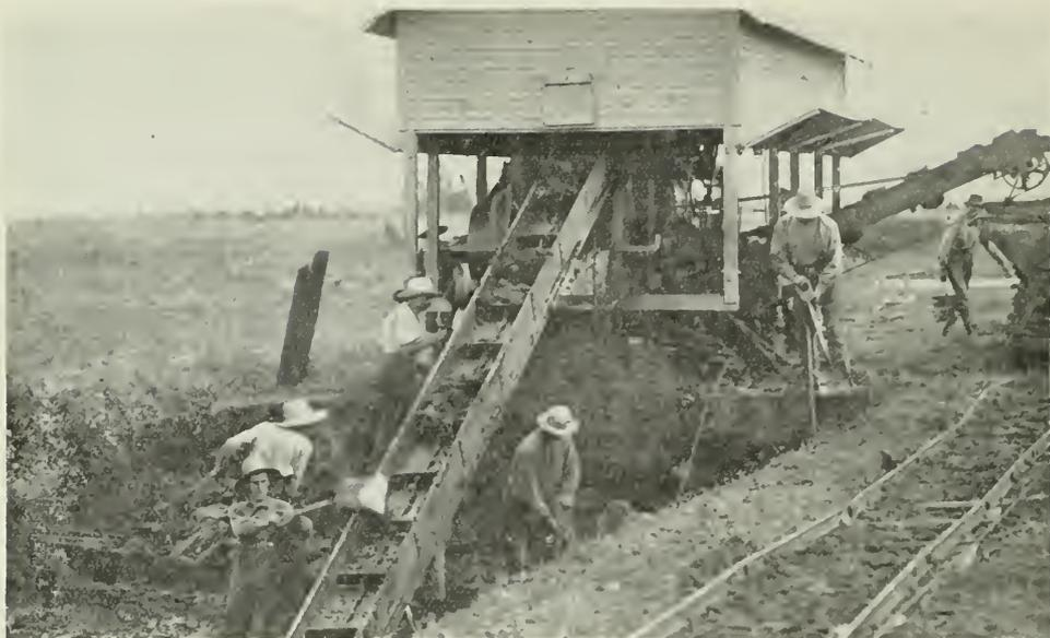
THE END ELEVATION OF A PEAT MACHINE. SHOWING THE ELEVATOR WHICH CARRIES THE PEAT OUT OF THE TRENCH. MEN AT WORK DIGGING THE PEAT AND THE TRACK ON WHICH THE CARS TRAVEL WHICH HAUL THE PEAT AWAY
