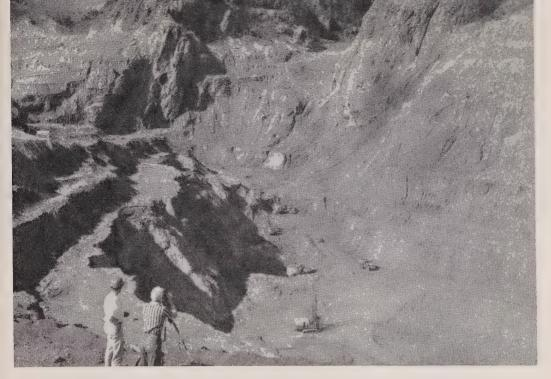
The famous open pit iron mine at Steep Rock, Ontario, where the ore is mined in 30-foot cuts or benches. Explosive is used to blast the ore into a size that can be carried away by diesel truck. Canada now ranks second (after France) among the world's iron ore exporting countries.
