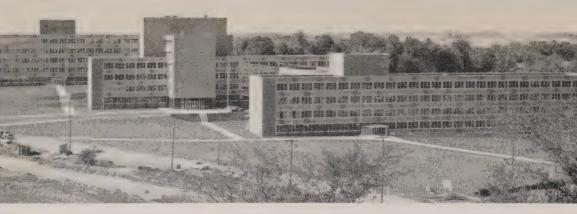
The \$7,000,000 Sir Charles Tupper Building, completed in 1960, consists of five blocks at different ground levels and has a total area of 421,380 square feet. Built to house the offices of various government departments, its exterior finish is of buff coloured brick with granite trim and porcelain enamel spandrels separating rows of metal windows.
