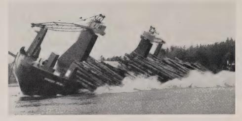
A self-dumping barge carrying 1,000,000 board feet of spruce and cedar discharges its cargo in three to four seconds on arrival at the booming grounds. Advantages over transport by deep-sea raft are that barges can be towed faster, there is less danger of losing logs in a storm and, since the logs spend less time in salt water, damage from insects is reduced.
