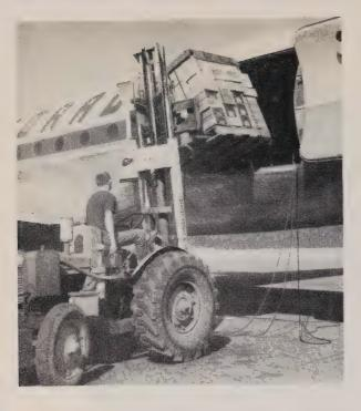
"Palletizing", or the strapping of loads of freight to pallets which are then forklifted into aircraft, has vastly speeded operations at both ends of the flight.
