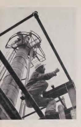
The stripper tower rises above a workman on the naphtha desulphurizer at a Calgary refinery. This unit is the largest addition in a \$1,500,000 expansion program which has increased crude running capacity from 7,500 to 10,000 barrels per stream day.
