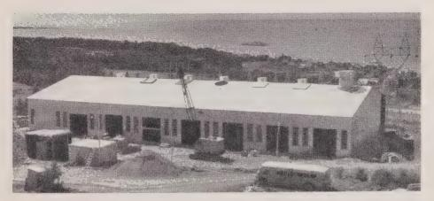
A 36,000 kw. gas turbine plant at Les Boules, Que. will act as a standby plant for the Gaspé Peninsula which is now served by 28 miles of underwater cable, laid in 1954. The present system has been difficult to maintain, due to severe weather and ice conditions. The new plant will also provide extra capacity to meet the winter peak and will act as a synchronous condenser for most of the time. This is Hydro Quebec's first thermal plant.
