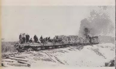
Laying the first transcontinental railway during the 1880's was a political necessity and an engineering achievement. For hundreds of miles the roadbed had to be blasted out of rock.
