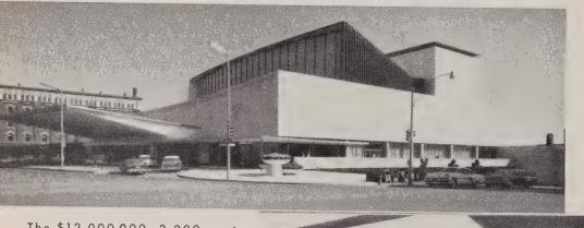
The \$12,000,000, 3,200-seat O'Keefe Centre for the Performing Arts opened in October, 1960, in Toronto. Special features include a mechanically elevated 50-piece orchestra pit; production, radio and television control rooms; remote-controlled stage lighting; full size rehearsal hall; kitchens; street-level access to theatre and stage and escalators to the balcony; special provisions for hard of hearing and invalids in wheel chairs.
