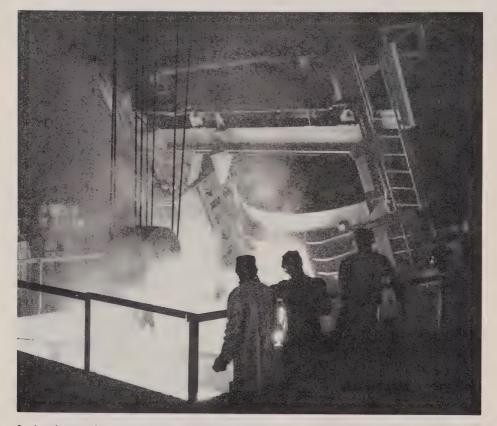
Saskatchewan has recently built its first steel plant, on the outskirts of Regina, for the production of pipes from  $3\frac{1}{2}^{"}$  to  $16^{"}$  in diameter. Here one of the two electric furnaces is tipped to pour molten steel into a huge bucket from which it will be poured into ingot moulds. The entire furnace tips forward for this operation.
