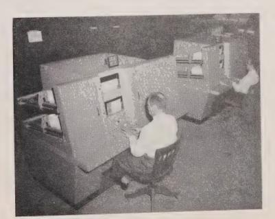
Two operators at the letter coding desks of the Post Office's new electronic sorting machine.
