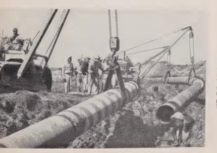
Laying the 51-inch pipeline from Winnipeg to the international border near Emerson, Manitoba. The first gas deliveries through this line to the United States took place in October, 1960. connection with this project, work commenced on the 108-mile, 36-inch pipeline which will carry gas from the Foothills Division line to the British Columbia-Idaho border.
