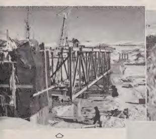
Steel erection on the cantilever section of the Champlain Bridge over the St. Lawrence Seaway continues during winter, thanks to Arctic clothing, safety precautions and improved machines.
