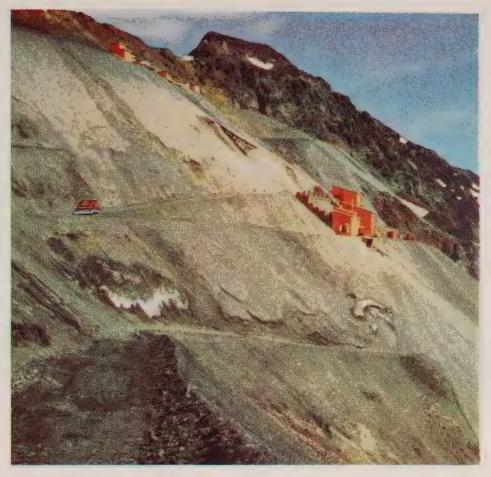
A six-mile road snakes up McDame Mountain in British Columbia to the upper levels where asbestos is mined. Mineral is dumped at the upper level, crushed and conveyed down to the lower plant where it is loaded into tramline buckets which carry it three miles to the mill at the foot of the mountain. This mine produces about 40,000 tons of asbestos a year.
