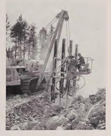
Four shot holes are made simultaneously by this "quad-drill", used in the construction of natural gas pipeline. The holes are tamped with explosives and detonated. In northern Ontario, granite first had to be blasted from the right-of-way to enable equipment to get through and then the five-footdeep ditch was blasted out, mile by mile.
