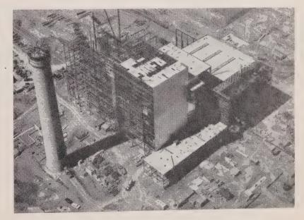
Installation of major equipment at the Nuclear Power Demonstration Station near Rolphton, Ontario, is going ahead. Canada's first nuclear power plant, known as NPD, is scheduled for operation during 1961. It will generate 20,000 kw. and is intended to be used as a demonstration plant to provide a training centre for operators who will be required in the large nuclear power plants planned for the near future.
