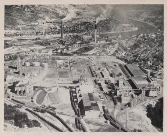
The Trail, British Columbia, operations of the Consolidated Mining and Smelting Company, showing the chemical fertilizer plants in the foreground and the metallurgical operations in the background, which includes the largest zinc plant in the world, producing 530 tons per day of zinc, 400 tons of lead, 1,600 tons of fertilizer plus significant quantities of silver, cadmium, bismuth, gold, antimony and indium.
