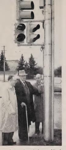
An experiment in the use of "traffic audio-lights" has been tried out in Edmonton, Alberta. A fast "beep" tone, synchronized with the lights, means it is safe to cross north and south, and a slow "beep", east and west.
