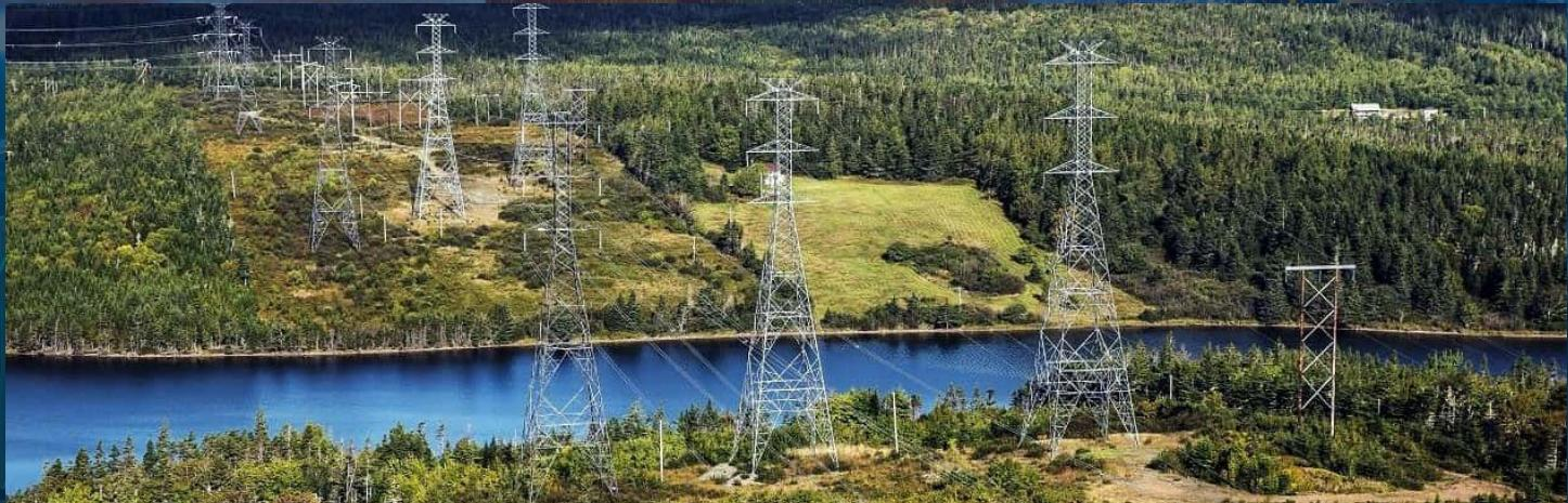
The Nova Scotia-New Brunswick Wasoqonatl Reliability Intertie is a 160-km, 345 kV transmission line running from Onslow, NS, to near Salisbury, NB. It will double the transfer capability between the two provinces, enabling more renewables, improving reliability and serving as the first phase of a modified Atlantic Loop.
