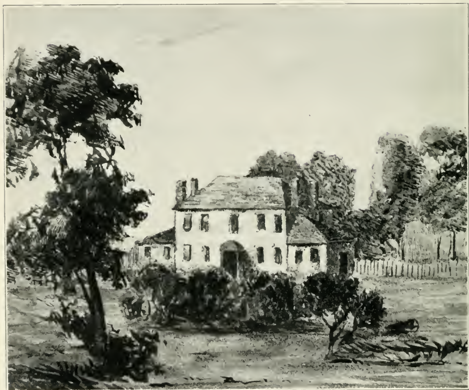
RESIDENCE OF ROBERT HAMILTON, QUEENSTON.
