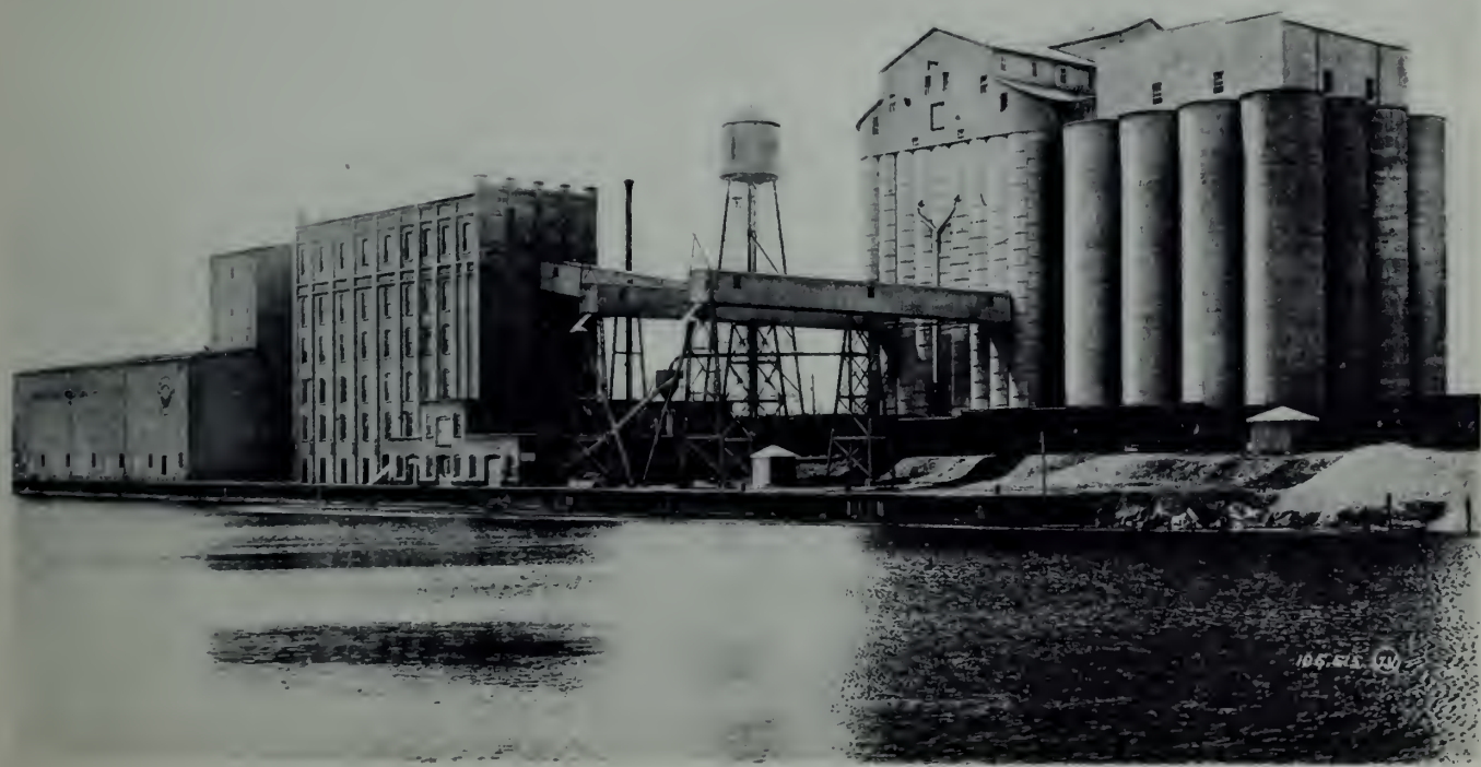
OGILVIE ELEVATOR AND FLOUR MILLS
