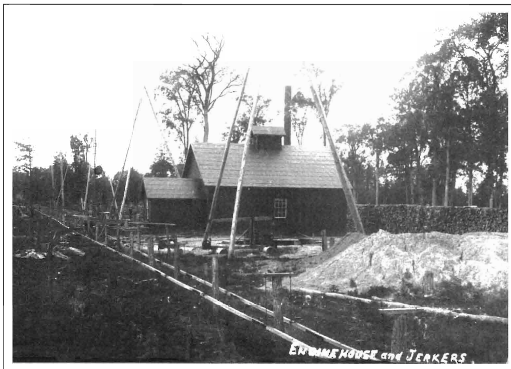
EXHIBIT 30: A Jerker Line Pumping System and Engine House Circa 1900.
