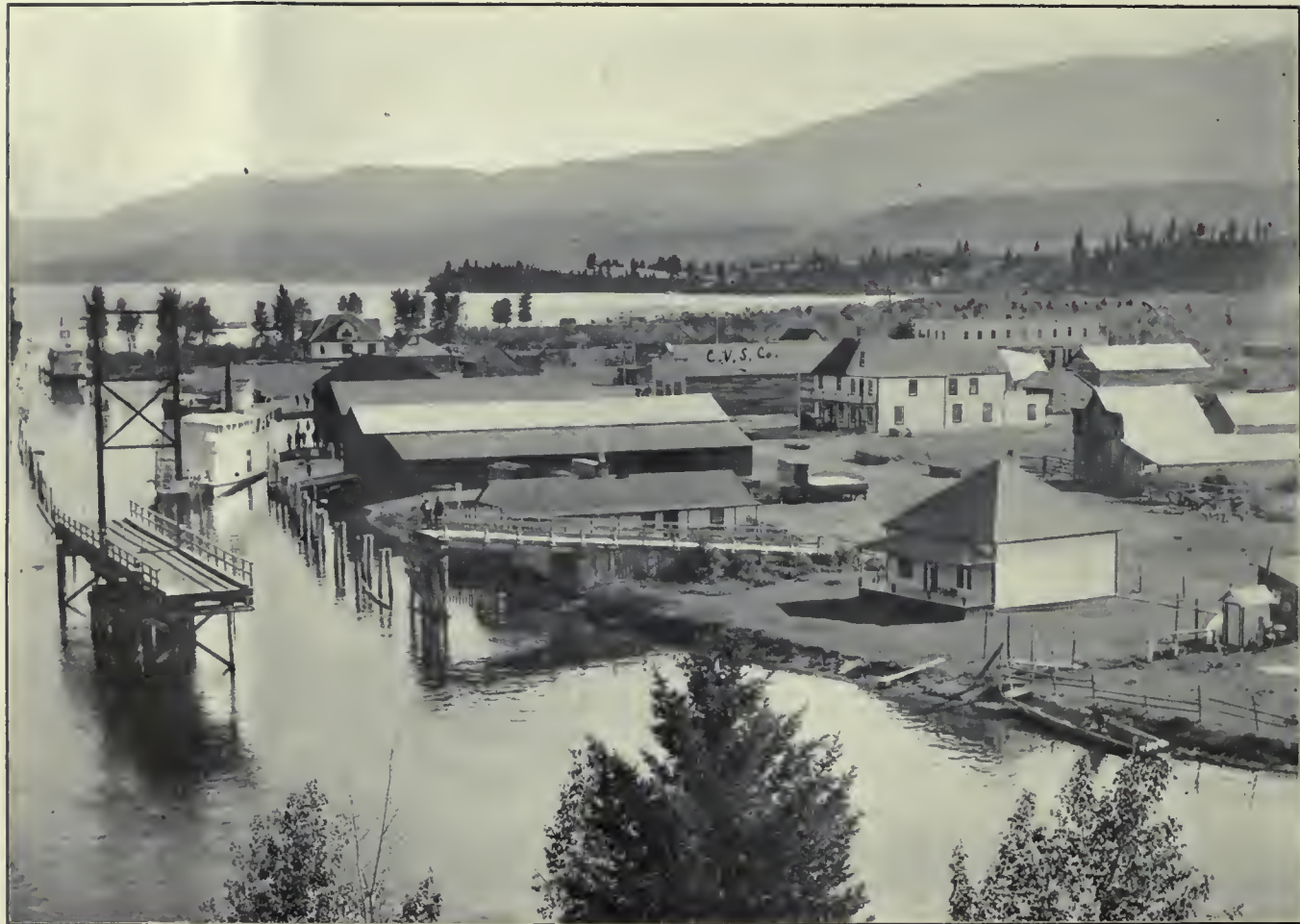
STEAMBOAT LANDING AND SWINGING BRIDGE, ATHALMER
