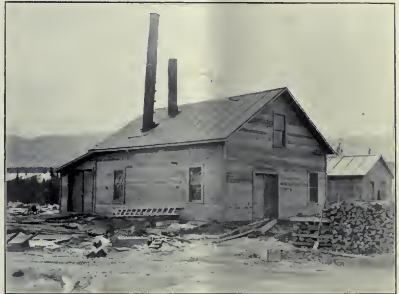
CITY ELECTRICAL POWER HOUSE, ATHALMER
