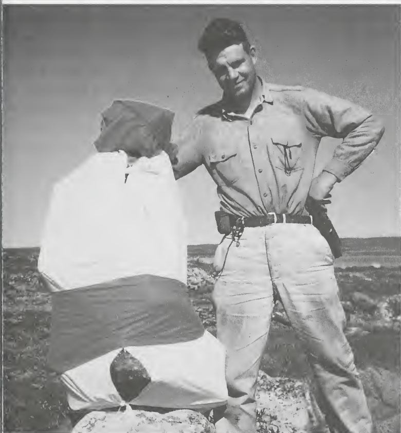
R. E. Follinsbee at a triangulation post, Mathews Lake, Northwest Territories, 1948. With no timber available, the topographer, Eric Fry, used an Inuit assistant versed in erecting Inukshuks to create an equivalent.
