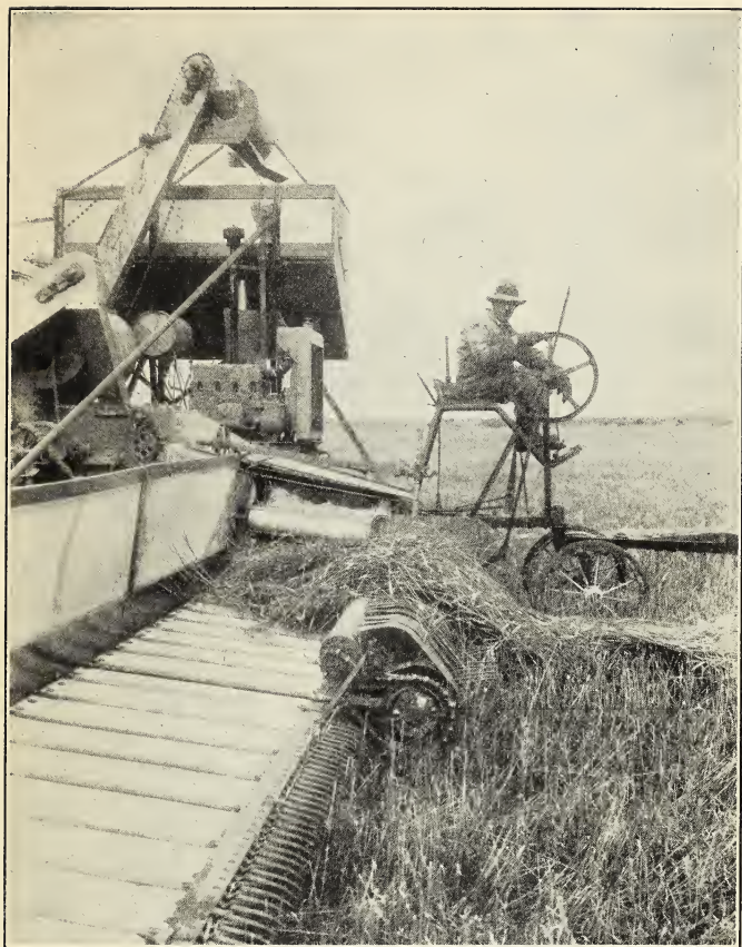
Fig. 142. Harvester-Thresher showing pick-up attachment in use. (Courtesy of McCormick-Deering.)
