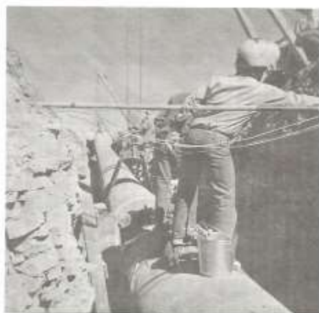
Laying the gas line across Lane's farm. 1970.
