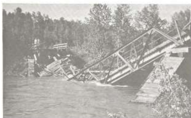
In 1951 the bridge went down with a D7 cat and scraper. River flooding over road, south of bridge. Bridge piles on north end of bridge broke and the bridge fell in. Russell Simpson was operating the cat.
