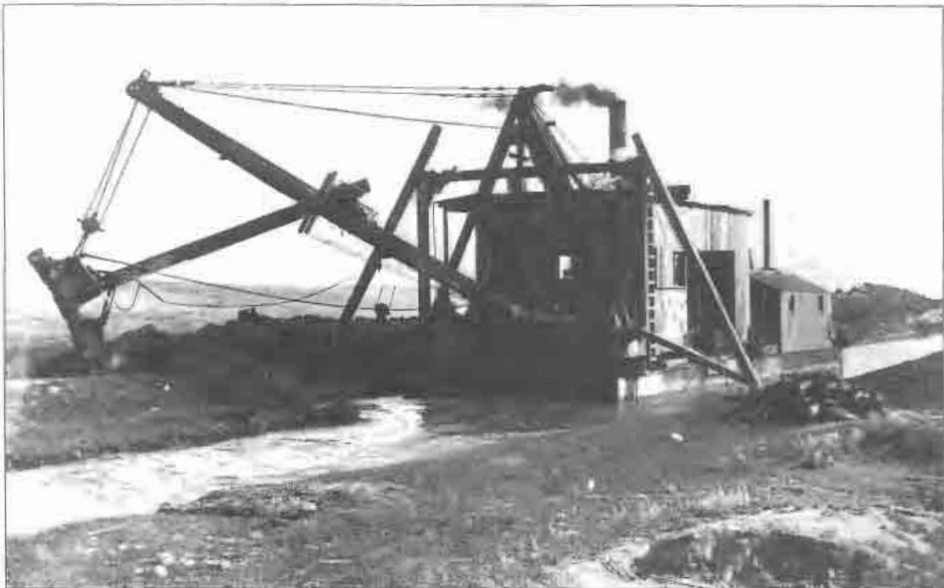
A dredge excavating an irrigation canal near Lethbridge in the 1890s.
