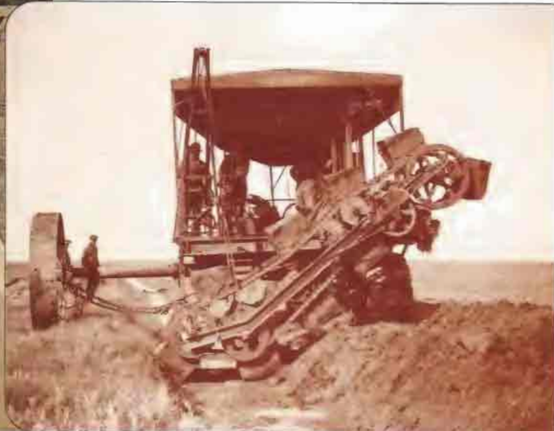
(Below) A Ruth dredger near Brooks, Alberta, in 1919. This dredge, which straddled approximately 18 feet when in operation, was used to clean up and enlarge irrigation ditches.
