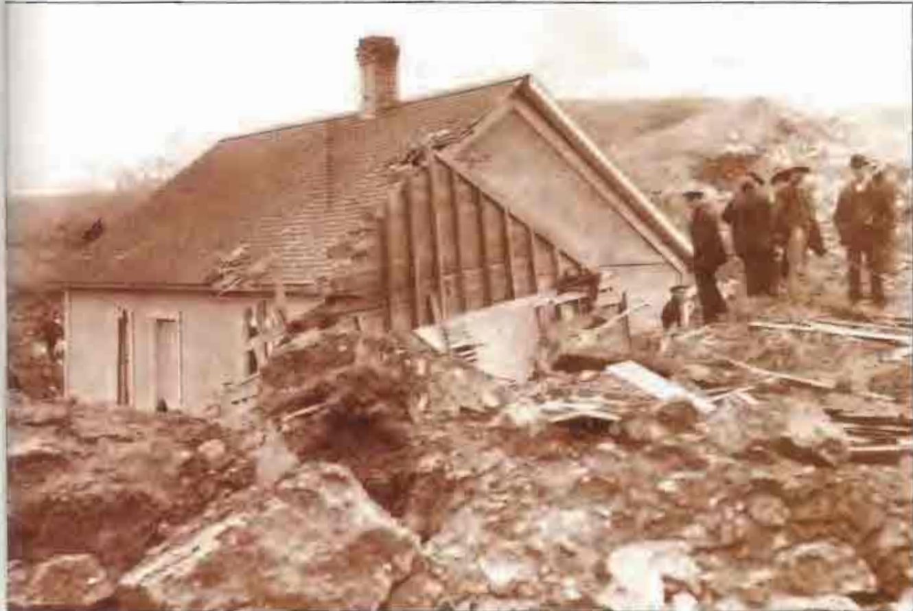
(Above) Although upright, the Bansemer house was badly damaged by the slide. The men in front of it are standing on the rubble which buried the Clark house, killing Mrs. Clark and her six children. Mr. Clark was also killed when the slide demolished the mine tippie.
