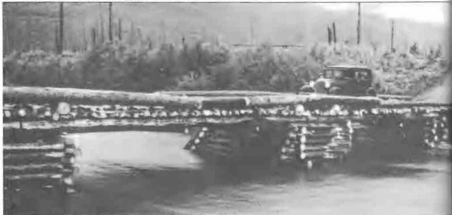
(Above) Constructing the Kinuseo Creek bridge in 1938. (Below) The completed Kinuseo Creek bridge, with its span of 112 feet that cost all of $50 in materials.
