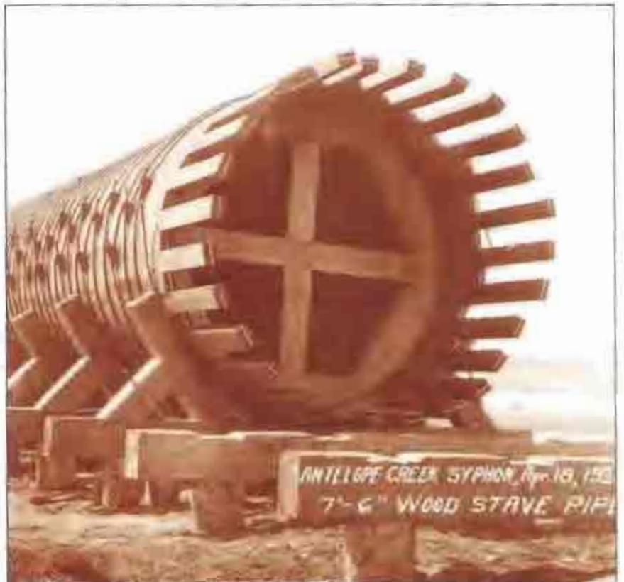
(Below) The Antelope Creek syphon, in the Eastern Irrigation Section of southern Alberta, during construction in 1921.
