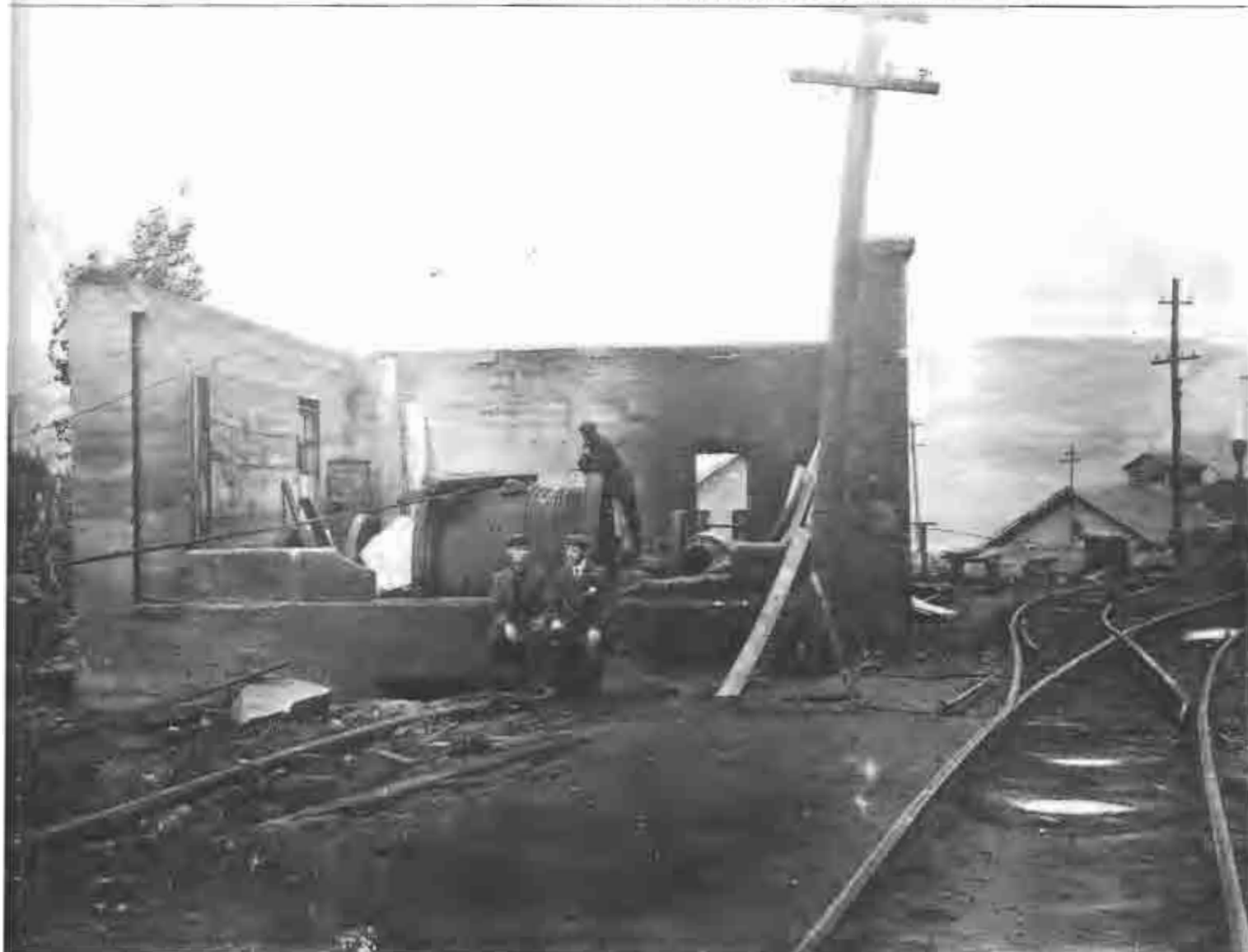
The No. 1 hoist house at the Hillcrest mine was wrecked by the explosion that ripped through the mine on June 19, 1914.
