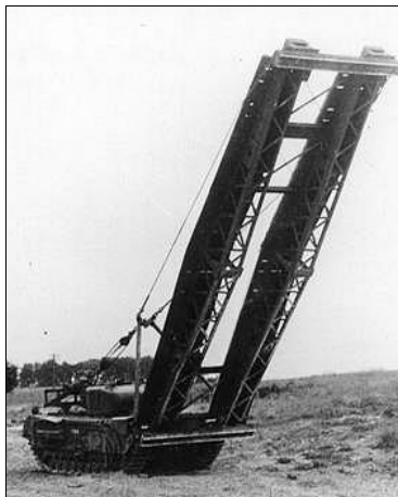
Churchill equipped with small box girder bridge.
