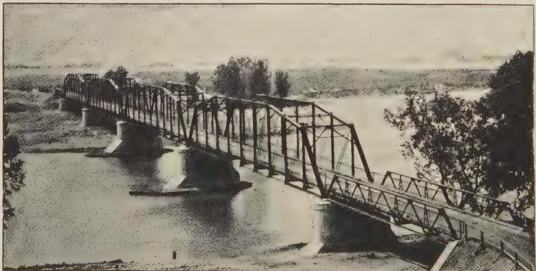
4 Pin Connected Pins 175 Feet Each and 2 Riveted 80 Feet Spans Over Belly River Near Lethbridge.
