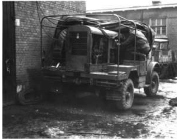
Left: 60-cwt CMP Wrecker - 1940s-1950s. General Motors/Ford 3-ton 4x4, Garwood (later Holmes) twin boom wrecker gear, powered winch. Dr. W.A. Gregg
