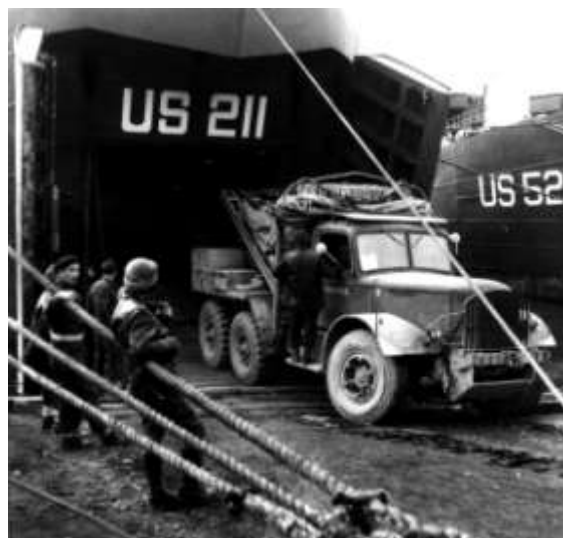
Offloading a heavy RCEME wrecker - Mack 5-ton 6x4 with Garwood 16-ton twin boom wrecker gear and rear mount 20-ton winch - Normandy summer 1944. DND courtesy Dr W.A. Gregg
