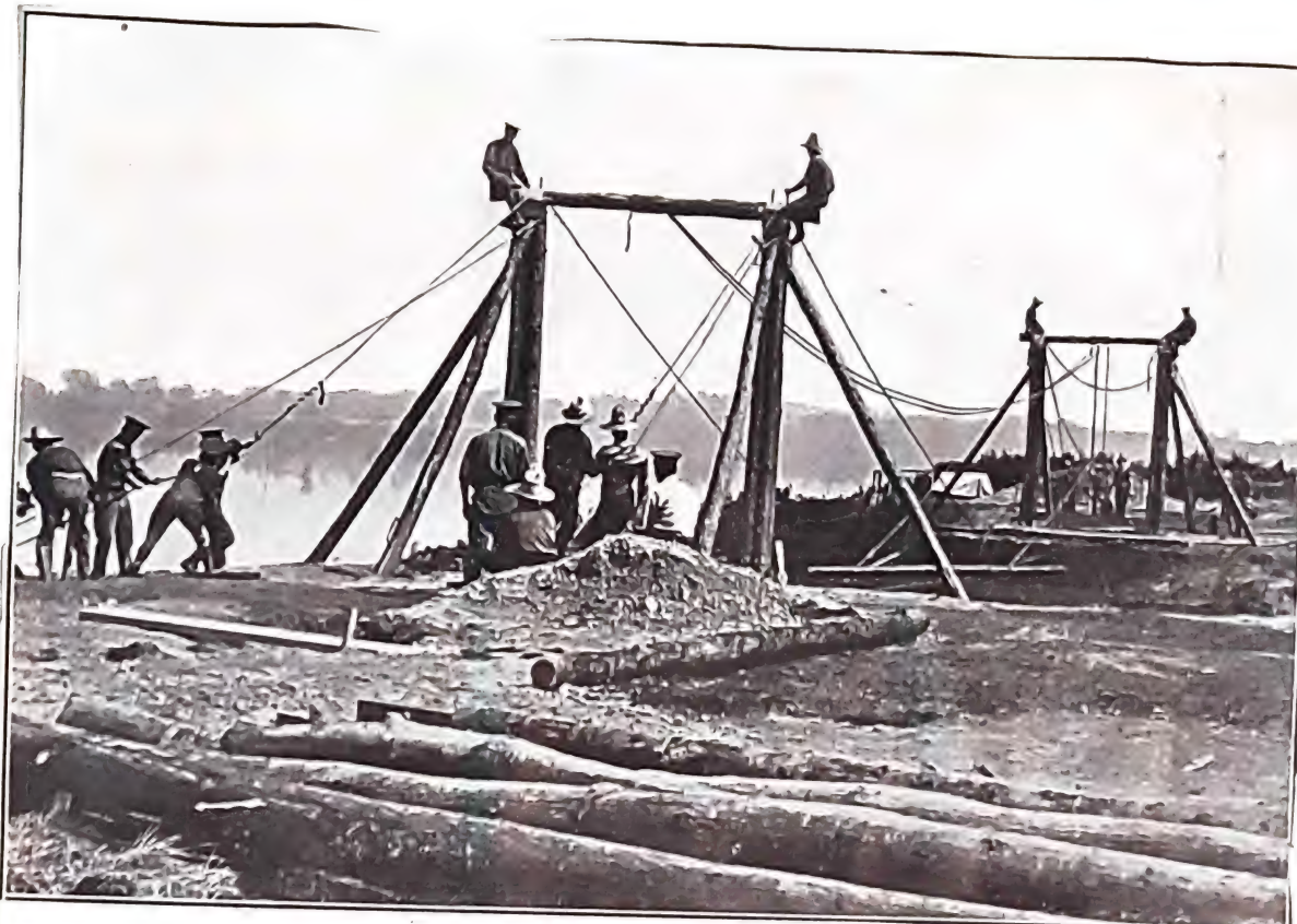
TRAINING CANADIANS FOR THE FIRING LINE. —Building a pontoon bridge over an inlet of the River Ottawa at Rockcliffe Camp.
