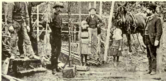
THE SPRING POLE DRILL.
