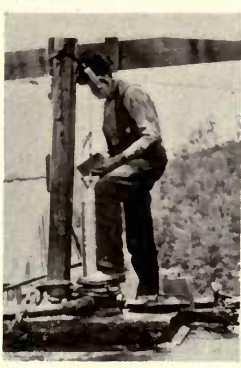
WELL SHOOTER FILLING THE TORPEDO.
