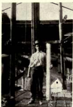
WELL SHOOTER LOWERING THE TORPEDO.
