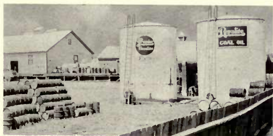
DISTRIBUTING STATION, LETHBRIDGE.
