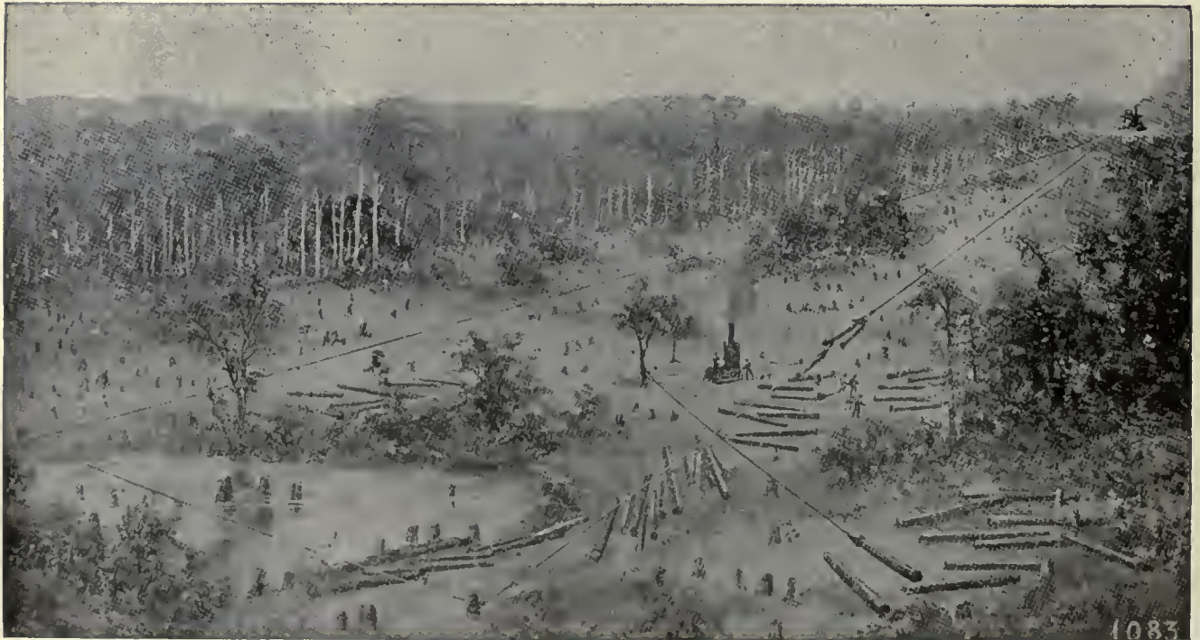
(2). Diagrammatic view of "Ground" Skidding using Baptist cones, vide para 45. (By permission of Messrs. The Lidgerwood Manufacturing Co.)
