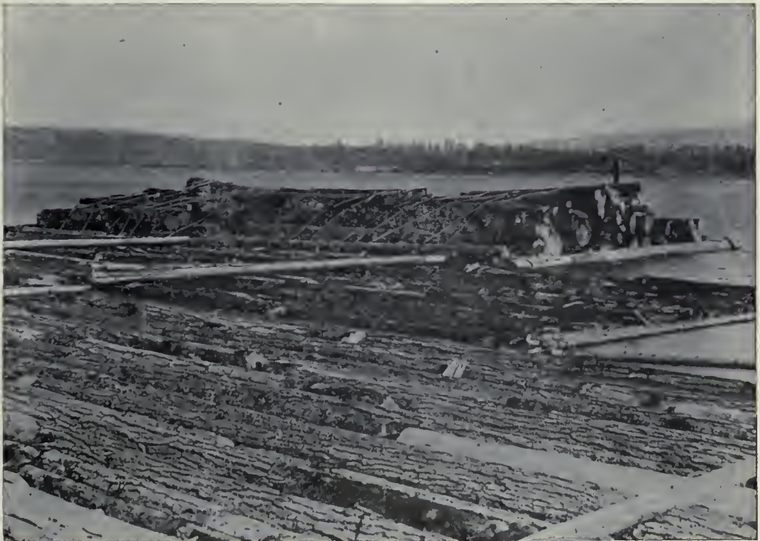
(2). VIEWS OF DAVIS RAFT; 2,000 TONS OF TIMBER.
