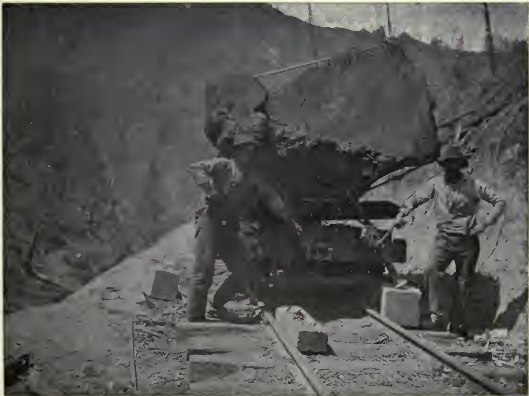
(2). Same as above, near view after the log had been deposited on the car ; note the use of hand jacks to make the log balance properly.—Elk, California.
