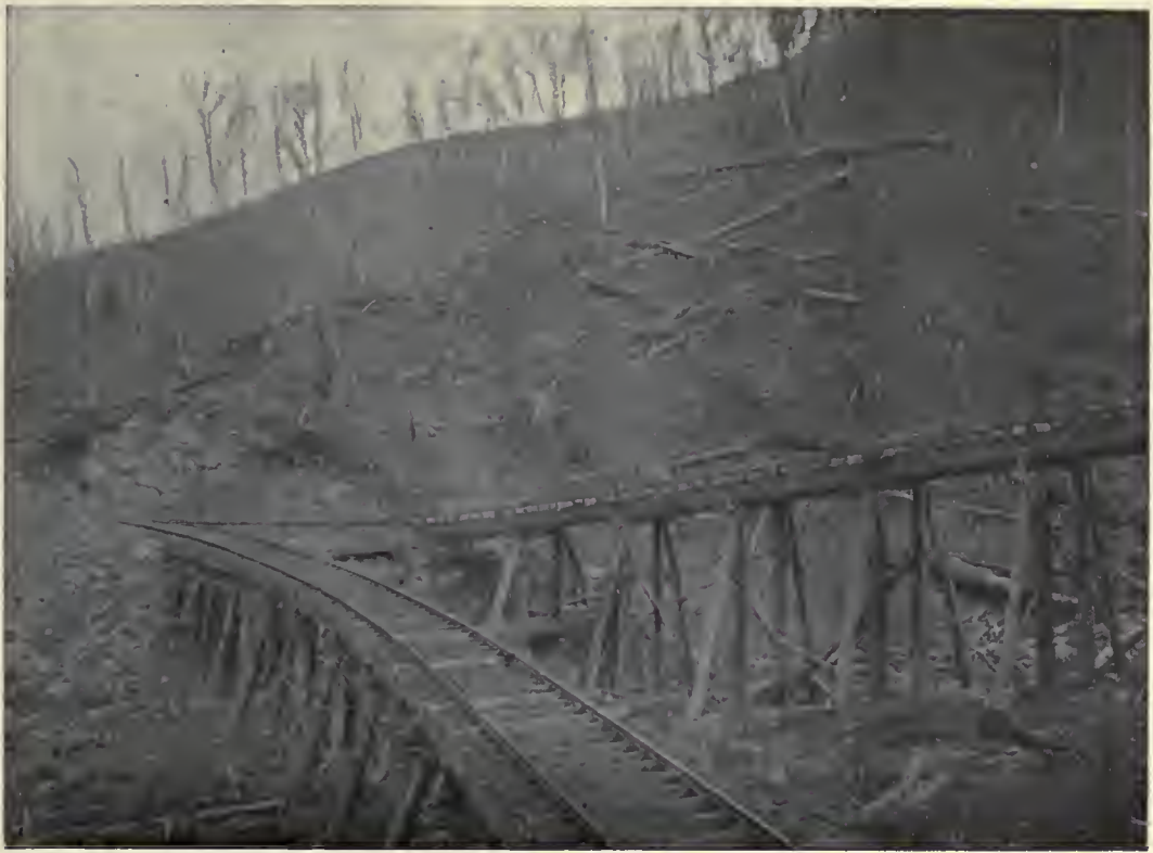
(1). Switch-back and trestles,—Townsend, Tennessee.
