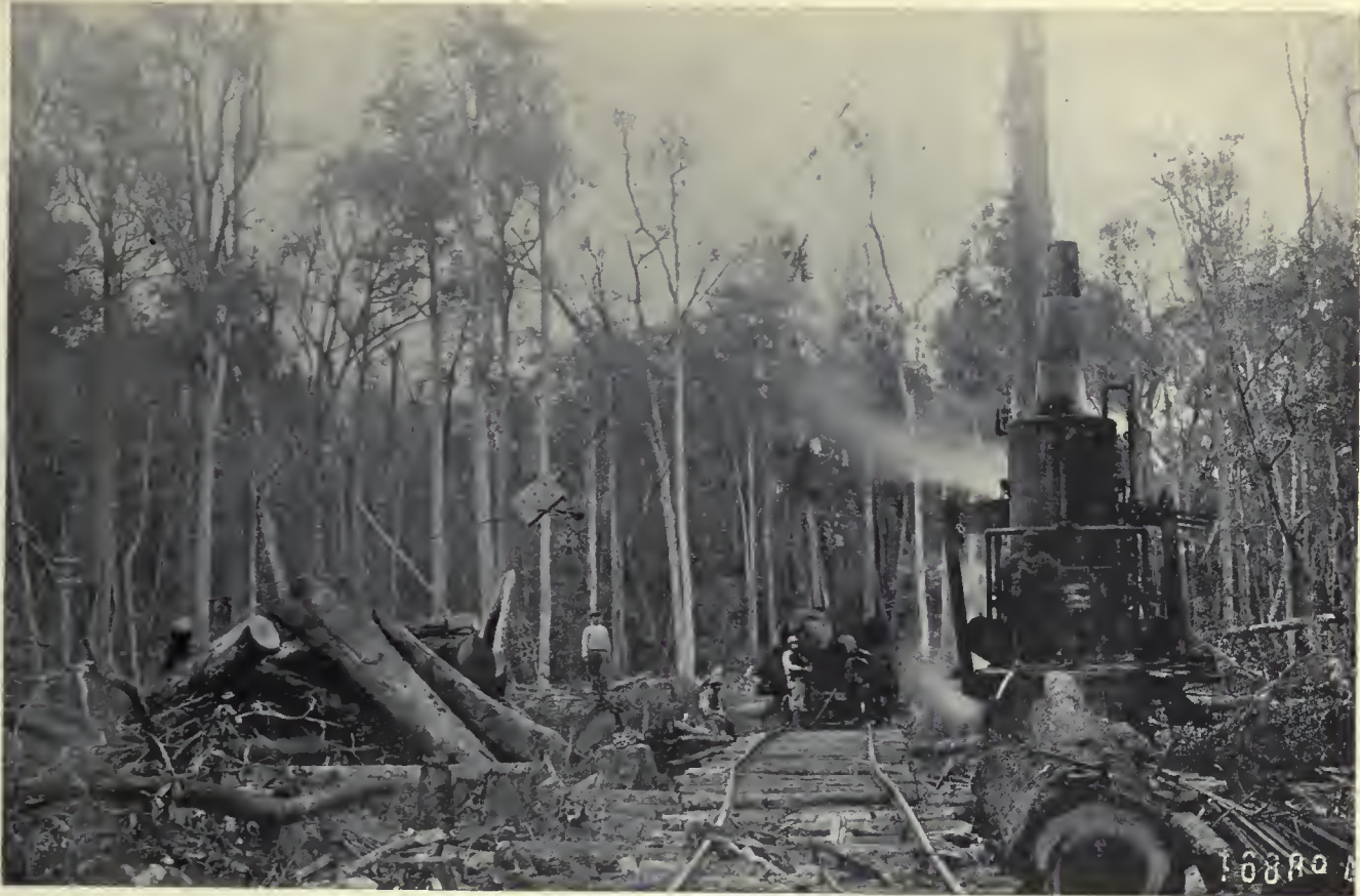
(1). Skidder at work in Cypress Swamp, showing rough character of the spur line,-Ware, Georgia. (U. S. Forest Service Photo).
