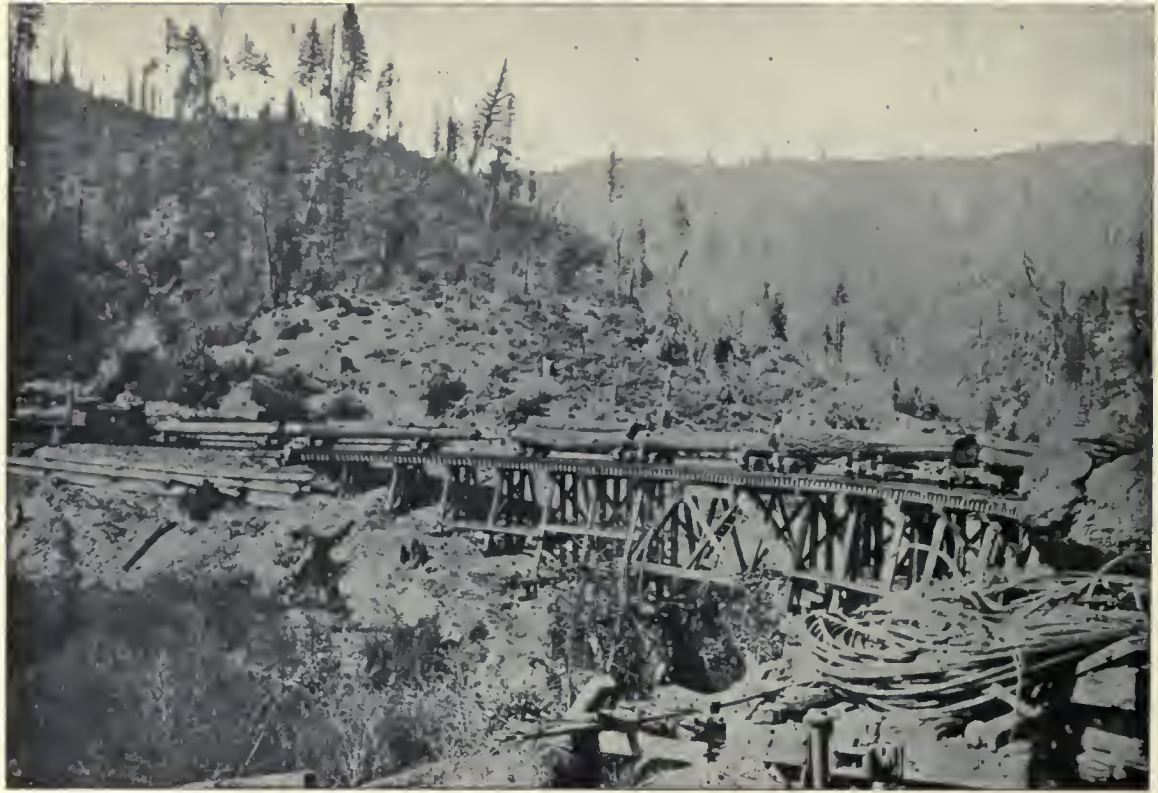
(1) Trestle and log train on 3-foot track, Elk,-California.
