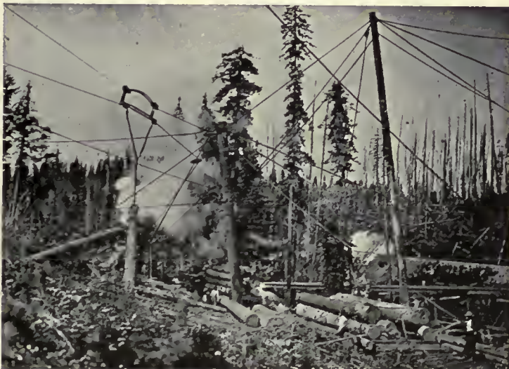
(2). Same as above at railway end of operation ; the smaller of the two spars is used for loading.—Keeler, Idaho.
