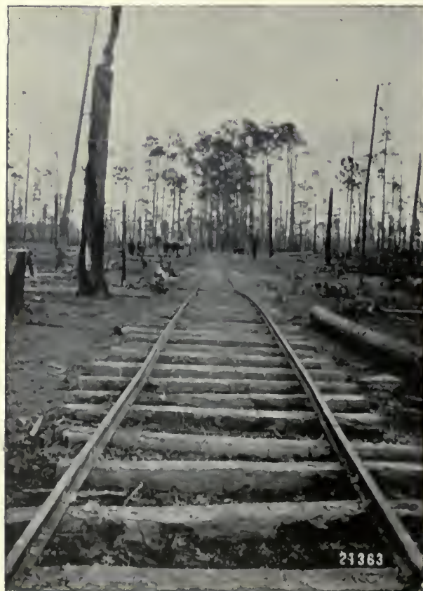
(2) Logging railway in the plains,-Buna, Texas. (U. S. Forest Service photo).
