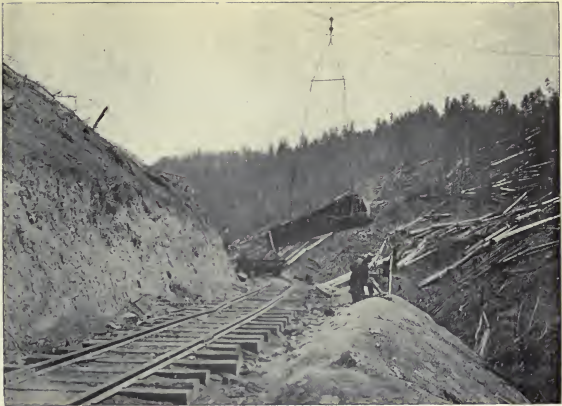
(1). SKY LINE SKIDDING AND LOADING. 8 ton log on 3 feet track ; telephone operator in the foreground.—Elk, California.
