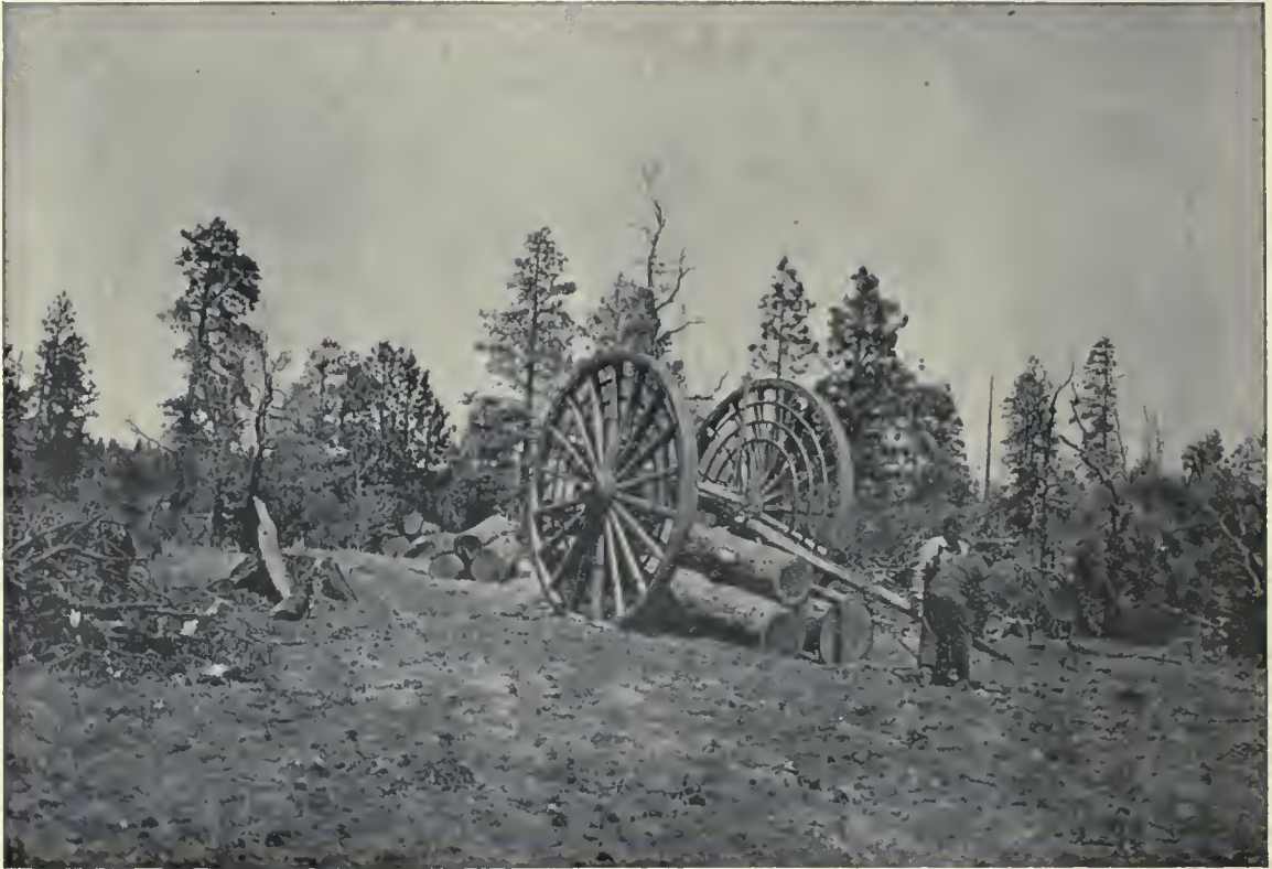
(1). Axle lever being tied to the logs.—Flagstaff, Arizona.
