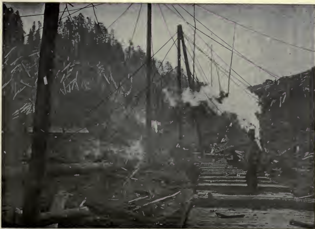
(2). Two-legged Gin Pole, 80 feet long.—Elk, California.
