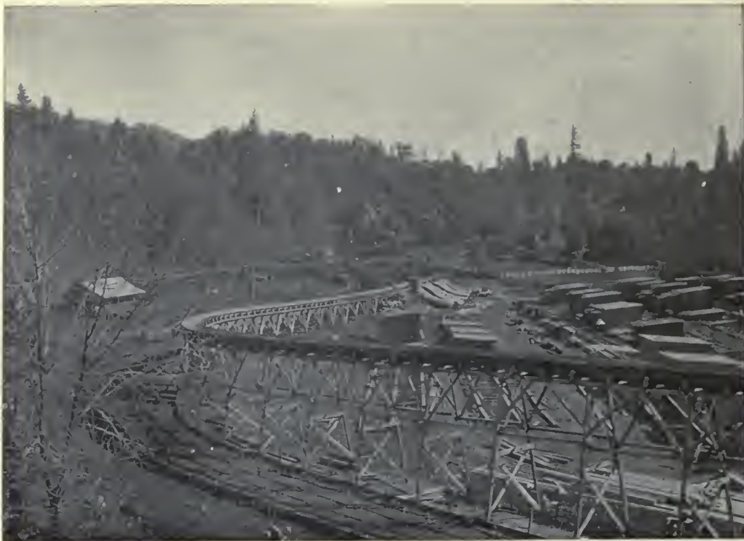
(1). Lower end of a flume bringing sawn timber from Mill to railway.—Lamoine, California.
