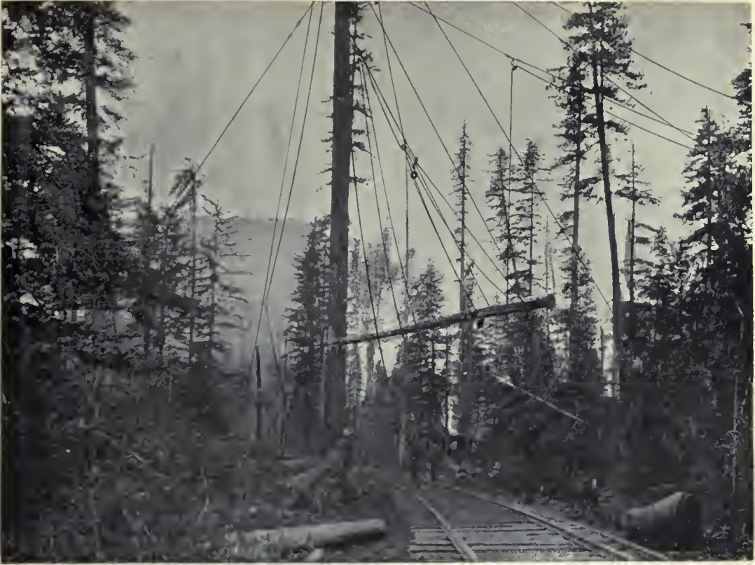
(1). McClean Tree Spar Boom Loader ;— Wind River, Washington.
