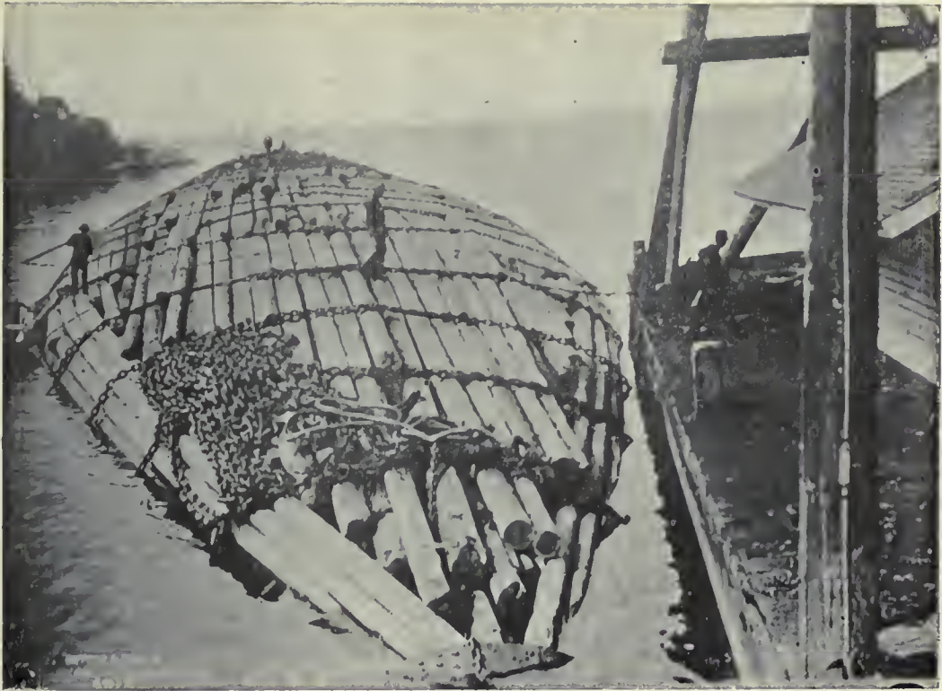
Benson Raft ready for sea, 8000 tons of logs, Length 1,000 ft.; Beam 60 ft.; Height 40 ft., (15 ft. above and 25 ft. below water) Photo by Gifford and Prentiss, Portland, Oregon.
