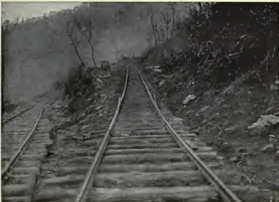
(2). Slip-Joints on log grades.—Townsend, Tennessee.
