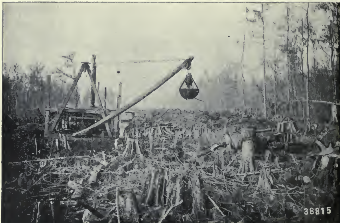
(1). Dredging Canal in Cypress Swamp, Terre Bonne, Louisiana. (U. S. Forest Service Photo.)
