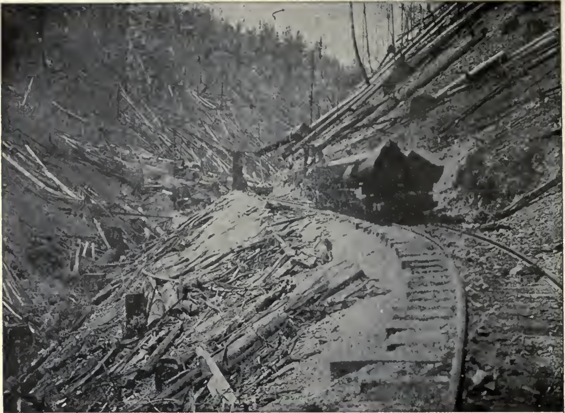
(1). Sky Line Skidding and loading in a single operation, (see also plate XXXII) ; one car fully loaded ; log suspended over the track (3 ft.) waiting for another car to be brought forward ;—Elk, California.
