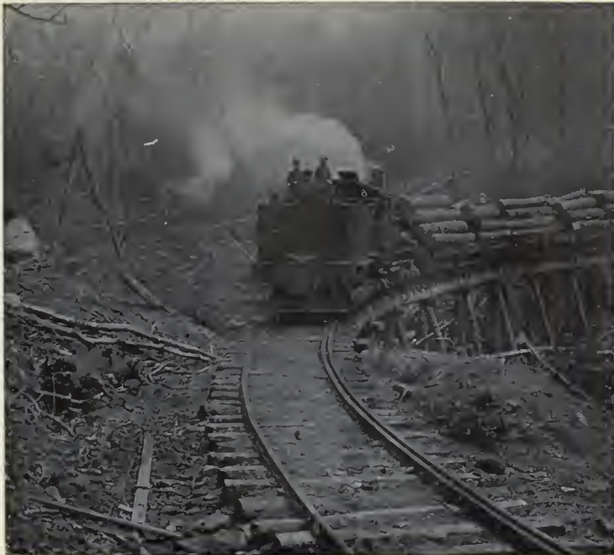
(1). Trestle and log train.—Townsend, Tennessee.
