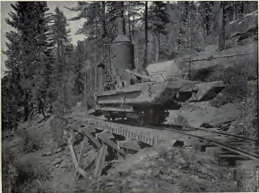
(2). Transporting skidder by rail on 3-foot track.—Lamoine, California.
