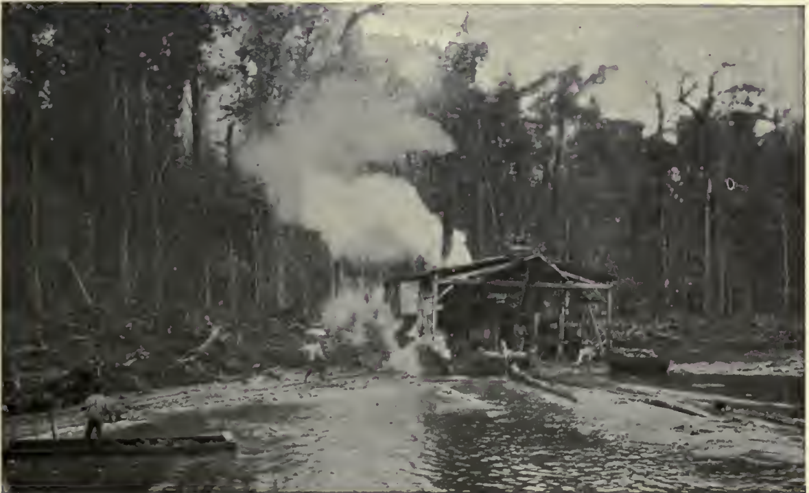
(2). Pull-boat at work in Cypress Swamp.—Donner, Louisiana.
