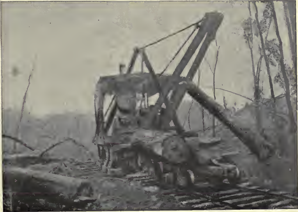
(1). Old Type of Lidgerwood Swinging Boom Loader mounted on a timber platform jacked up over the railway track.—Sardis, Mississippi.
