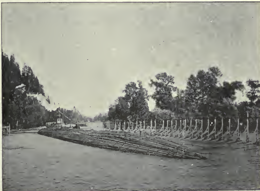
(2). Benson Raft completed ; cradle removed.
