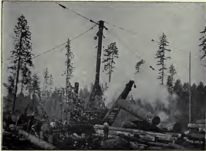
(1) Lidgerwood latest type of Combined Skidder and Loader. (see also plate XXVI); -Kapowsin, Washington.
