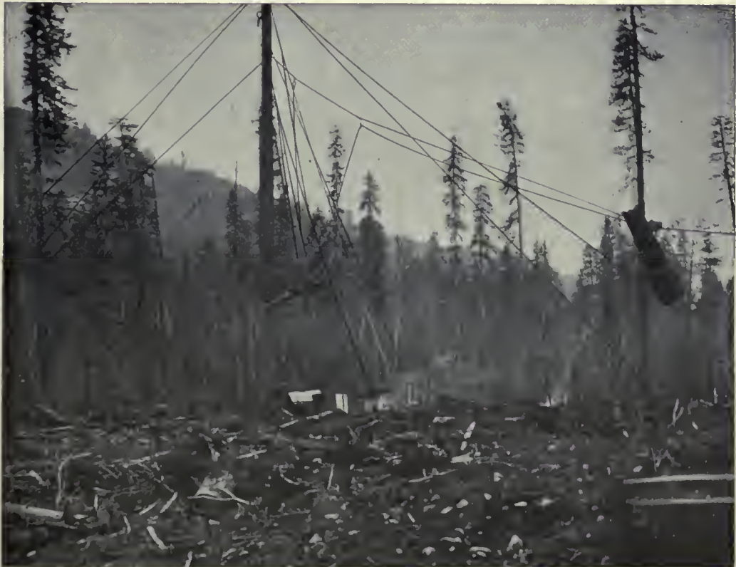
(2). Same as above ; counterpoise log running on Guy Line shown to the left. Wind River, Washington.
