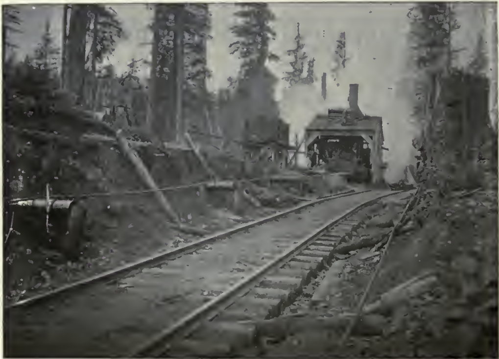
(2). Hoisting engine at top of Incline.—Arlington, Washington.
