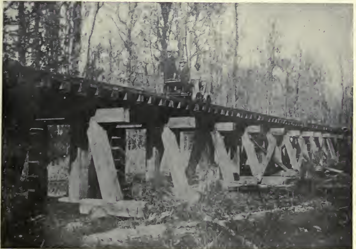
(2). Trestle across swamp,-New Bern, North Carolina.
