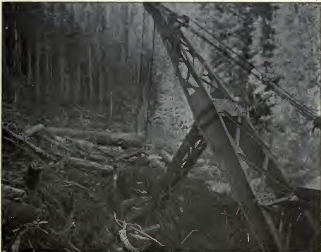
(2). Track being cleared by Shovel.—Elk River, Idaho.
