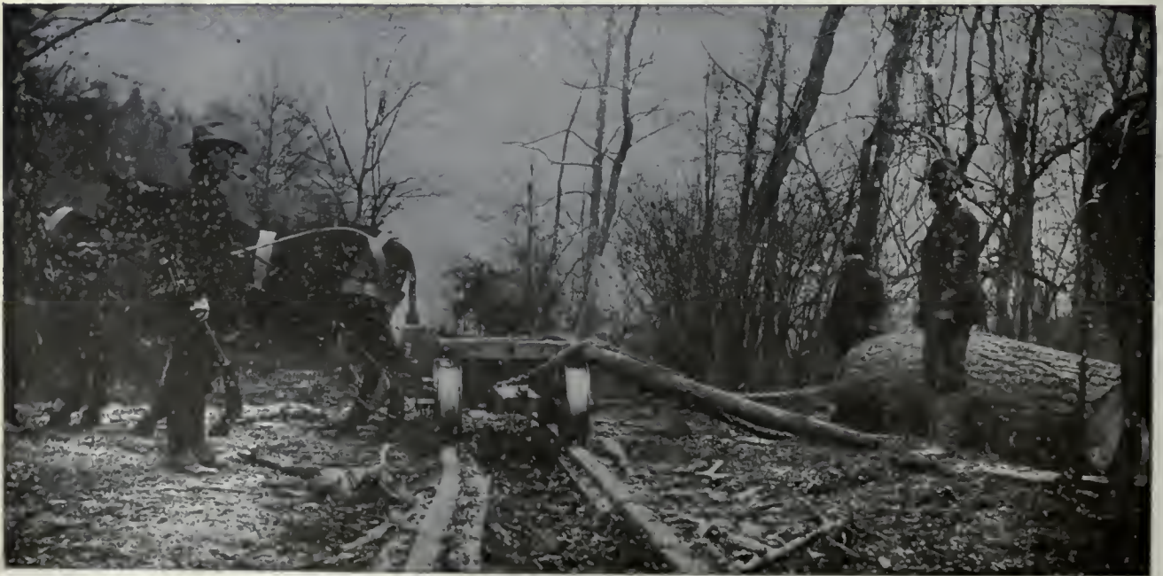
(2). Wood Rail Tramway ; log being loaded by parbuckling, vide para 63.—Overton, Tennessee. (U. S. Forest Service Photo)
