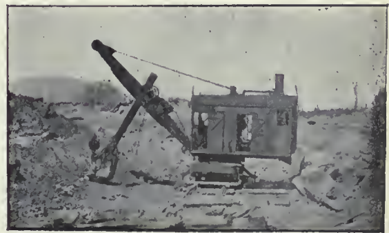
(3). Shovel mounted on railway track.
