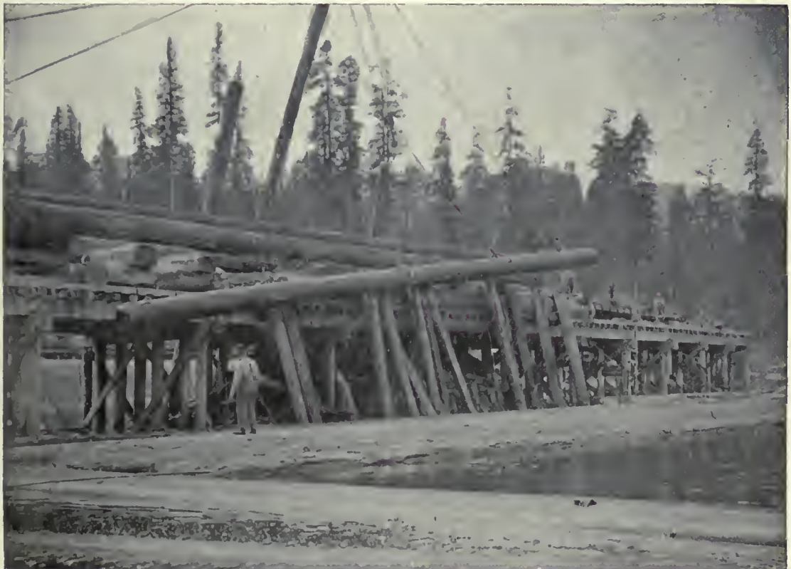
(2). Gin Pole Loading from water.—Lake Cowichan, B. C.
