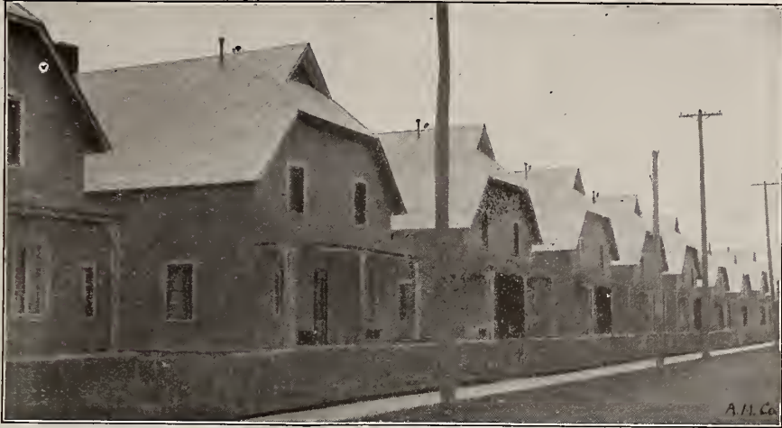
Montreal Cotton Co. Operatives' Houses at Valleyfield, P.Q., roofed with ASBESTOSLATE
