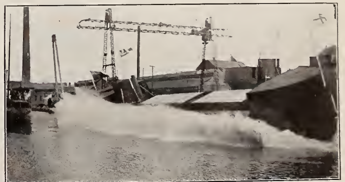
Launching a Lighter at Polson's Iron Works, Toronto
