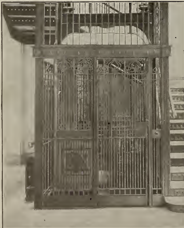
ELEVATOR ENCLOSURES AND STAIRS ONTARIO PARLIAMENT BUILDINGS.
