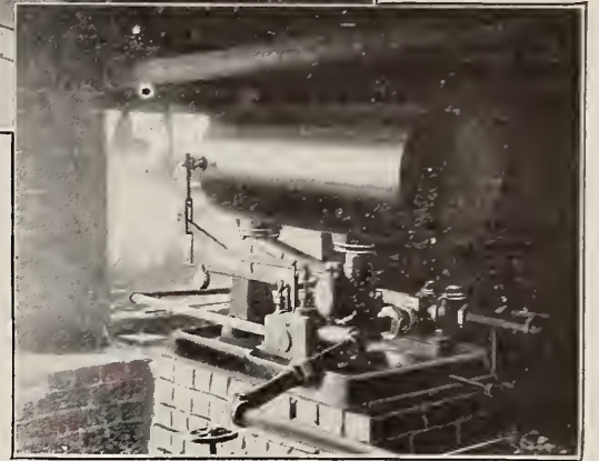
Upper illustration shows a Detroit Return Trap draining an office heating system. Lower illustration shows Detroit Return Trap draining steam coils of a Lumber Dry Kiln at Fox Bros., Windsor, Ontario.
