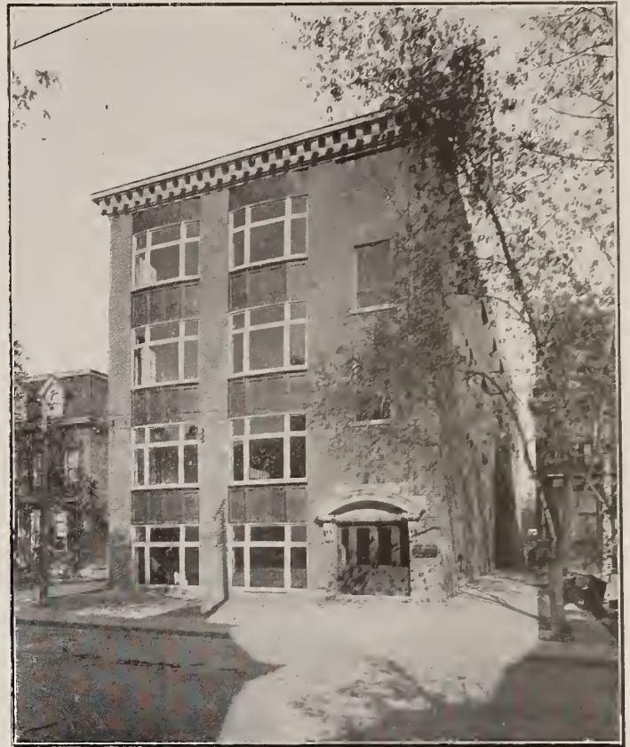
W. E. Dillon Sheet Metal Works just completed in Toronto
