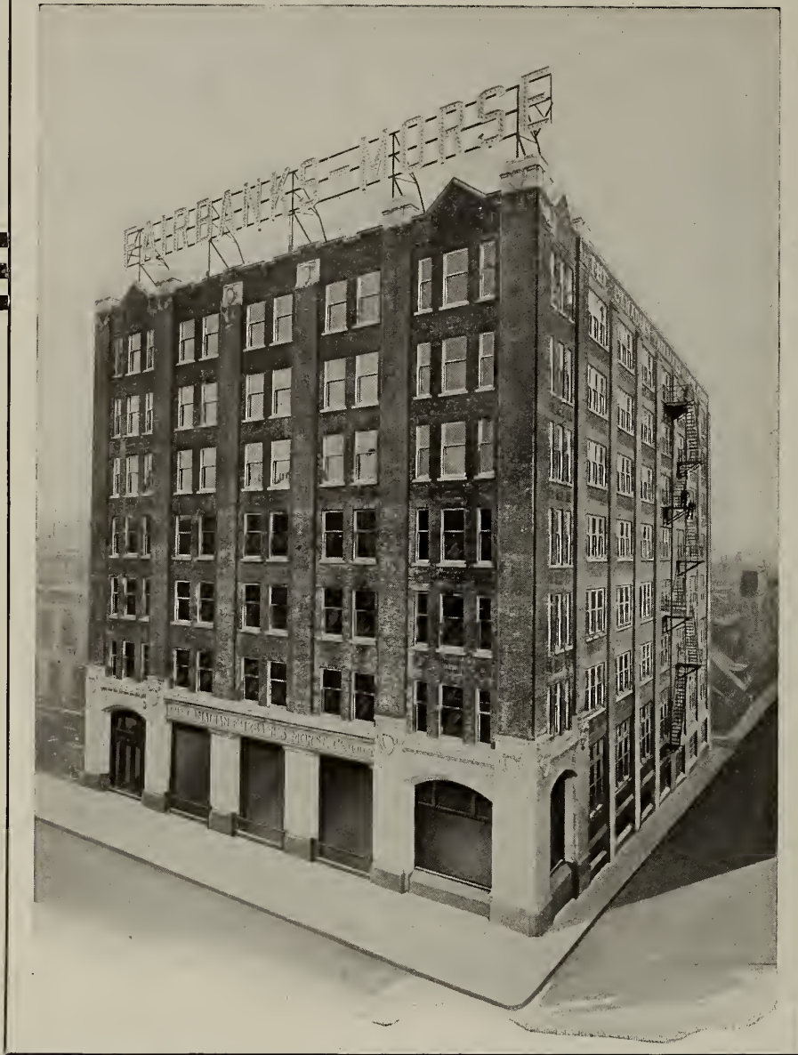
New Montreal Offices and Warehouses of Canadian Fairbanks-Morse Co., Limited Designed and Constructed Under Our Supervision.
