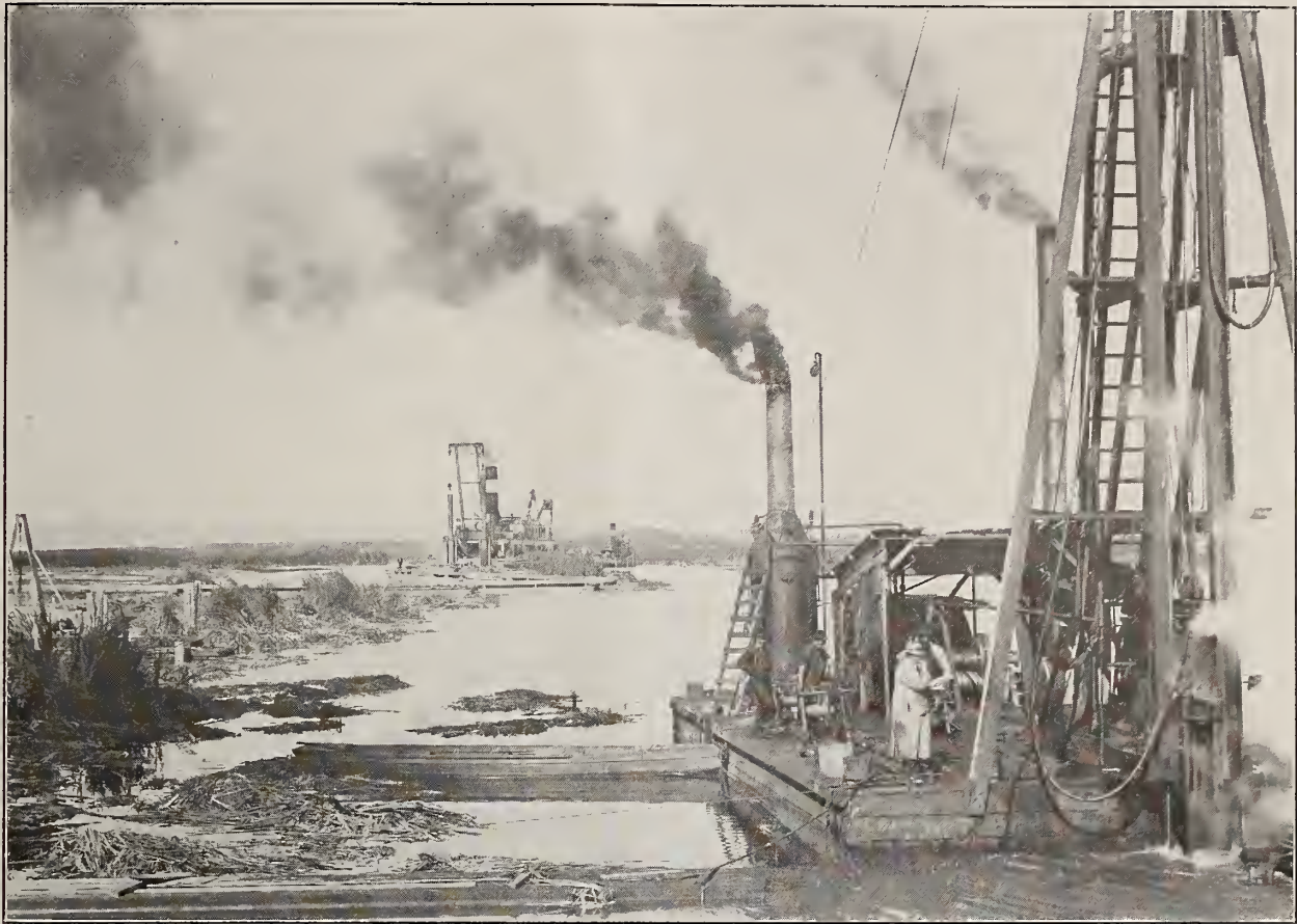
CONSTRUCTING A SHIP CHANNEL IN THE TORONTO HARBOR INDUSTRIAL DISTRICT
