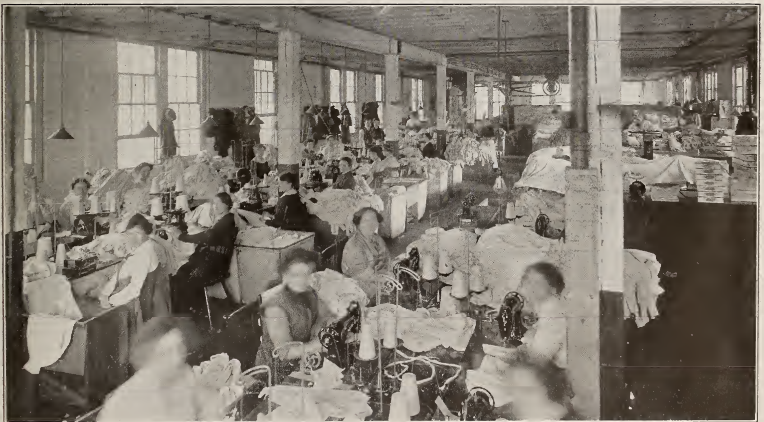
Mercury Mills Limited, Hamilton, Ont., Manufacturing Underwear and Hosiery for the War.
