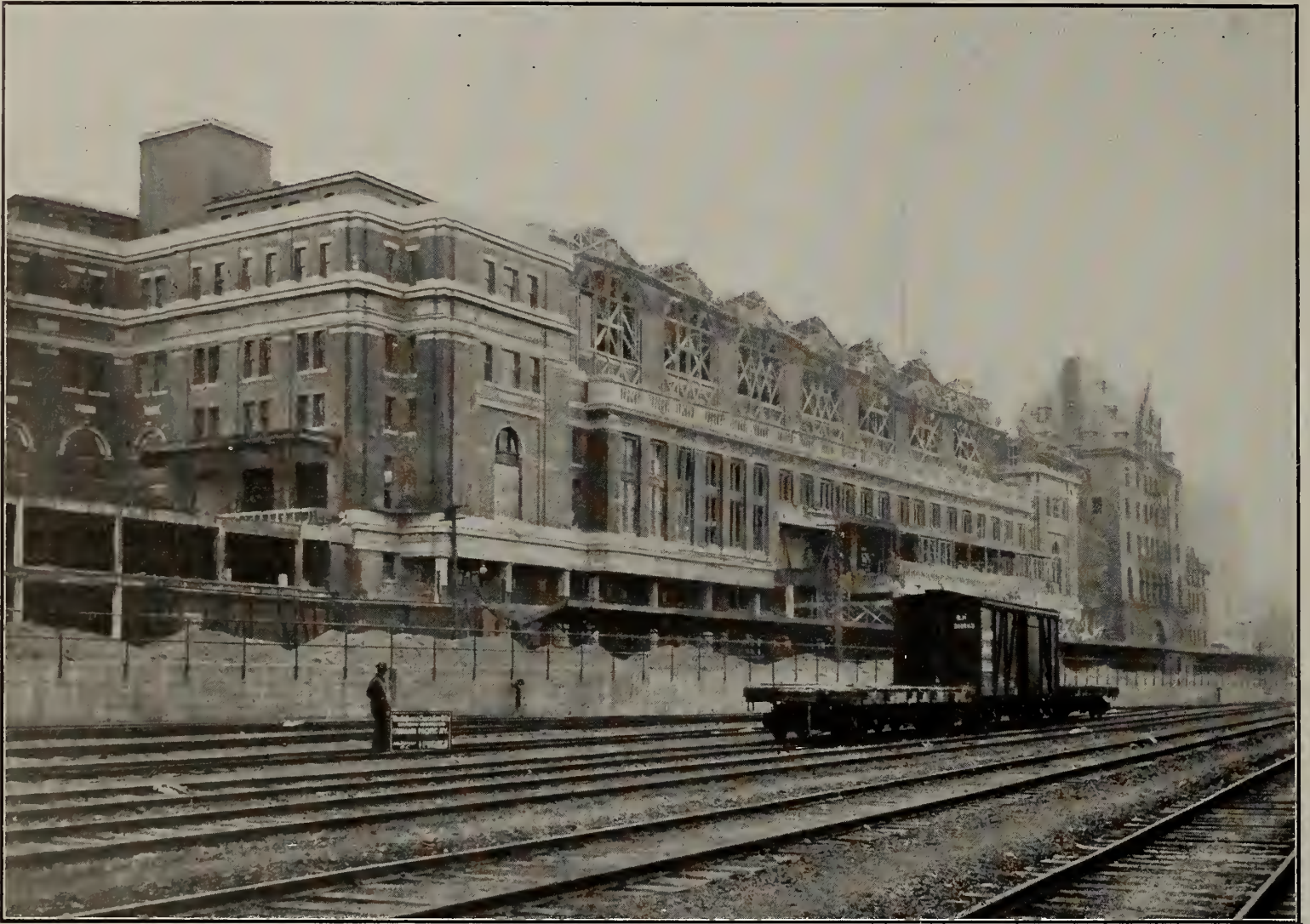
Elevation Track Side of the New Canadian Pacific Railway Passenger Station, Vancouver, B.C.
