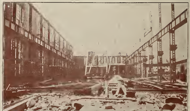
Canadian Locomotive Company's Plant at Kingston
