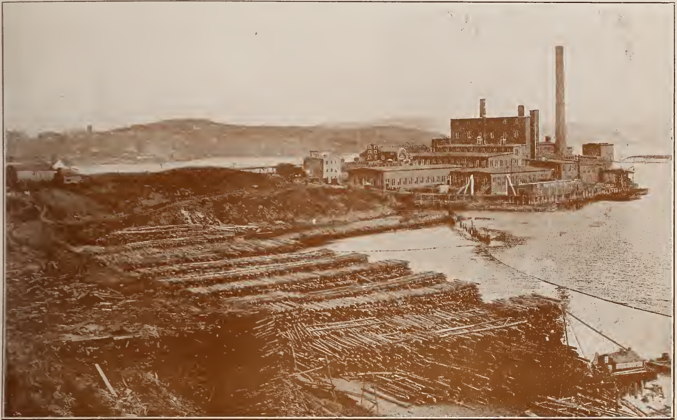
The Partington Pulp Company's Plant at St. John, N.B.
