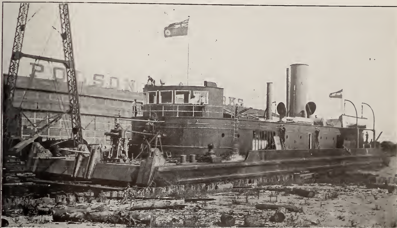
The "Port Nelson," the Steel Hydraulic Dredge built by the Polson Iron Works, Limited, for the Dominion Government in 100 days. It is now on its way to Hudson Bay, where it will be used to deepen the terminal port of the Hudson Bay Railway, by which Western Canada hopes to ship grain to Europe.
