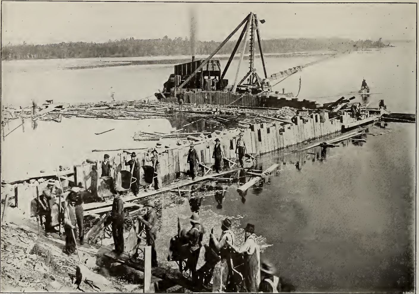
Building Cofferdam in Connection with the C.N.R. Causeway Across Rainy River
