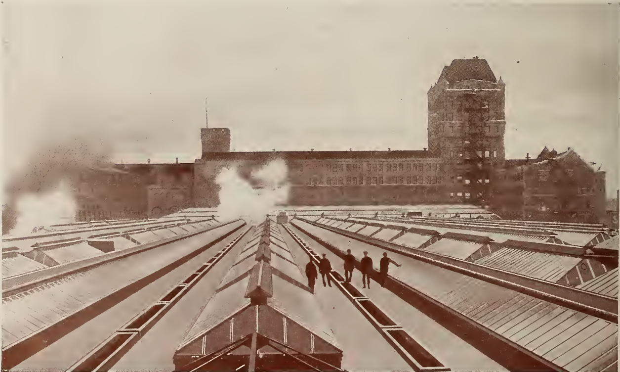
Showing the Skylights on the new C.P.R. Train Sheds at the Windsor St. Station, Montreal. This is one of the Largest Sky-light Contracts ever let in America and was awarded to a Canadian Firm—The Metal Shingle & Siding Co. of Montreal. Over 100,000 Feet of 3-inch Ribbed Wired Glass, 30-Tons of 16-oz. Cold Rolled Copper and over 100-Tons of 16-gauge Lead Coated Bars were used on this Contract.
