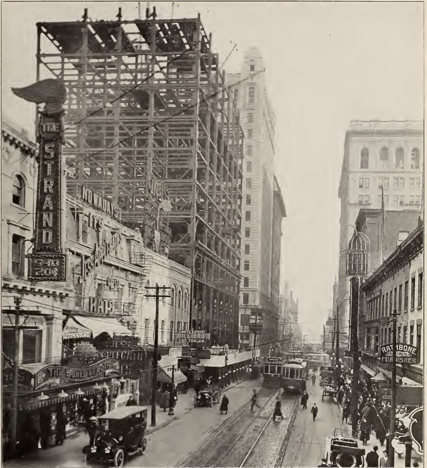
This photograph shows the highest buildings in the British Empire. They are situated in a group on the corners of King and Yonge Streets, Toronto. On the left, in course of construction, is the new skyscraper of the Royal Bank, which will be 250 feet high, containing 20 storeys. The white building behind the Royal Bank building has just been completed by the Canadian Pacific Railway. It is 238 feet high, containing 15 storeys. Next in line is the Traders Bank Building, which now belongs to the Royal Bank. It is 15 storeys, or 200 feet high. Opposite these "three sisters" is the new building of the Dominion Bank, 183 feet high and containing 9 storeys.
