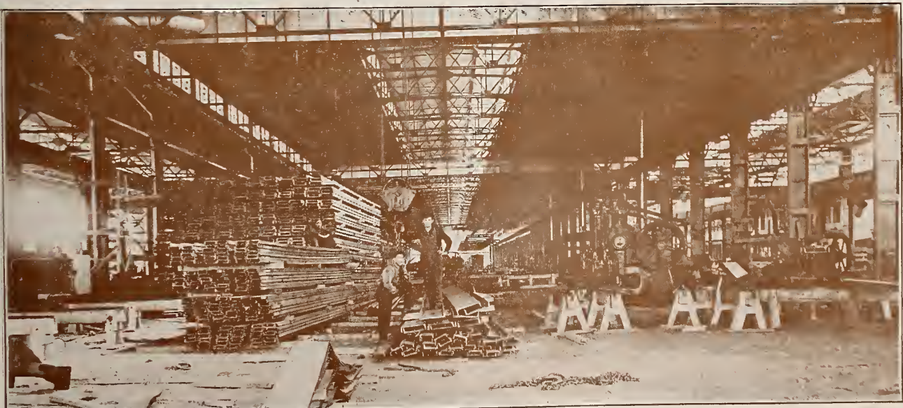
View of Punching, Shearing and Steel Erecting Bays of Eastern Car Co., New Glasgow, N.S.
