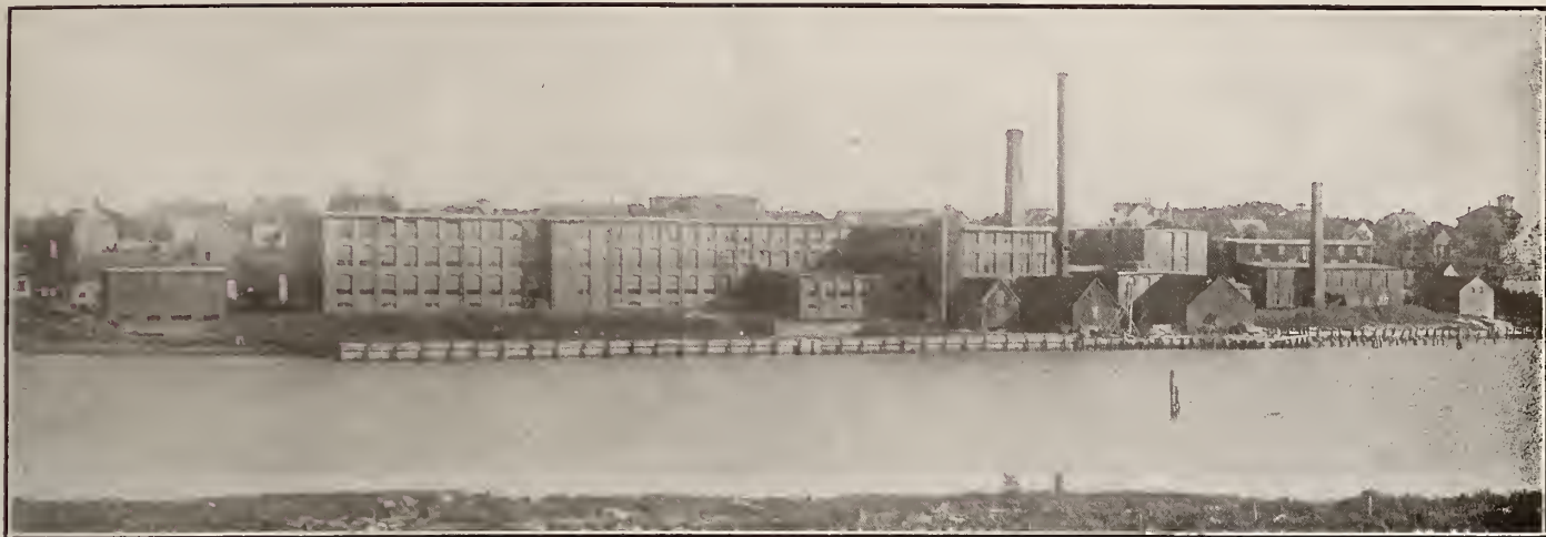
A NEW MILL ADDITION AND STOREHOUSE COSMOS COTTON COMPANY, YARMOUTH, NOVA SCOTIA
