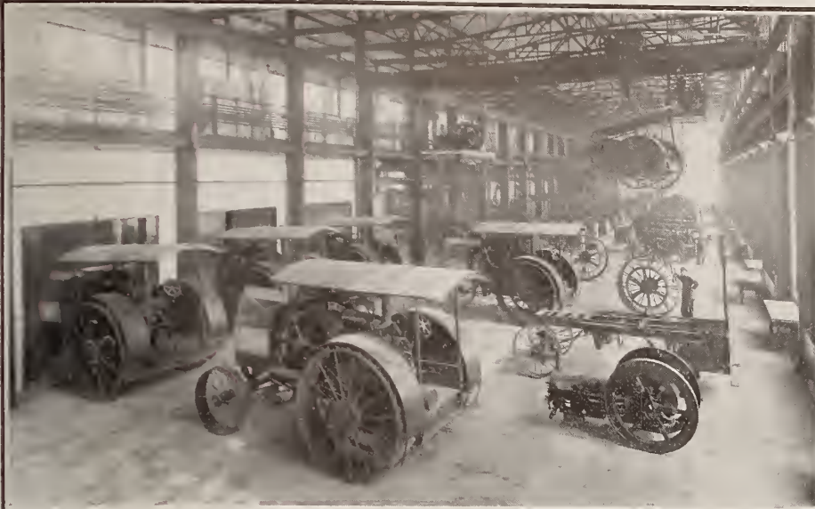
Traction Engine Shop-- CANADIAN FAIRBANKS MORSE CO., LIMITED Toronto, Ontario
