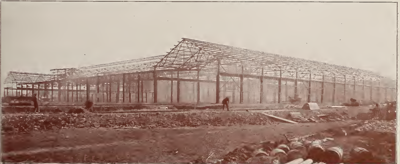
Steel Work Completed for Factory
