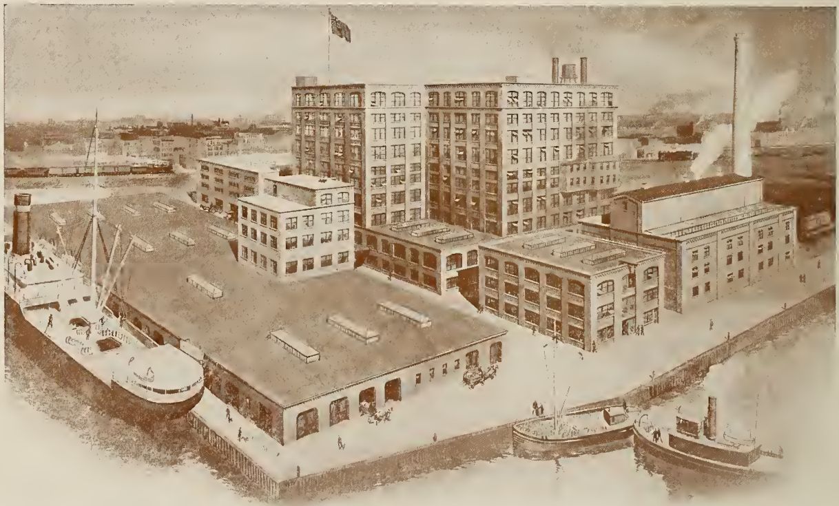
Atlantic Sugar Refinery, St. John, as it will appear when complete
