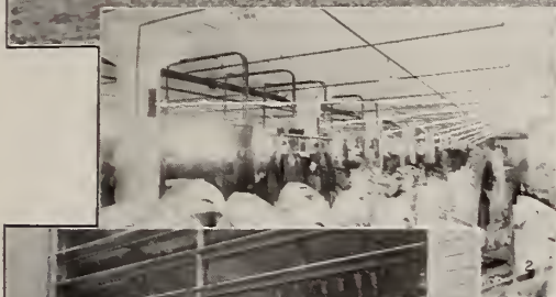
1 Air Supply Ducts leading from Fans to columns. 2 Columns from which air is delivered. 3 One of two fan units looking through fresh air inlet of Fan House.
