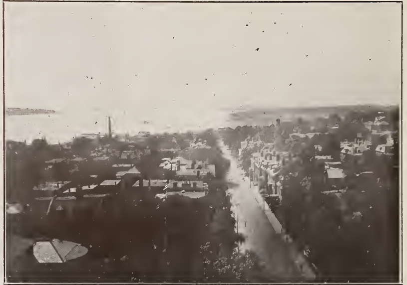
A Residential Street in Halifax
