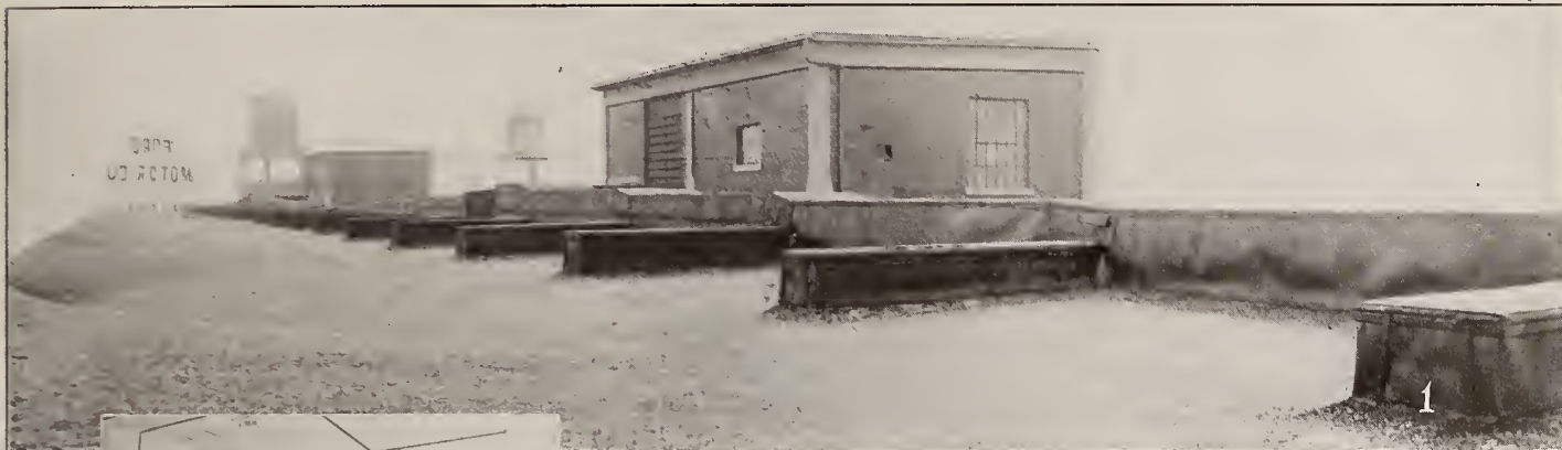
1 Air Supply Ducts leading from Fans to columns. 2 Columns from which air is delivered. 3 One of two fan units looking through fresh air inlet of Fan House.
