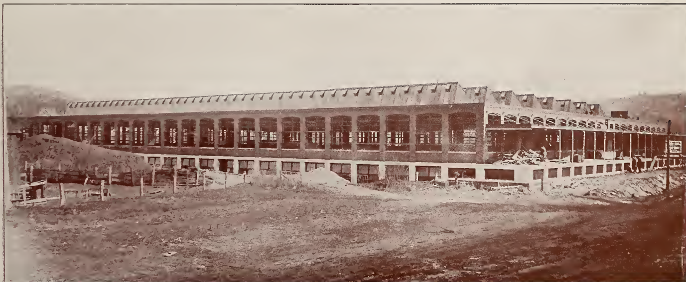
Saw-Tooth Windows Give Good Light (Courtesy of Factory).
