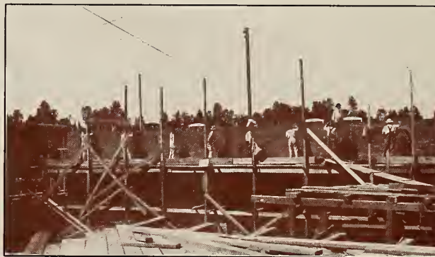
Adjustable Scaffold Showing Men Working on Both Sides at Once
