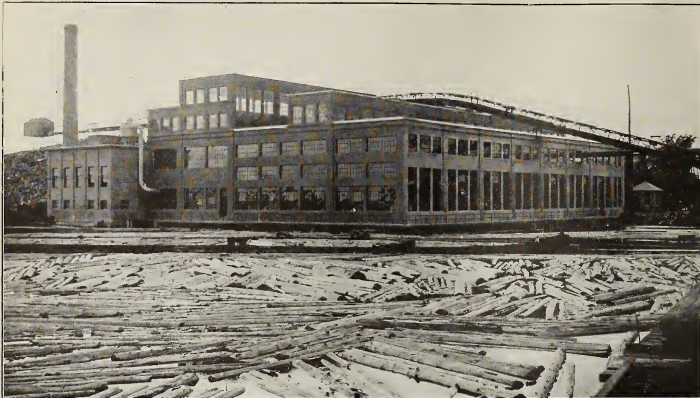
The $750,000 Pulp Mill, Pulp Wood Conveyor and Pulp Storage Yard now being built in Hull, Quebec, by the E. B. Eddy Company, Limited
