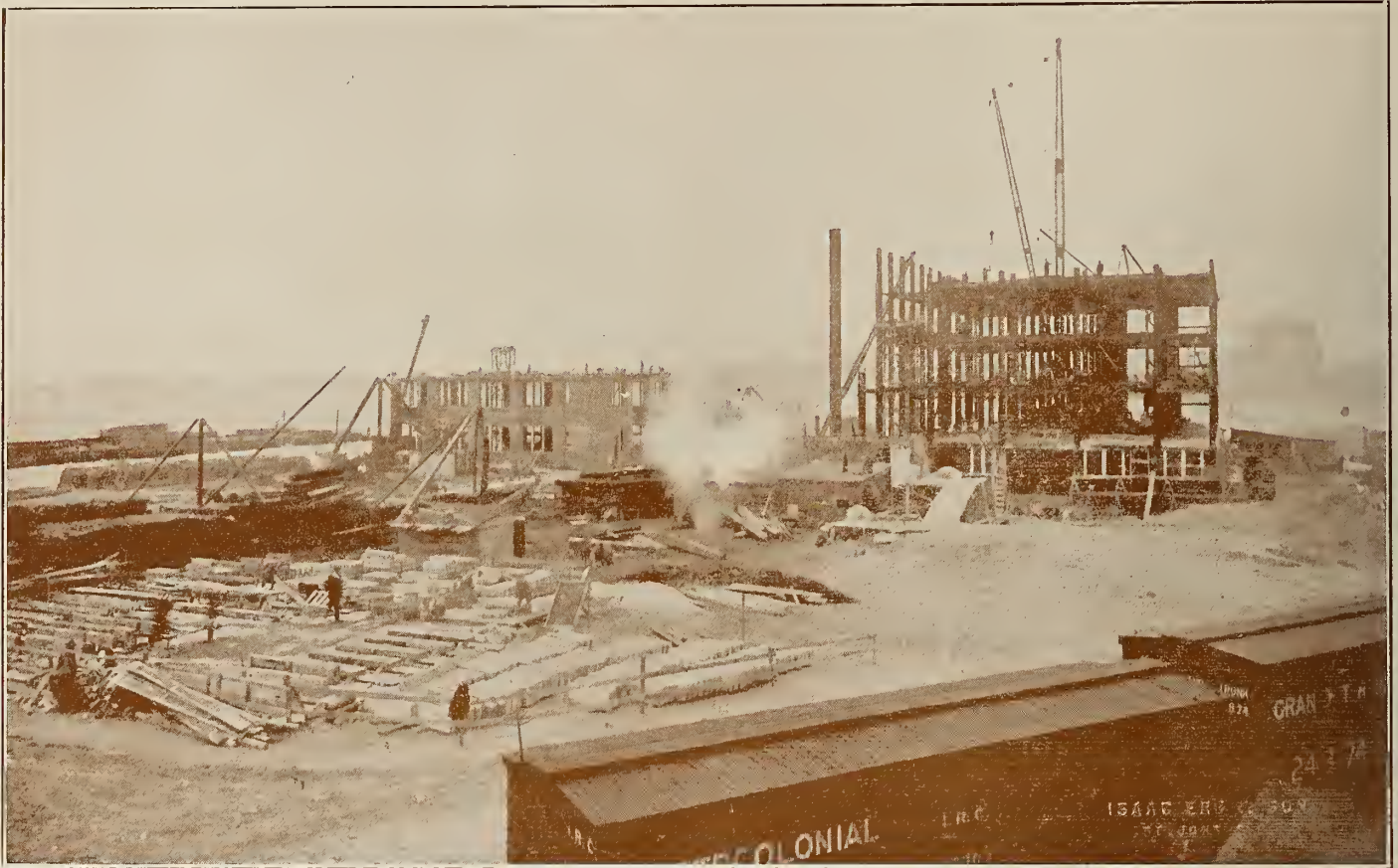
Great Plant of the Atlantic Sugar Refinery, under construction at St. John, N.B.
