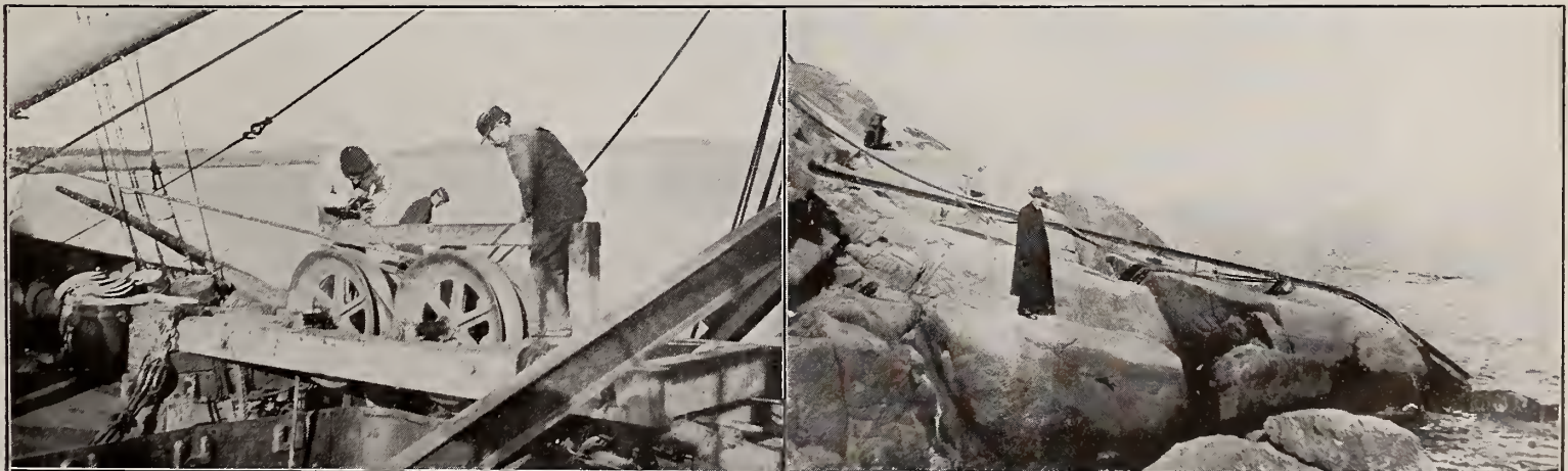
Cable Laying Gear Used at Louisburg, Yarmouth and Negro Head
