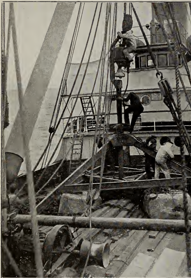
Erecting Tripod on Deck
