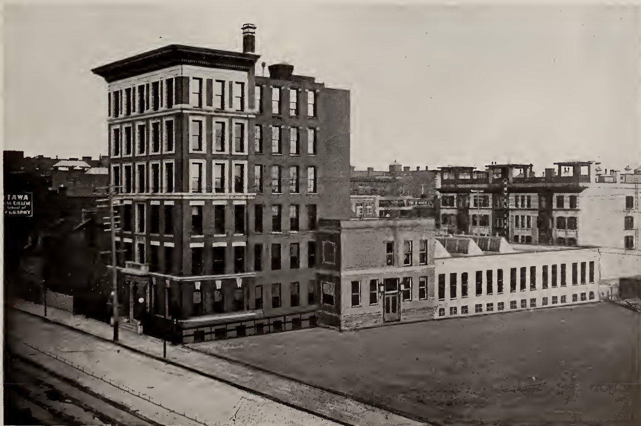
HEAD OFFICE AND WORKS, OTTAWA.
