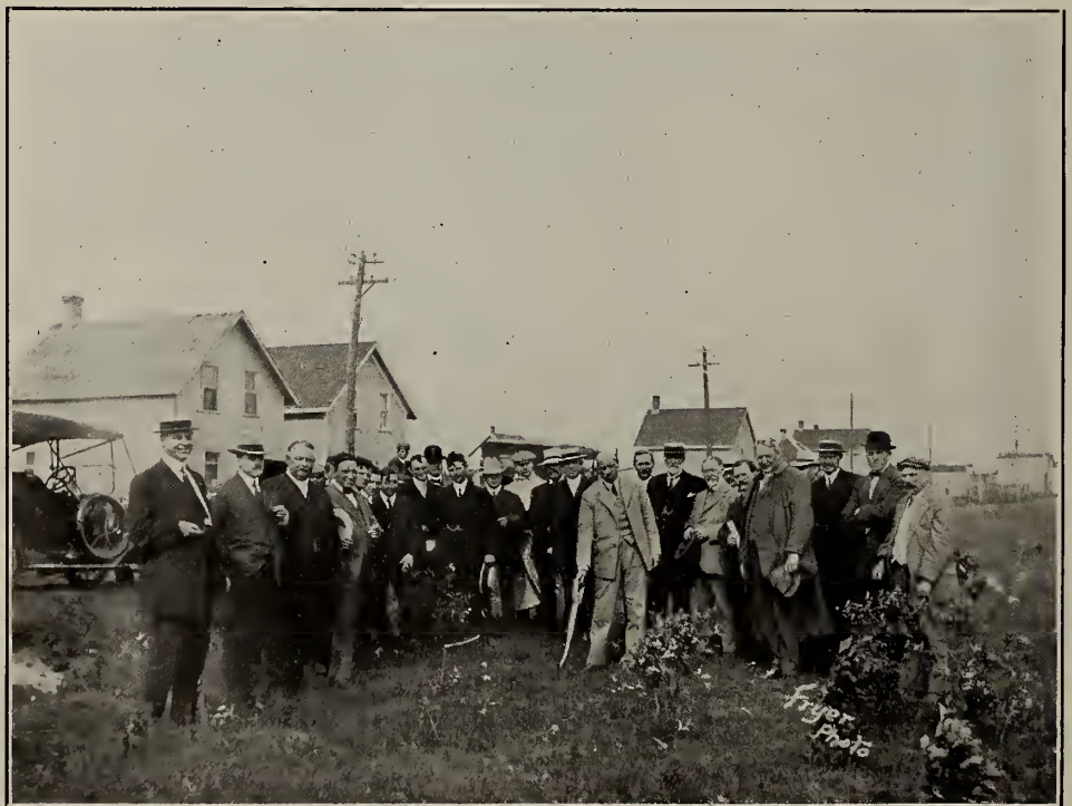
TURNING THE FIRST SOD FOR THE NEW $1,500,000 PLANT OF THE CANADIAN CAR & FOUNDRY COMPANY AT FORT WILLIAM.—This interesting ceremony took place recently in the presence of the Mayor and civic officials of Fort William and others. It was performed by Mr. D'Arcy Scott, of Ottawa, Chairman of the Board of Railway Commissioners, who is seen (shovel in hand) in the above picture. Included among those on his left are Mr. Hansard, Solicitor for the G. T. P., Winnipeg; Mr. Mills, Member of the Board of Railway Commissioners; F. Litchfield, General Superintendent of the C. C. & F. Co., Limited; ex-Mayor S. C. Young, and H. A. K. Drury, of the Board of Railway Commissioners. On Mr. Scott's right are W. W. Butler, Vice-President of the Canadian Car & Foundry Company, Limited; Mr. Lanorgan, Traffic Manager of the C. P. R., Winnipeg; R. O. Shaw, Construction Superintendent of the C. C. & F. Co., Limited; Mr. Bond, Solicitor for the C.P.R., Winnipeg; Mr. Dewey, Traffic Manager of the G. T. P. at Winnipeg; the Mayor of Fort William, and Mr. J. E. Walsh, Traffic Manager of the Canadian Manufacturers' Association.
