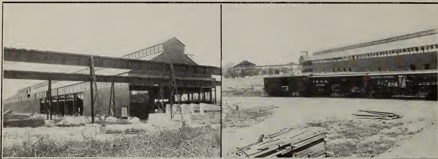
Views of the Steel Company of Canada's great plant in Hamilton, where additions costing $1,600,000 are still under construction. 250 extra men will be employed.
