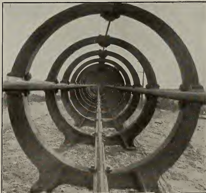
Four Tracks are laid on the Inside of the Railway, one at the Bottom to support the Car, one on each side to keep it Upright, and a Conductor Rail on Top.
