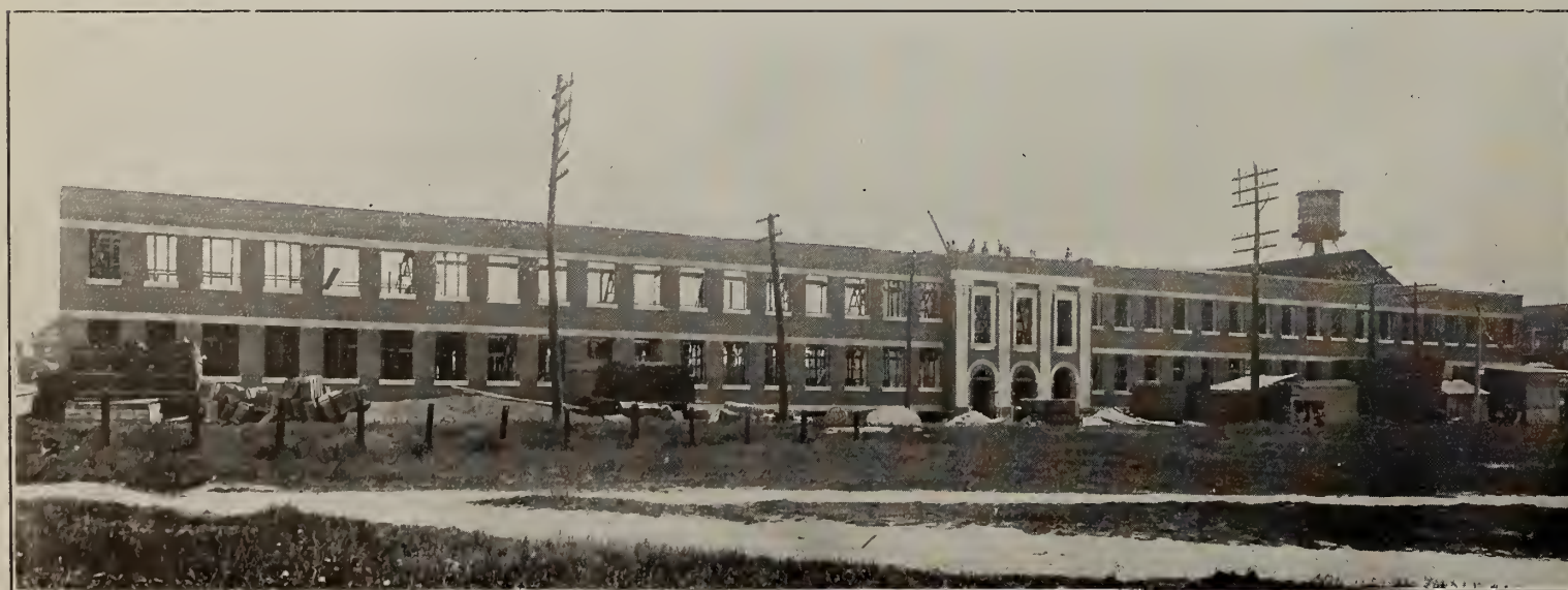
The $300,000 factory of Rolph and Clark, Limited, now being built in Toronto A good example of long, low construction.
