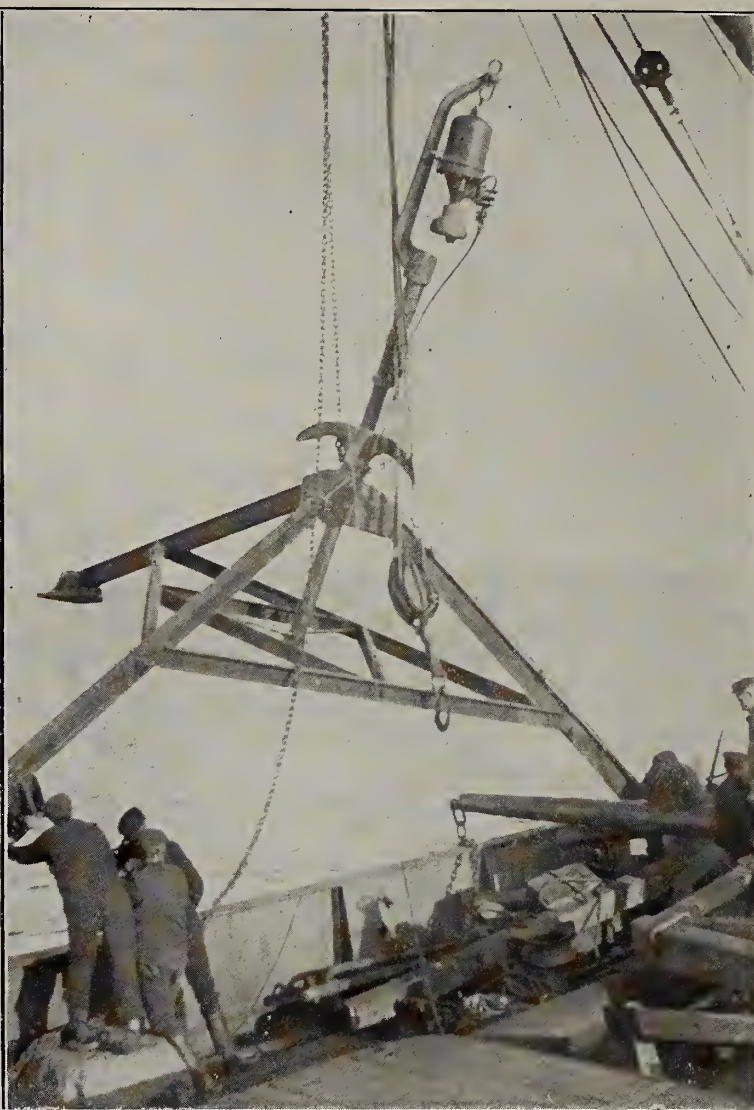
Lowering a Tripod into Position Beneath the Water
