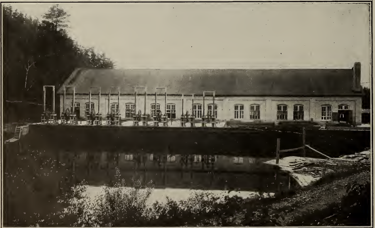
Kenora Power House which generates power for factories.
