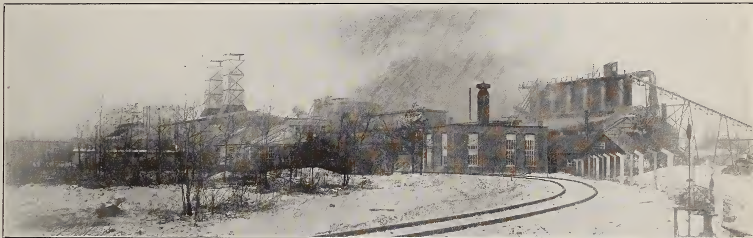
Plant of the American Cyanamid Company at Niagara Falls. The Company are building a $500,000 addition, which will employ 300 extra people and increase the output by 100 per cent.
