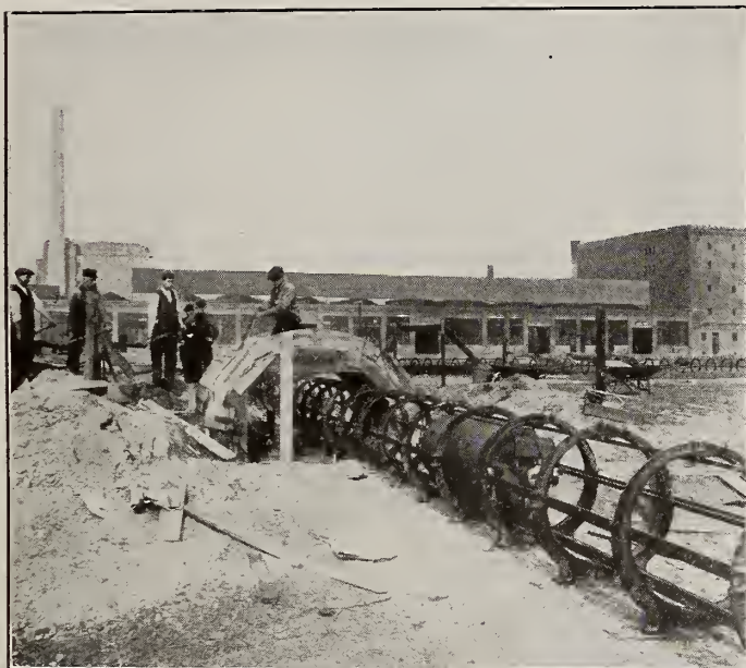
A Demonstration of the New Automatic Railway Tunnel System. It Comprises a Tunnel and Track Nearly One-third of a Mile Long and Begins and Ends in the Station in the Background. Car in Position on the Track.
