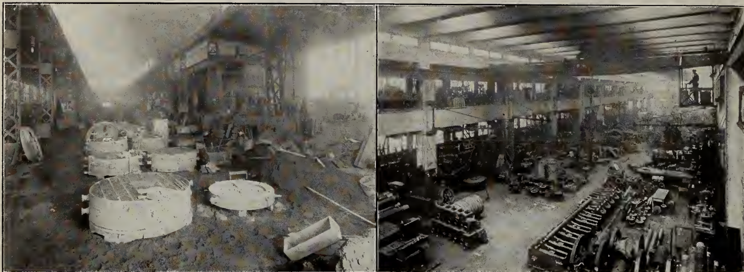
Views of the interior of the $250,000 addition which the Canadian Fairbanks Morse Co., Ltd., are building in Toronto This brings their investment up to $1,000,000.
