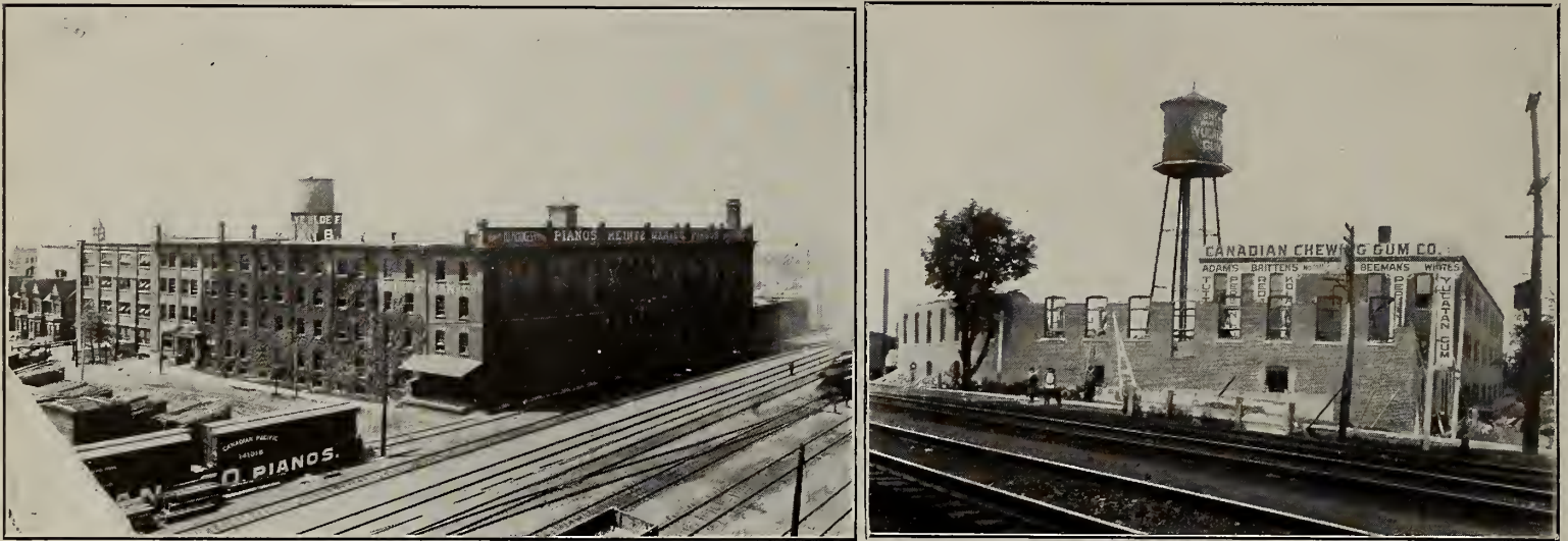
Plant of Heintzman & Co., Toronto, on the left and of the Canadian Chewing Gum Co., Toronto, to which additions are being made
