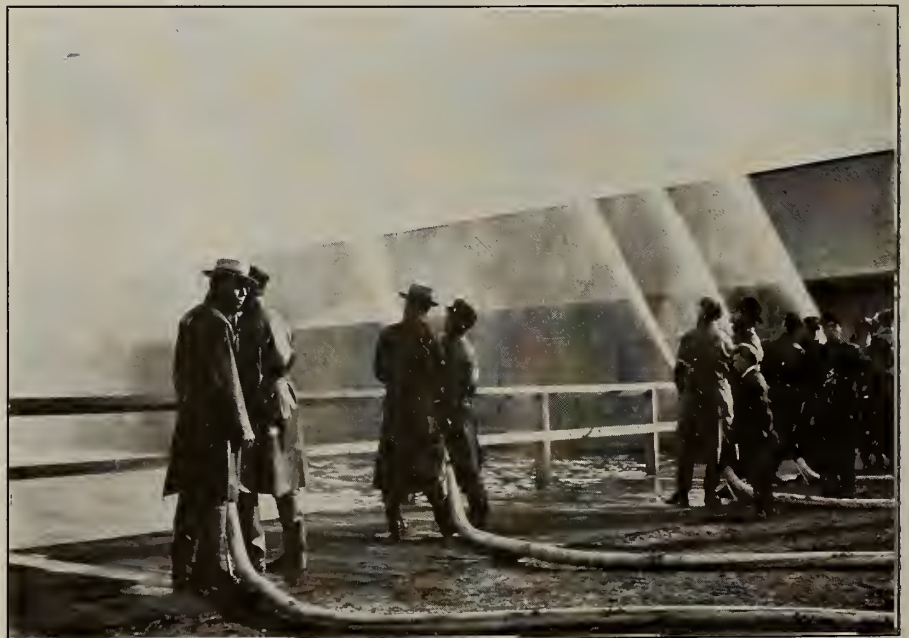
The hose can do little to fight fire in a tall building
