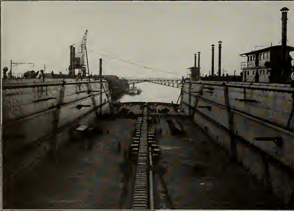
Interior of the Montreal Dry Dock
