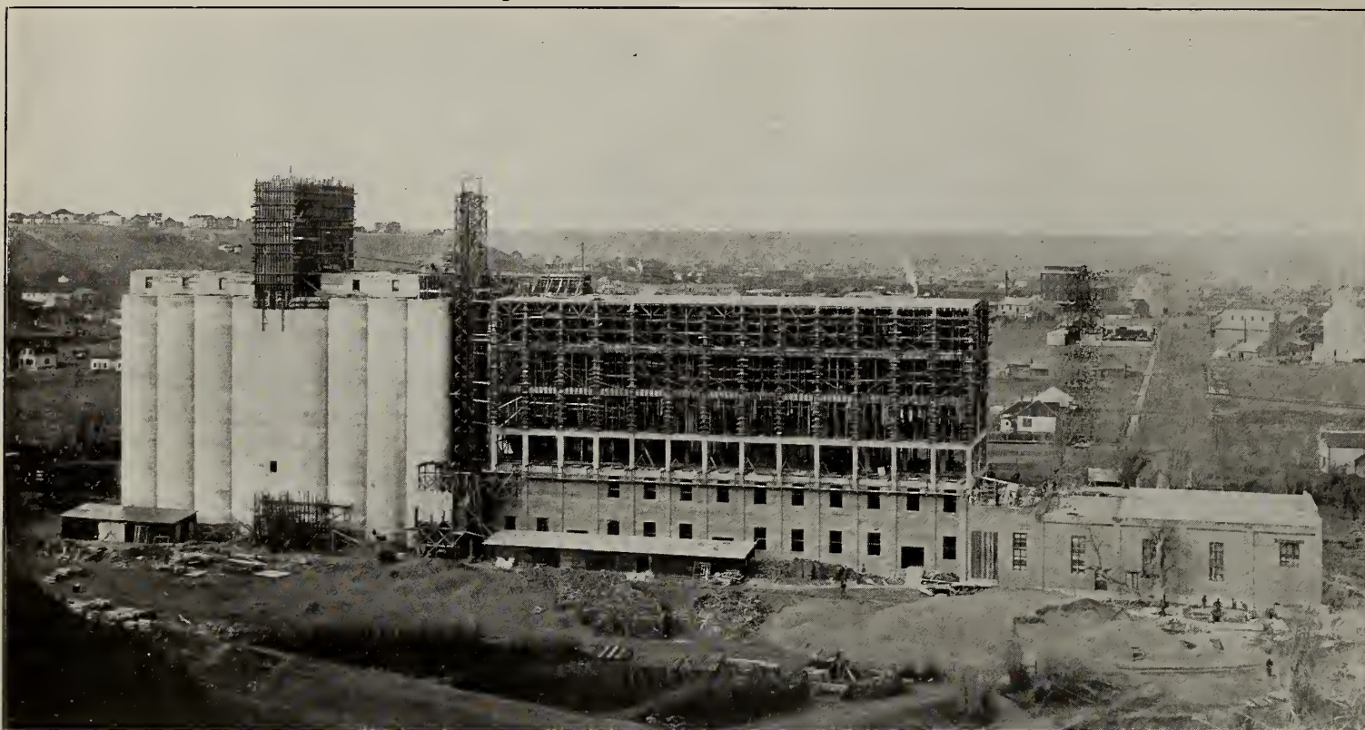
Ogilvie's 6,000 Barrel a Day Flour Mill Under Construction at Medicine Hat.
