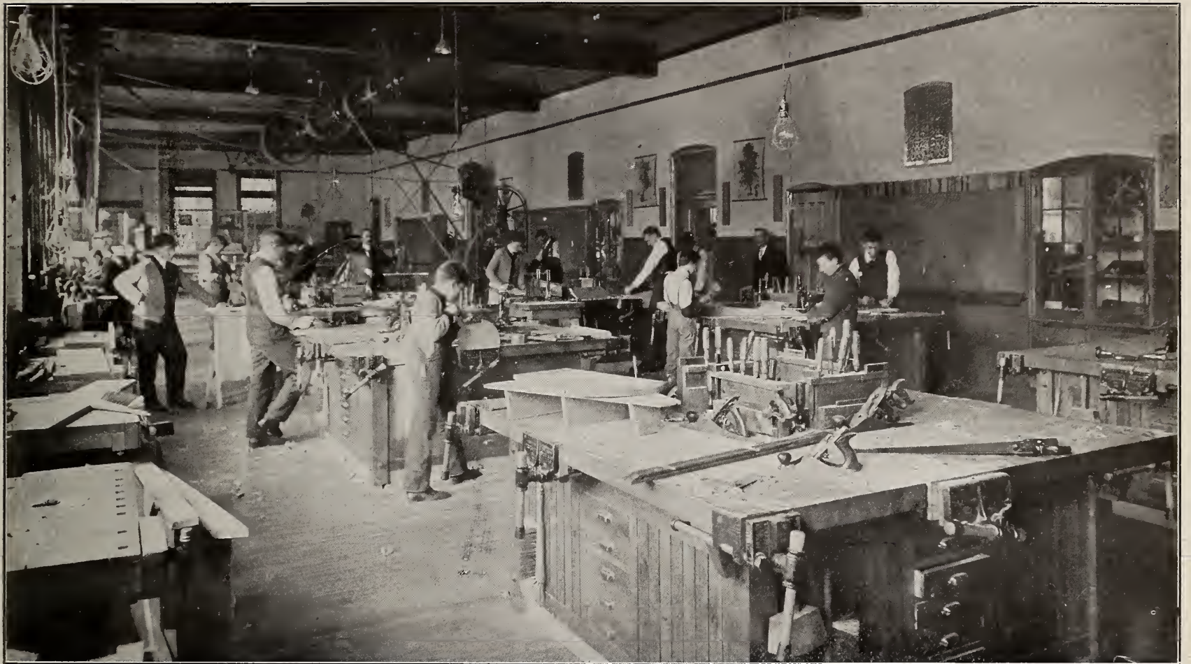
Industrial, Technical, and Art Schools, Hamilton—Wood Shop
