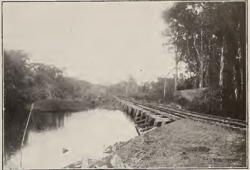
A Trestle which will be Replaced by a Steel Structure.
