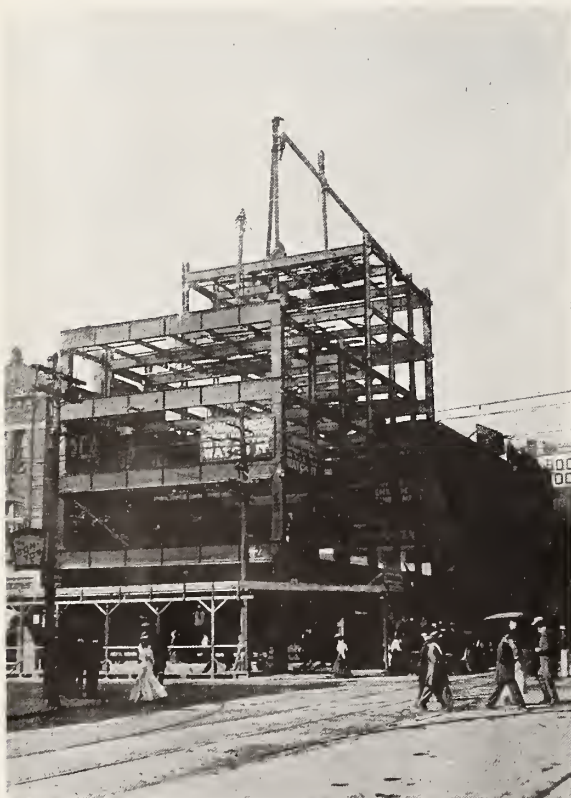
Erection just begun, July 27th
