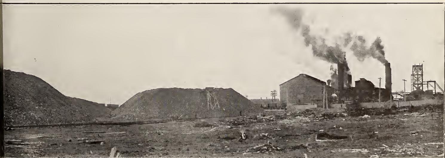
THE COAL PLANT AT GLACE BAY.
