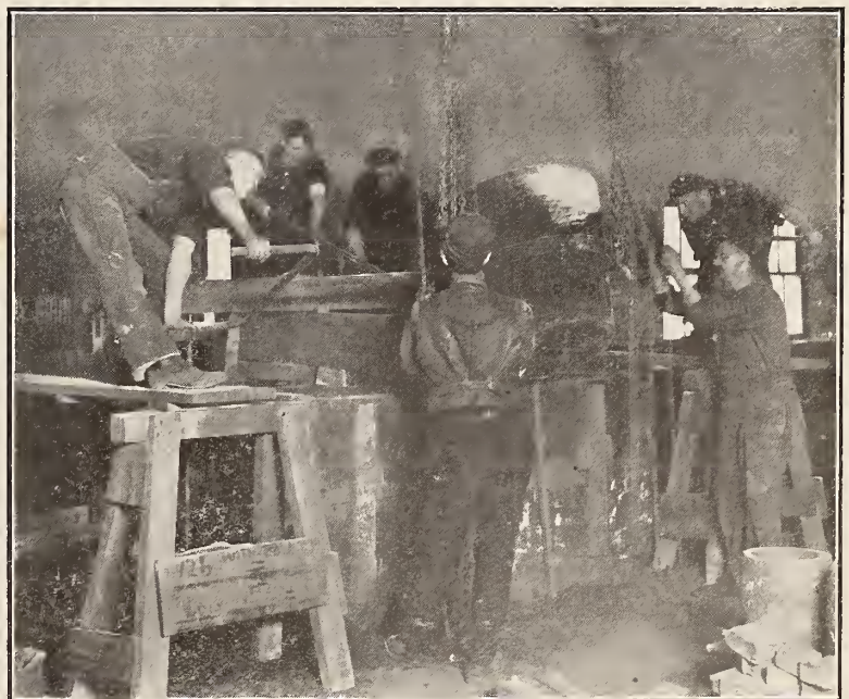
A big mould. The largest brass moulding ever made in Canada being made at the Lumen Bearing Co.'s Plant.
