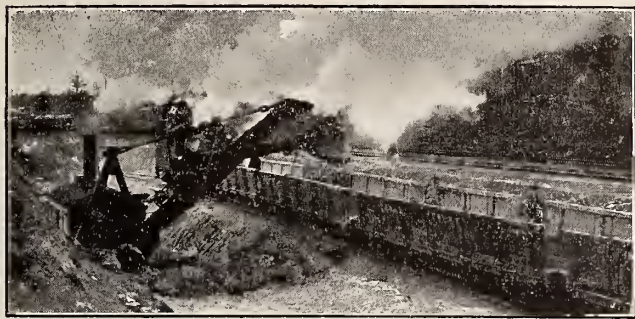
Reducing the Grade on the G.T.R. Entering Toronto
