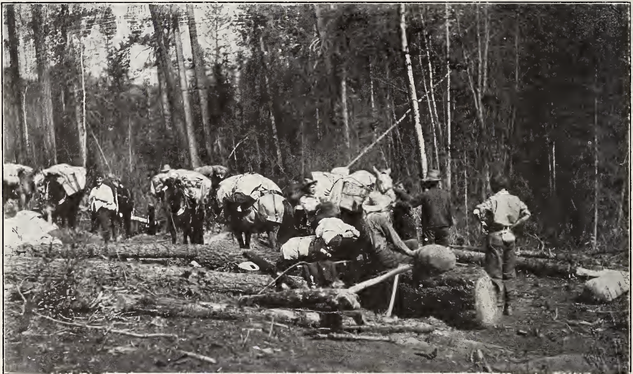
Clearing the Way—Packing the Provisions in over a trail which is being made along the surveyed line of a railway in British Columbia.
