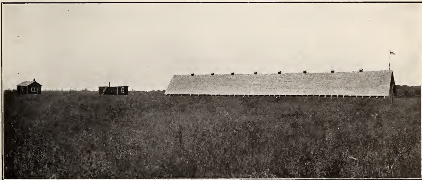
A Storage Shed for Peat.
