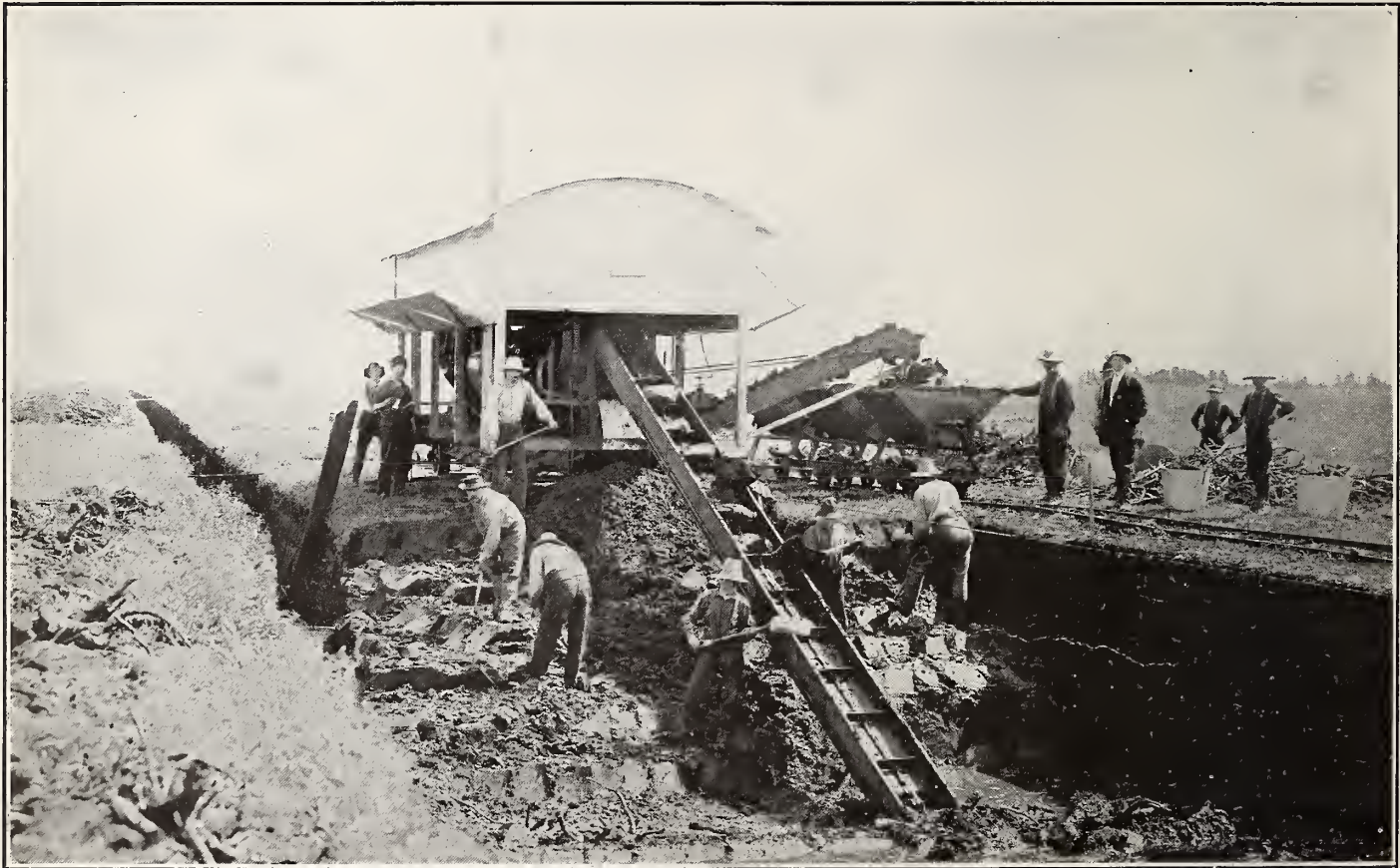
Excavating and Pulping the Peat.
