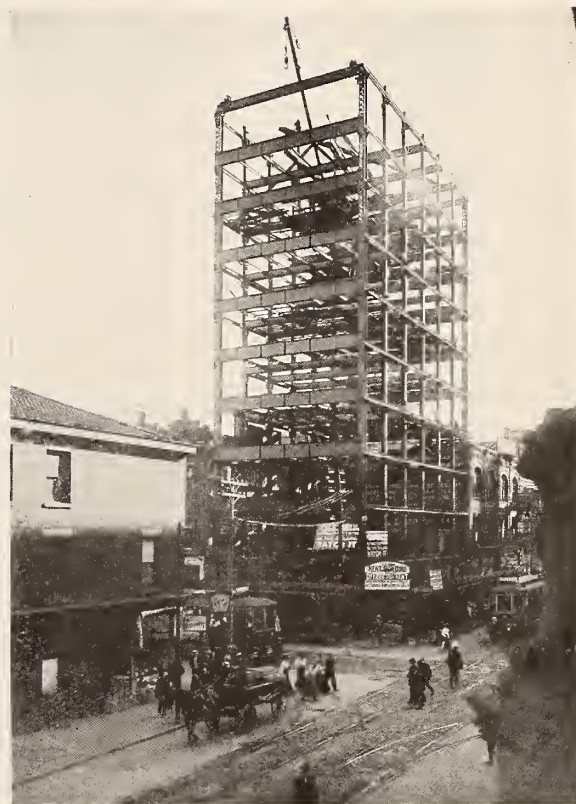
The Construction on Aug. 4th
