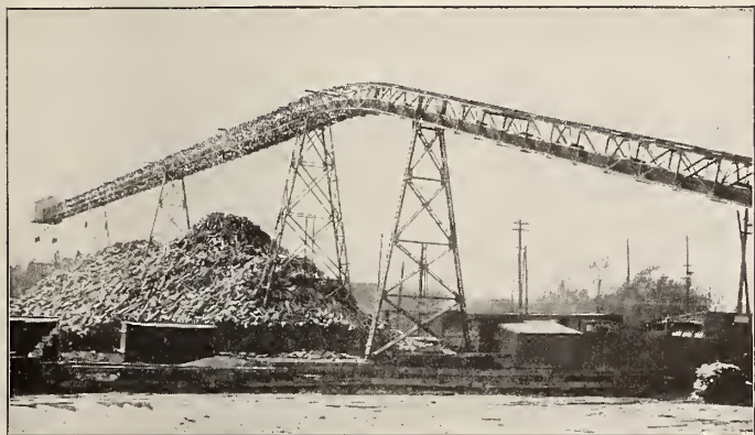
Pulpwood Conveyer E. B. Eddy Storage Yards
