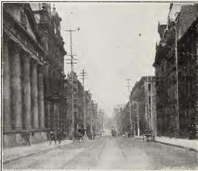
A Business Street in St. John
