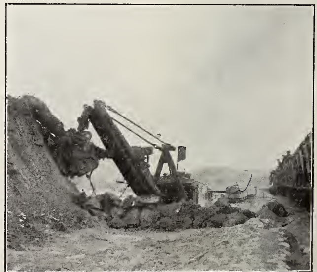
Cutting Away a Hill to Lower a Grade
