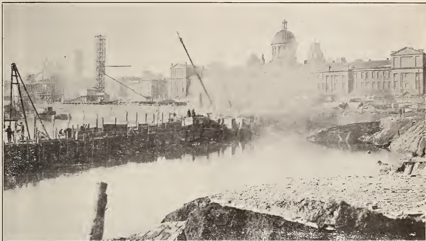
Concrete Quay Wall of the Victoria Pier, Montreal Harbor
