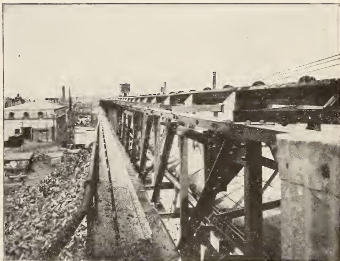
Rear View of Cable Conveyer Line Method of Delivering Stick Pulpwood.
