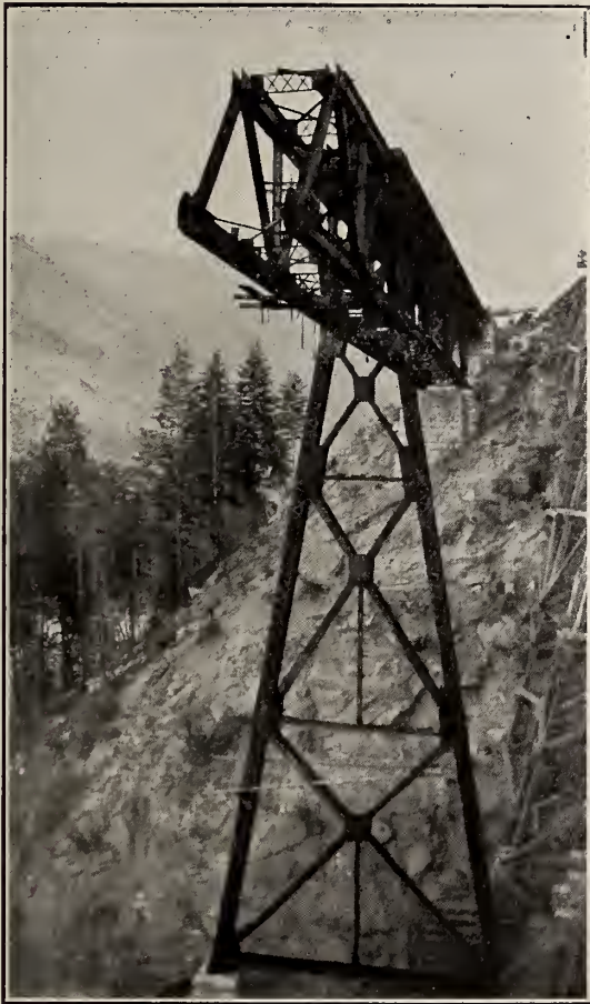
Placing the First Span.
