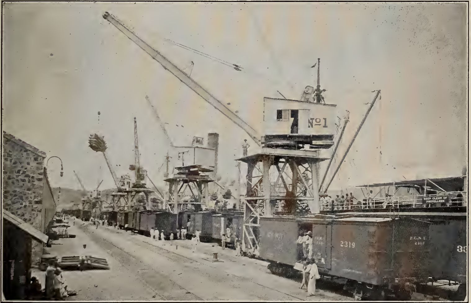
Terminal Facilities at Puerto, Mexico.
