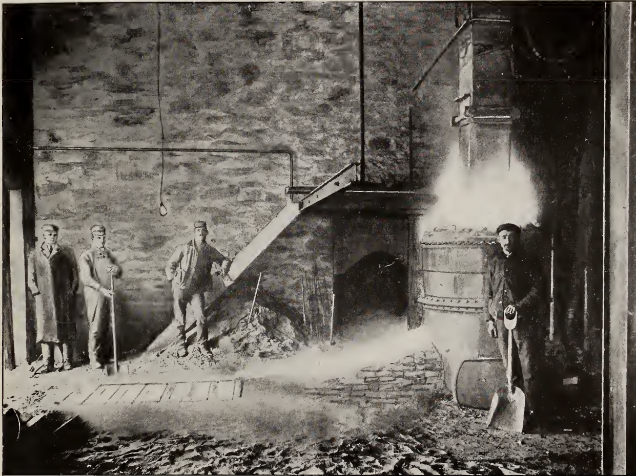
Electric Furnace Used in the Government Experiments at Sault Ste. Marie, Ont.
