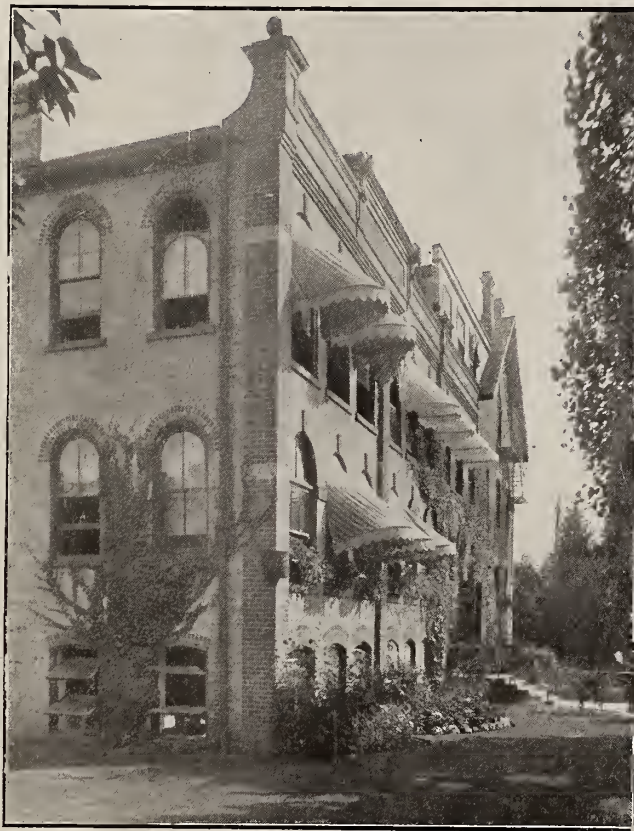
A Factory Like a Residence—The W. G. and R. Plant at Berlin.
