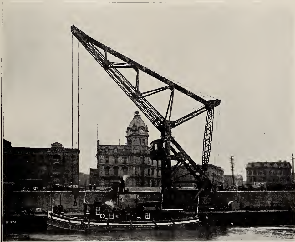
The New 75-Ton Crane Just Erected in the Montreal Harbor. With this New Equipment Montreal is Placed in the First Rank of Ocean Ports.
