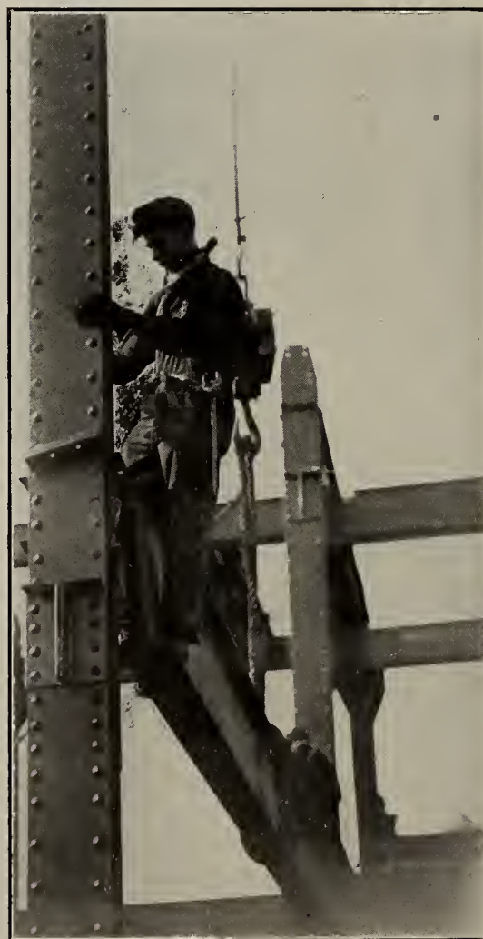
"They cling to an upright with a scanty foothold, while a piece of steel is being guided to its position."
