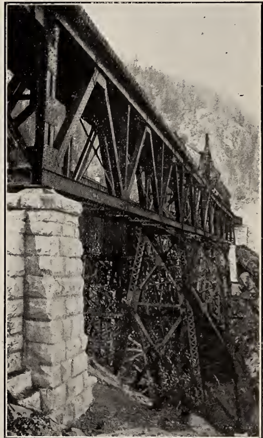
Bridge Almost Completed.
