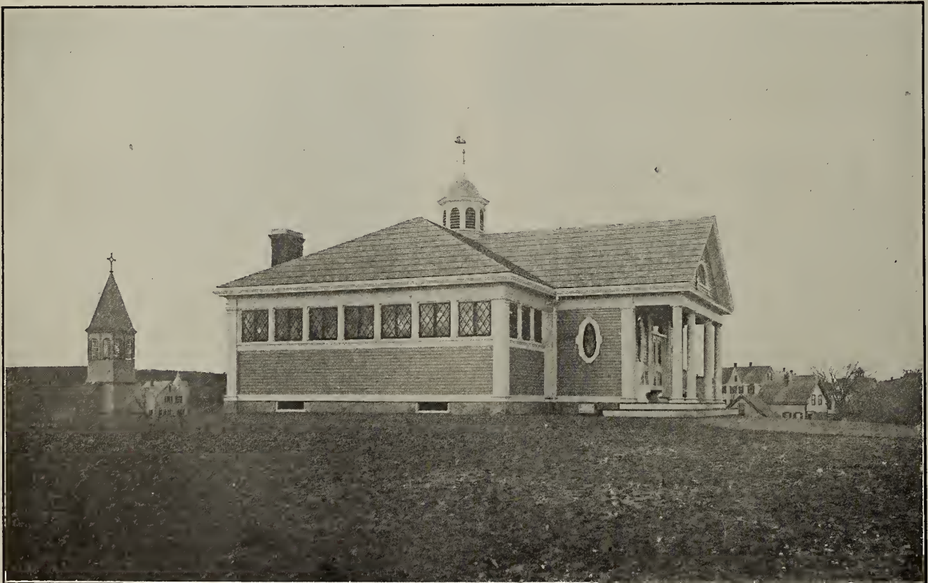
Library for Employees of the Plymouth Cordage Company
