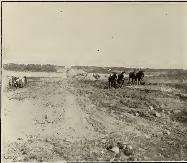
Grading on Main Line, Grand Trunk Pacific Railway.
