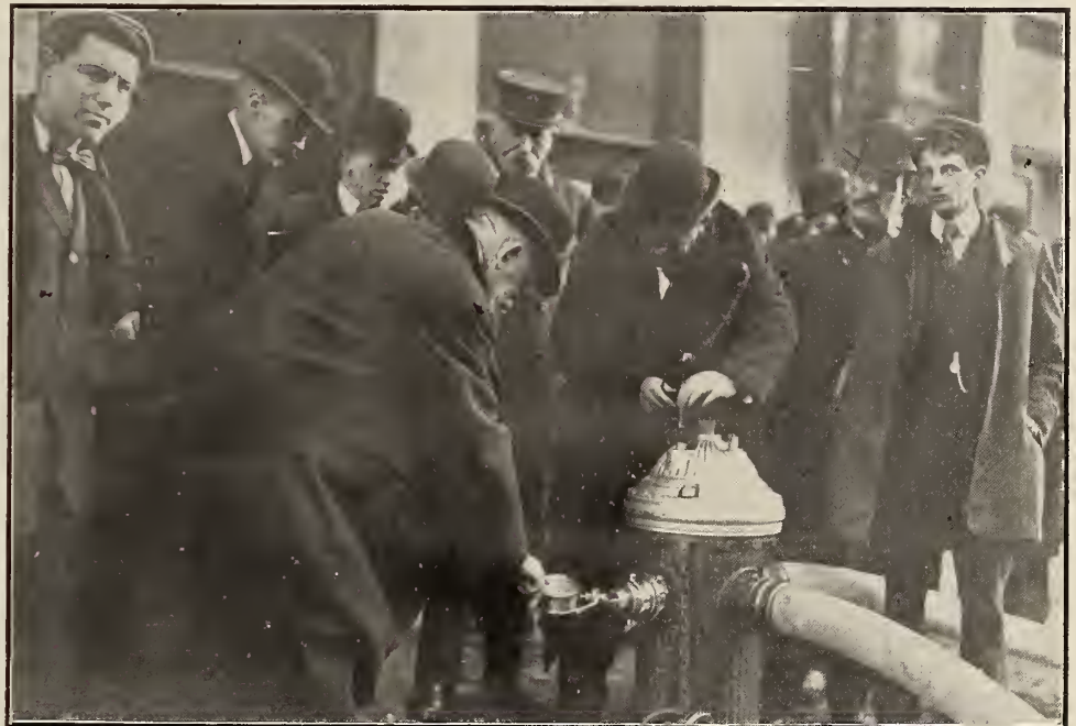
Reading the Gauge at Test of High Pressure System, Toronto
