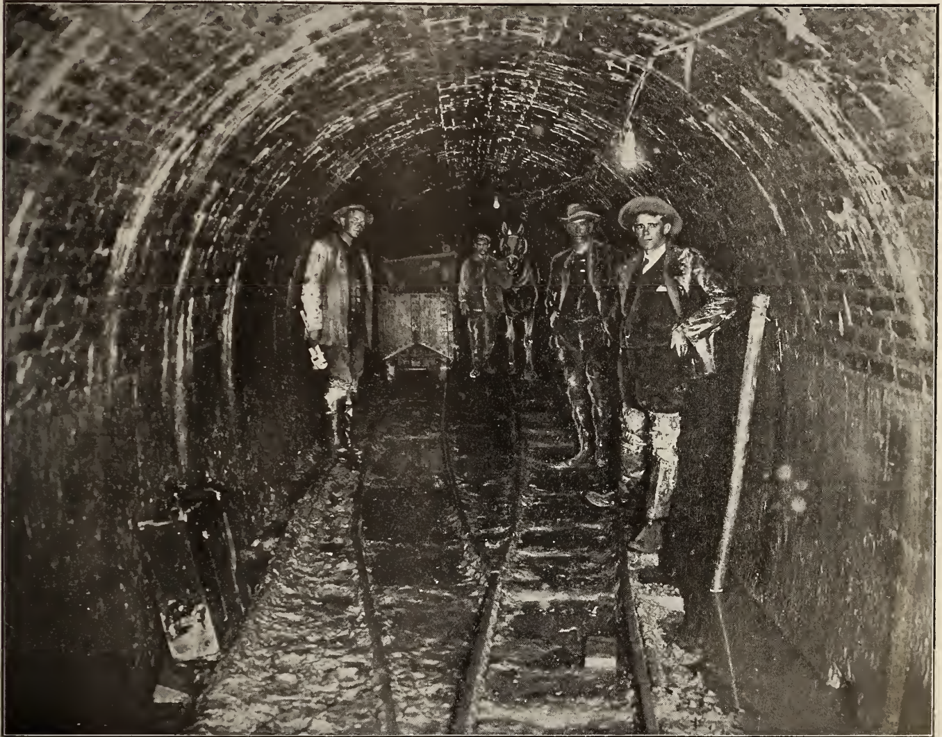
This illustration shows a section of the completed tunnel. Its size may be judged by comparing its height with that of the men working in it. The whole tunnel was finished a few days ago. Through it will pass all Toronto's water supply.
