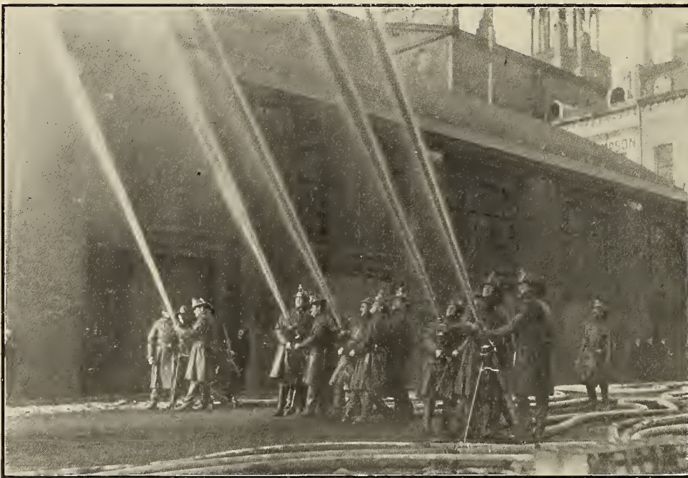
Testing Toronto's High Pressure Water System.
