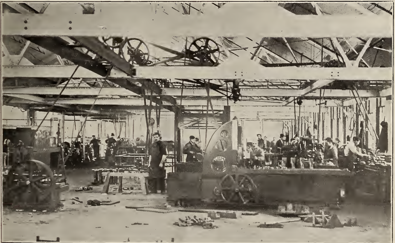
The Berlin Machine Works, Limited. An Example of Modern Factory Construction, Showing the Maximum of Light by Side Windows and Saw-Tooth Roof.
