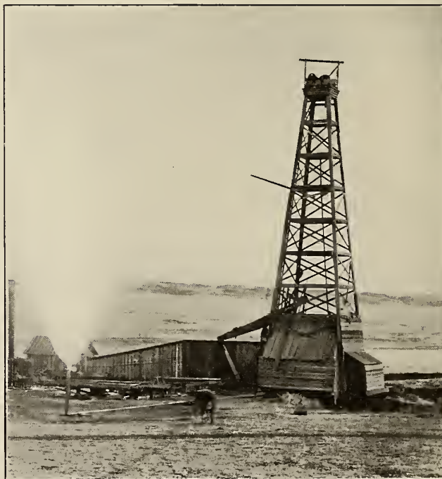
Natural Gas Well Shot in the Medicine Hat District. It has a Capacity of 7,500,000 Feet a Day.
