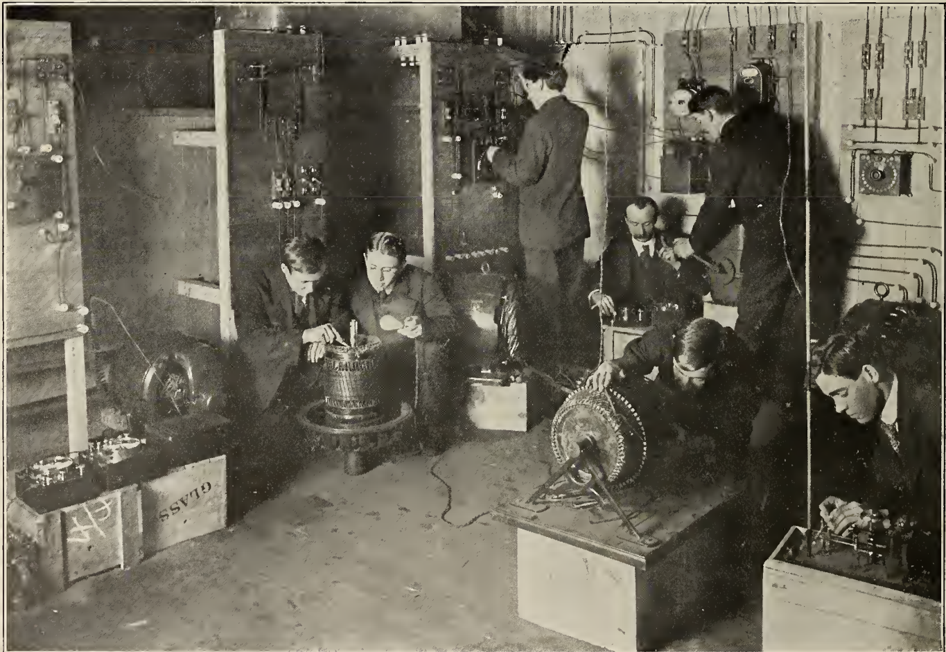
The Electrical Laboratory in Nova Scotia's Technical School.
