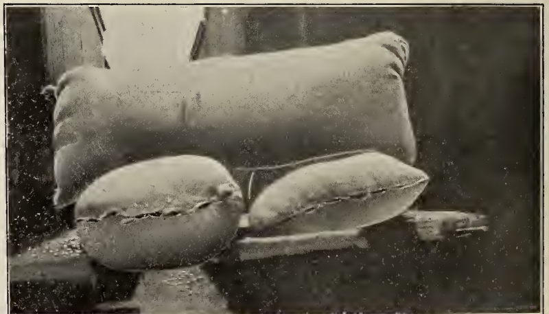
No. 8.—Bags that Leak.
