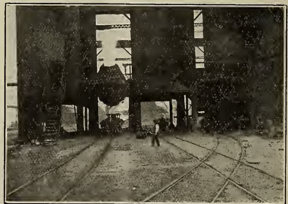
Bessemer Converter in Action
