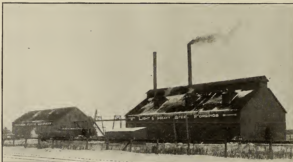
Plant of Canada Forge Co., Welland.
