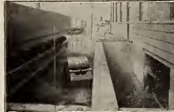
Jeffrey Grab Bucket Taking Coal from Storage Yard.
