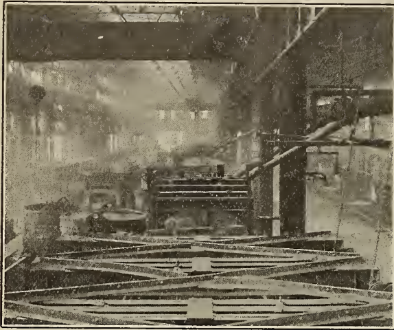
View along tops of open hearth furnaces.
