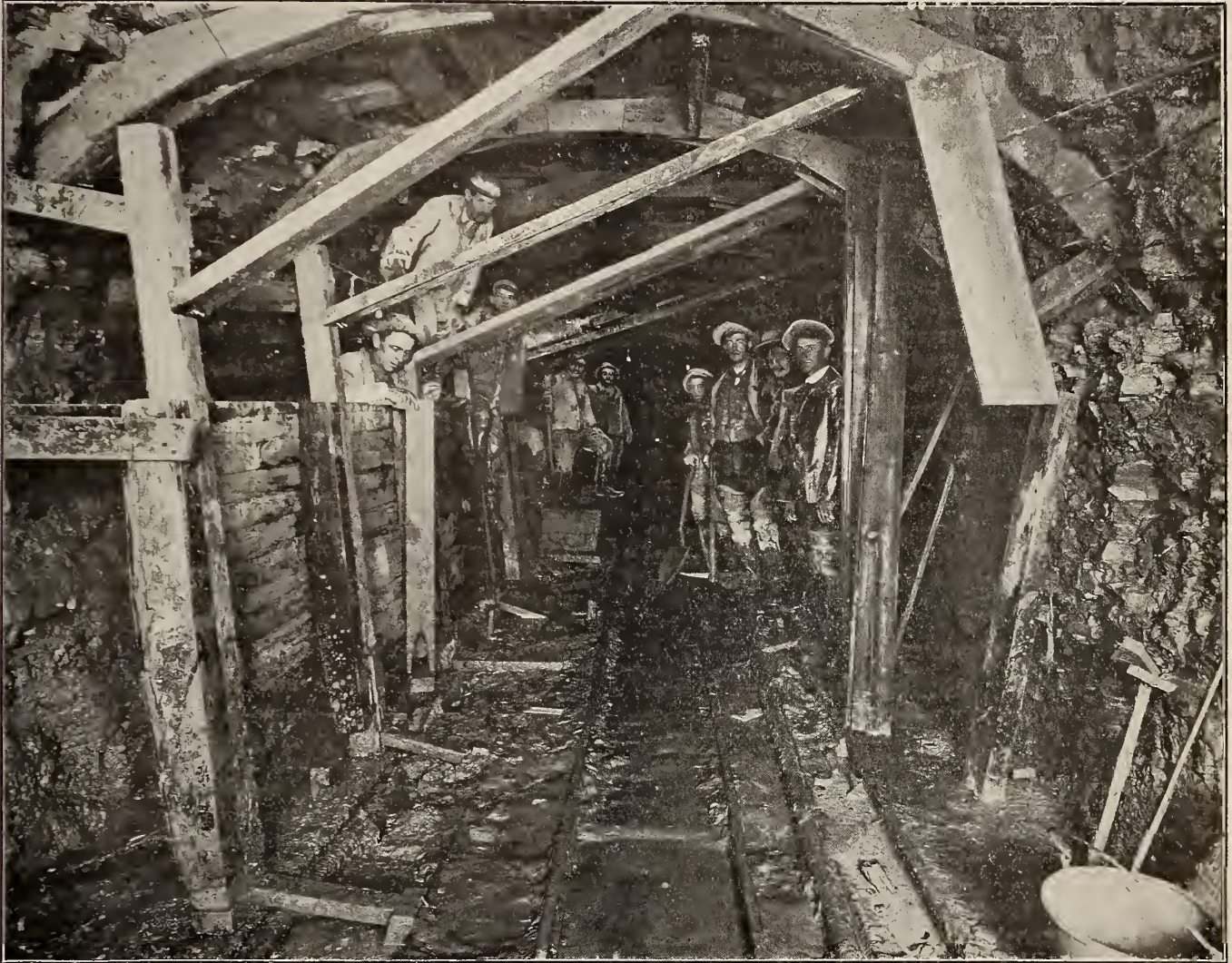
The above cut shows the tunnel under the Toronto Bay, in course of construction. The tunnel was built by Haney and Miller, Toronto.
