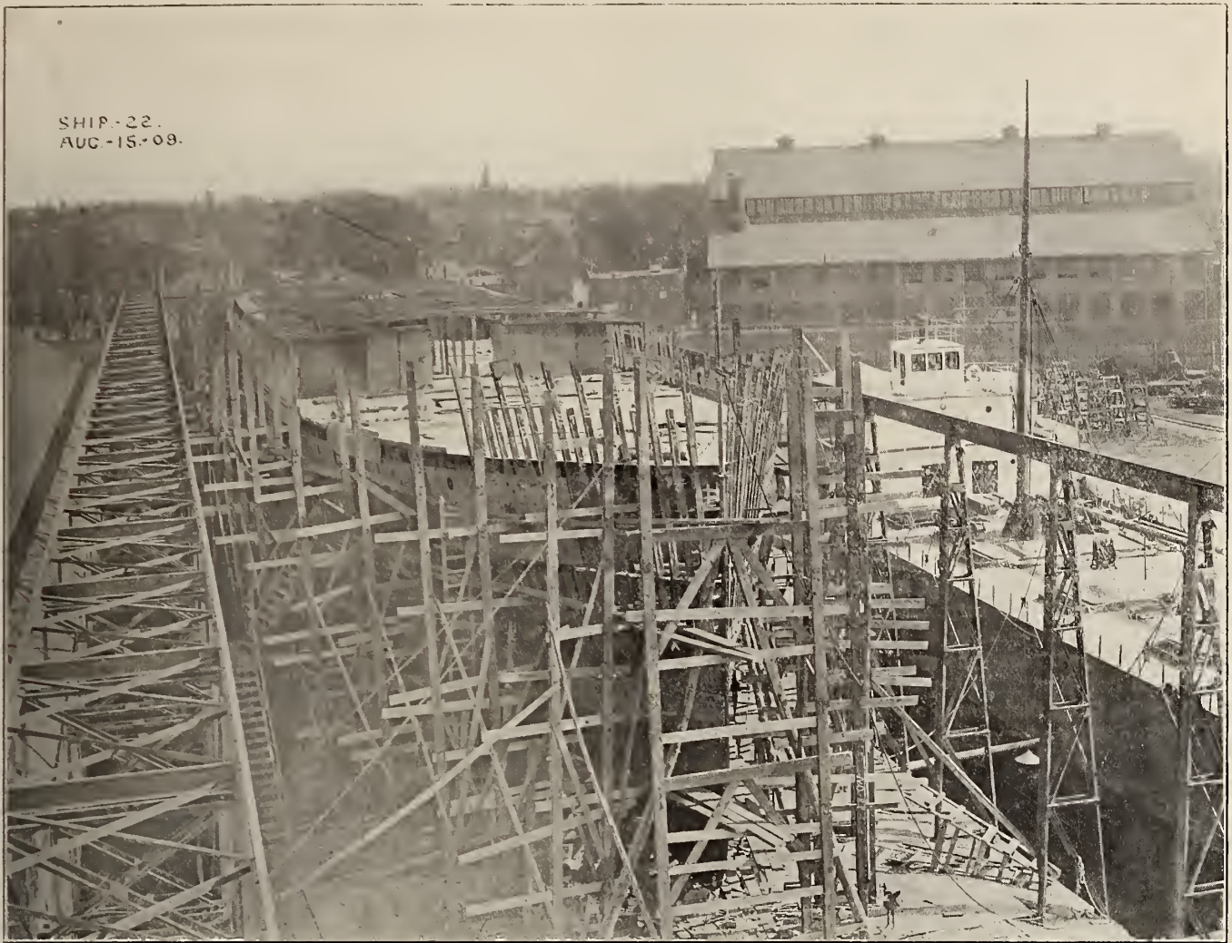
Steamship in Advanced Stage of Construction.
