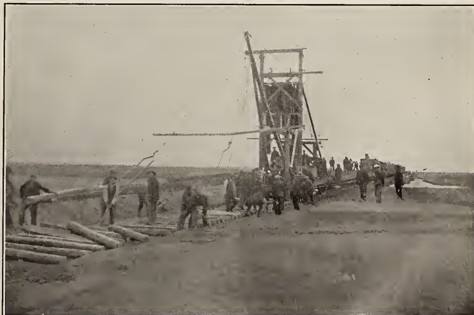
Track Laying on the Prairie.
