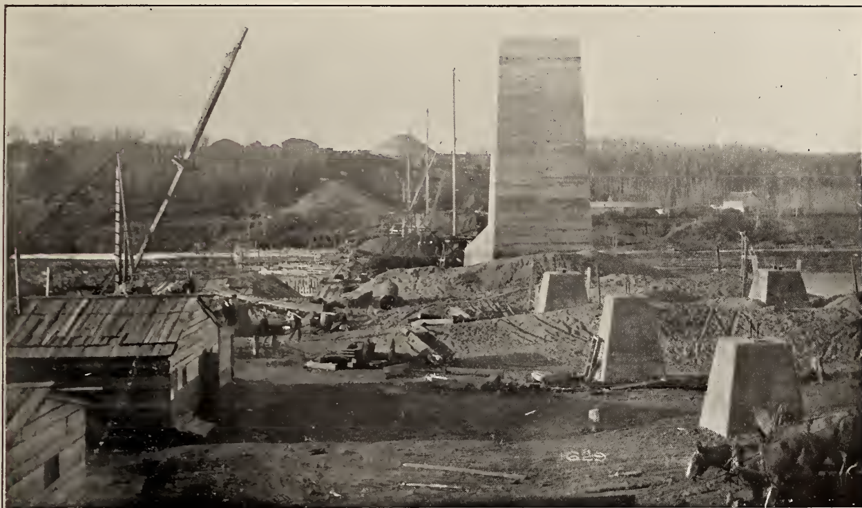
General View of Work from Pier No. 5, Near Edmonton.
