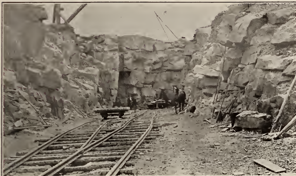
Rock Cutting on National Transcontinental Railway, 178 miles east of Winnipeg.
