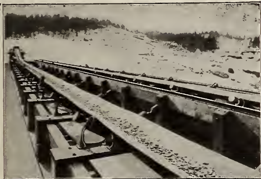
Jeffrey "Century" Rubber Belt Conveyor Handling Stone.
