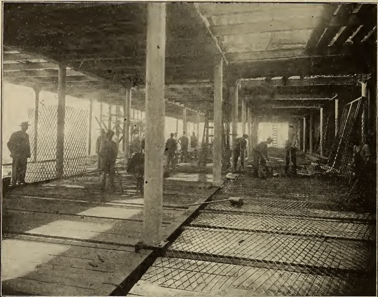
Re-inforced Concrete in Flooring
