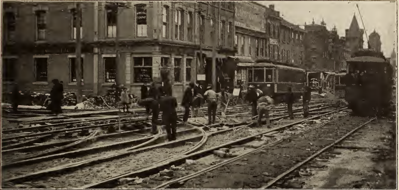
Tracks are now renewed without much interruption to traffic. This cut shows the method of operation in Toronto. Temporary tracks are laid on each side of the street and cars are operated on these, leaving the centre of the road free for work.
