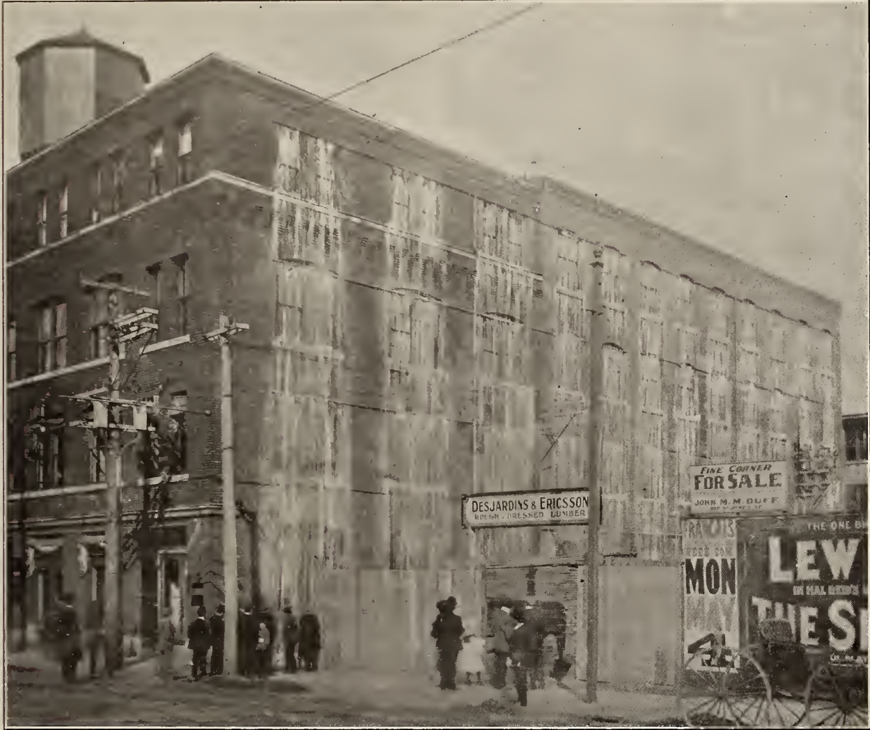
The above illustration shows a water curtain in actual operation. By protecting the windows it makes the building practically proof against fire from without.
