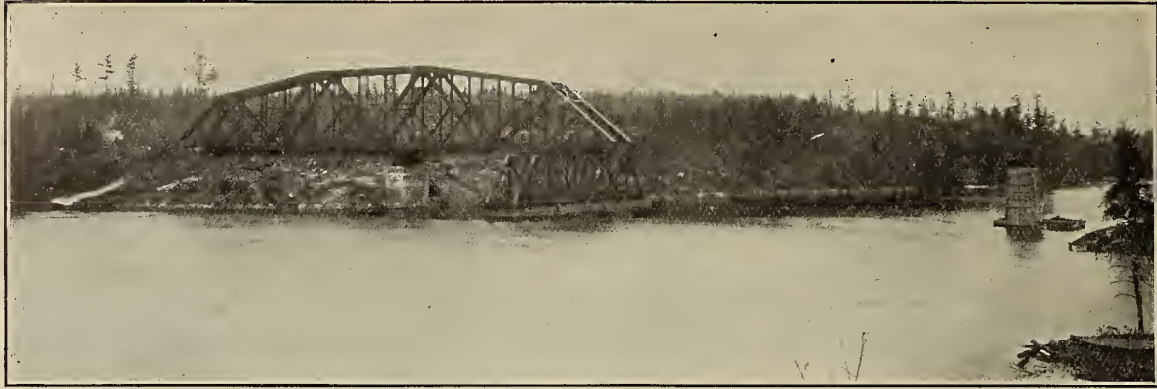
The Span ready to be carried across the French River
