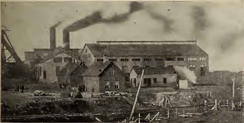
No. 2 Colliery, Dominion Coal Co., Glace Bay. Walls, Roofs and Floors by Expanded Metal System.
