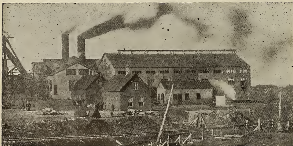
No. 2 Colliery, Dominion Coal Co., Glace Bay. Walls, Roofs and Floors by Expanded Metal System.
