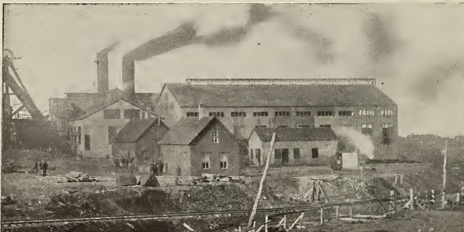
No. 2 Colliery, Dominion Coal Co., Glace Bay. Walls, Roofs and Floors by Expanded Metal System.
