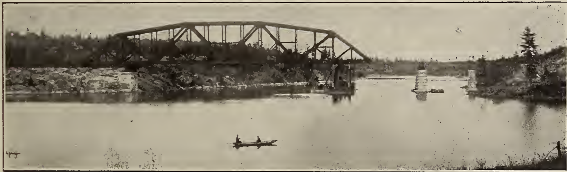
The Span being carried out to Second Pier.
