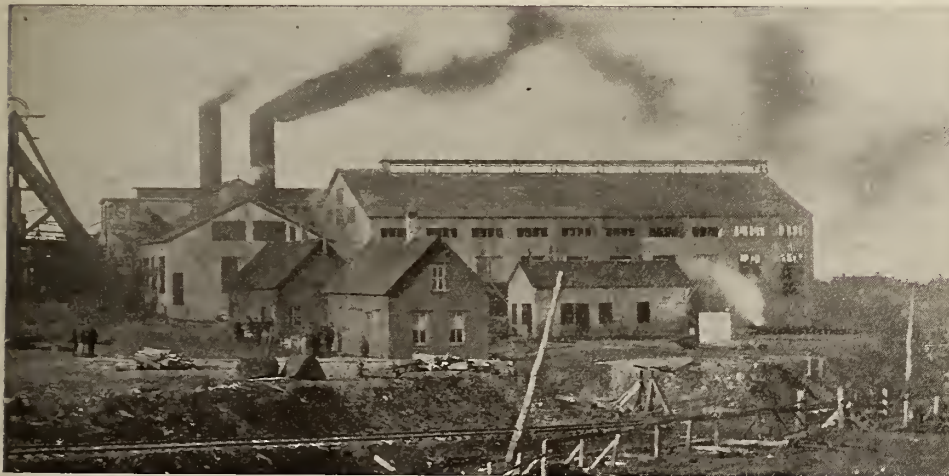
No. 2 Colliery, Dominion Coal Co., Glace Bay. Walls, Roofs and Floors by Expanded Metal System.
