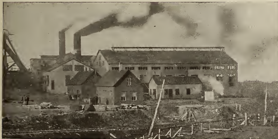
No. 2 Colliery, Dominion Coal Co., Glace Bay. Walls, Roofs and Floors by Expanded Metal System.
