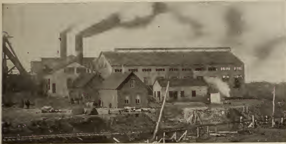
No. 2 Colliery, Dominion Coal Co., Glace Bay. Walls, Roofs and Floors by Expanded Metal System.
