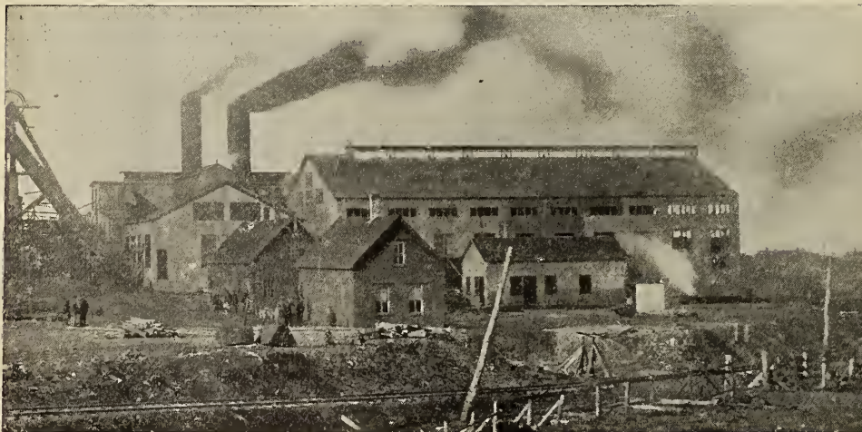
No. 2 Colliery, Dominion Coal Co., Glace Bay. Walls, Roofs and Floors by Expanded Metal System.
