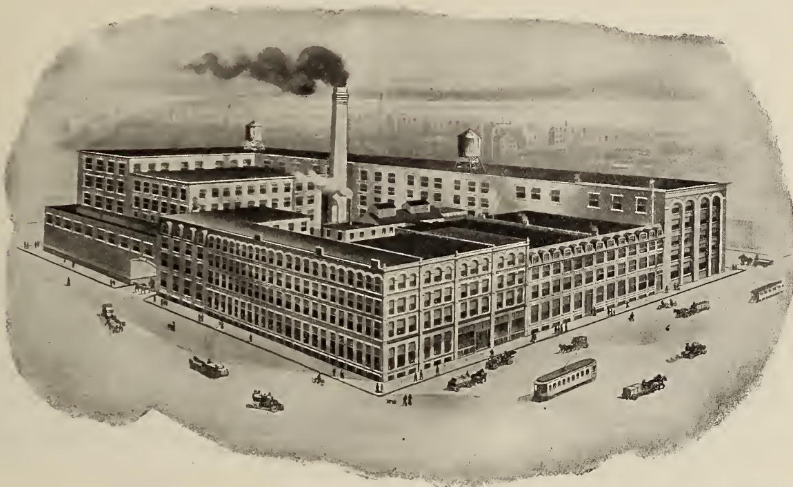
A Modern Factory Building (Robertson Bros, Toronto), where the Absence of Heavy Machinery Admits of a High Building.
