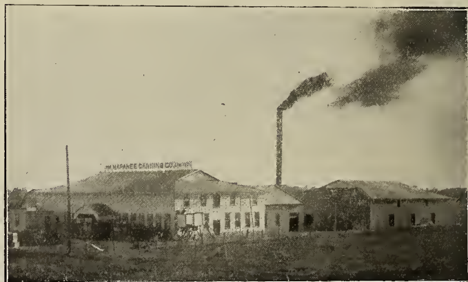
Canning Factory in which Metal Siding is used to Advantage.
