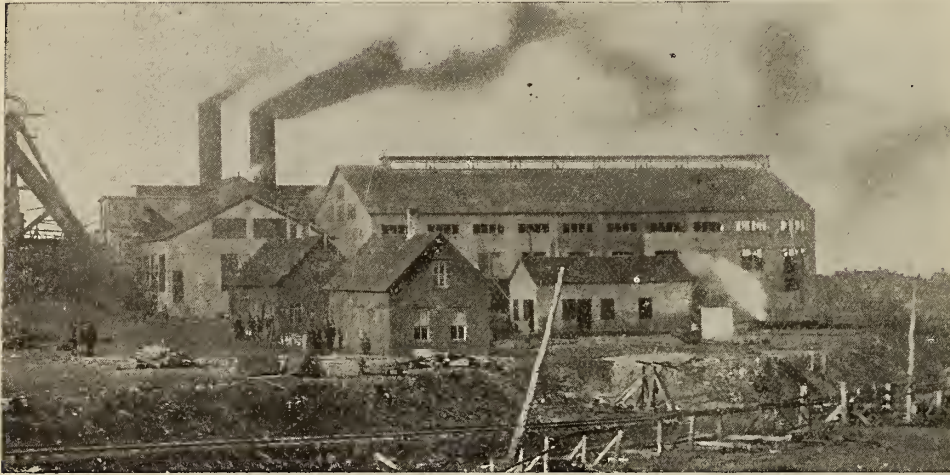
No. 2 Colliery, Dominion Coal Co., Glace Bay. Walls, Roofs and Floors by Expanded Metal System.
