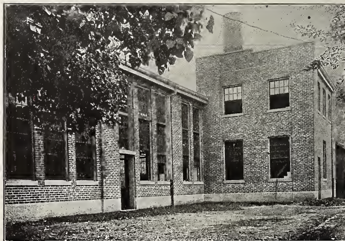
School for Iron Moulders, Winona Technical Institute.
