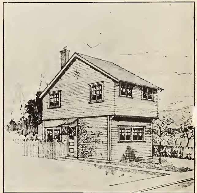
A house designed by F. S. Baker, Toronto, which could be built for $900.
