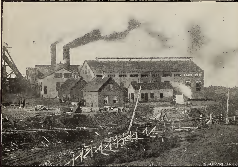
No. 2 Colliery, Dominion Coal Co., Glace Bay. Walls, Roofs and Floors by Expanded Metal System.
