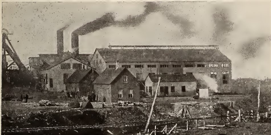
No. 2 Colliery, Dominion Coal Co., Glace Bay. Walls, Roofs and Floors by Expanded Metal System.
