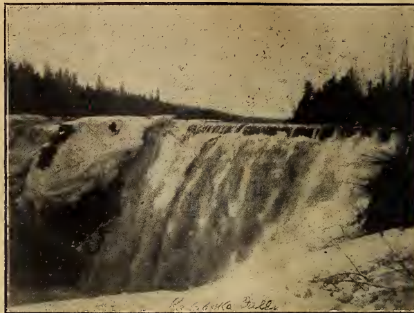
KAKABEKA FALLS, NEAR FORT WILLIAM, NOW HARNESSSED. Producing 30,000 horse power of electrical energy, distributed at Fort William.
