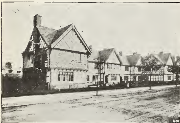
Row of Workingmen's Cottages at Port Sunlight, England. They rent for $1.25 a week.
