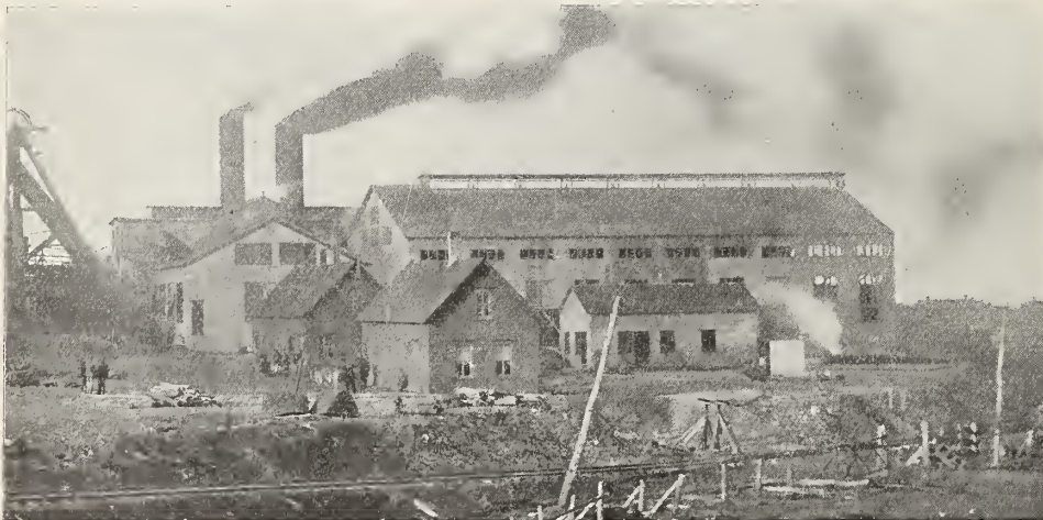
No. 2 Colliery, Dominion Coa. Co., Glace Bay. Walls, Roofs and Floors by Expanded Metal System.
