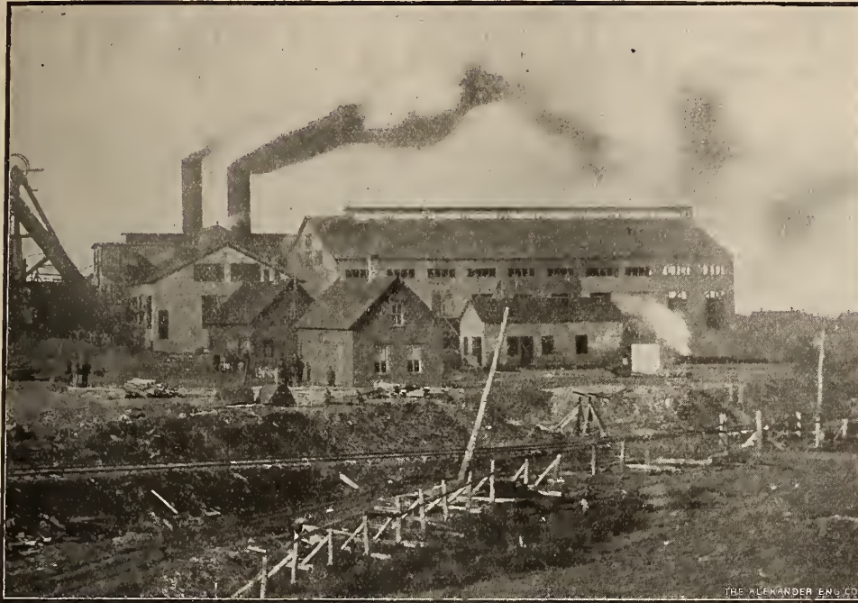
No. 2 Colliery, Dominion Coal Co., Glace Bay. Walls, Roofs and Floors, by Expanded Metal System.
