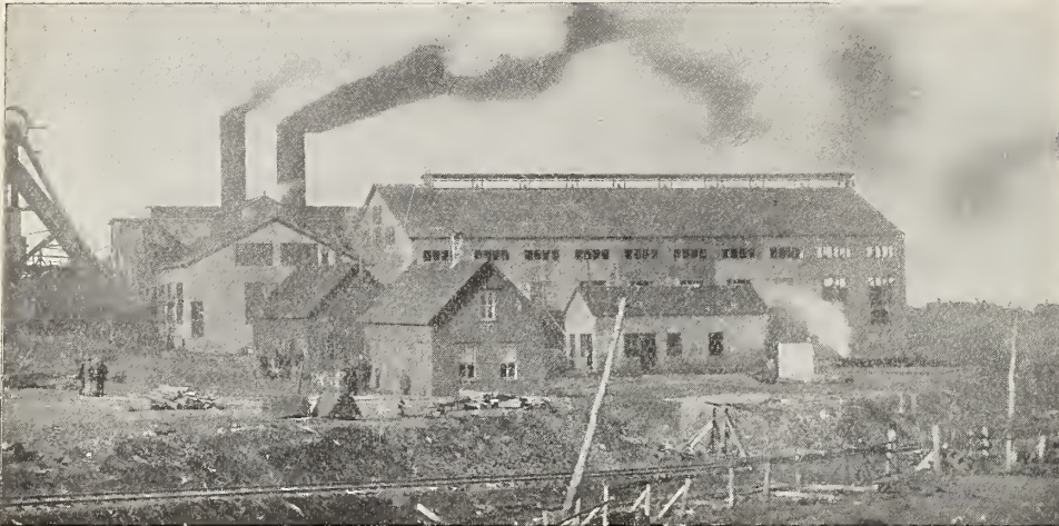
No. 22 Colliery, Dominion Coal Co., Glace Bay. Walls, Roofs and Floors by Expanded Metal System.
