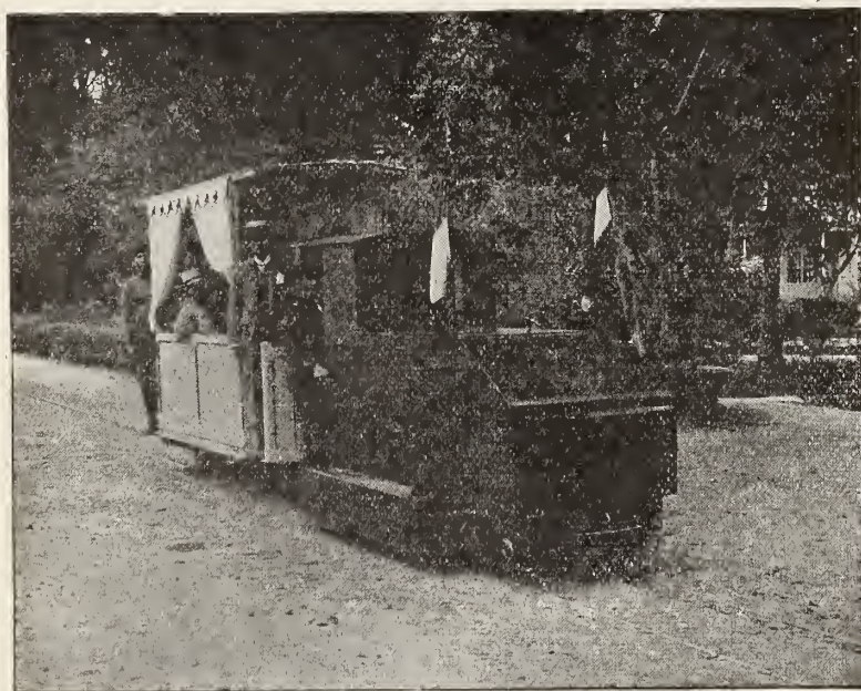
Fig. 2.—An 8 H.P. Alcohol Locomotive, built at Deutz, in Germany, for Service at Lima, Peru.
