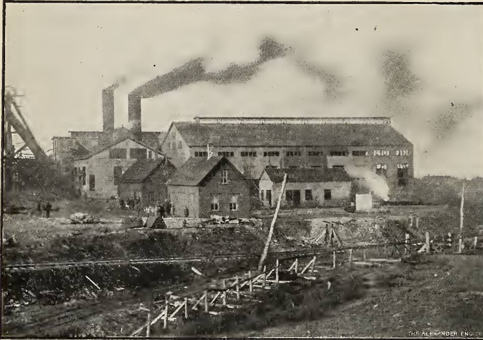
No. 2 Colliery, Dominion Coal Co., Glace Bay. Walls, Roofs and Floors by Expanded Metal System.
