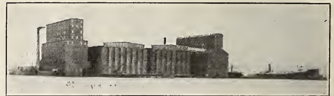
The Elevators from the Bay.
