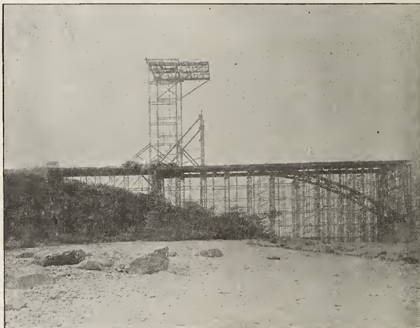
Traveller at Work, South Shore Anchor Arm.
