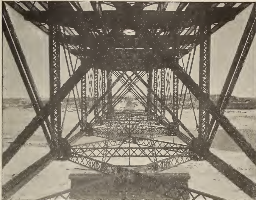
General View from underneath the Approach Span.
