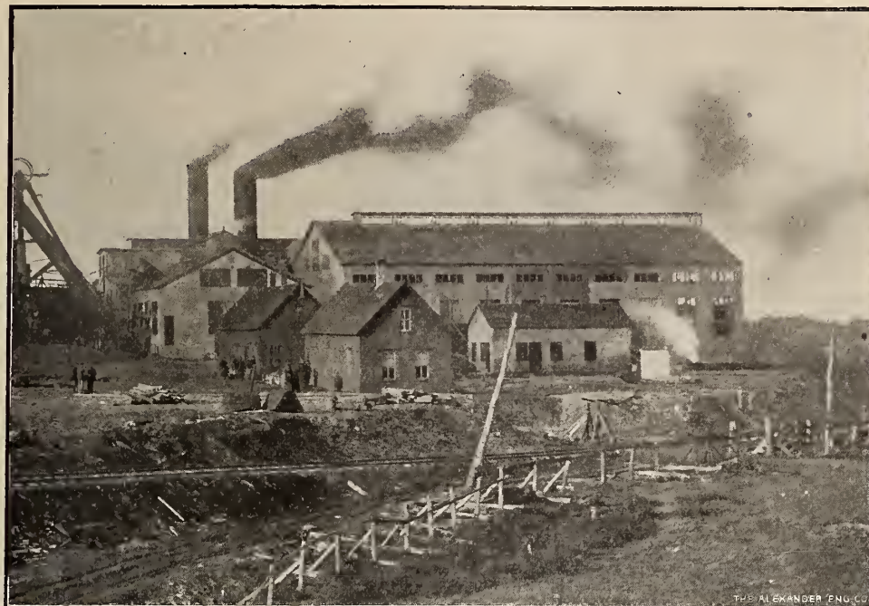
No. 2 Colliery, Dominion Coal Co., Glace Bay. Walls, Roofs and Floors by Expanded Metal System.
