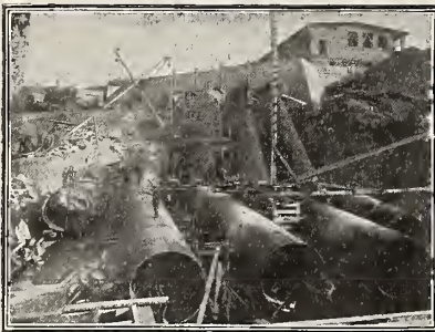
Erecting Steel Penstocks at Spanish River Pulp Mill, Espanola, Ont.
