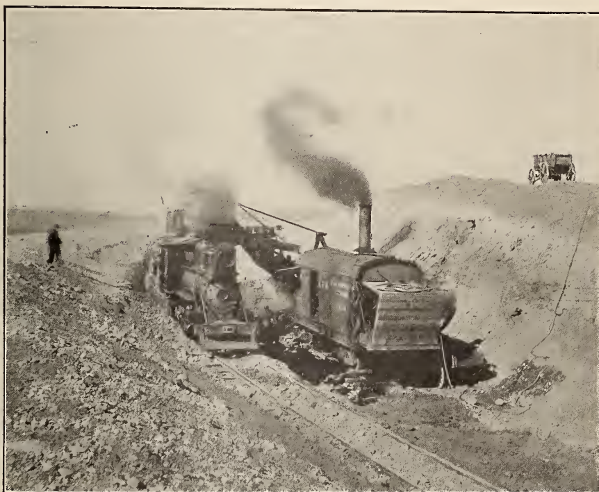
Steam Shovel Excavating on Main Canal.
