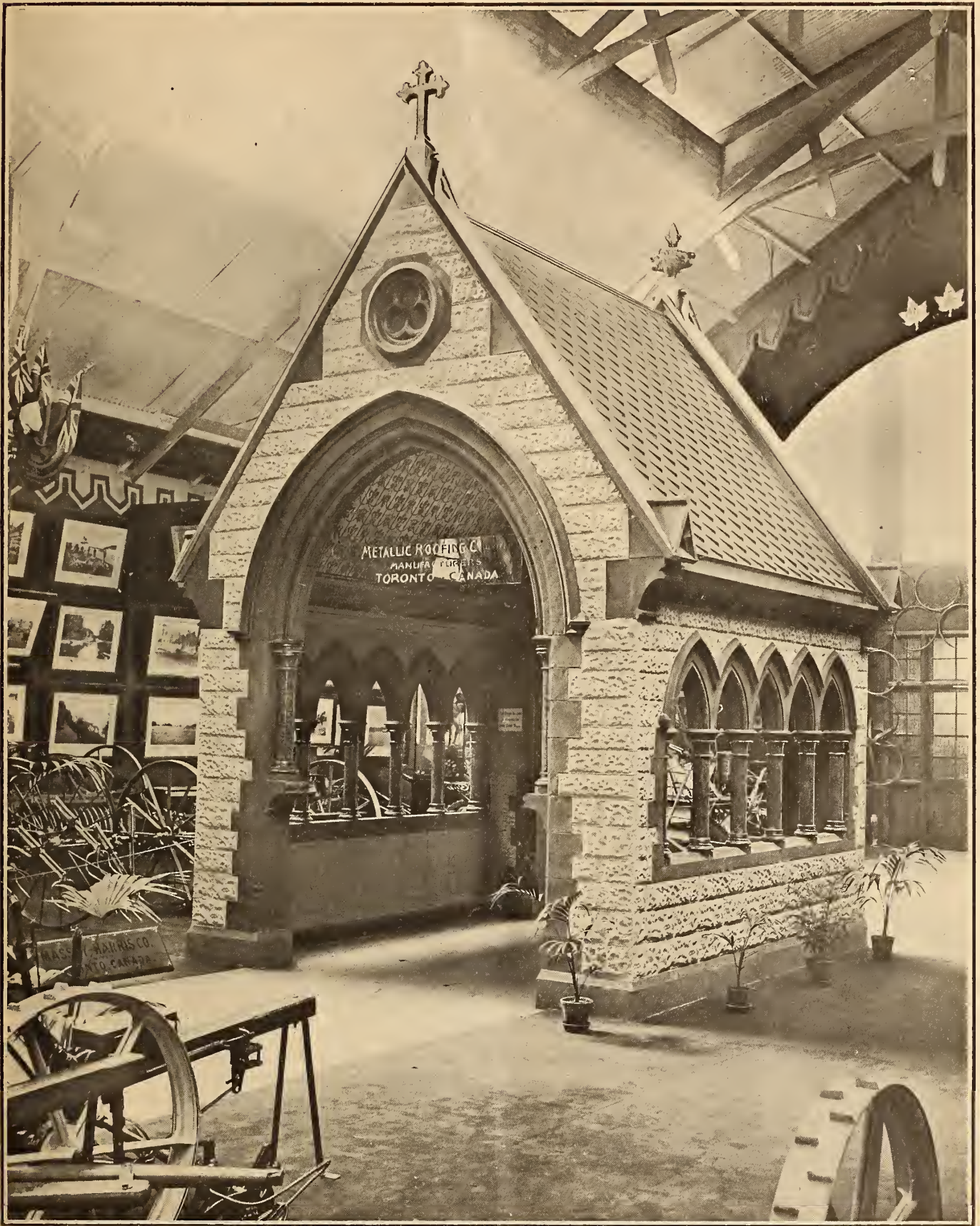
EXHIBIT OF THE METALLIC ROOFING CO., LIMITED, TORONTO, AT THE GLASGOW INTERNATIONAL EXHIBITION, 1901.
