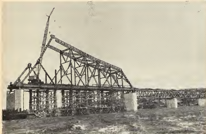
Interprovincial Bridge, Campbellton, N.B.—CROSS POINT, Que. —showing anchor span.
