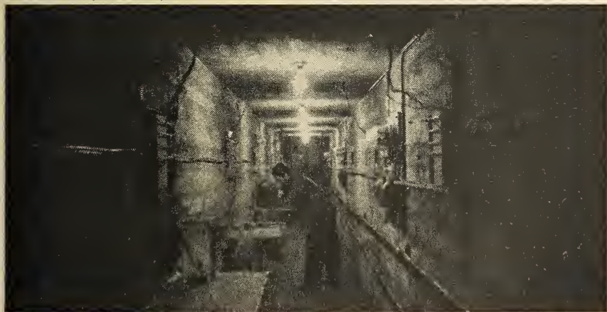
Fig. 3. View of the tunnel at Saskatoon providing access and services to the test huts above. Readings of thermocouples, power inputs and other instrumentation can be taken in the tunnel without disturbing the hut conditions. (Photo: National Film Board of Canada).
