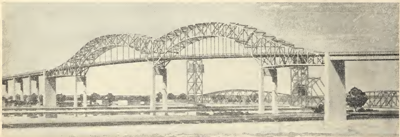
Fig. 3. View of Canadian Canal Crossing
