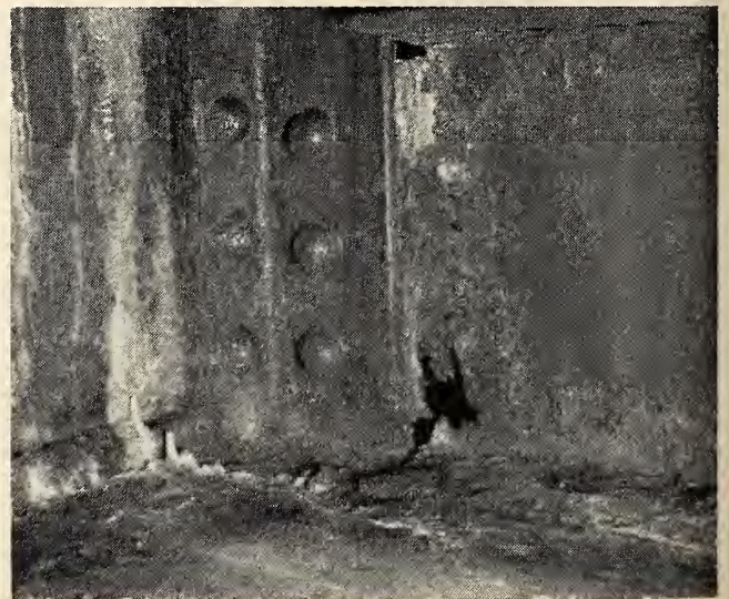
Fig. 10. Examples of Corroded Steelwork — Dundas Street Bridge.
