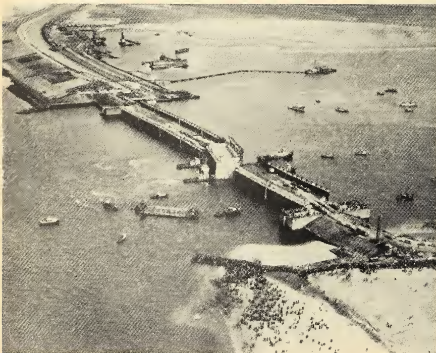
Fig. 1 The Final stage in closing the Veerse Gat estuary
