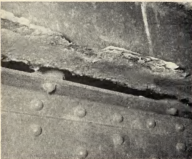
Fig. 10. Examples of Corroded Steelwork — Dundas Street Bridge.
