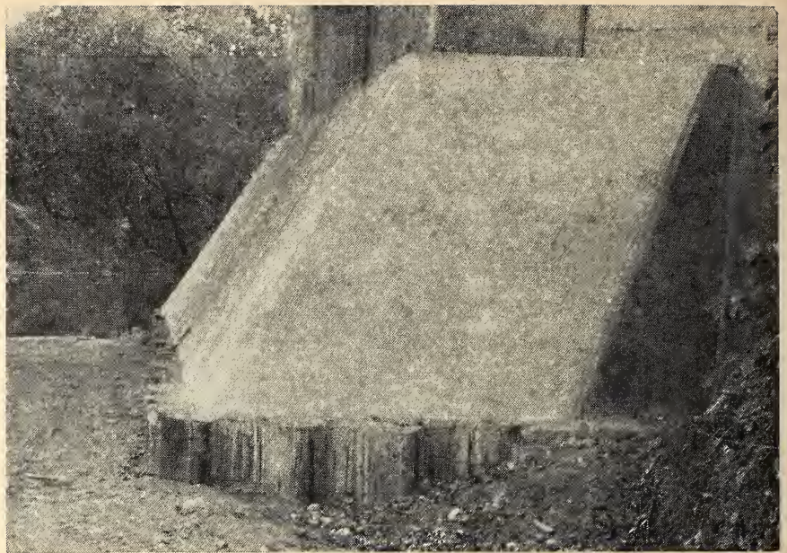
Fig. 7. Complete stabilization of South abutment of Richmond Street Bridge.
