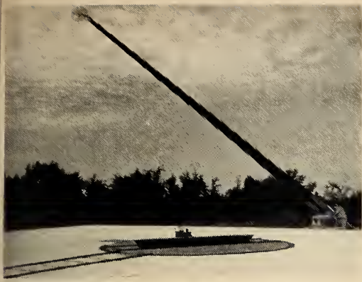
Fig. 1. 60 ft. boom in elevated position.
