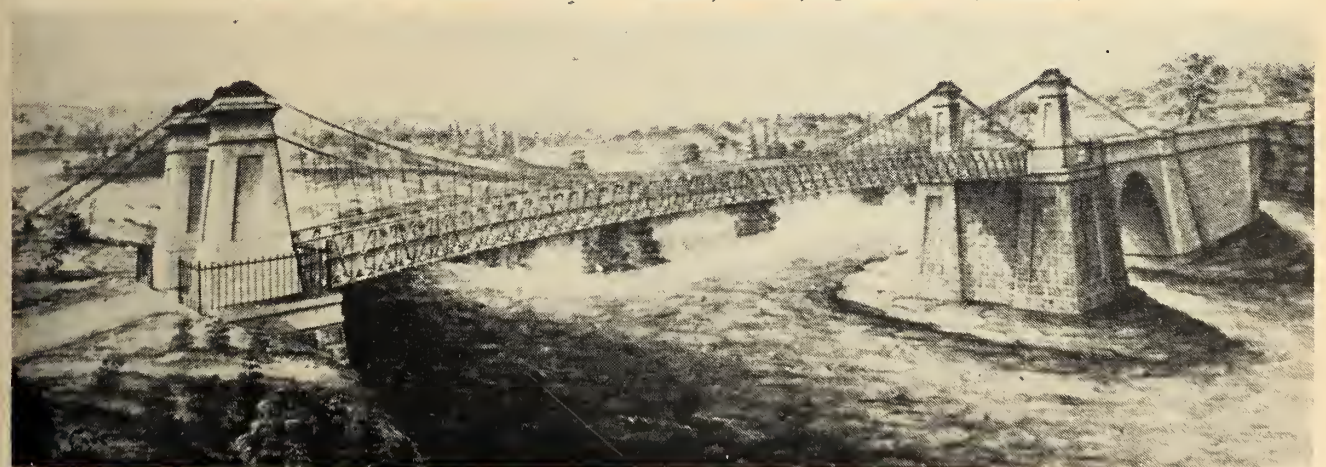
Fig. 1. The Second Union Bridge, designed by Samuel Keefer, having a clear span of 243 ft. 6 in.; opened in 1844 (From a water colour in the Public Archives of Canada, Ottawa; reproduced by permission).
