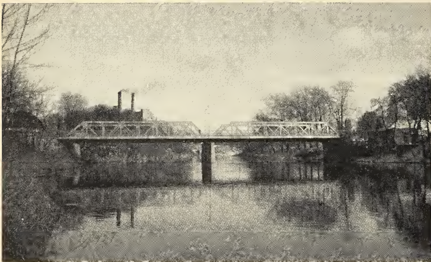
Fig. 2. Typical Bridges: Wellington St. & Blackfriars St.
