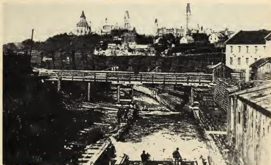
Fig. 3. Part of a timber raft going down one of the Chaudière timber slides towards the end of the nineteenth century. (From a Tapley photograph in the Public Archives of Canada; reproduced by permission.)
