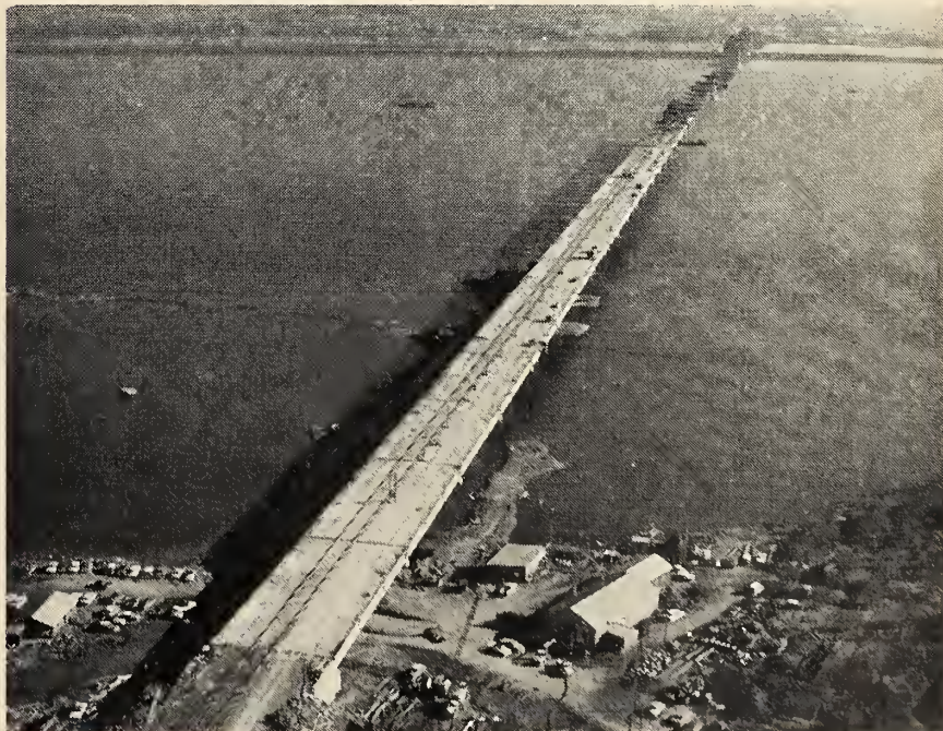
Fig. 2. Part of section three south of Nuns' Island.
