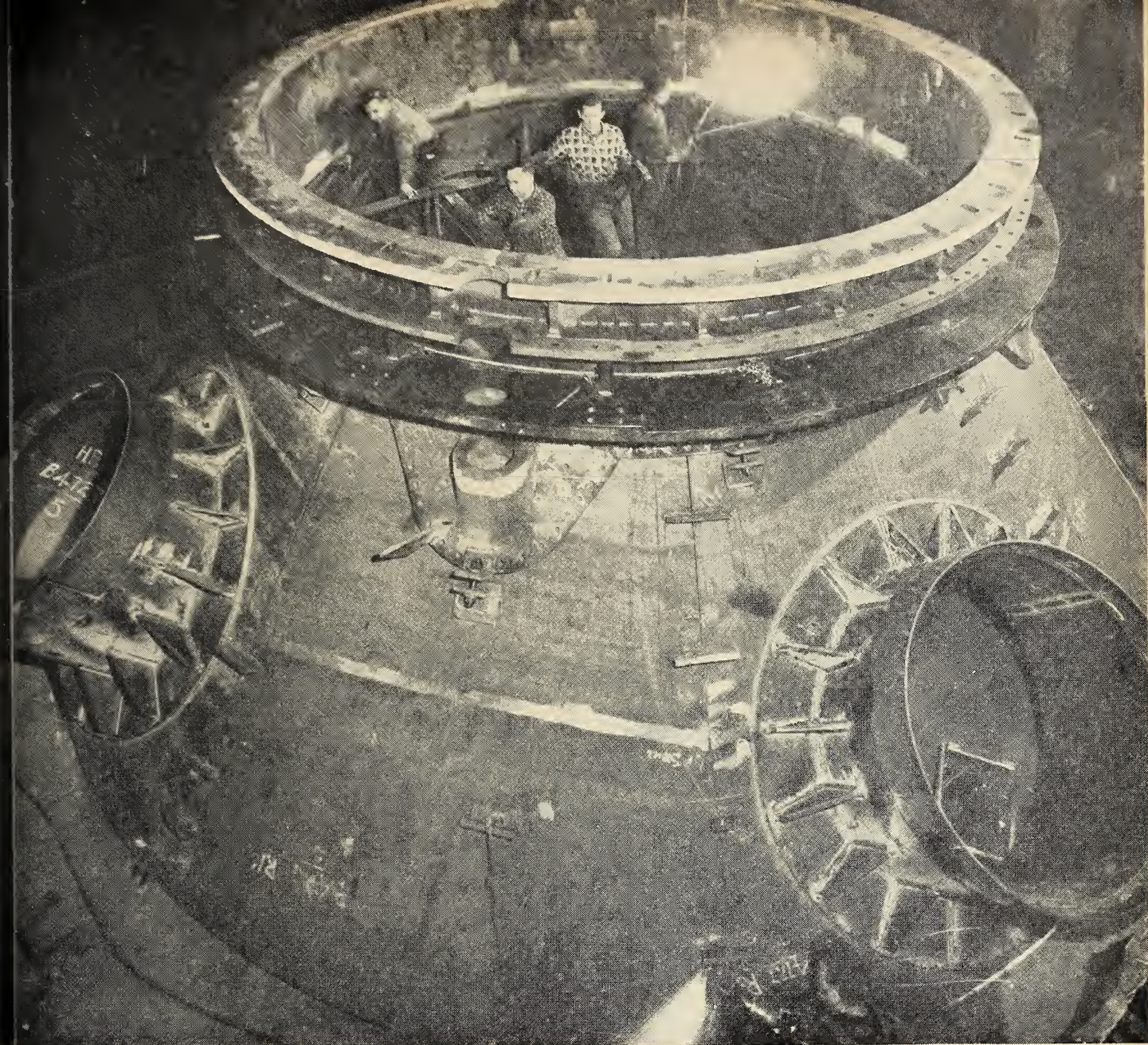
...ing a ring casting to top cone section of blast furnace. Furnace shell is 76 ft. high ranging in diameter from ... at the bottom to 14 ft. 9 ins. at the top. It was made in Montreal.
