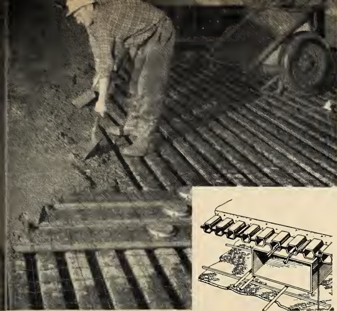
Light gauge steel cellular floor is covered with thin layer of concrete. Material is available in several shapes and sizes to suit span and service requirements. Cellular floors can provide built-in air conditioning duct, and raceways for electrical services, etc.
