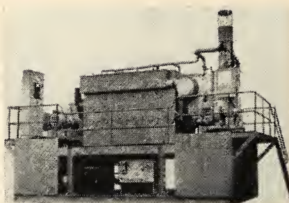
Sea Water Distillation Plant For Arabia Designed To Produce 25,000 Gallons Daily
