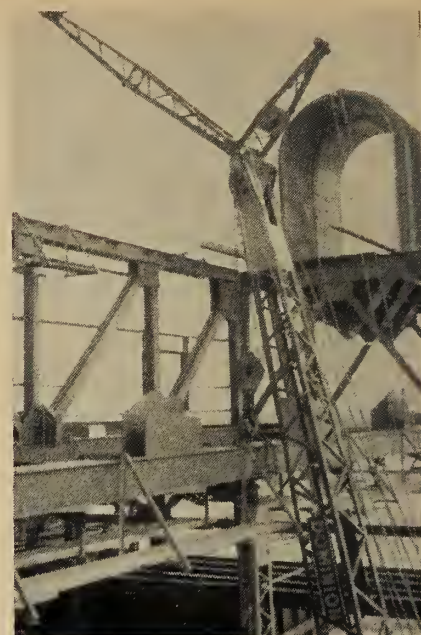
Fig. 3. Crawler boom section is used as falsework under cross flue trusses.
