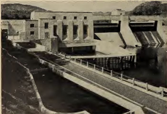
Pitlochry Dam and Power Station, Tummel-Garry Hydro-Electric Scheme.
