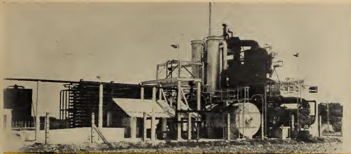
Sulphur burning sulphuric acid plant (20 tons per day) for Shaw Wallace & Co. Ltd. in India.
