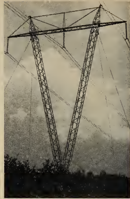
Fig. 9. Guyed aluminum tower—76 ft. to crossarm.
