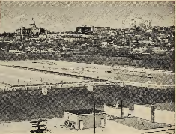
Modern water filtration plant at Edmonton, Alta., supported on "CCC" timber piling — shown at top during installation.
