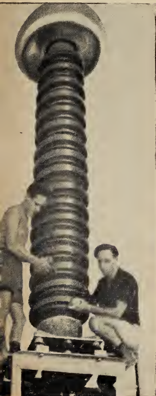
Fitting a high oil-pressure cable-end cap.
