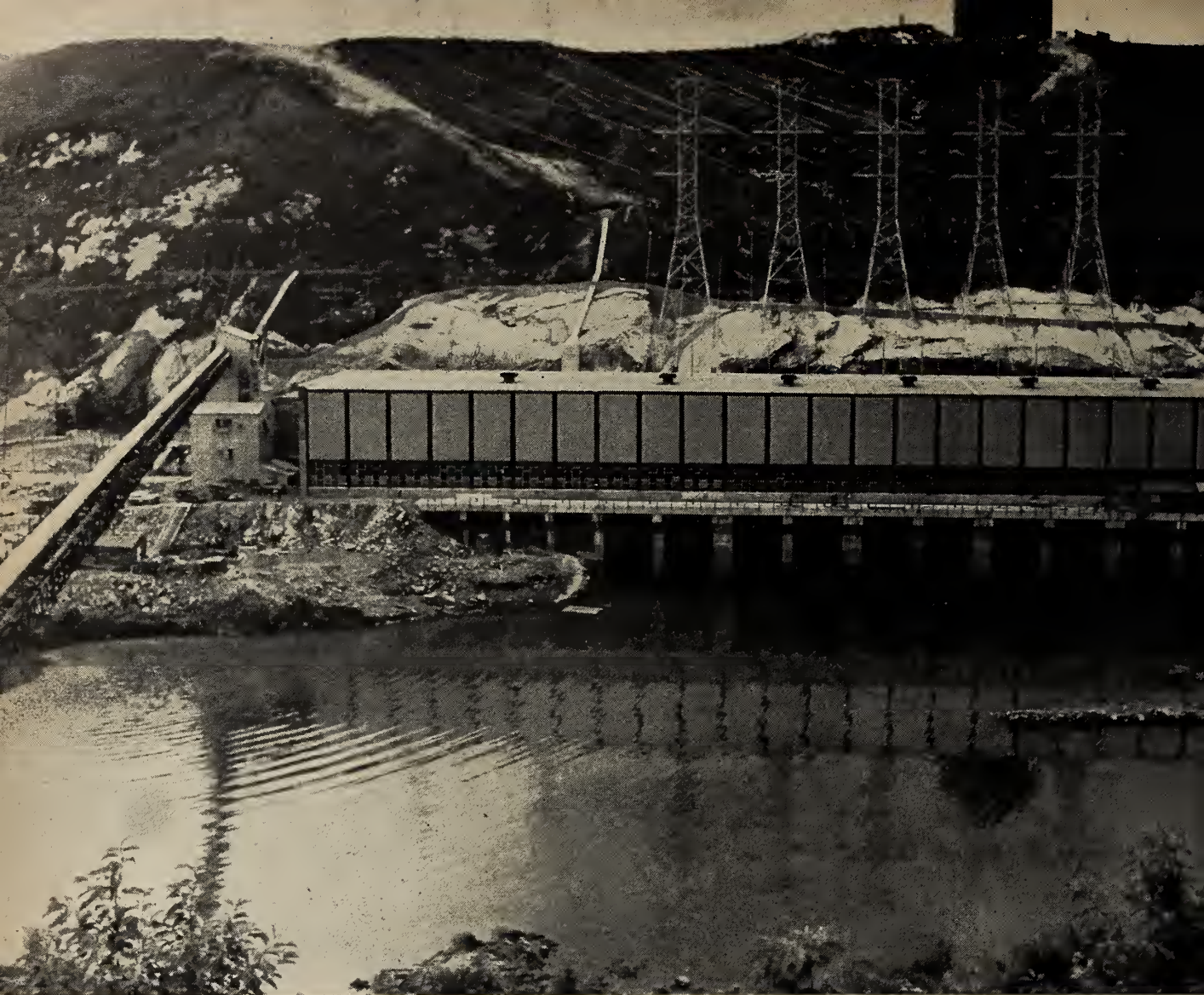
All 5 generators at Bersimis No. 2 are C.G.E. Three are already "on-line". This station is logically a second stage development of Bersimis No. 1, although a separate station with its own storage lake and transmission lines.
