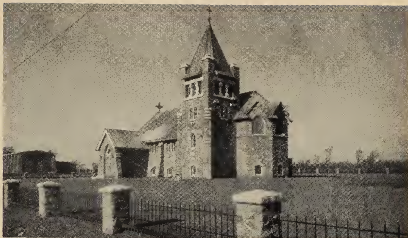
Fig. 7 Trinity Church as it was rebuilt using salvaged material. Note even the stone and iron fence has been relocated.
