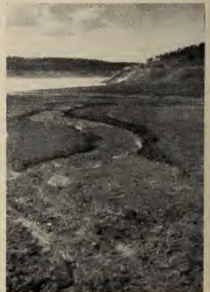
Fig. 5 Excavated silt flowing after being dumped from dragline bucket
