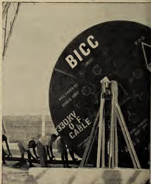
A length of 330,000 volt cable being drawn off the drum.
