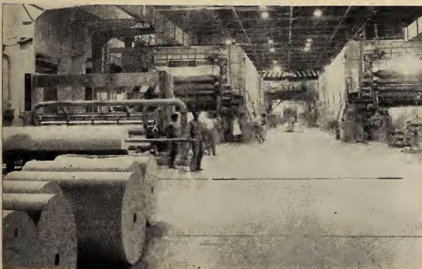
Fig. 4. General view of the Paper Machine Room.
