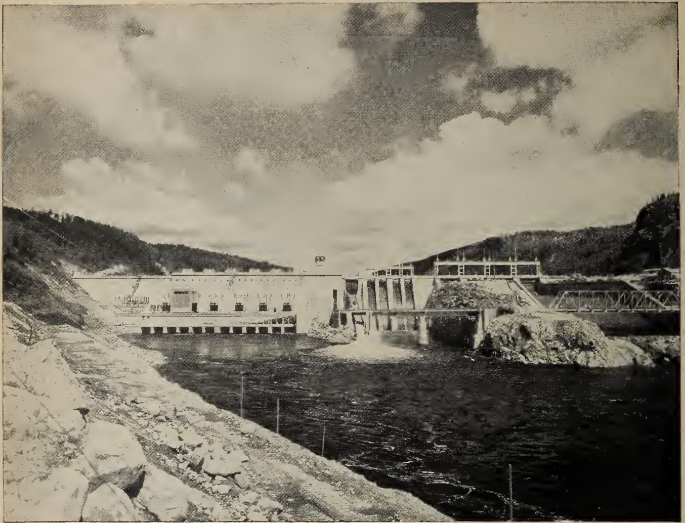
General view of power development looking upstream
