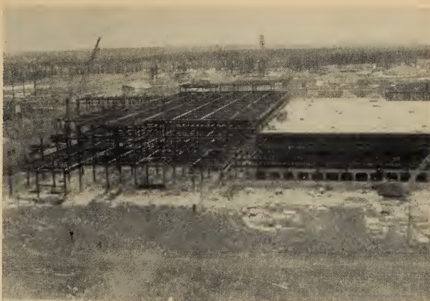
Fig. 4. Erection of Refinery Steel during the fall of 1959.
