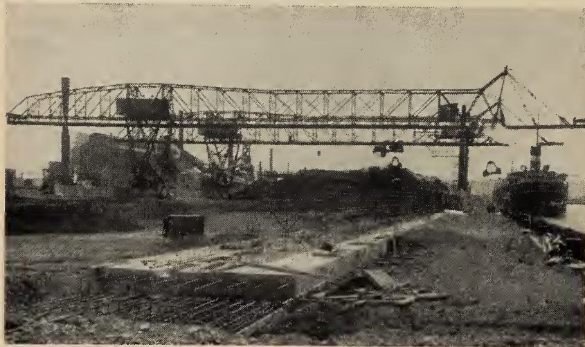
Fig. 2. View of two bridges unloading a boat and stocking. Construction of recent extension to bridge runway in the foreground. Sinter plant is at the left.
