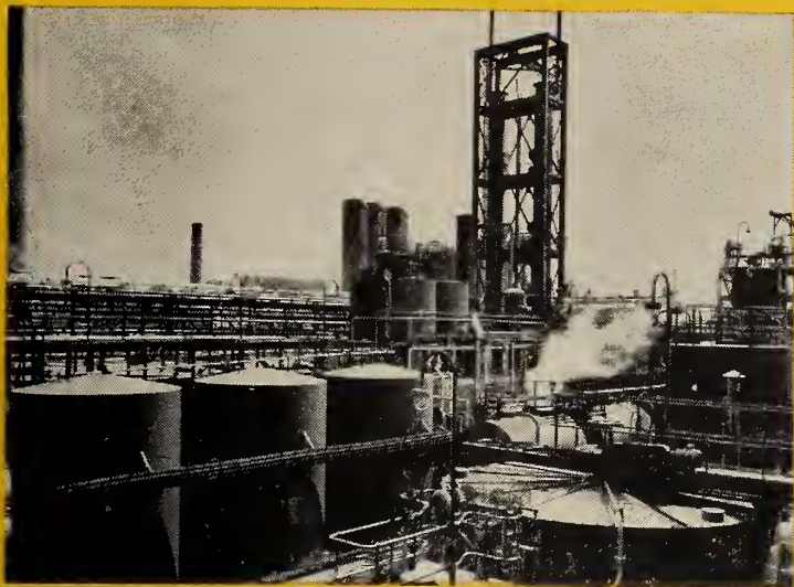
Tar acid plant, part of a complete tar works for National Coal Board, Chesterfield, England.
