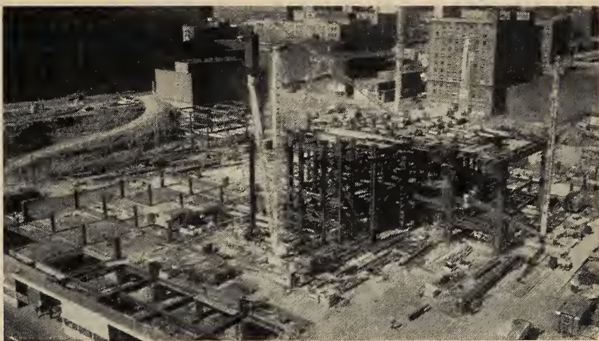
View Looking North
