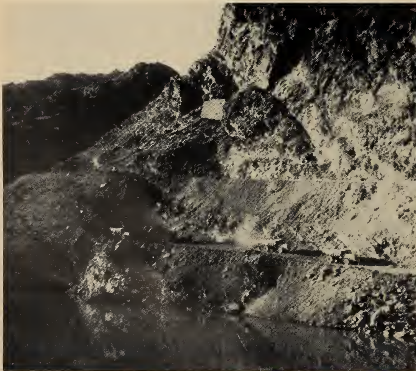
Fig. 5. Excavation for Diversion Tunnel outlet portal
