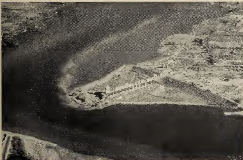
Fig. 3. Iroquois dam just before flooding of first stage (October 11, 1956).
