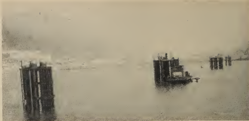
Fig. 8 Complete Installation of Mooring Dolphins
