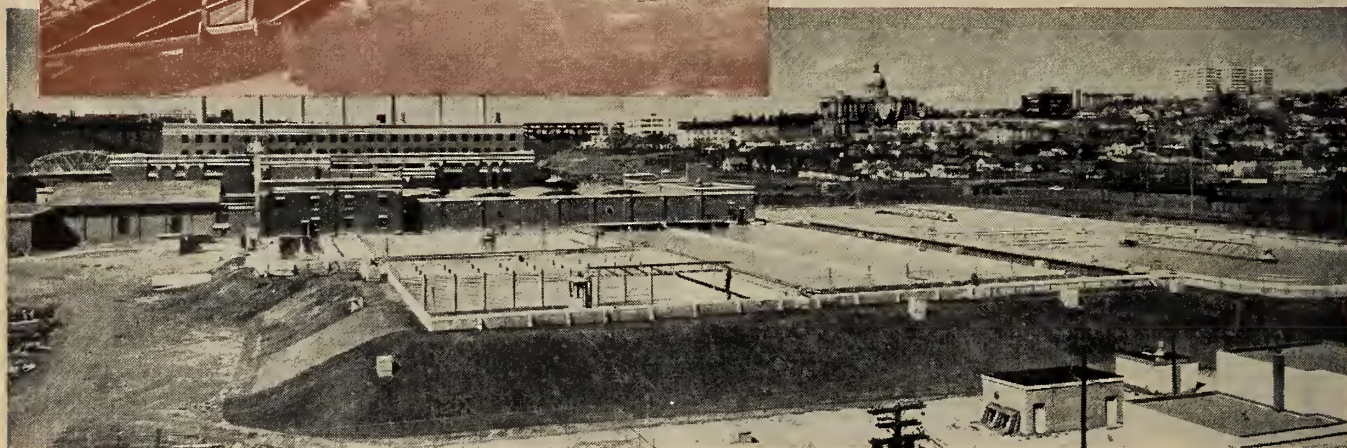
Modern water filtration plant at Edmonton, Alta., supported on "CCC" timber piling — shown at top during installation.
