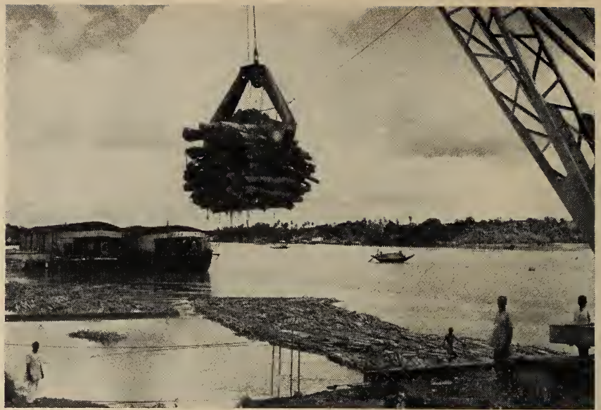
Fig. 3. Log bundles being hoisted from the river at the Khulna, East Pakistan pulp and paper mill, designed and constructed by Canadian firms.
