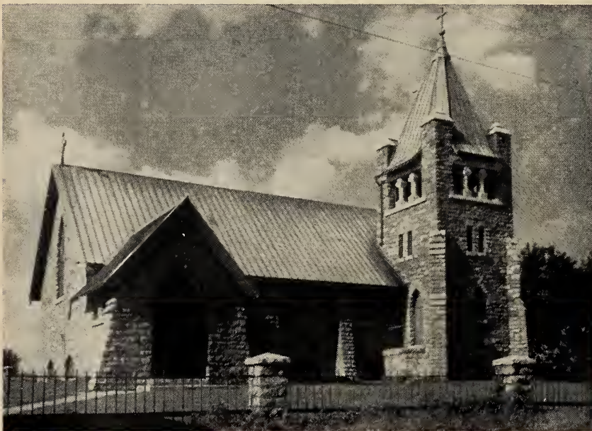
Fig. 6 Trinity Anglican Church, Riverside, before dismantling.
