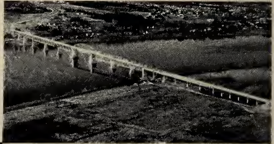
The Princess Margaret Bridge at Fredericton, N.B.
