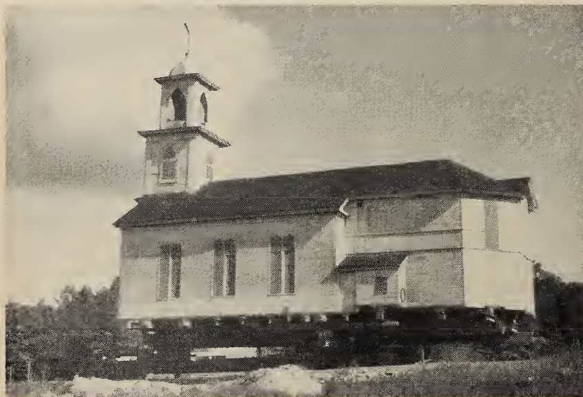
Fig. 3 Moving historic church on house moving trailer. Note extra "dollies" at rear to distribute load. This church was moved approximately 15 miles.
