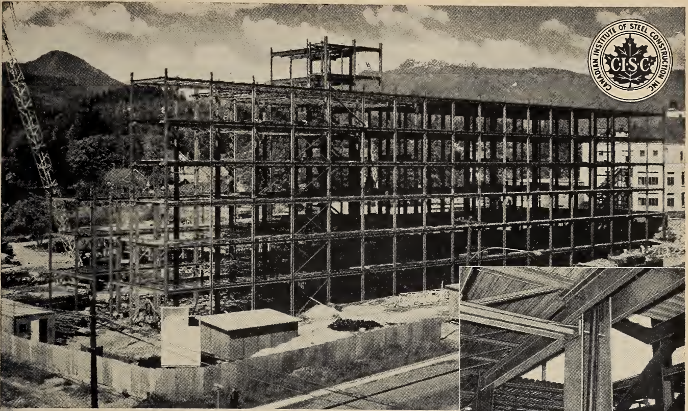
BESIDES PROVIDING continuous shallow depth floor girders, twin channels placed on opposite flanges of the columns allow more efficient positioning of vertical pipe runs.
