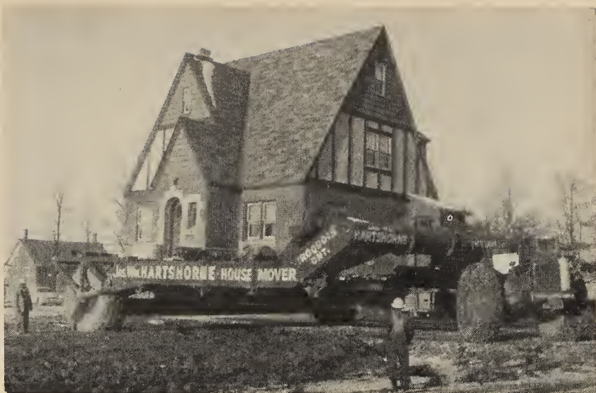
Fig. 4 Brick home in Morrisburg being moved by Hartshorne mover.
