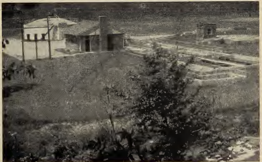
Fig. 4 The Streetsville plant built by the OWRC is a good example of a small plant producing a clear effluent.
