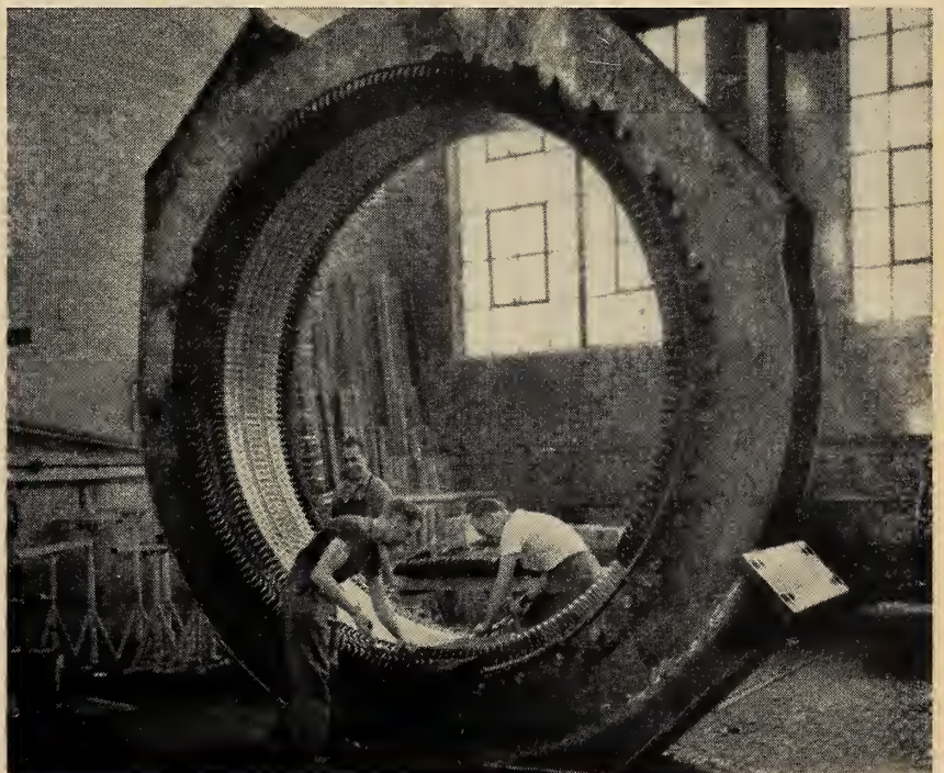
Fig. 3. 4500 hp., 0.8 pt., 272 r.p.m. 6000/3/50 engine type synchronous motor (showing stator being wound).
