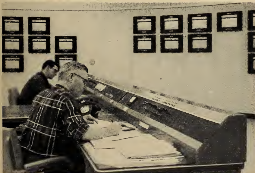
Fig. 4. M.H.E.B. load despatch office telephone duplex switchboards.
