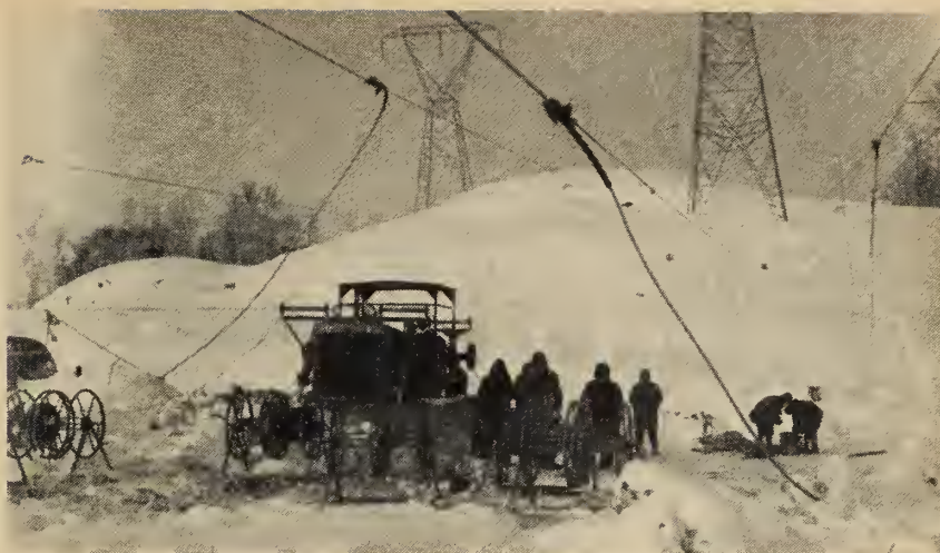
Fig. 7. Mid-winter stringing operations.
