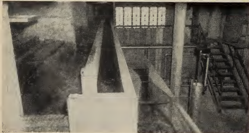
Fig. 4. Effluent end of manure settling tanks and the flow measuring and sampling equipment
