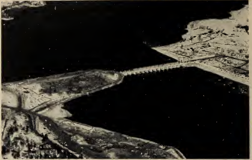
Fig. 4. Iroquois dam with cofferdams for second stage complete (February 5, 1957).
