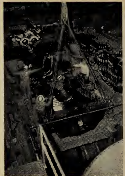
Fig. 4. A gas turbine unit during erection
