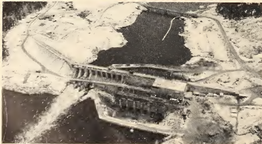
Fig. 5. Whitedog Falls second stage unwatering.
