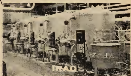
Boiler Feed Softening: Oil Refinery
