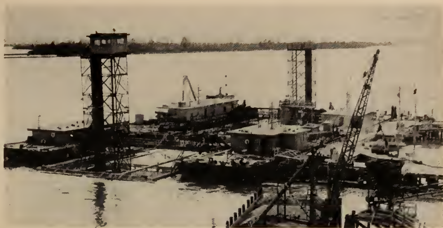
Fig. 15. Preparations for sinking.
