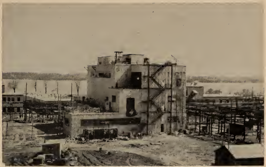
Fig. 2. Photo of completed Bldg. 216.
