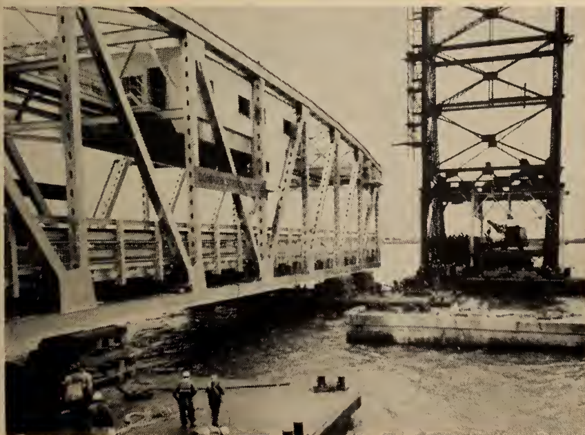
Fig. 15. Floating span into place at the Valleyfield bridge.
