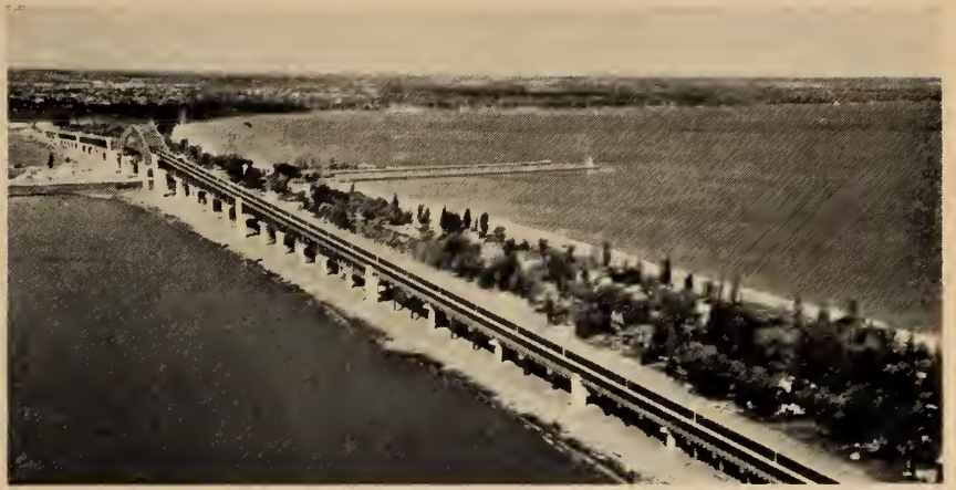
Burlington Bay Skyway, near Hamilton, Ontario, a 4½ mile long elevated highway. This four-lane skyway eliminates a major traffic bottleneck on one of Canada's most heavily-travelled roads.
