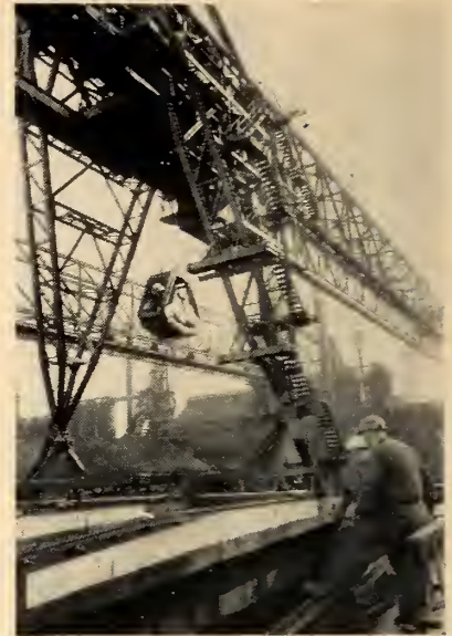
The new ore bridge of Algoma Steel Corporation, Limited has a bucket capacity of 22½ tons, making it one of the largest of its type in existence. Large bucket capacity and the fast operating speed of the bridge have reduced ship unloading time.
