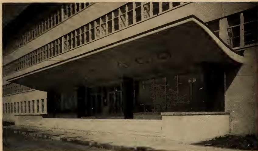
Fig. 3 - The torsion supported concrete canopy over the front entrance.
