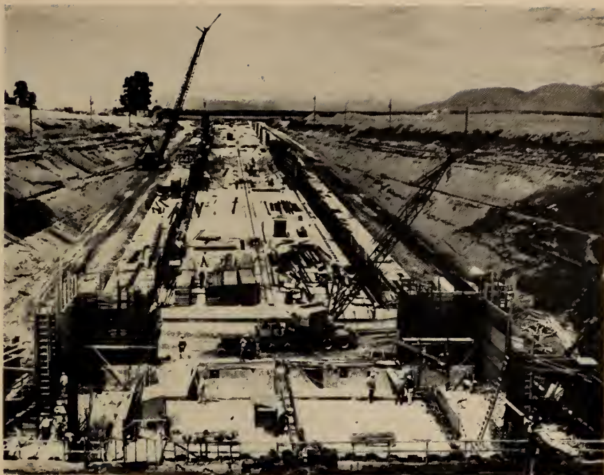
Fig. 10. Lulu Island approach during construction.
