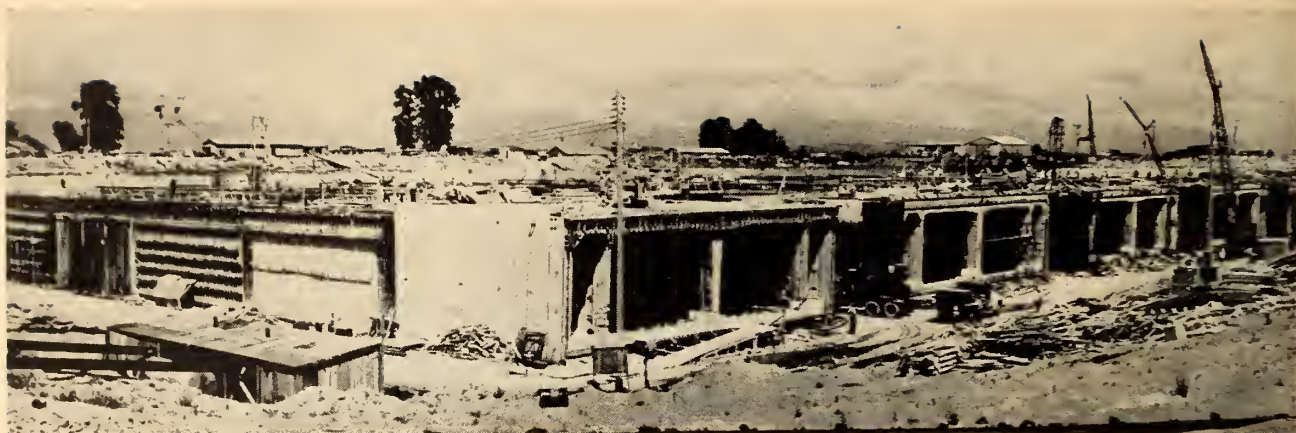
Fig. 11. Tunnel elements during construction.
