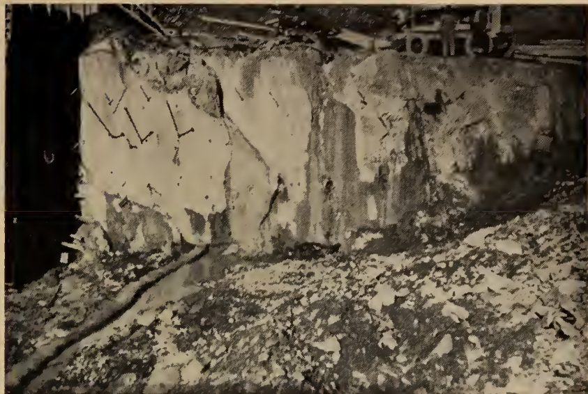
Fig. 7 Near Vertical Rock Face on Completion of Excavation
