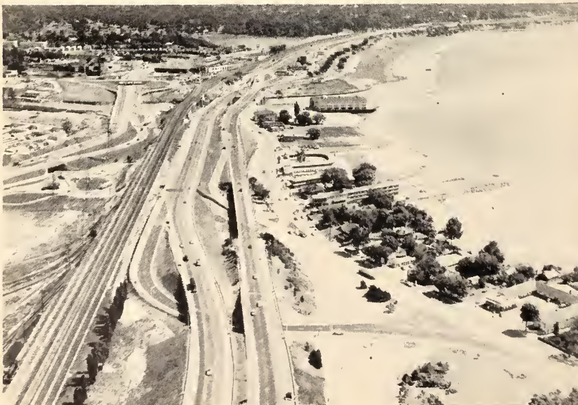
Part of the Frederick G. Gardiner Expressway. Shown are the Humber River bridges, T.T.C. underpass and C.N.R. overpass, constructed by Foundation Company for the Department of Highways of Ontario. The Municipality of Metropolitan Toronto, Toronto Transit Commission and Canadian National Railways, Consulting engineers were Lakeshore Expressway consultants and Canadian National Railways.
