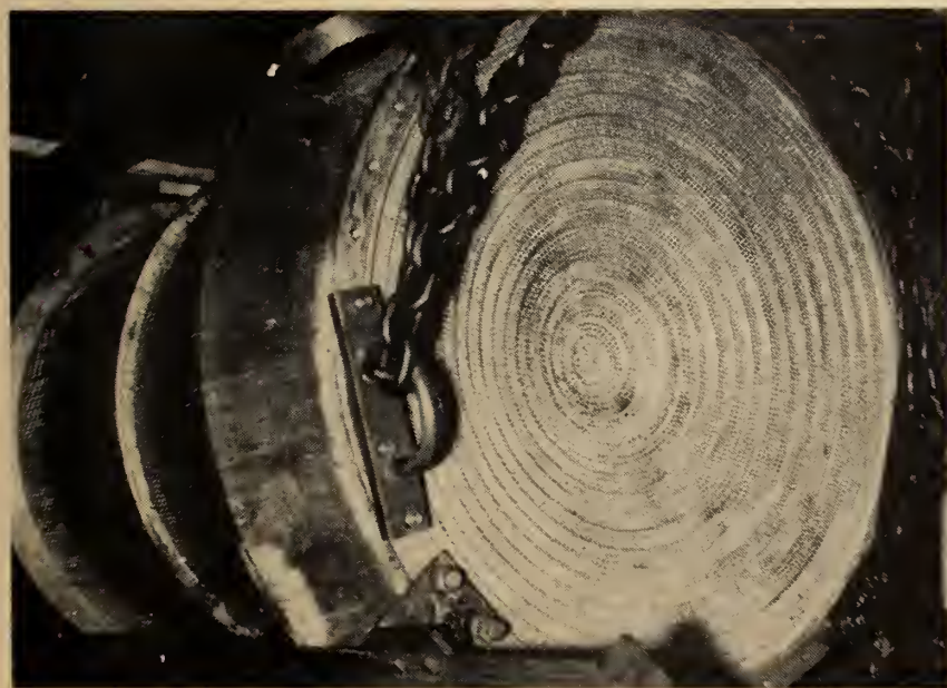
Fig. 5. MP column overhead condenser tube nest.
