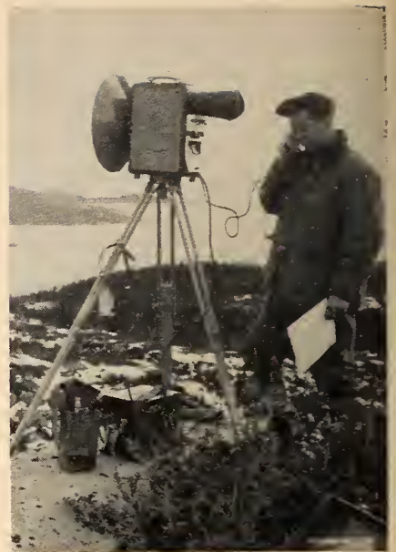
Fig. 7. A field crew on location in Northern Quebec using the Tellurometer, electronic instrument for distant measurement.
