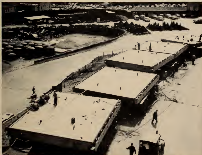
Head Gates for Beauharnois Hydro-Electrical development, Beauharnois, Que.
