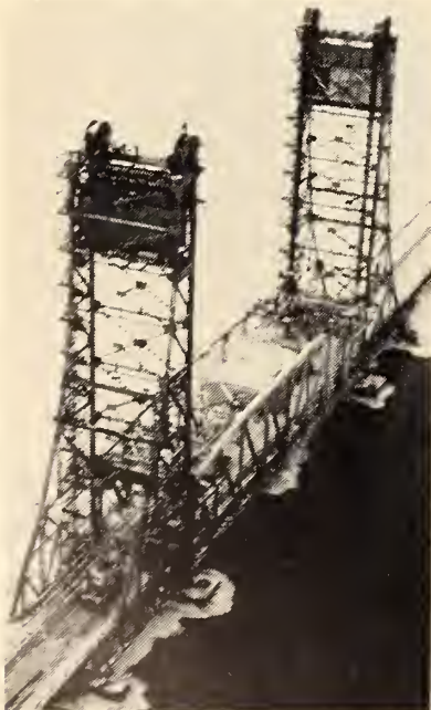
Fig. 6. St. Louis lift bridge which replaces two spans in the north end of the St. Louis bridge.
