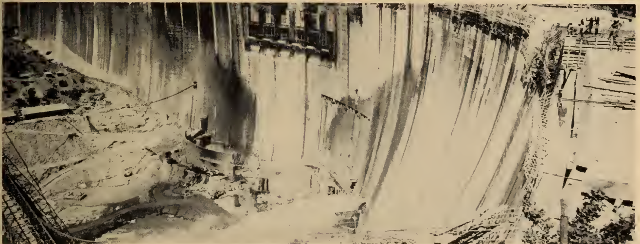
KARIBA HYDRO-ELECTRIC PROJECT, ZAMBESI RIVER, RHODESIA
