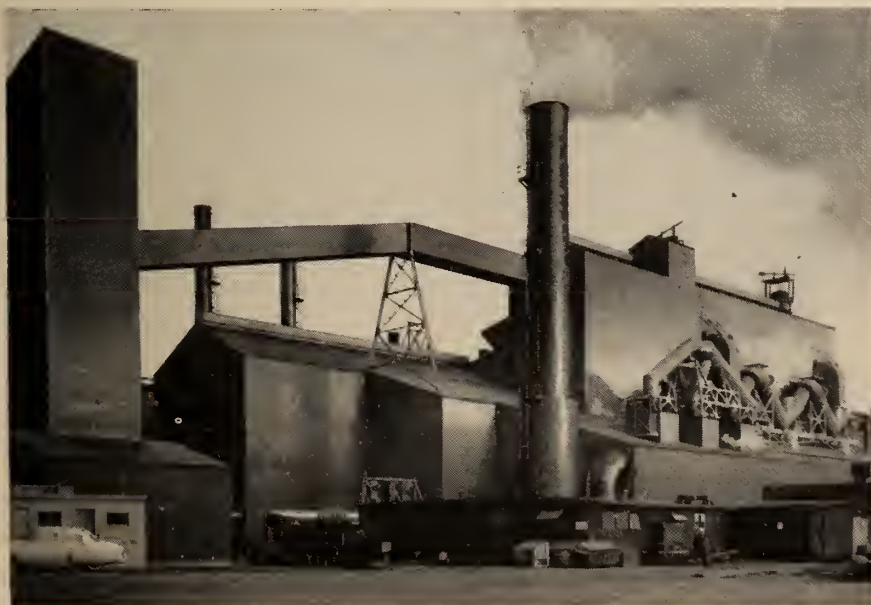
Two L-D Oxygen Steel-making furnaces at the Algoma Steel Corporation, Limited are housed in the large building shown here. It is equivalent to a 10-storey structure spread over the length of a city block.
