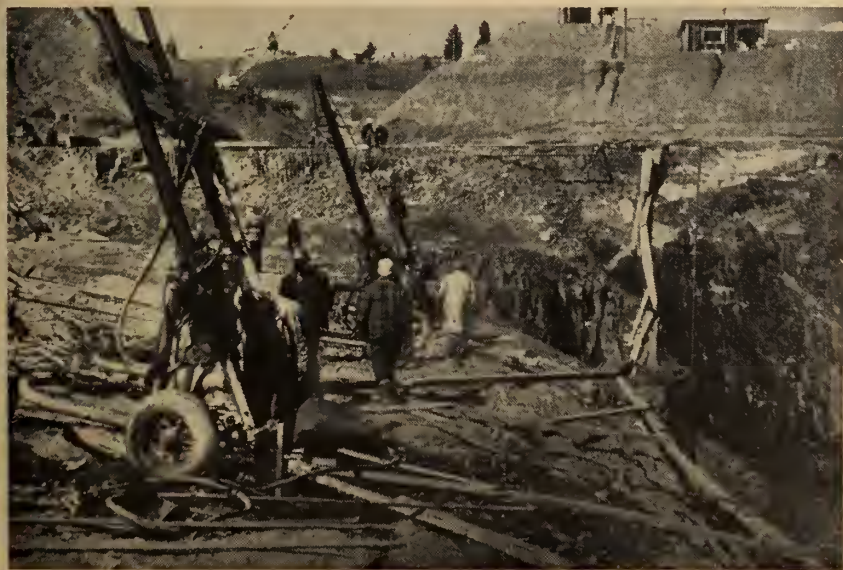
Fig. 8 Drilling for Blanket in Intake
