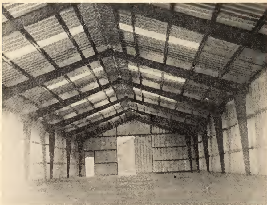
Fig. 1. Photo of Kingston Bldg. 5 completed.
