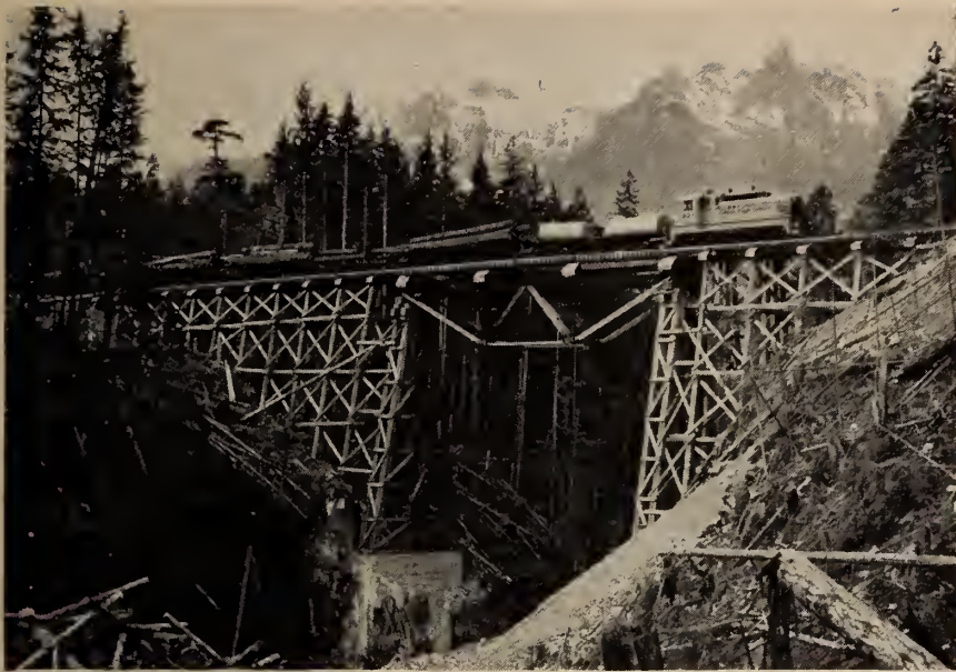
By means of a new 23-mile railway extension from Nimpkish, Vancouver Island, Canadian Forest Products Ltd., can haul logs to Beaver Cove. From there the logs are towed in booms to the company's processing plant at Vancouver. One of the nine major bridges on the new extension is shown above.
