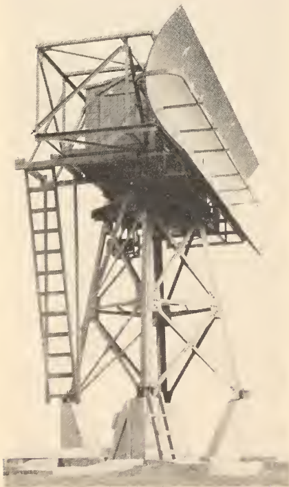
Fig. 15 Aerial of the first Canadian designed and built micro-wave radar
