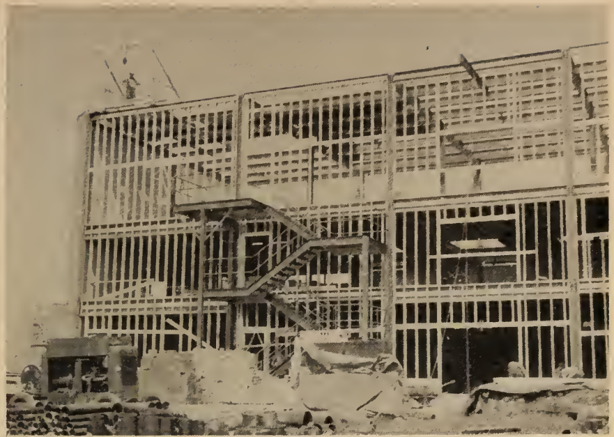
Fig. 7. Photo of Kingston under construction.
