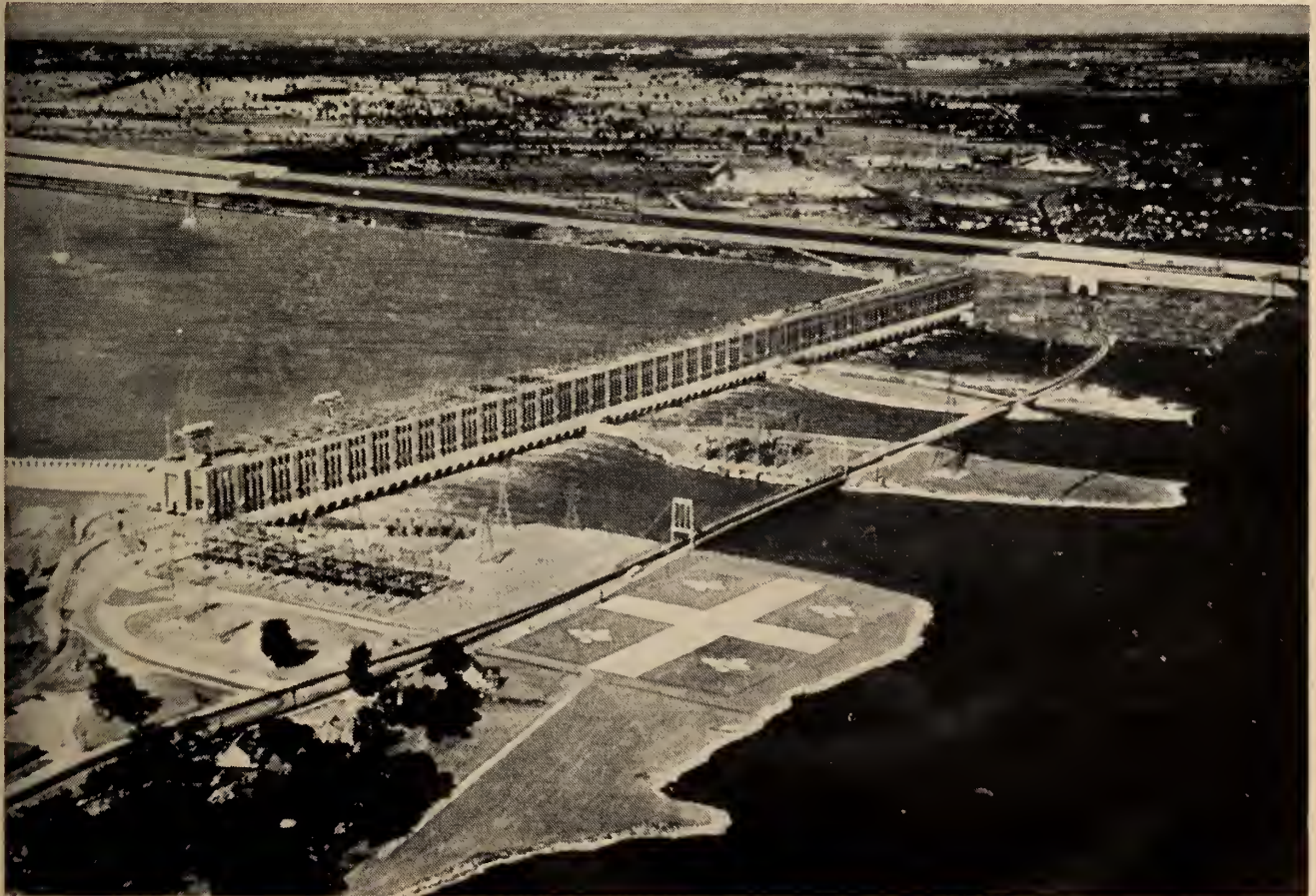
Fig 2. Aerial view—powerhouses 1, 2 and 3
