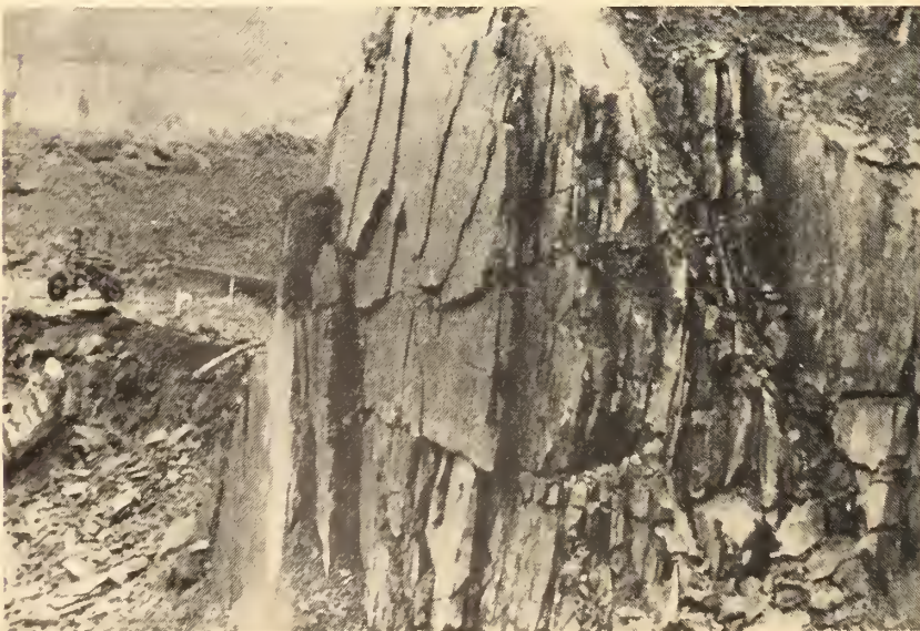
Fig. 6 Bedrock Cleavage during excavation
