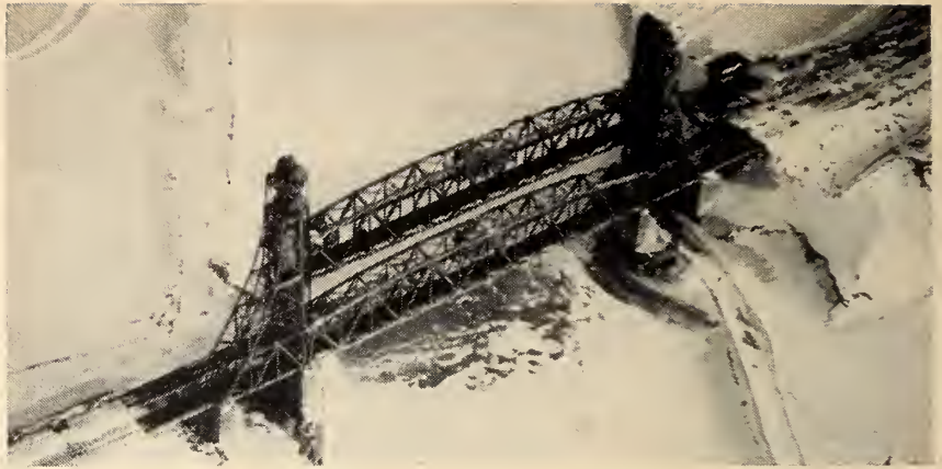
Fig. 5. Caughnawaga twin lift bridge which provides flexibility of railway operation. Cross overs were provided between the two tracks approaching from either side so that if one span is damaged all trains can use the remaining span.
