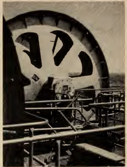
Fig. 7. Counterweight sheaves with integral trunnions fabricated in welded steel.
