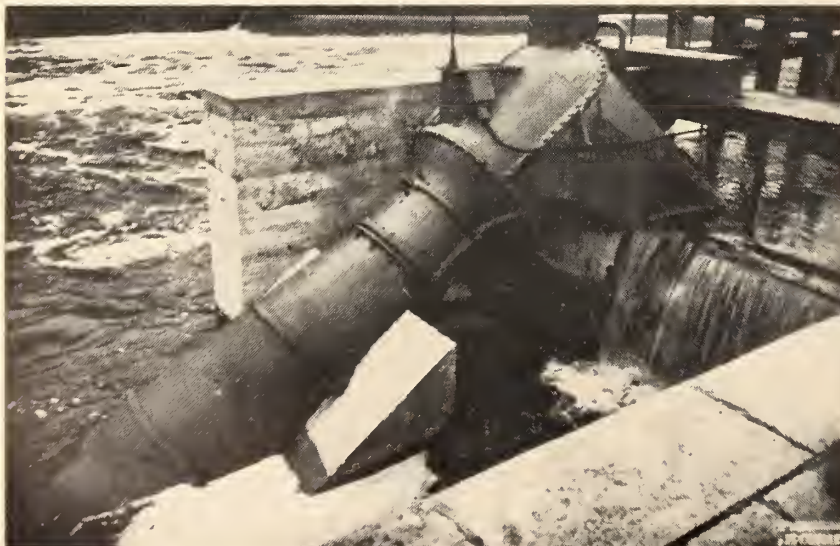
54-kw. package power plant — “La Maignannerie” — on the Mayenne River (France).
