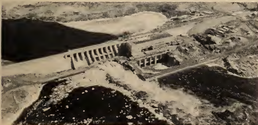
Fig. 7. Caribou Falls second stage unwatering.
