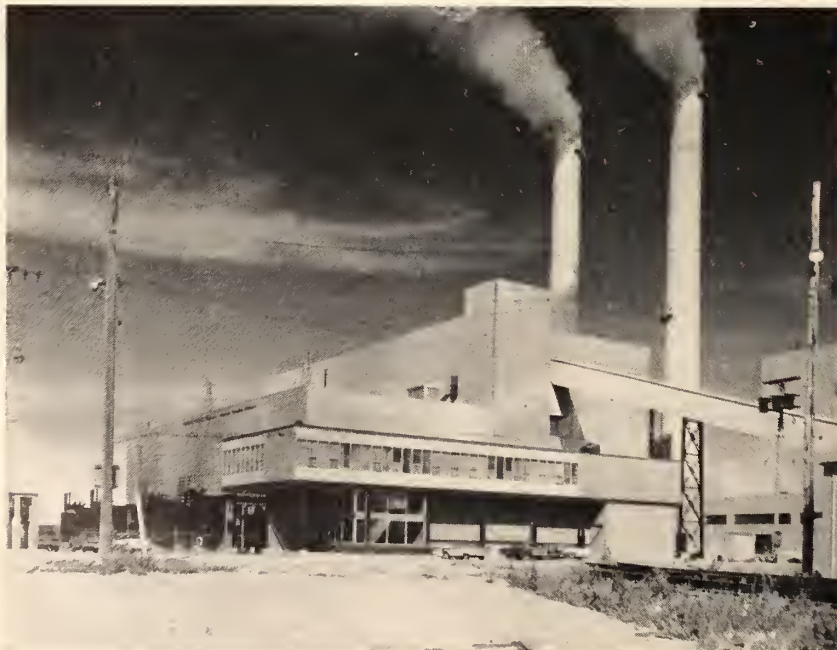
Fig. 1a. General appearance of office section and south side of Brandon generating station.
