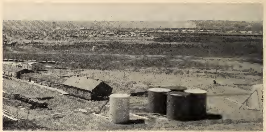
Fig. 1. View of general area of site before commencement of foundation preparations.
