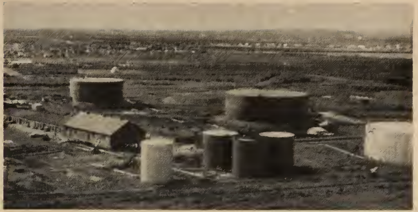
Fig. 7. View of site near completion of construction of new tanks, in middle distance. Between tanks and at extreme right of photograph can be seen preloading fill for two tanks to be constructed in 1959. The wellpoints have been discontinued at the larger of the two tanks and water can be seen at the ground surface.
