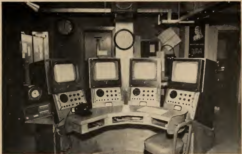
Fig. 7. Master Control Monitoring Facilities.
