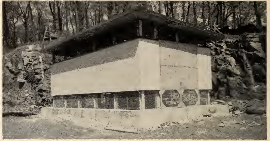
Fig. 4 — Outside storage tank of propane gas.
