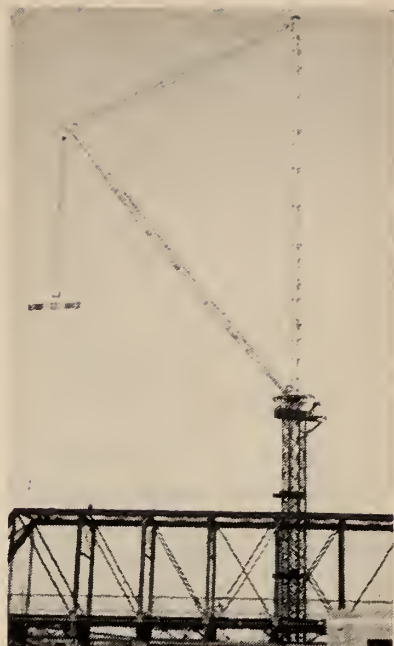
Fig. 10. 109 ton tower derrick used to construct the lower St. Lambert bridge.
