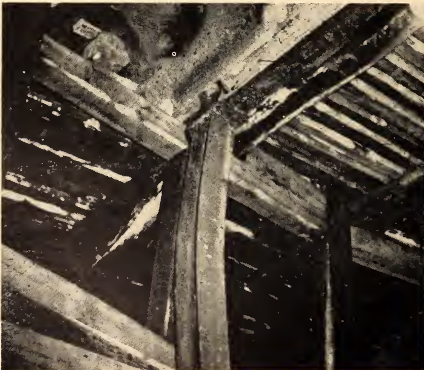
Fig. 5. Excavation maintained in a yielding rock.
