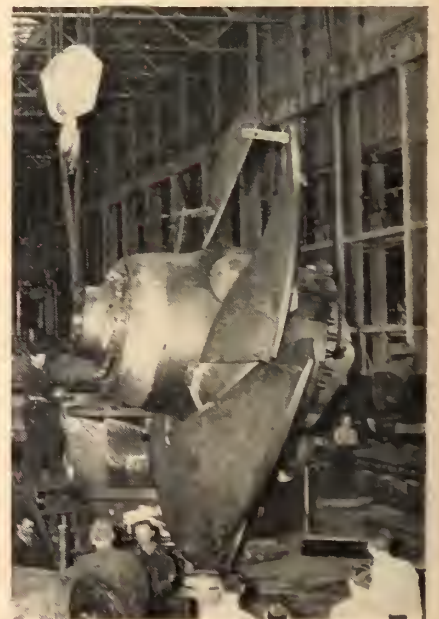
Turning runner in shop after installation of blades
