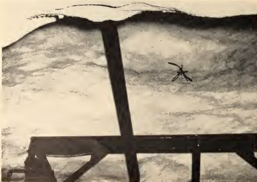
Fig. 3. An example of effective guniting at the McIntyre mine.
