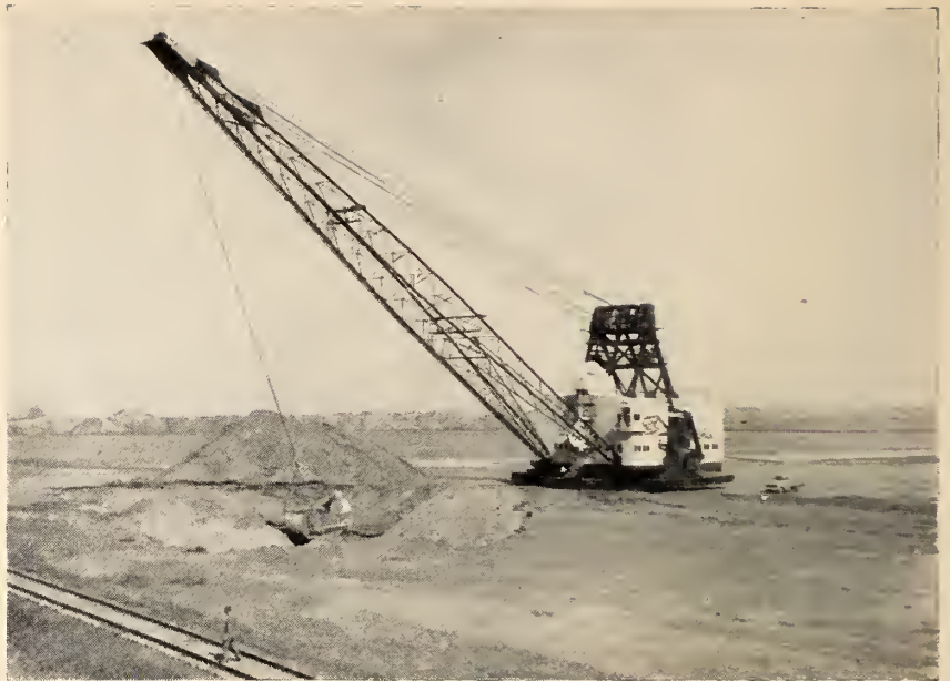
View of "Mr. Klimax" Marion 7800 dragline with its 35 yard bucket. A truck is parked beside the dragline showing comparative size.
