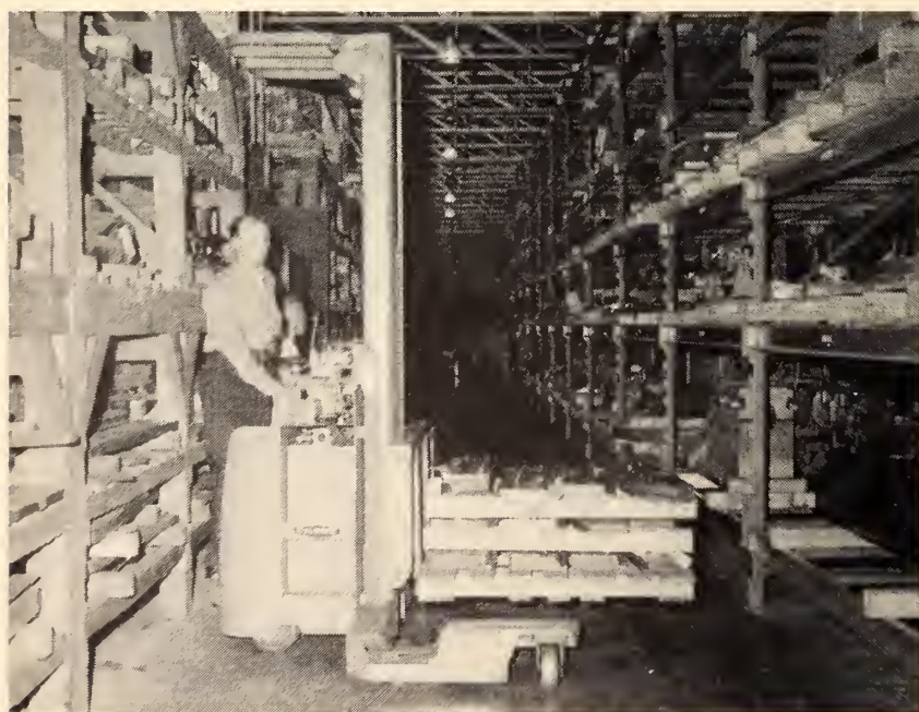
Fig. 8 Four-directional stacker with load preparing to move sideways down aisle. Note position of rotatable front wheel. Stacker can raise loads to a height of 15 feet.
