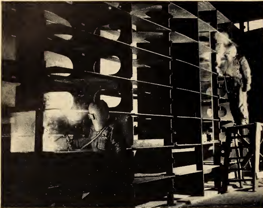
A pre-fabricated bottom section of a new ice-breaker for the Department of Transport being constructed with Liquid Air 6024 Mild Steel Electrodes at Marine Industries Ltd., Sorel, Que.
