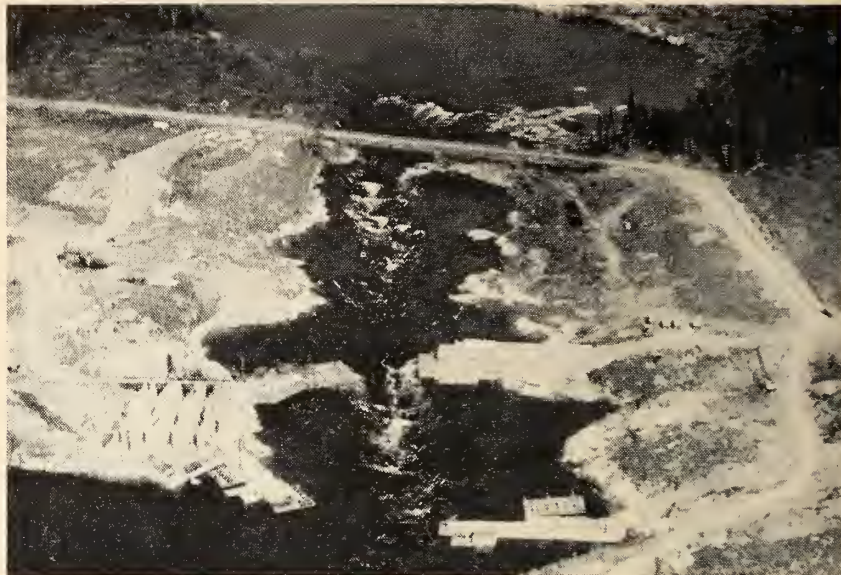
Fig. 4. Whitedog Falls first stage unwatering.
