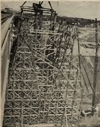
Fig. 12 Span 10 erection falsework.
