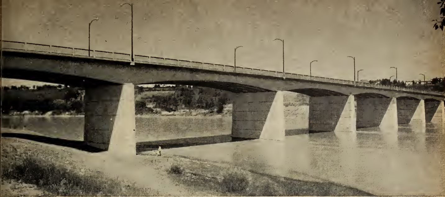
Groat Bridge, Edmonton, Alta.—Owner: City of Edmonton—Designer: Structural Engineering Services Ltd.—Contractor: Mannix-Burns & Dutton.
