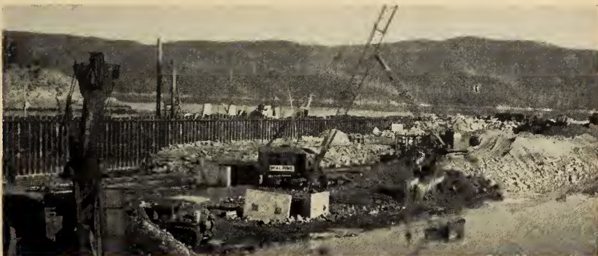
Fig. 8. General view illustrating placing of tie rods and fill material.
