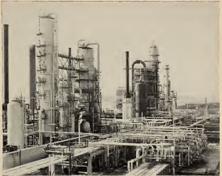
Central control facilities serve the a. and v. unit, cat. cracker, light ends recovery unit, and the cat. poly. plant. Figure 5 shows a section of the graphic panel which uses miniature
