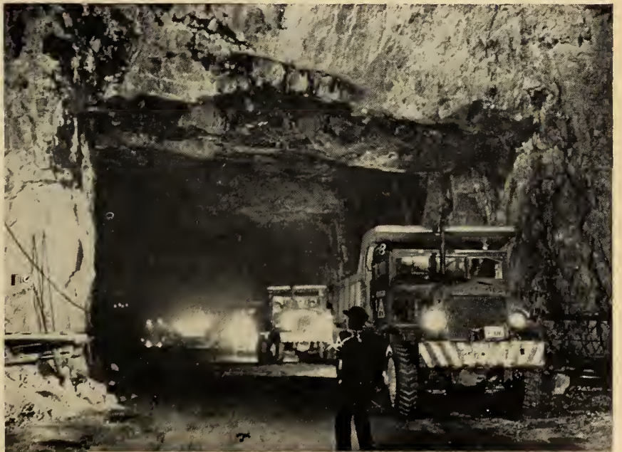
Fig. 9. McCormick Dam. View of trucks in unwatering tunnel. June 18, 1951.
