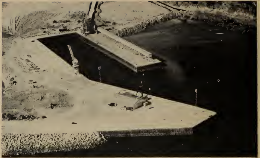
Fig. 13. Dock largely completed.
