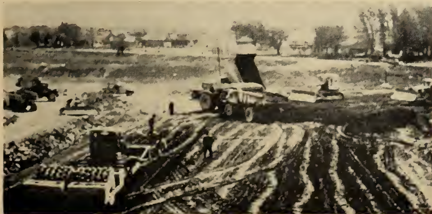
Fig. 6. Compacting glacial till in impervious core of dyke.
