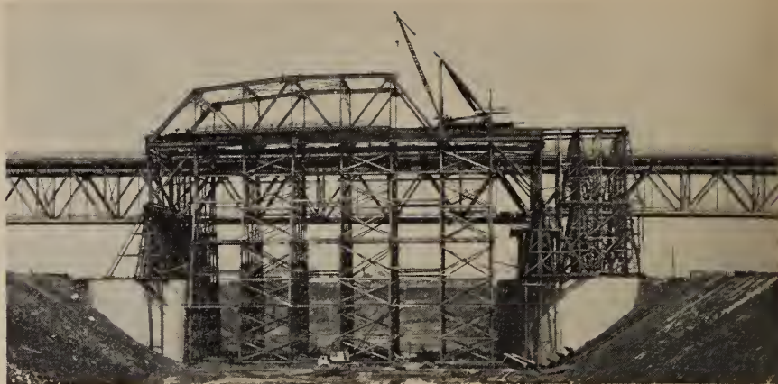
Fig. 13 Erection of new span 10.
