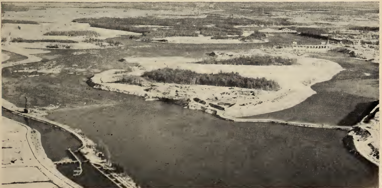
View of site after start of construction of cofferdam 'E'. Water ripples left of island indicate location of partially built cofferdam. Cut 'F' across Long Sault Island is also seen at right; upstream plug is still in place. Dickinsons Landing (lock 21) is at left. Long Sault Dam under construction in background at right. (PASNY)
