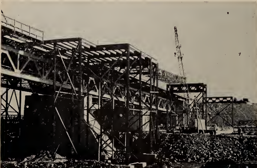
Fig. 5 Supporting steel for Bailey bridges and turnout.
