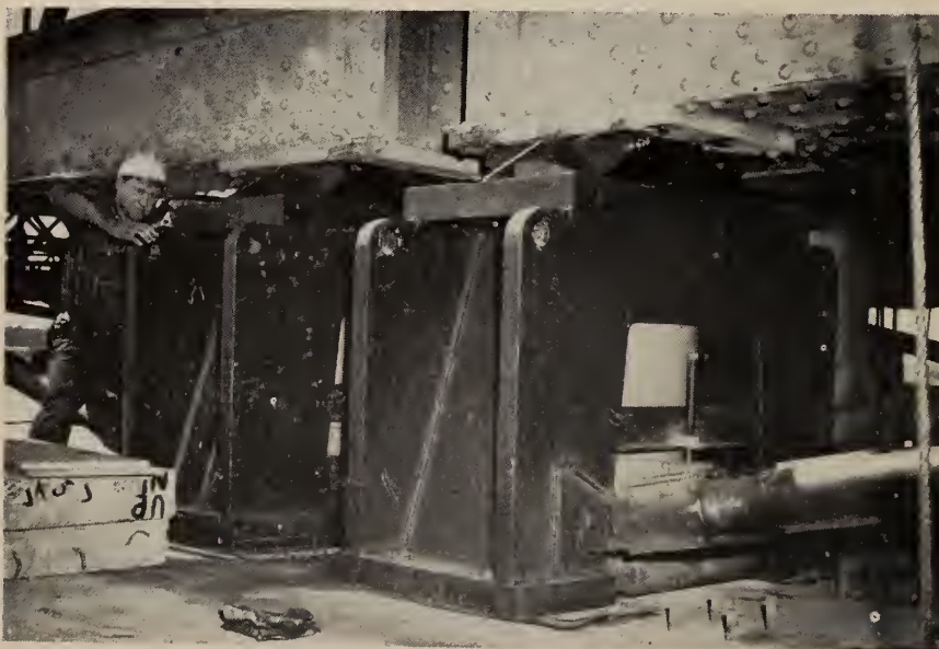
Fig. 10 Climbing jacks in place under the bridge trusses.
