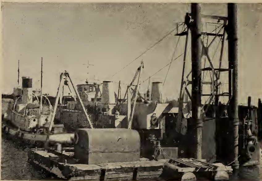
Fig. 14. Twenty-inch suction dredge and tug at anchor.
