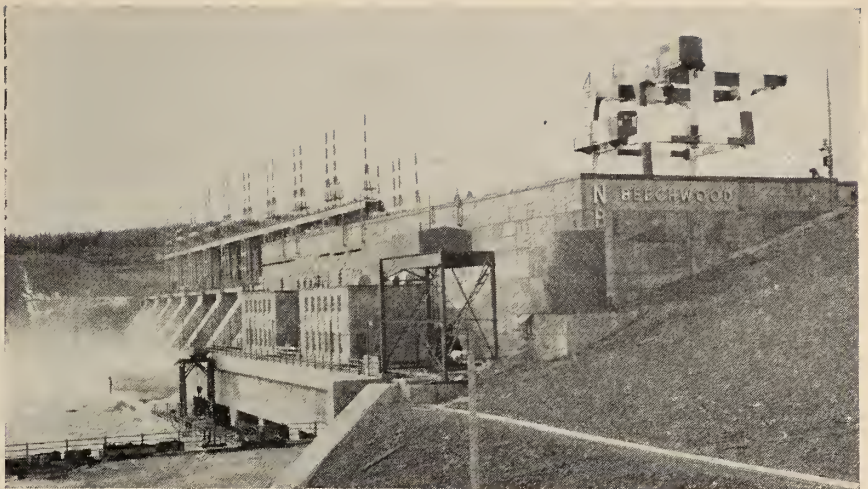
The New Brunswick Electric Power Commission's hydro-electric station at Beechwood.
