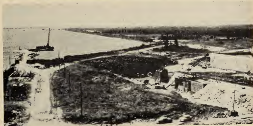
Fig. 10. Identical views of approach to Upper Beauharnois lock, looking west along power canal: (a) before work started; (b) before flooding to dredge out canal dyke.
