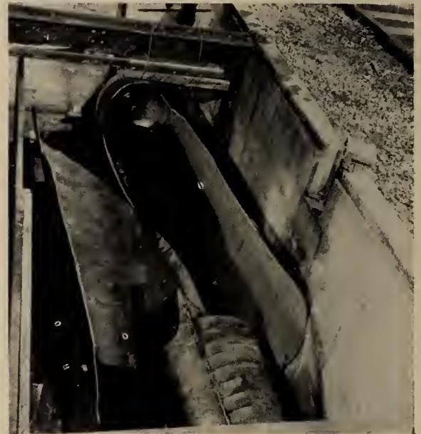
Fig. 13. Burst tested pipe C-1.
