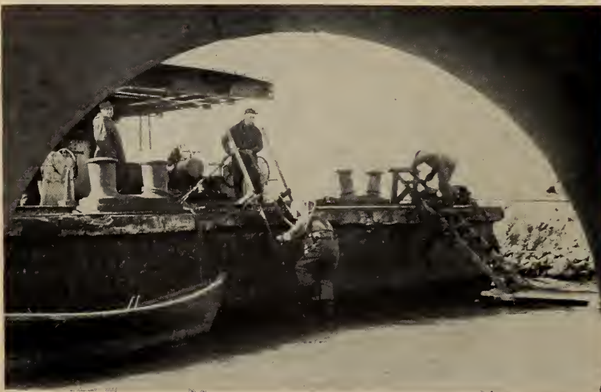
Fig. 16. Divers laying 7 ft. diameter salt water intake line 160 ft. into harbour.
