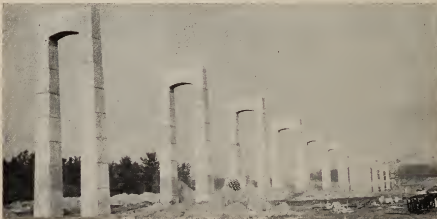
Piers for the substructure of the new high-level bridge across the St. Lawrence between Cornwall Island and Roosevelttown, N.Y.
