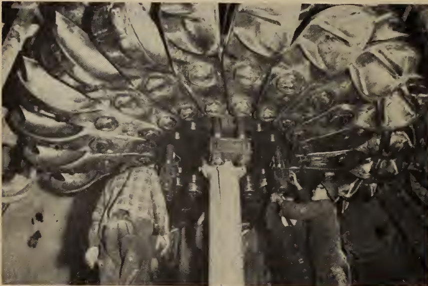
Fig. 15. Turbine No. 2 runner lifted into position.
