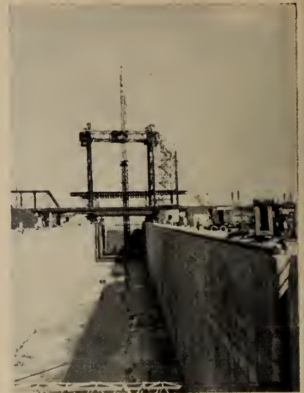
Fig. 10. St. Lambert lock completed. Victoria bridge lift span being erected.
