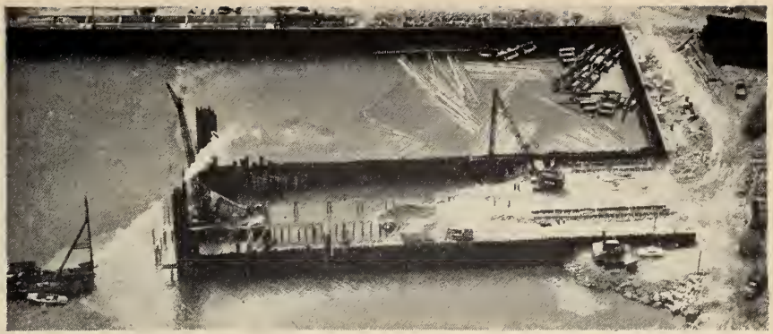
Fig. 11. Aerial view of jetty construction, June 1957.
