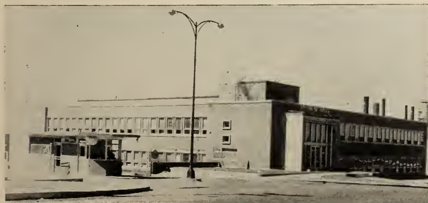
Fig. 14. Technical building housing laboratory, personnel, medical, administrative and technical departments.
