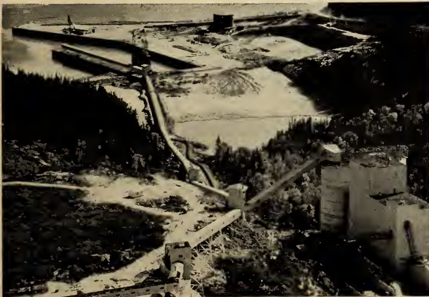
Fig. 8. Conveyor from wharf to silos.
