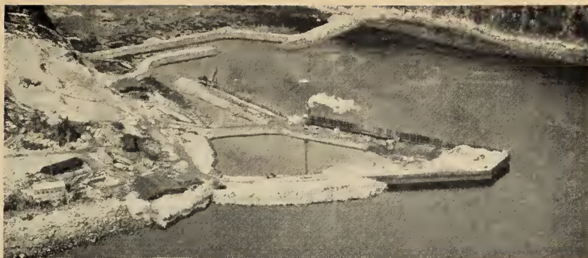
Fig. 7. Aerial view of dock construction, October 1956.
