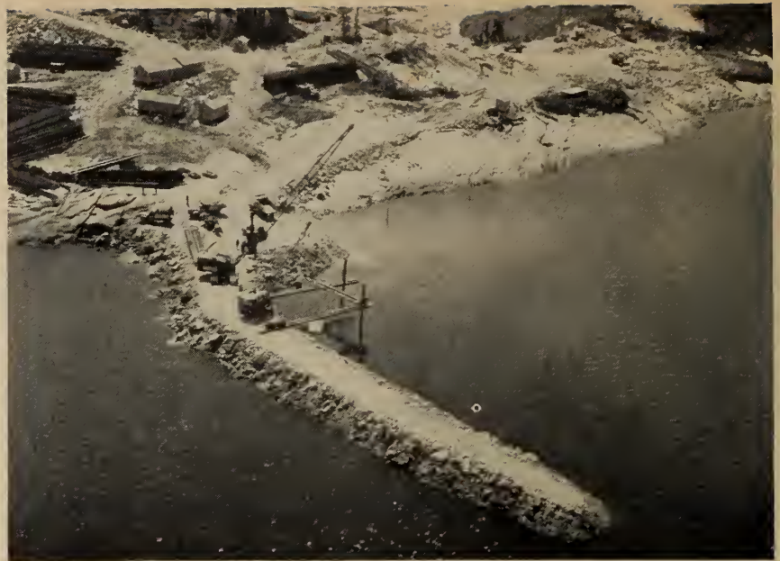
Fig. 5. Construction of breakwater.
