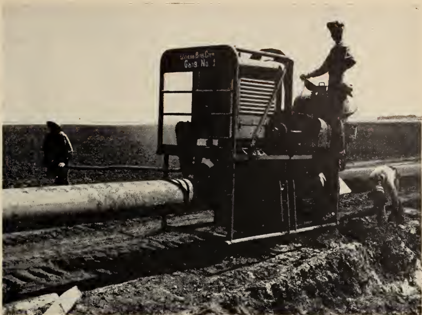
A view during construction of the Interprovincial Oil pipeline in Manitoba.
