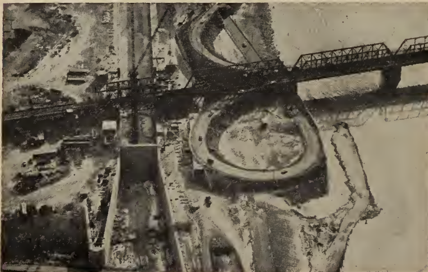
Seaway construction and traffic diversion, Victoria bridge, Montreal.
