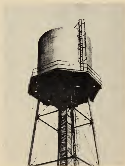
Fig. 9. Welded aluminum water storage tank (50,000 gallons) erected in 1948 at Shawinigan Falls, Que.
