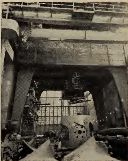
MODERN TREND IN CRANES. This completely enclosed 300-ton gantry crane—the largest ever built in Canada—was designed and fabricated by Dominion Bridge for the Canadian half of the St. Lawrence Power Project. Photo courtesy Ontario Hydro
