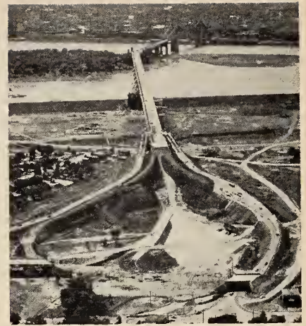
Fig. 1 Before and after view of bridge over channel.
