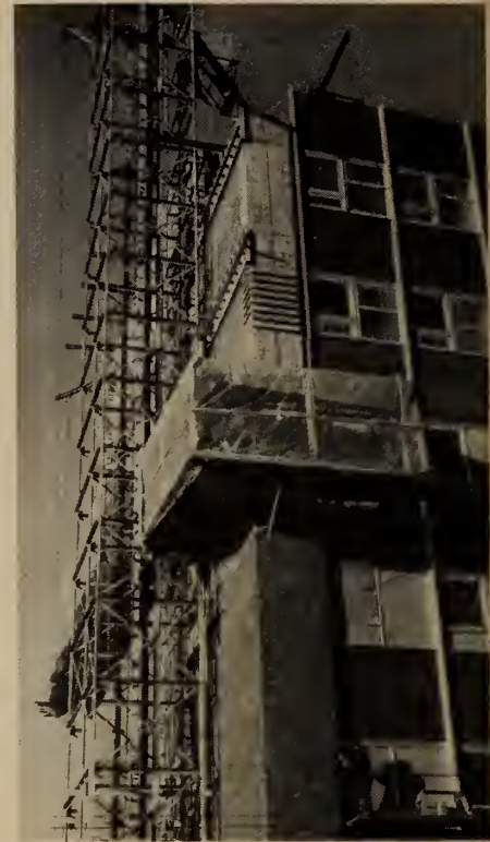
Fig. 3. Winter construction in Edmonton. Photograph: Goertz Studios
