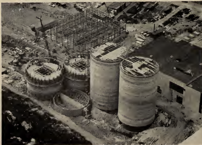
Fig. 9. Alumina silos under construction.
