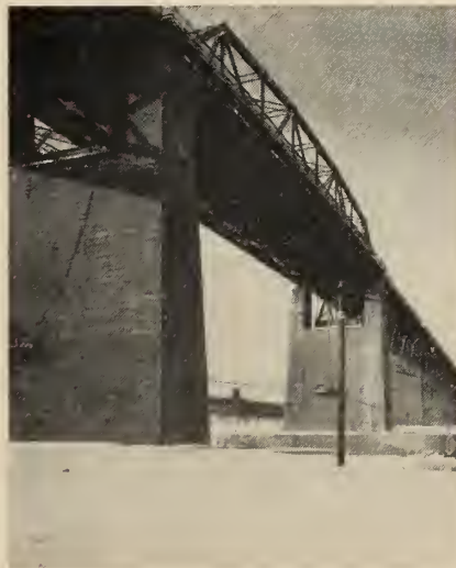
The completed span.
