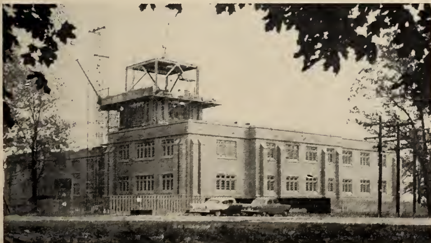
Engineering Science Building under construction at the University of Western Ontario.
