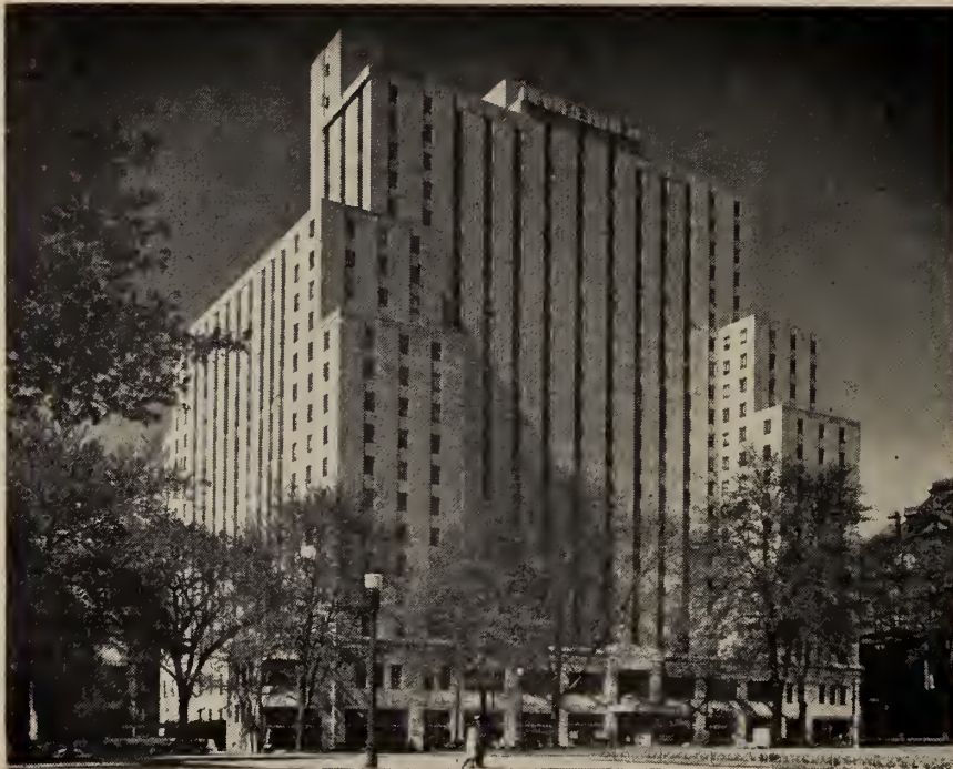
Fig. 1. The Laurentien Hotel, Montreal, Que., erected in 1946/47, was the first multi-story building on this continent to be faced with aluminum.
