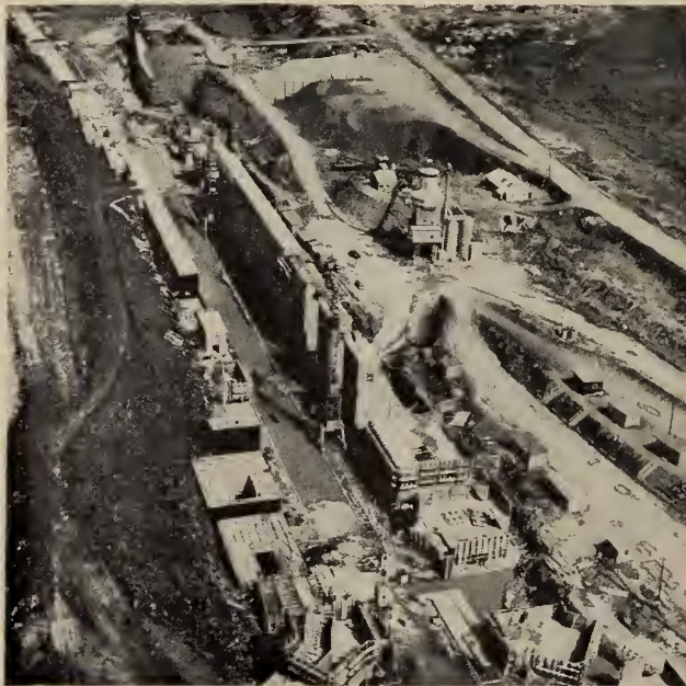
Fig. 11. General view of construction of Cote Ste-Catherine lock.
