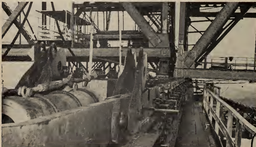
Fig. 15 Right: New Span on erection legs during translation.
