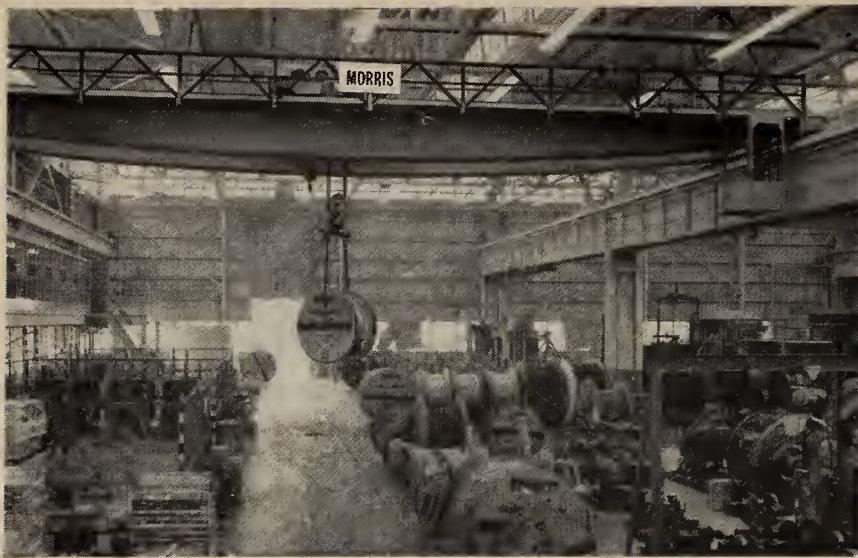
Photograph courtesy of Pirelli Cables, Conduits, Limited.
