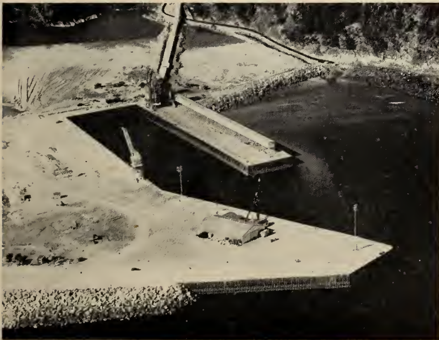
Fig. 5. Completed wharf. November, 1957.
