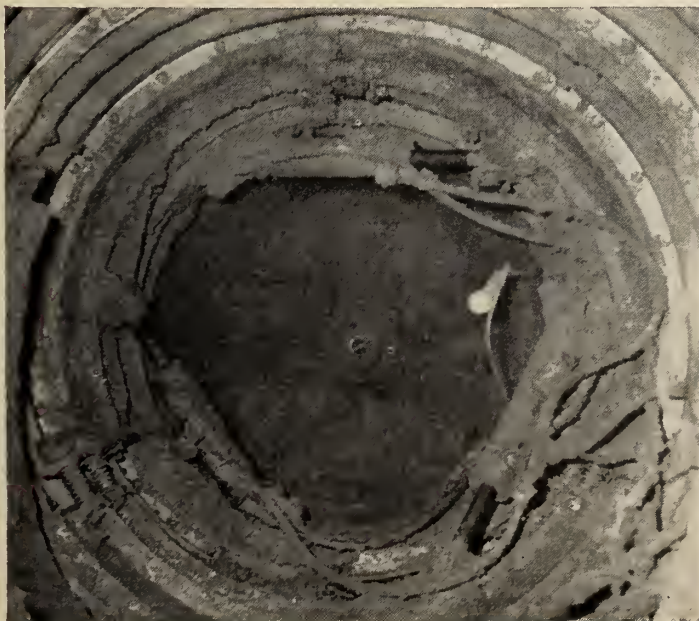
Fig. 3. Auger type shield installed.
