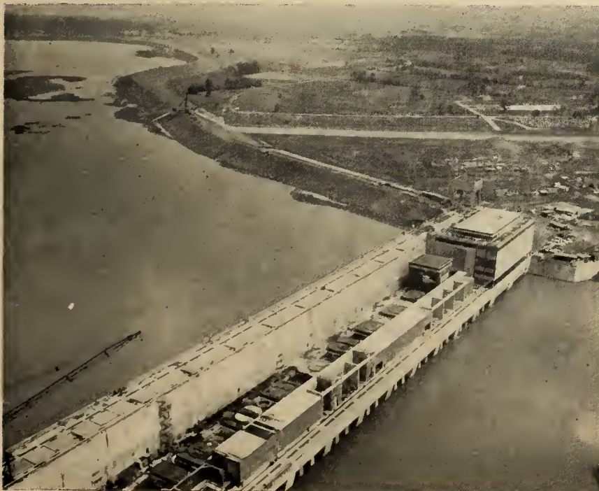
Fig. 6. A section of the powerhouse with part of the Cornwall dyke stretching into the background. The 3½-mile long dyke, which helps to retain the headpond, involved placing and compacting more than 5 million cubic yards of glacial till. (all photos: Ontario Hydro.)
