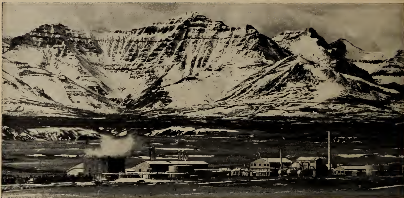
The first British American Oil plant at Pincher Creek, Alberta. A second stage plant is being built. Pincher Creek will be the largest single supplier of natural gas to the Trans-Canada Pipe Line when the expansion has been completed.
