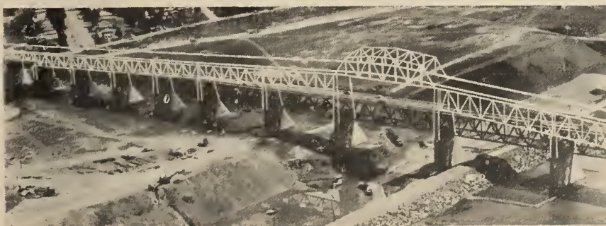
Fig. 2 Aerial view of the Jacques Cartier Bridge—showing some work in progress on the south shore.
