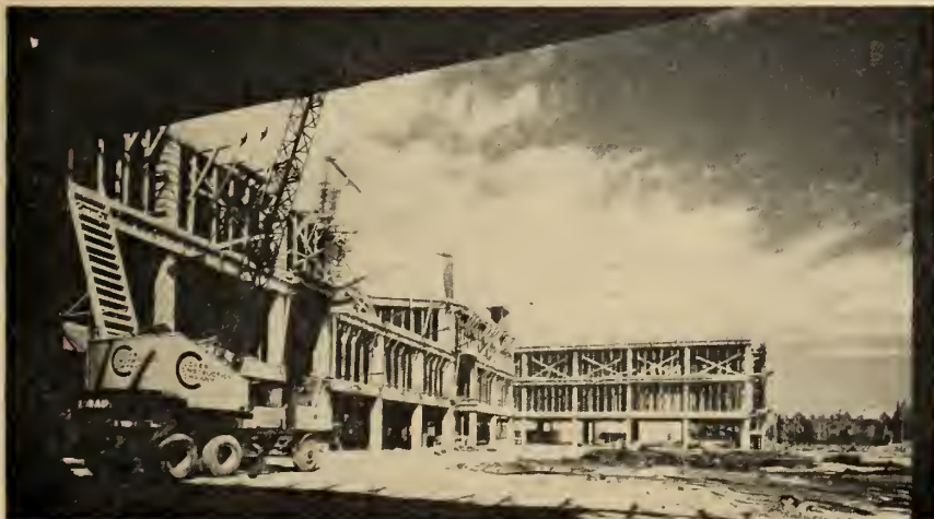
Progress on McMaster's Engineering Building, August, 1958.
