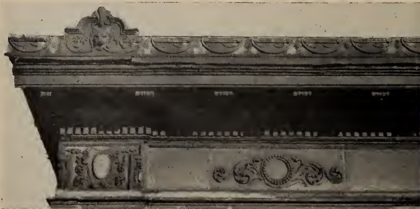
Fig. 7. Aluminum cornice installed in 1896 on the Canada Life building, Montreal, Que.
