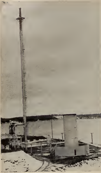
Fig. 9. 175 ft. high elevated flare and ground flare.
