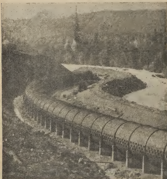
"Pacpipe" continuous Wood Stave Pipe line at B.C. Power Commission's Puntledge River Development.
