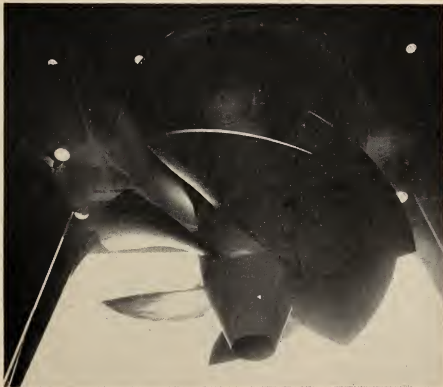
St. Lawrence Power dam. The runner assembly for Unit 28 is suspended by gantry crane before lowering into place in unit.
