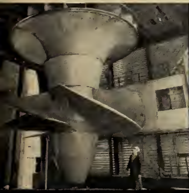
One of sixteen 75,000 H.P. English Electric fixed blade propeller runners being assembled with turbine covers, being fitted into position.
