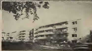
Kensington Tower Apts., Toronto, Ont., basement garage Crong & Booke Ltd., architects Kensington Industries, Ltd., general contractors
