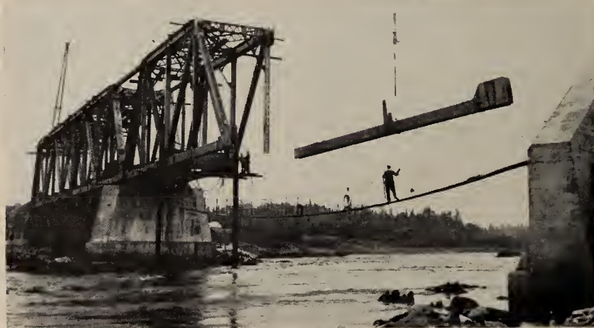
Bell River bridge on the C.N.R. Chibougamau line, Quebec.
