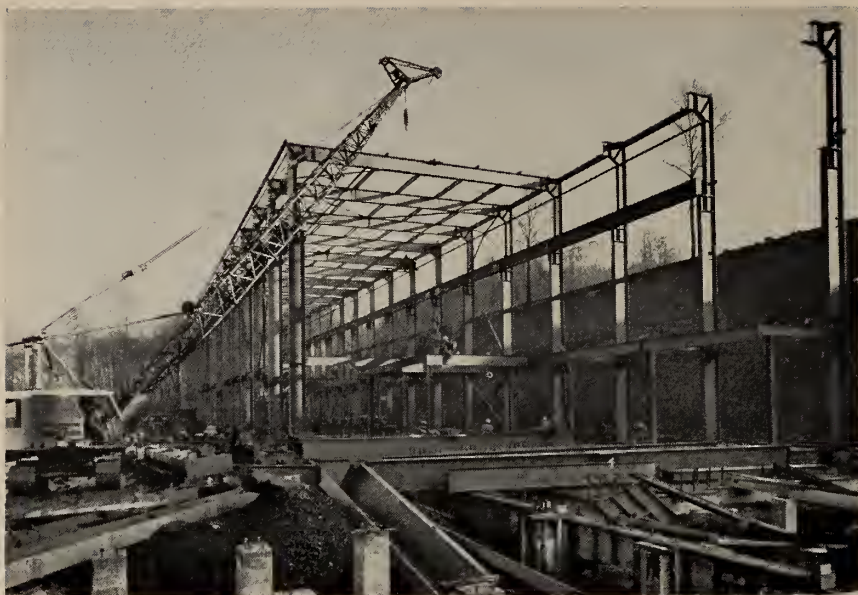
Gas turbine thermal-electric generating plant under construction at Port Mann, B.C.
