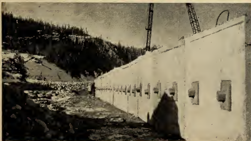
Fig. 9. Precast anchor walls in position.
