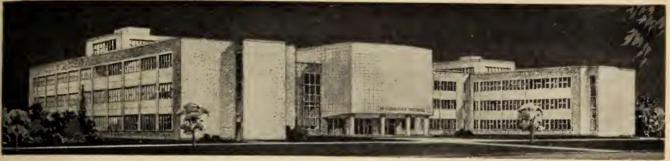
Engineering building, McMaster University, is being built.
