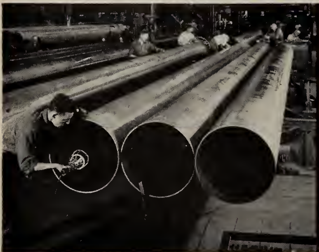
Fig. 26. End facing to required bevel for field welding.
