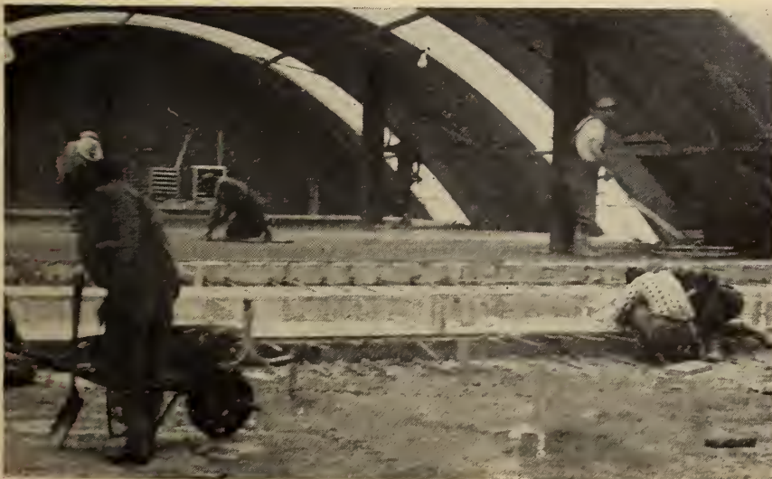
Fig. 4. Laminated wood arch enclosure. Photograph: Brian Akins, "Techniques of Winter Construction"
