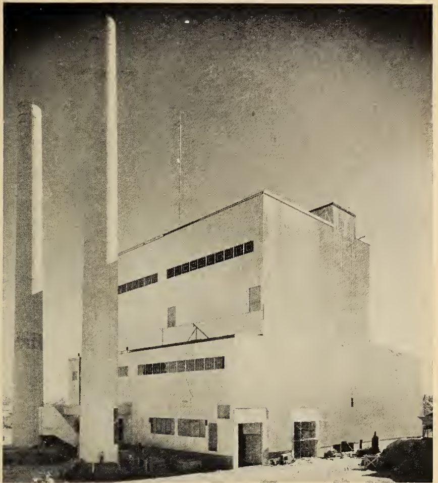
The Wabamun power plant of the Calgary Power Limited, showing the new stack and extension to the plant which will house a second 66,000-kw. generating unit.
