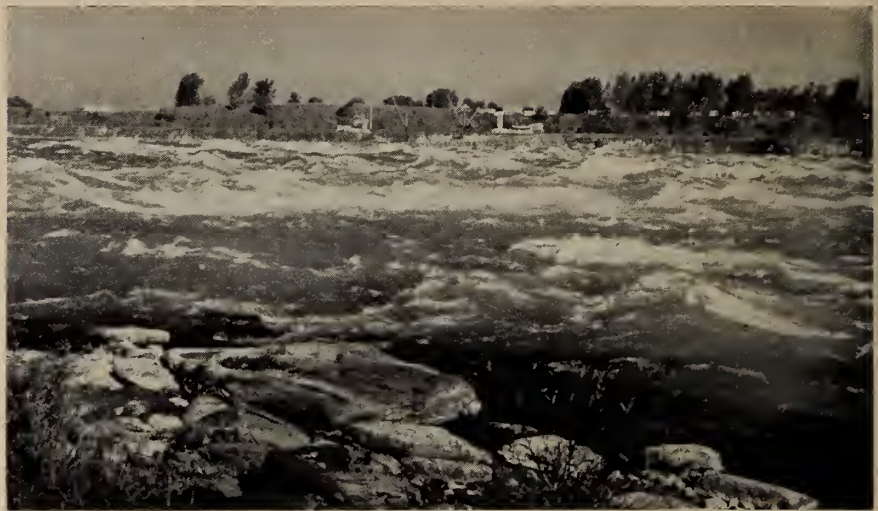
Long Sault Rapids before construction of cofferdam 'E' (PASNY)
