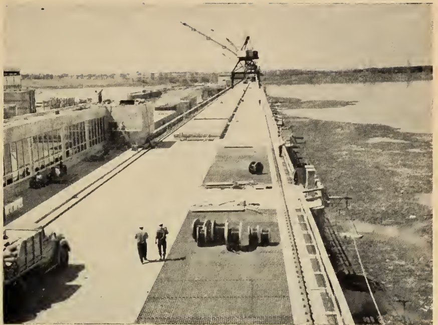
Fig. 5. This close-up view of the headworks of the generating station was taken shortly after the headpond was flooded. Debris visible in the forebay was flushed down the channel when a cofferdam was breached some 2½ miles upstream from the powerhouse.
