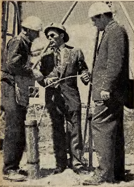
Loading "Nitron" blasting agent at the cofferdam. Since some of the charges were placed as much as 3½ months before the July 1st blast, it was essential that they be unaffected by water. "Nitron" which comes in hermetically sealed steel containers, was accordingly recommended by C-I-L Explosives Technical Service Representatives, seen in the picture above consulting with an Ontario Hydro blaster.
