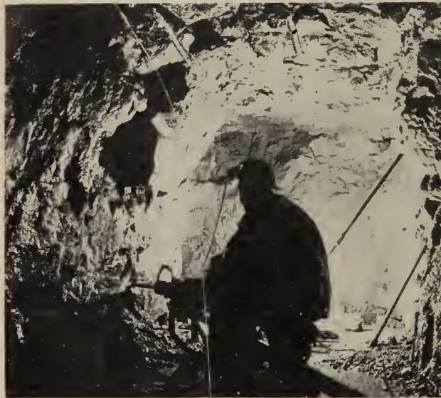
Fig. 11. McCormick Dam. Ring drilling the coyote tunnels, underneath the river. October 31, 1951.
