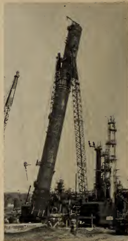
Fig. 15. Erection of the feed splitter tower at the powerformer.
