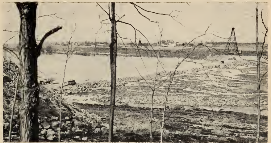
View of downstream slope of completed cofferdam. Note increasing width of downstream berm nearing closure gap. (HEPCO)
