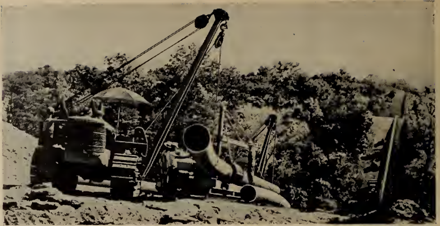
Fig. 30. On-the-spot cold field bending of 26-in.-OD line pipe.
