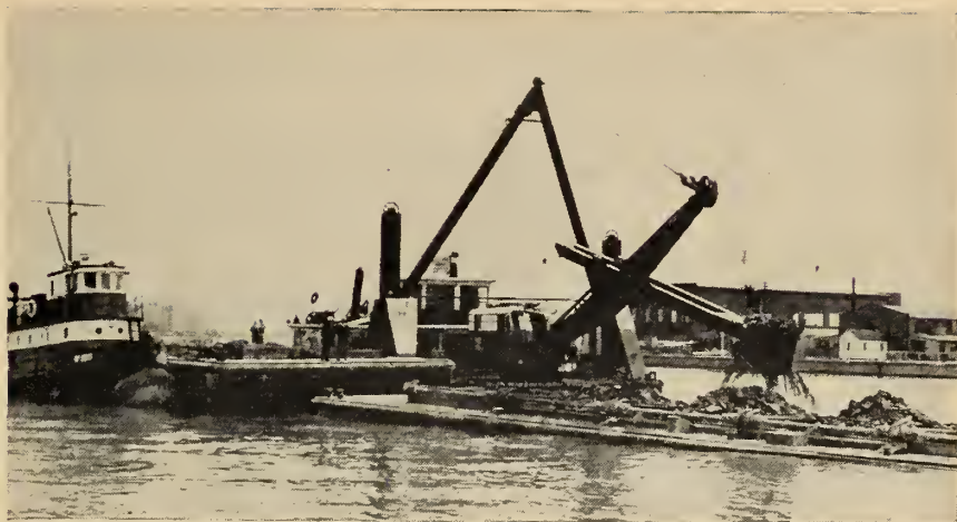
Fig. 2. Western entrance to Toronto Harbour. Channel dredging by dipper dredge A. L. Quinlan.
