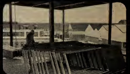
Panels stored within structure
