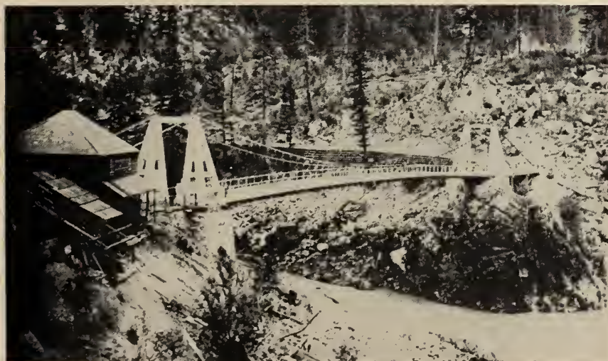
The old Alexandria Suspension Bridge at Spuzzam.
