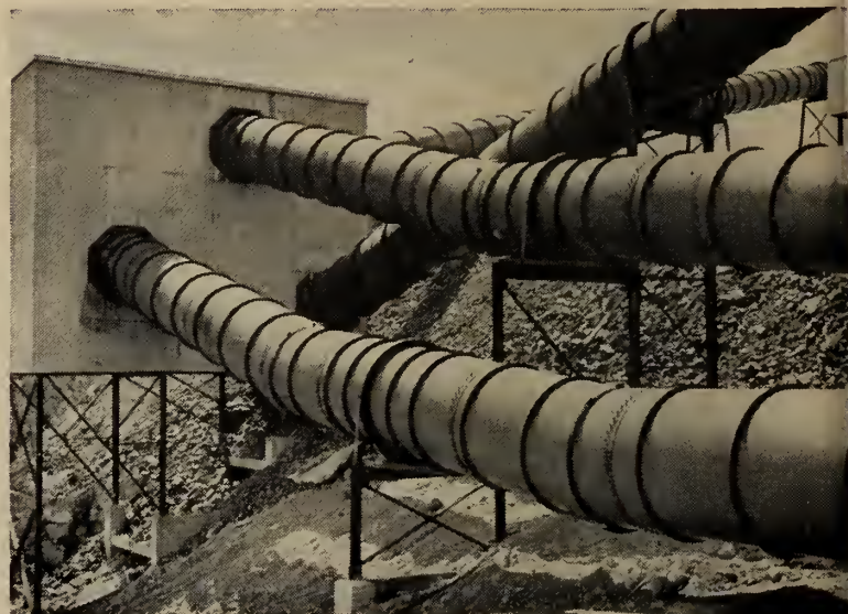
INTERESTING PATTERN is woven by these conveyer tubes installed at Consolidated Denison Mines Ltd. in Blind River region of Northern Ontario. They were constructed by Dominion Bridge which also supplied structural steelwork for many other uranium mines in this booming area.
