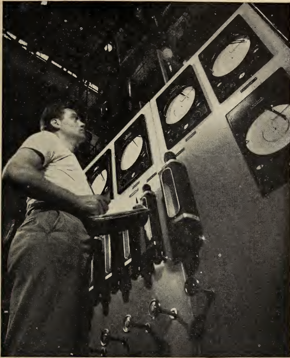
In the Still House, Honeywell instruments control temperatures, flow and pressure.
