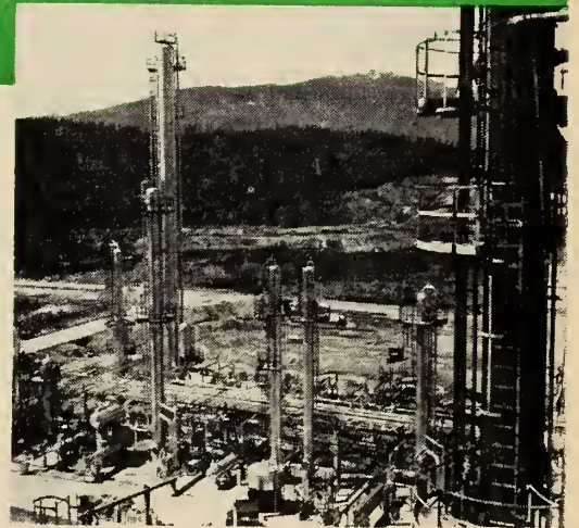
Latest Canadian Kellogg Alkylation Unit constructed at the British American Oil Company Limited refinery in Vancouver.
