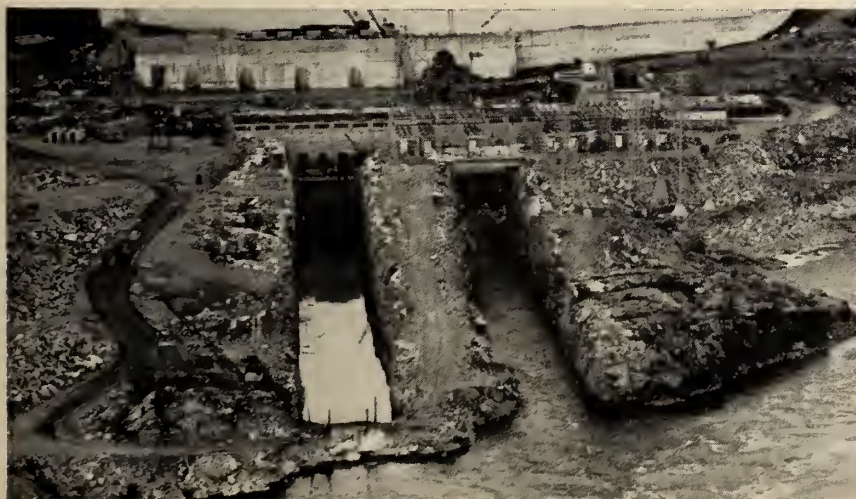
Fig. 24 (below). Drilling tailrace plug after toe blast.
