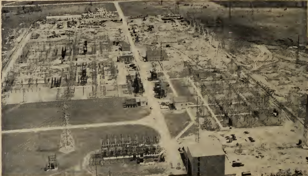
Fig. 1. Aerial view of the St. Lawrence transformer station. The 230 kv. switchyard is at left, the existing 115 kv. area right, and the 44 kv. facilities and part of the control building in the foreground. The terminal towers of the transmission lines from the St. Lawrence generating station are visible, upper right.
