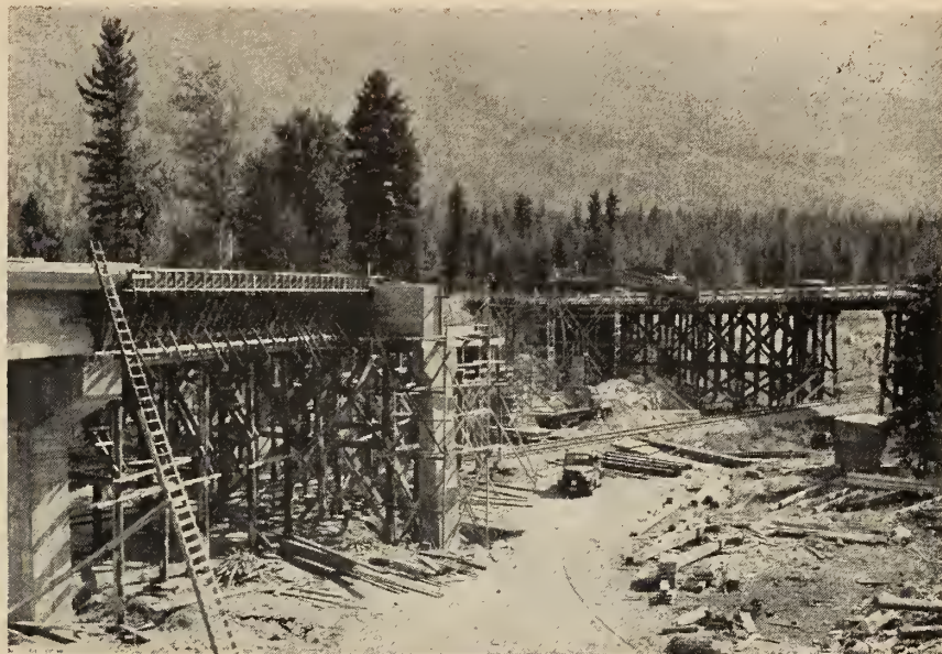
Road construction near Alexandria Bridge (October 1957).
