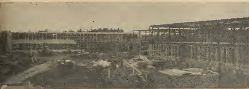
Centre Consolidated School under construction at Lunenburg, N.S.
