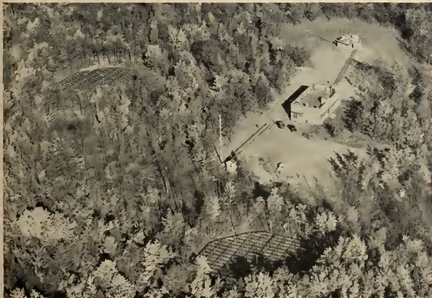
Fig. 2. General view, showing radar antennas.
