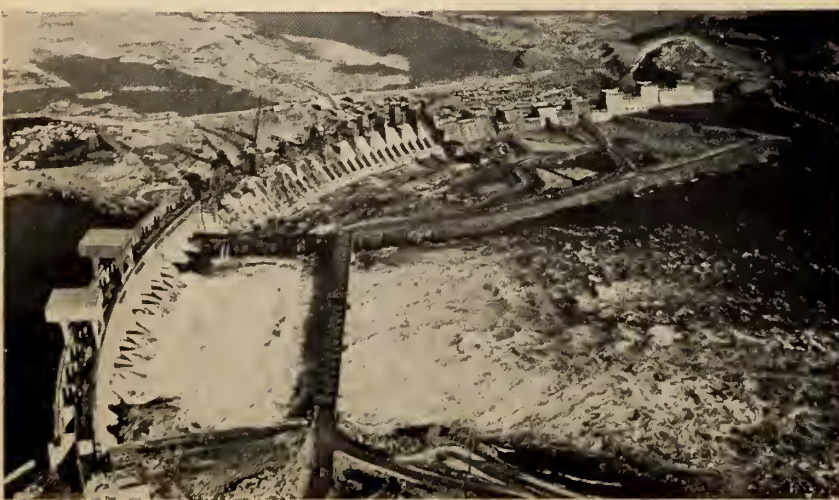
Long Sault dam. This view shows, left to right, the Stage 1 structure, the Stage 2 spillway section and the north bulkhead.
