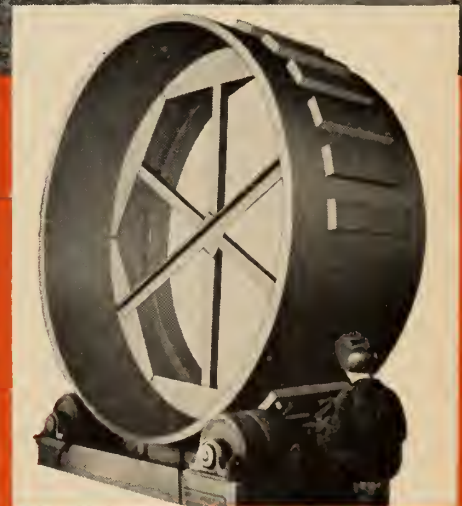
CEMENT KILN TIRE SECTION
