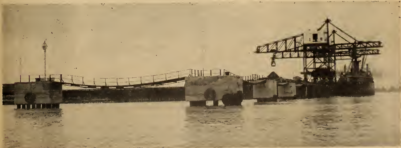
Fig. 4. Dolphins, spaced 80 ft. apart, at Contrecoeur transshipment area allow large ships to manoeuvre without tugs.
