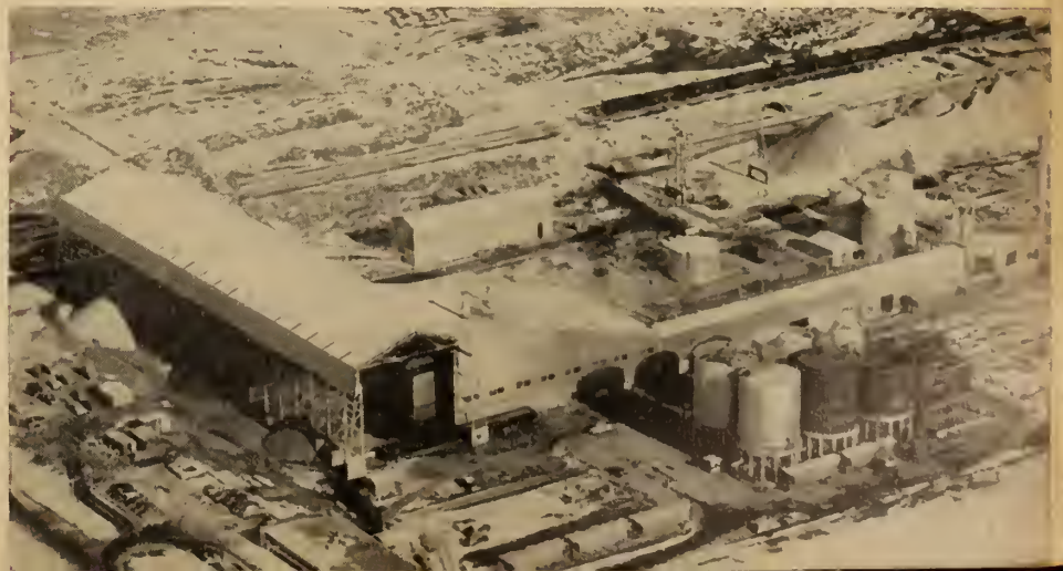
Cement plant at Regina for the Saskatchewan Cement Corporation Ltd.
