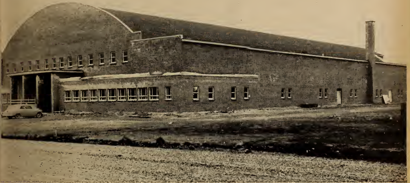
Sorel Arena, Sorel, P.Q. Consulting Engineers: Structural — Brouillet and Carmel, Montreal, P.Q.; Soil Mechanics — Foundation Engineering Co. of Canada, Montreal, P.Q. Contractor: Lucien Lachapelle, Sorel, P.Q.
