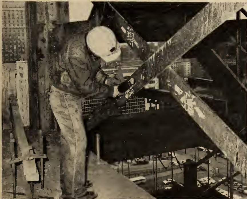
Fig. 13. Checking stress with extensometer.
