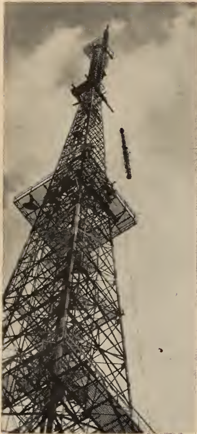
The channel 9 antenna being removed from the CBLT tower, in Toronto, during the change-over to channel 6.
