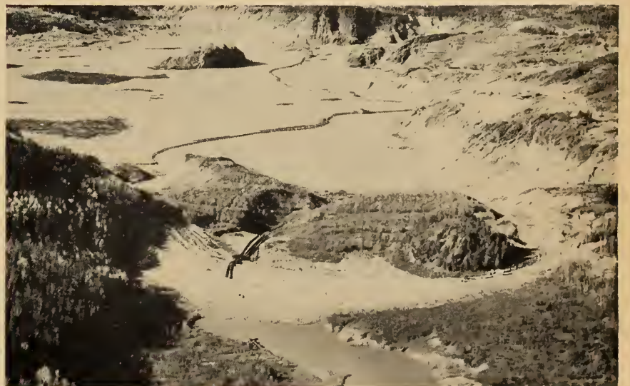
Fairweather Dam on completion of the second lift, 1956.
