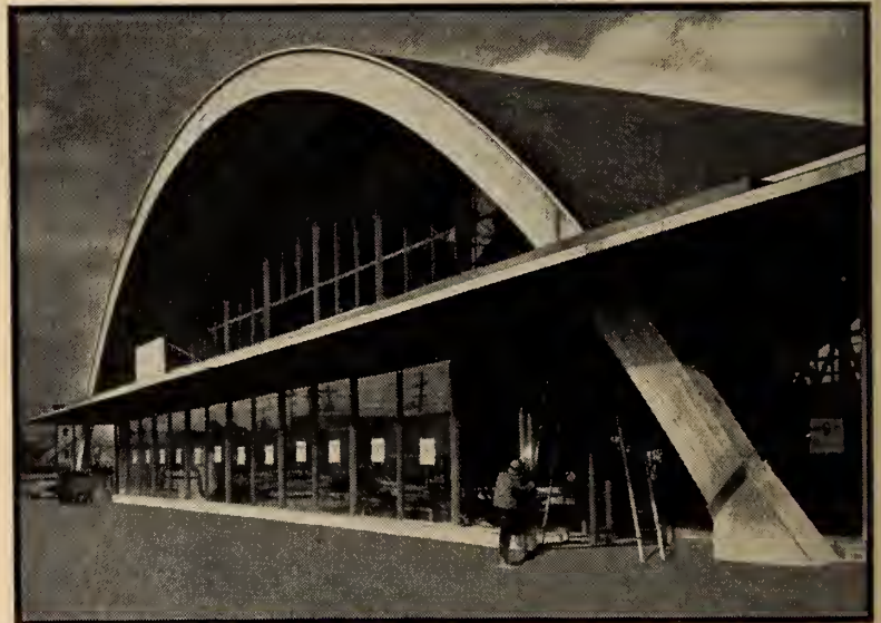
Grand Union Shopping Center Architects: Husband Wollock & Baldwin Contractors: Louis Donolo (Ont.) Ltd. Arches up to 150' span by Timber Structures
