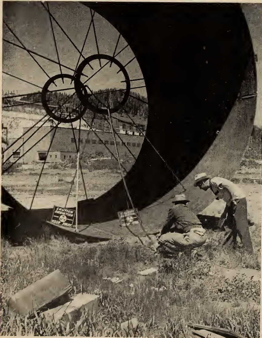
Testing Penstock Welds at Trench Development, June, 1955. This photograph, contributed by The Shawinigan Water and Power Company, Montreal, received an award of merit in the E.I.C. photographic exhibit, 1956.
