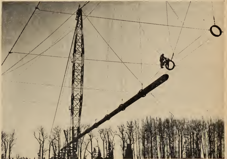
Stringing pipe for the Shelley Crossing of the Fraser River.
