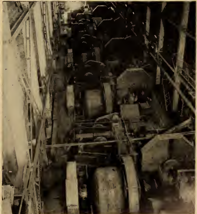
The Flin Flon mine, in Manitoba, is the second largest Canadian producer of zinc. The general view of the crushing plant (left) shows the main belt conveyors; ball mills and classifiers for secondary grinding are seen (right) in the concentrator plant. (Photo: Hudson Bay Mining and Smelting Co. Ltd.)
