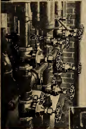
TOP: An installation of Jenkins Bronze Gate Valves on the fuel oil pump manifold in the power house.
