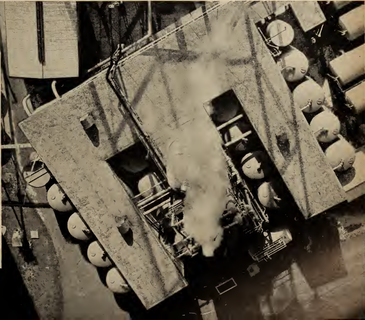
Water-tower view of PERMUTIT water-treatment equipment at Gulf States Utilities Company's Louisiana Power Station, North Baton Rouge, La. Engineered and constructed by Stone and Webster Engineering Corp.
