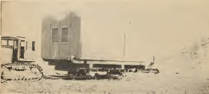
Module on sled is being towed by a D-8 tractor.
