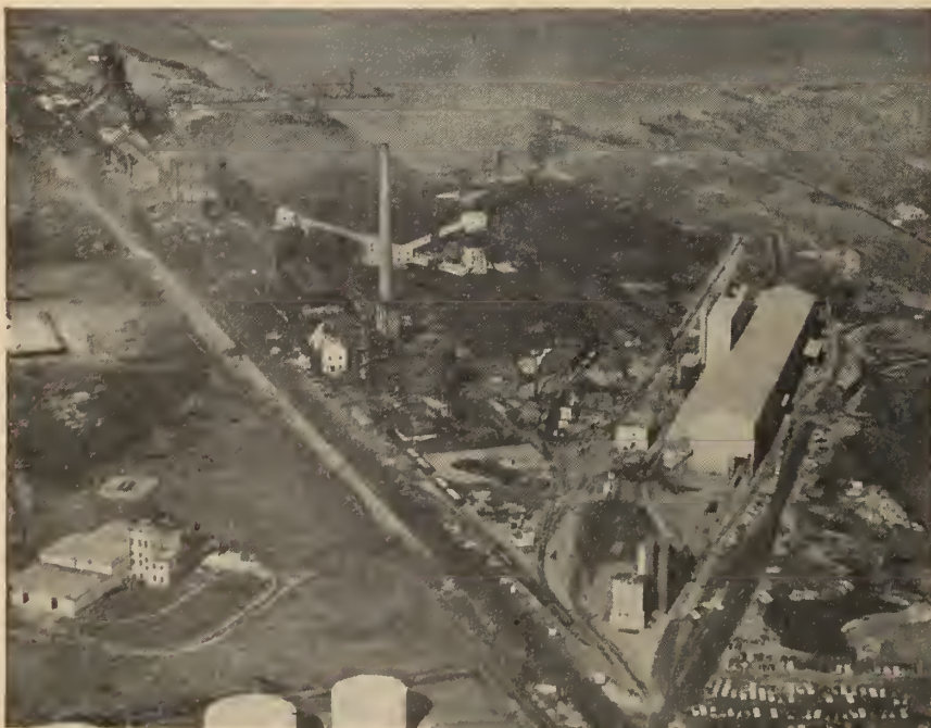
In this general view of the Dominion Foundries and Steel Company's plant at Hamilton, Ont., may be seen the oxygen steel-making plant (prominent high building, right centre). Coal handling plant and coke ovens are immediately behind the stack, and the blast furnace is at the top left.
