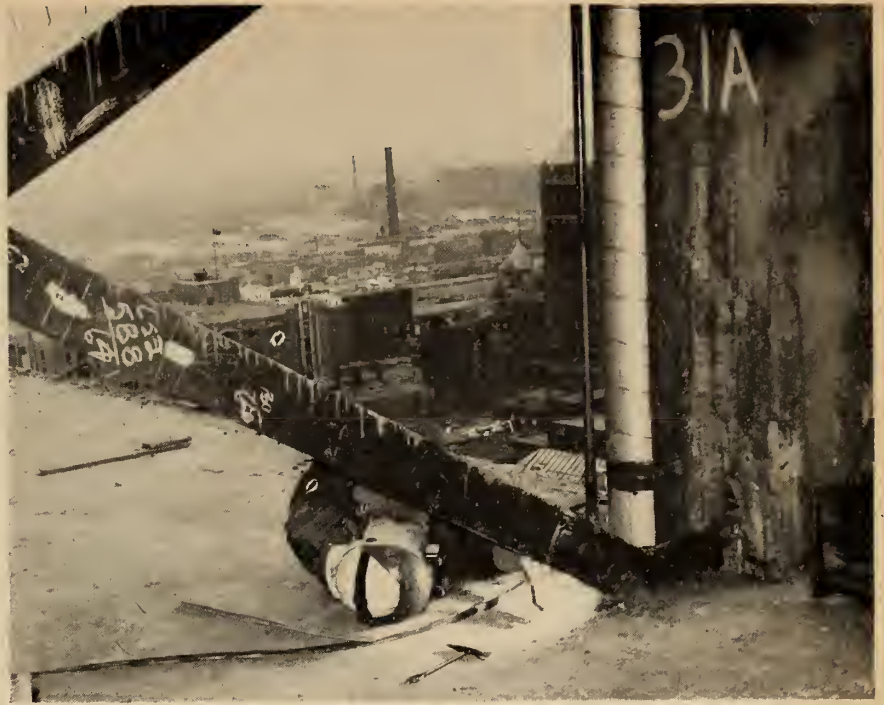
Fig. 12. Welding the final connection.
