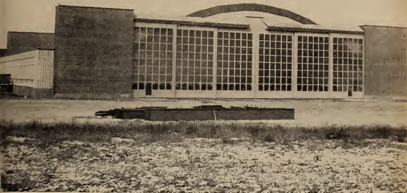
Arch-type steel hangar at Uplands Airport, Ottawa, built for the R.C.A.F. by Defence Construction Limited. Contractors: Arga Construction Ltd., Montreal. Architects and Engineers: Ross Patterson Thompson & Fish, Montreal.
