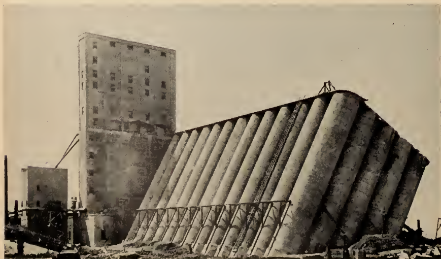
Above: West side of elevator, showing tilt and soil upheaval. Below: East side following foundation failure; early stages of righting operations are shown under way. (Photos: Foundation Company of Canada Limited.)
