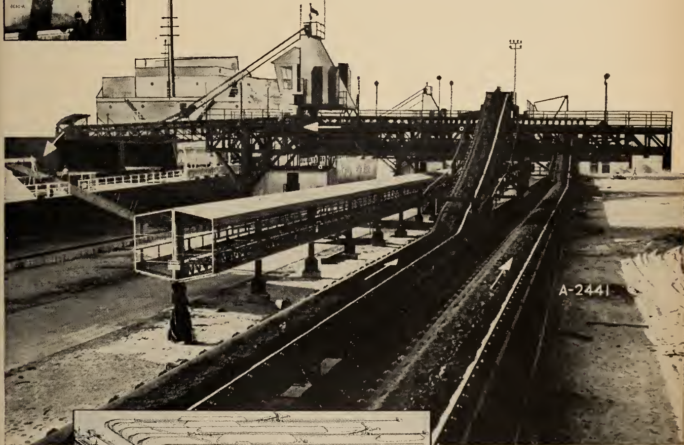
Here, the traveling stocker is building a stockpile at the rate of 3750 net tons per hour. Conveyor booms stockpile to either side.
