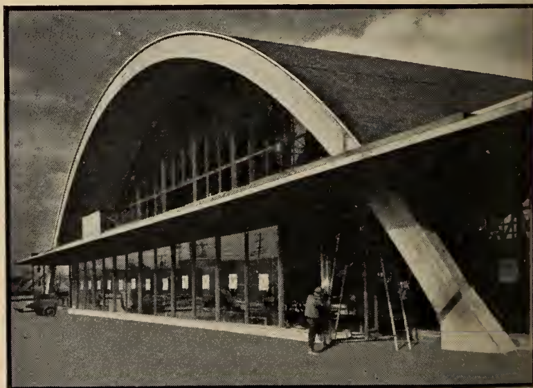
Grand Union Shopping Center Architects: Husband Wallace & Baldwin Contractors: Louis Donolo (Ont.) Ltd. Arches up to 120' span by Timber Structures
