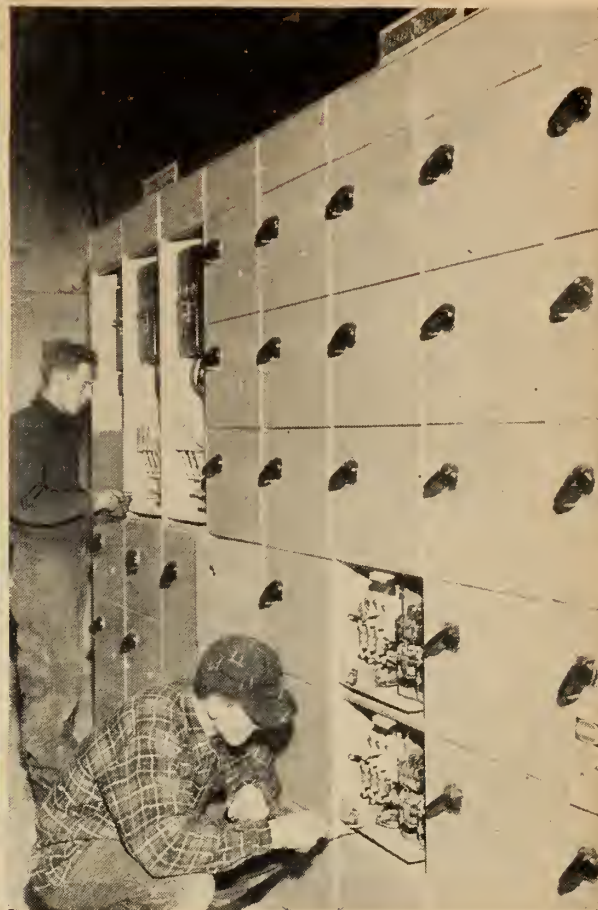
A General Electric Motor Control Centre is shown being installed in an Ontario uranium processing mill. To slide each unit into its compartment is a simple, quick operation.
