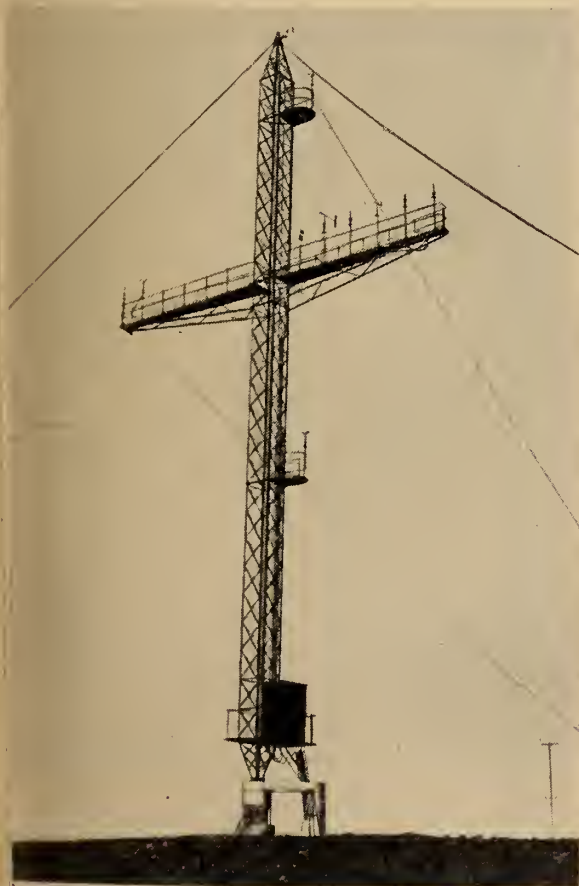
Fig. 5. 120 ft. rotatable mast used for wind measurements on Costa Hill, Orkney.
