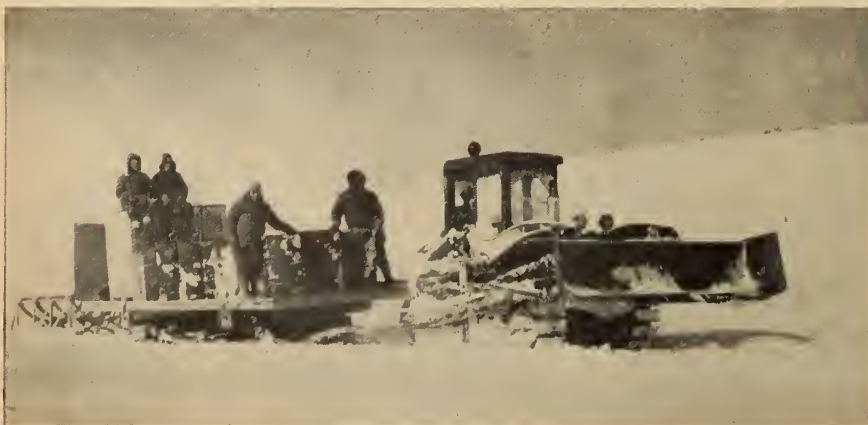
A load of fuel and equipment being hauled to a site on the Mid-Canada Line.
