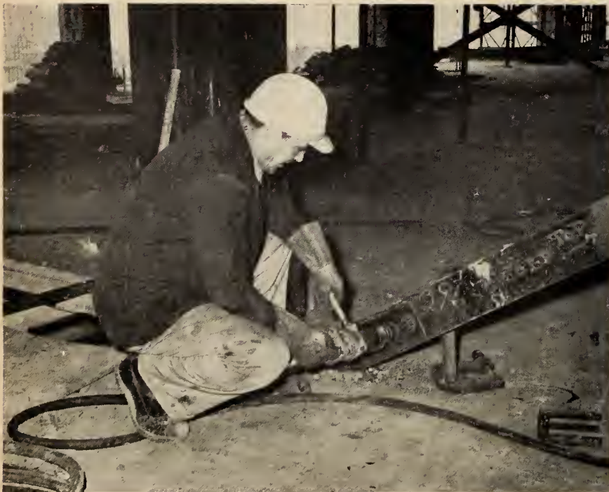
Fig. 11. Bolting with high strength bolts.
