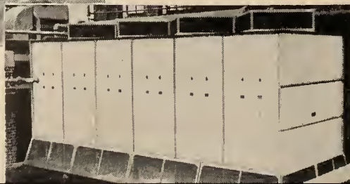
Evaporative condenser handling 330 tons of refrigeration
