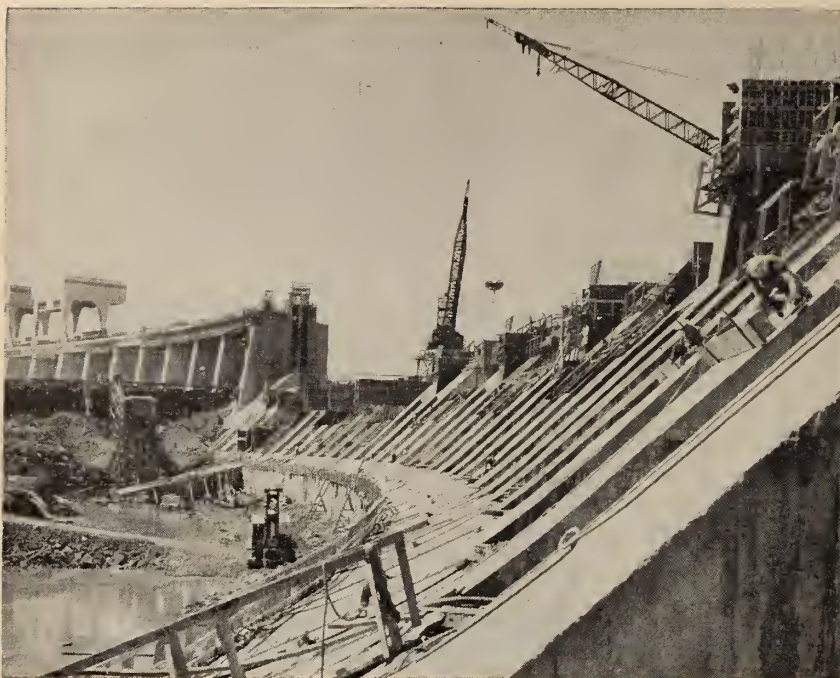
Long Sault dam. The stage 2 portion of the structure.
