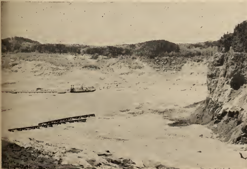
Lime Point, location of future pit.
