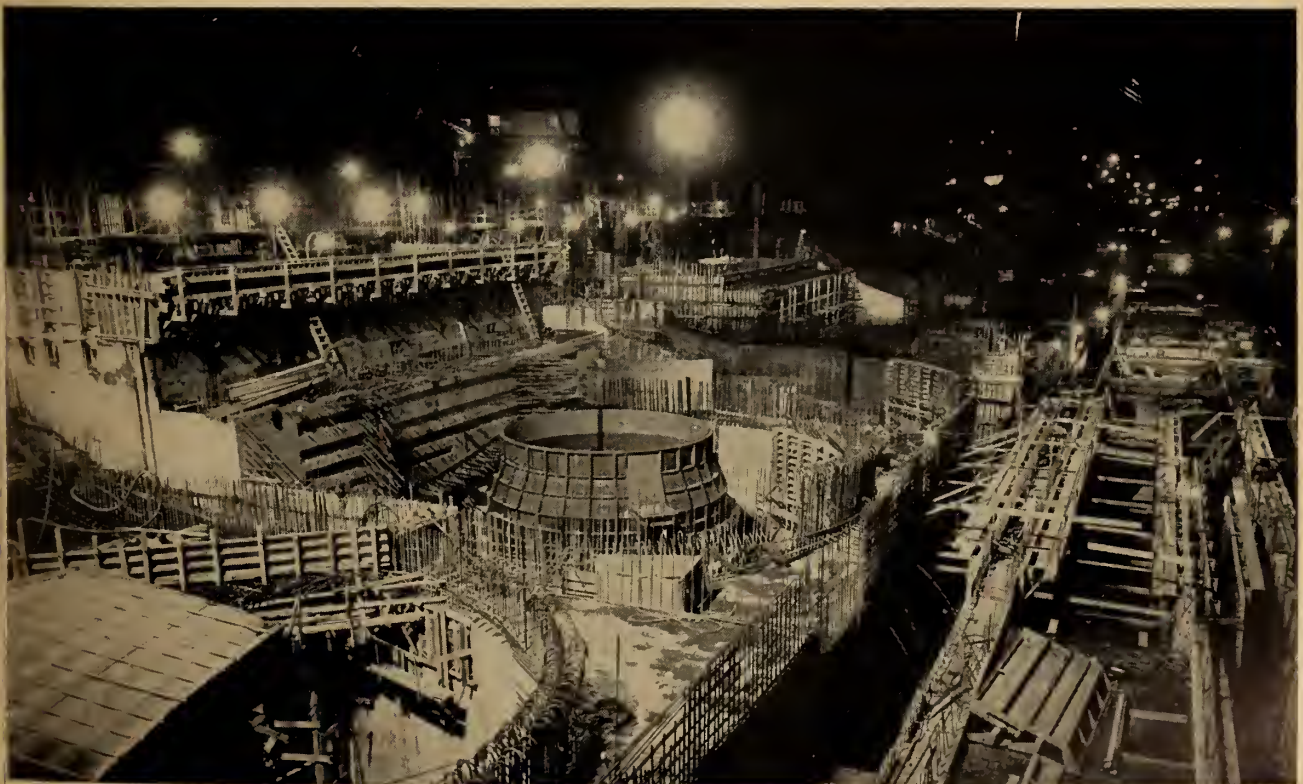
The power-house takes shape.
