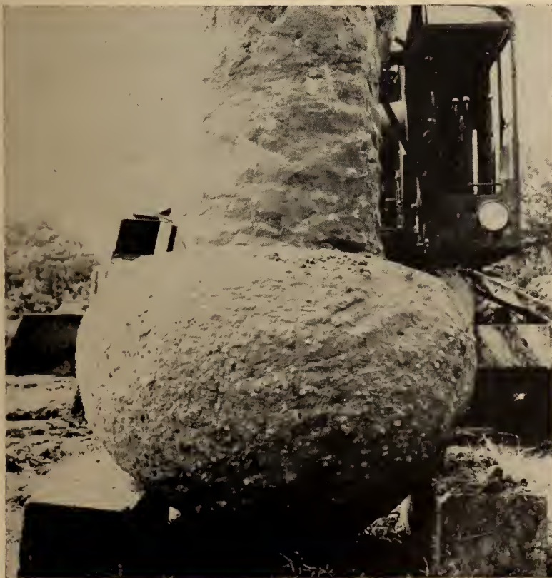
Fig. 6. Base of typical caisson pile.
