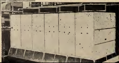
Evaporative condenser handling 330 tons of refrigeration
