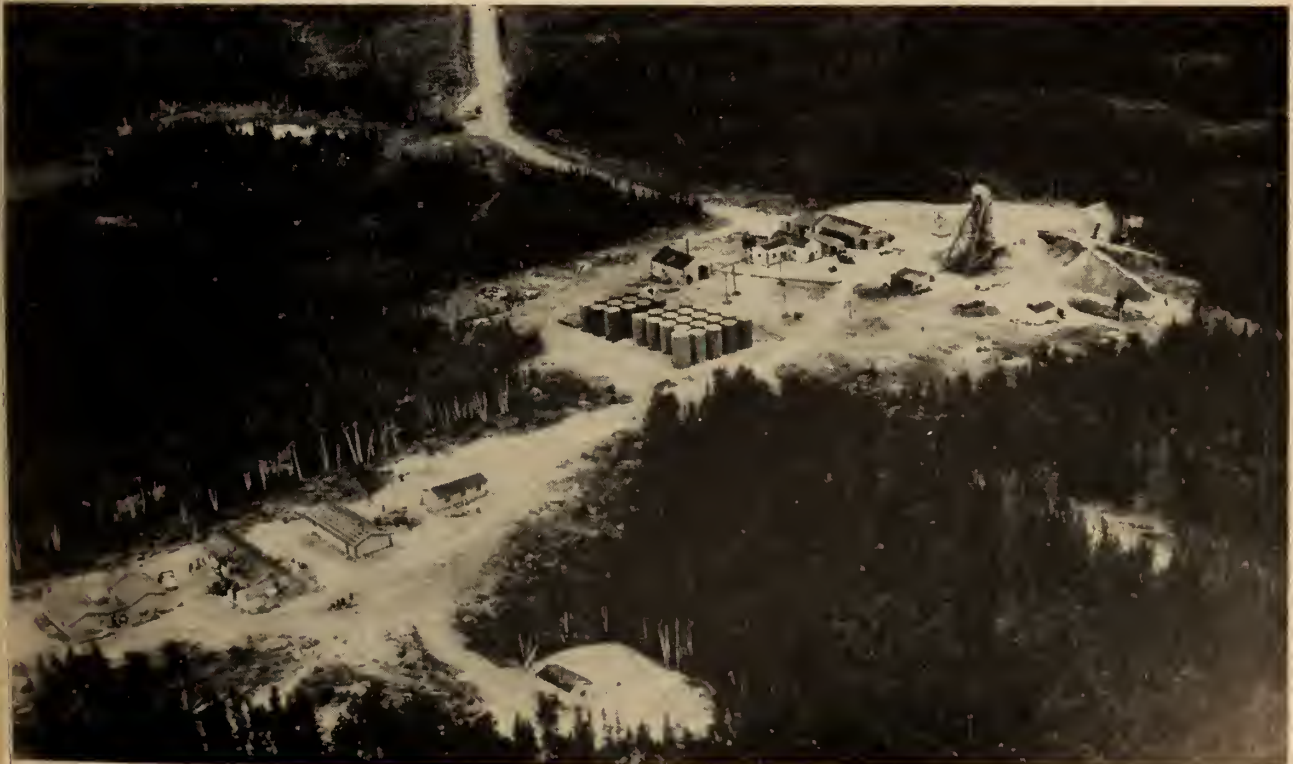
Exploration shaft at International Nickel's Moak Lake development, which will be used as the main entrance to the nickel mine when operations begin. (Photo: Manitoba, Dept. of Industry and Commerce.)
