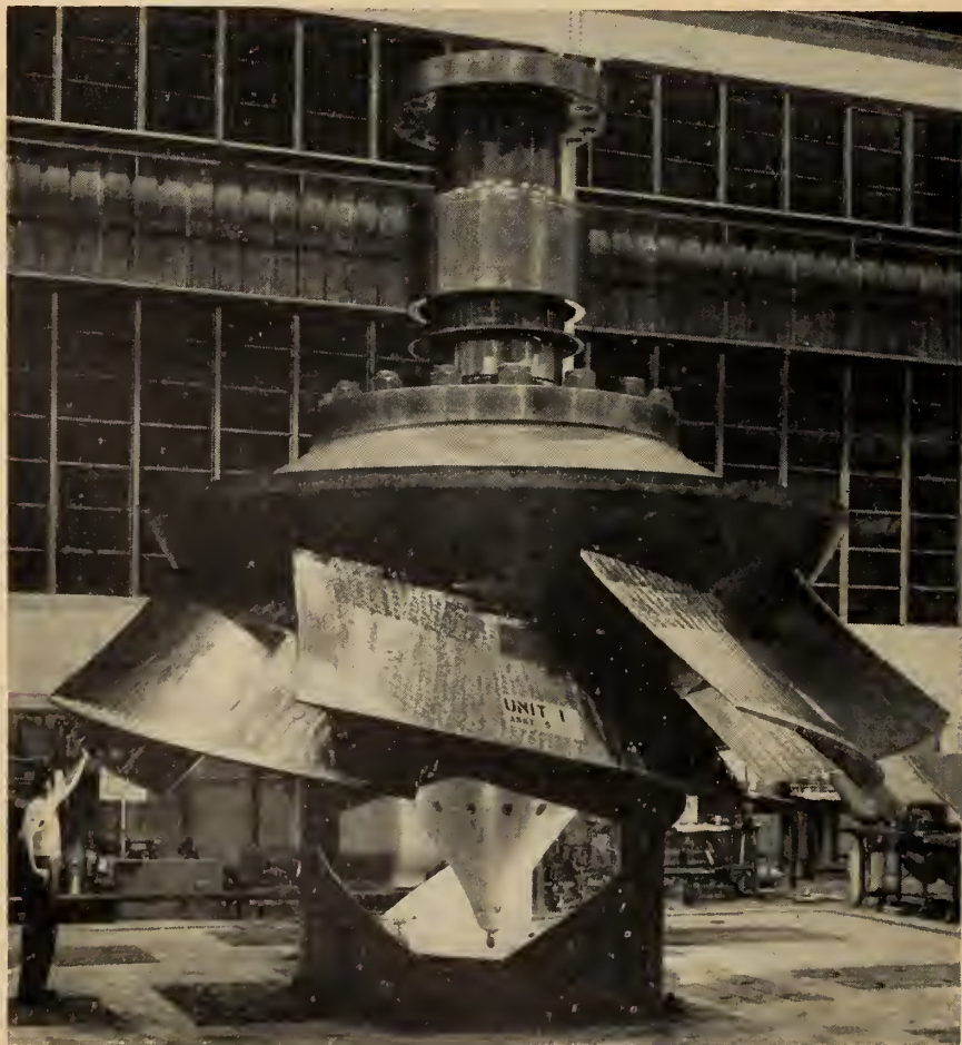
The runner hub assembly of one of the turbines for the Niagara pumped storage scheme. Six such units will pump off-load water into a reservoir; by reversal of the units power can be generated. (Photo: English Electric Company of Canada.)
