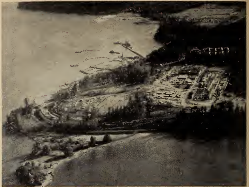
An aerial view of the site of a $38-million pulp mill being constructed near Duncan, B.C., for British Columbia Forest Products Limited. Deep-sea wharf, ferry slip, and scow dock are in centre, rear. Town of Crofton is in the right background.
