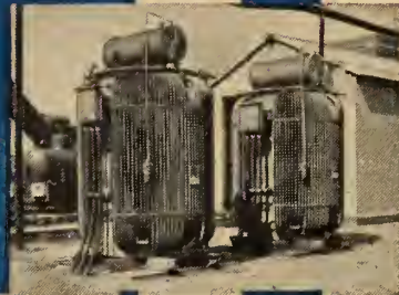
2-20 MVA 11 kV reactors.
