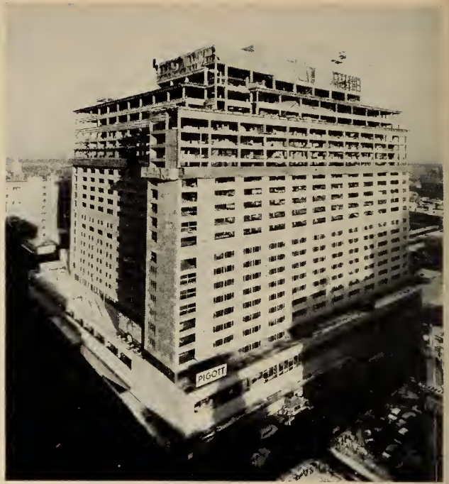
Fig. 14. View of hotel on completion of pretensioning.
