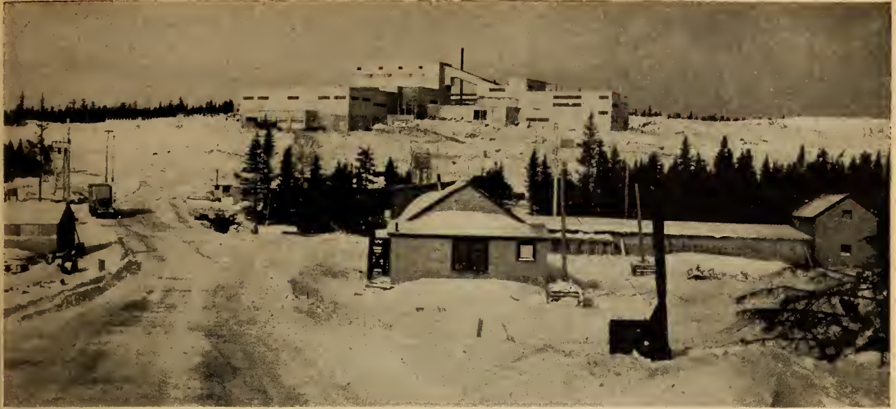
Due to go into production early in 1957 was Heath Steele's 1500-ton mill at the lead-zinc-copper operation at Little River, near Newcastle, N.B. (Photo: New Brunswick, Dept. of Lands and Mines.)
