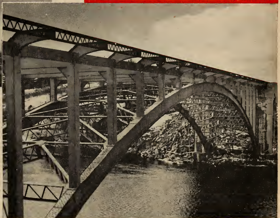
Above — New Canadian Steel Corporation plant at Etobicoke, Ont., during construction. Right — Hingeless arch span highway bridge near Kenora, Ont.
