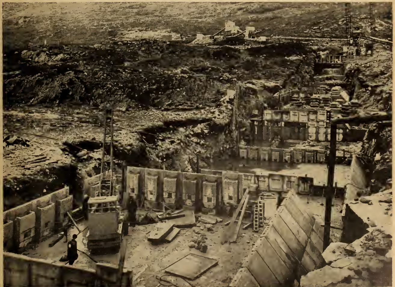
Fig. 3. View along the dam showing panels in position
