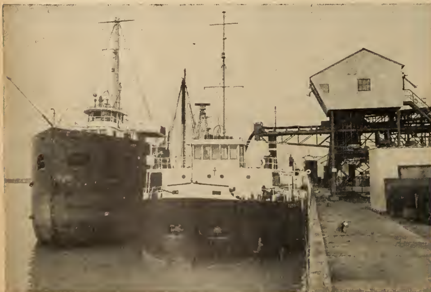
Fig. 3. Discharging from loading tower. Empty canaller moored at left.
