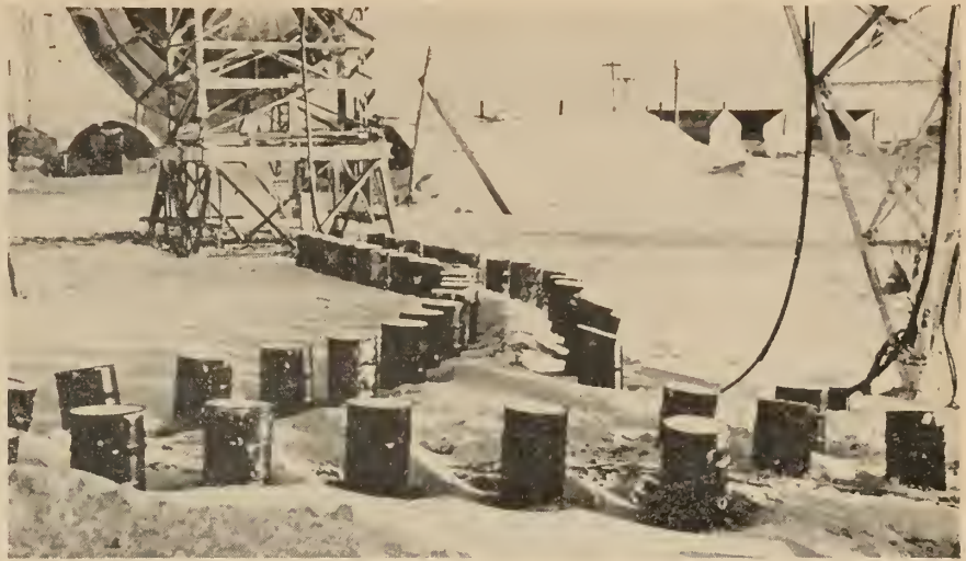
Styroflex cables to 30 ft. parabolic reflector and guyed tower are covered with gravel and marked with empty oil drums. Note corner reflectors in rear. Foreground building is a Simpson hut, while those to the rear are framed tents.
