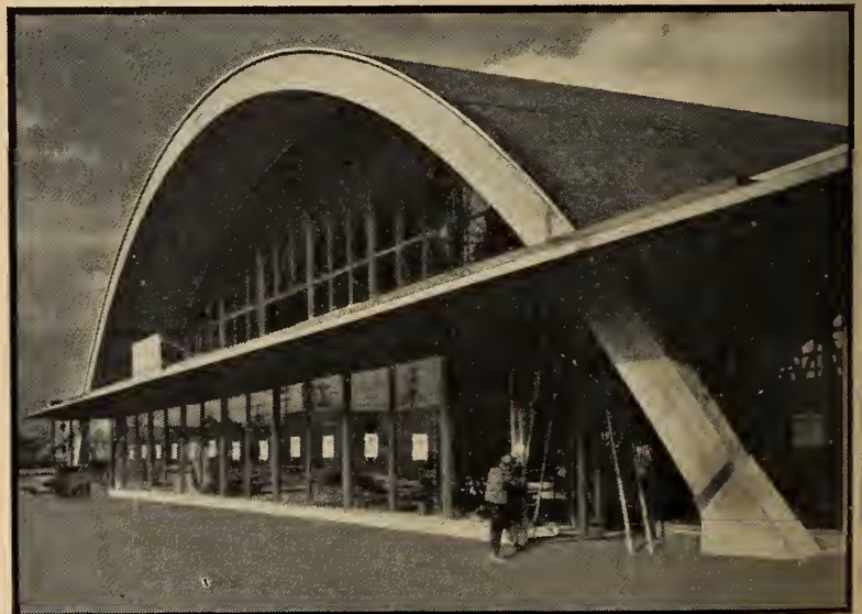
Grand Union Shopping Center Architects: Husband Wallace & Boldwin Contractors: Louis Donolo (Ont.) Ltd. Arches up to 120' span by Timber Structures
