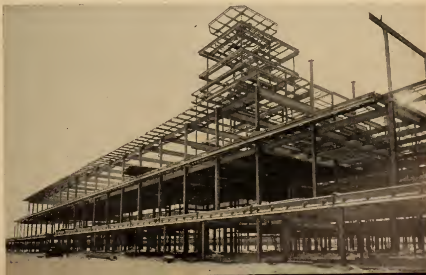
Steelwork for Montreal's Dorval Airport building. (Photo: Dominion Bridge Co.)
