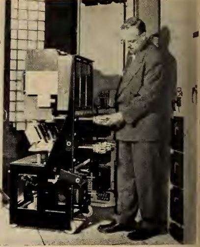
"Notice the complete accessibility. The full floating primary contact fingers can be serviced conveniently because they are on the breaker, not in the cell."
