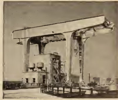
60-ton headworks gantry crane
