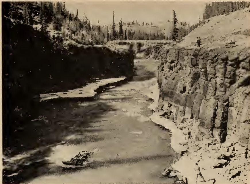
Fig. 6. Echo-sounding raft at the damsite, Miles Canyon, Yukon River.
