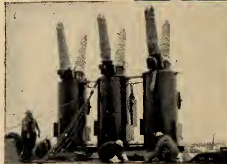
Huge Westinghouse step-up transformers like this are now being built at Westinghouse in the St. Lawrence Generating Station.
