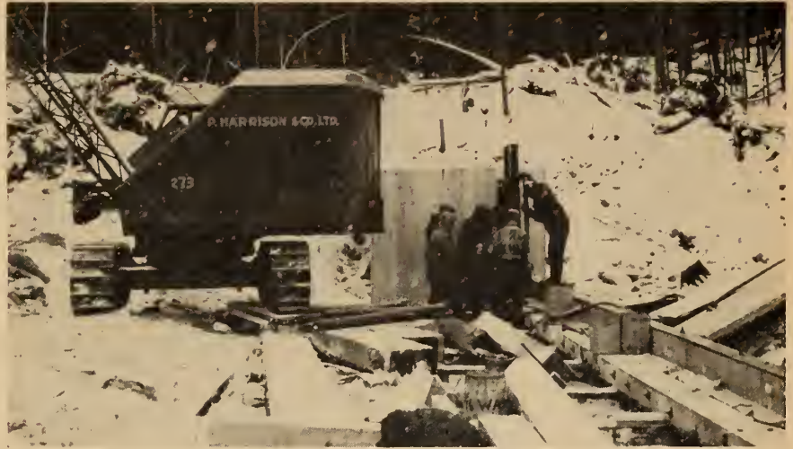
Construction of cribwork at one of the North Marmion Dams.
