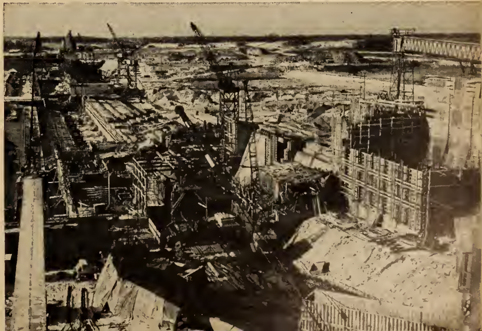
Construction progress at Ontario Hydro's power-house project.
