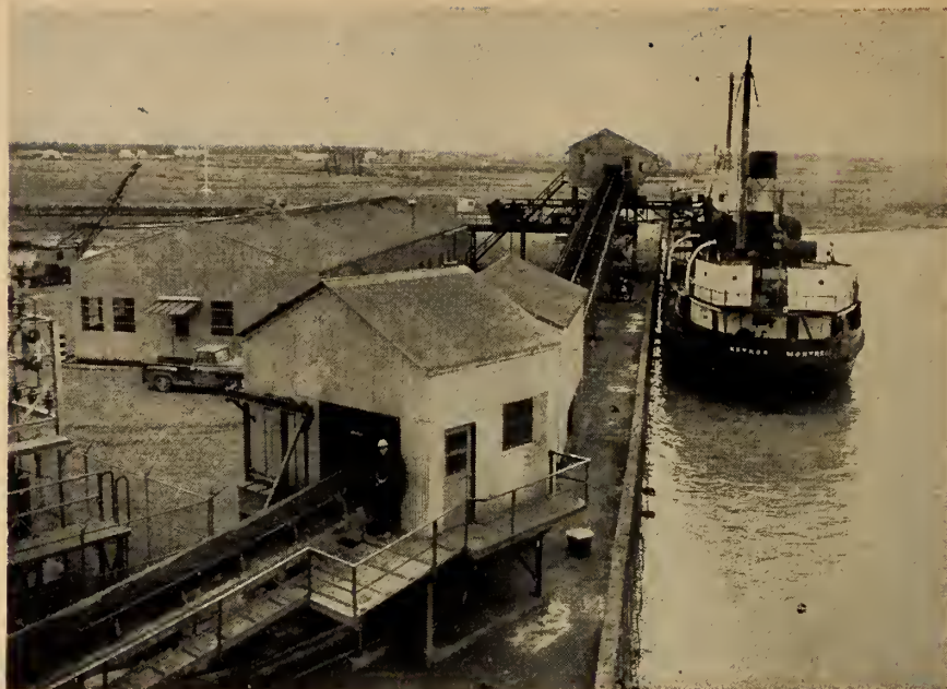
Fig. 2. View of the dock conveyor (left) and inclined belt feeding the canaller loading tower (right centre).
