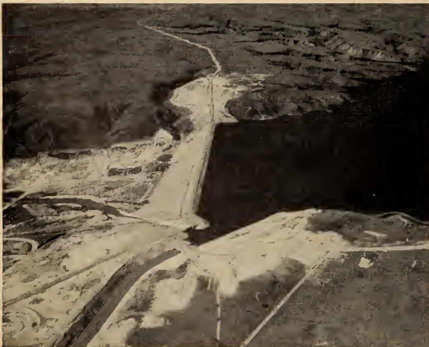
Fig. 1. Travers Dam; spillway and outlet canal from reservoir in foreground.
