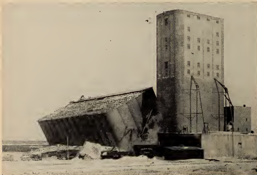
Above: West side of elevator, showing tilt and soil upheaval. Below: East side following foundation failure; early stages of righting operations are shown under way. (Photos: Foundation Company of Canada Limited.)
