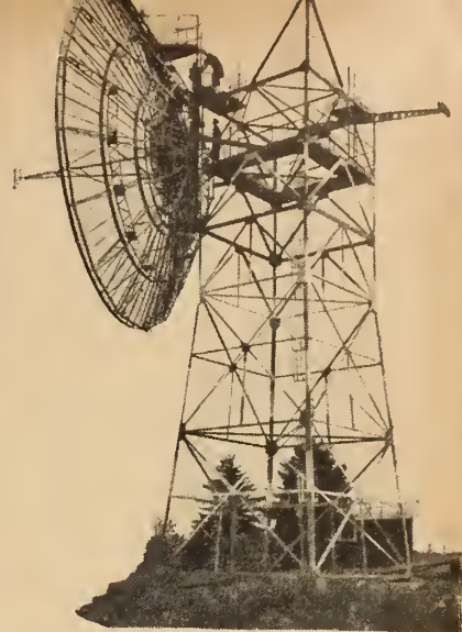
Microwave parabolic reflector for transmitting ultra-high frequency waves. Mechanical design, fabrication and erection by Dominion Bridge for RCA Victor Company Limited.
