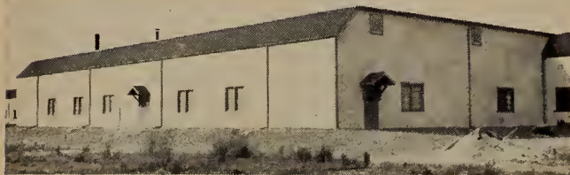
The new addition being heated by a Dravo Counterflo Heater.
