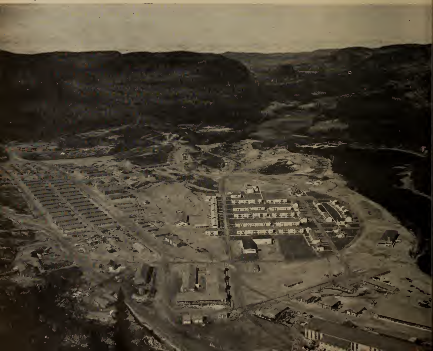
Fig. 19. Aerial view of Labrieville showing camp site (left), permanent town site (right), and permanent machine shop (right foreground).
