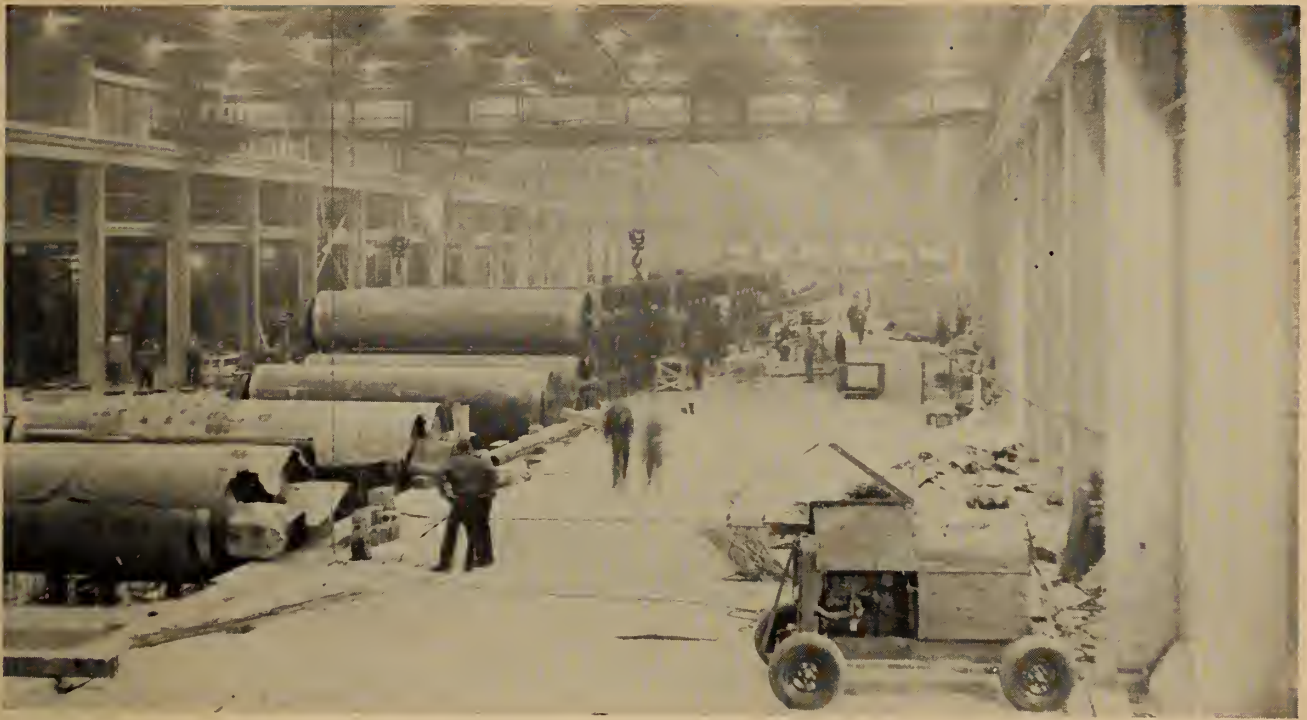
Fig. 12. Paper machine dryers partly erected in the new machine room.
