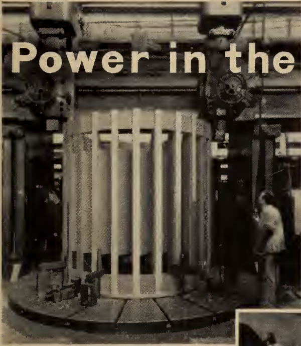
Machining the rotor spider
