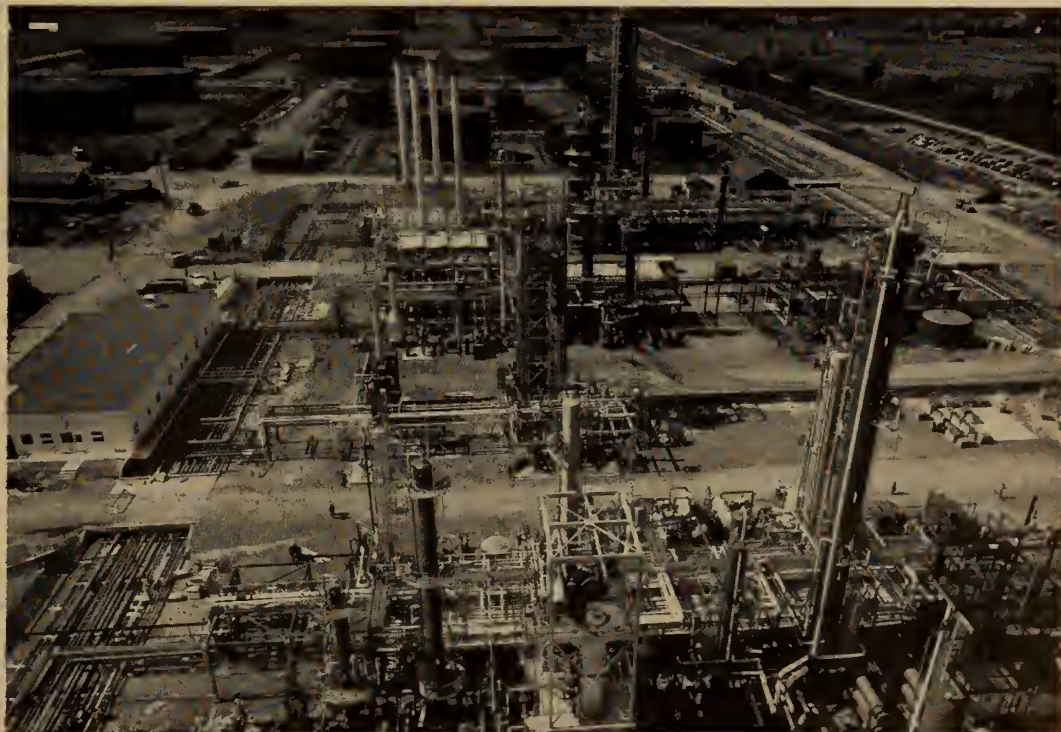
Fig. 11. The central control house (left) serves all the process units, some of which are seen here. Alkylation and catalytic polymerization unit in foreground; hydrodesulphurization unit; ultraforming and acid treating; crude treatment units at far end of process area, beyond which are the crude tanks. Pipe runways are seen flanking the process area.
