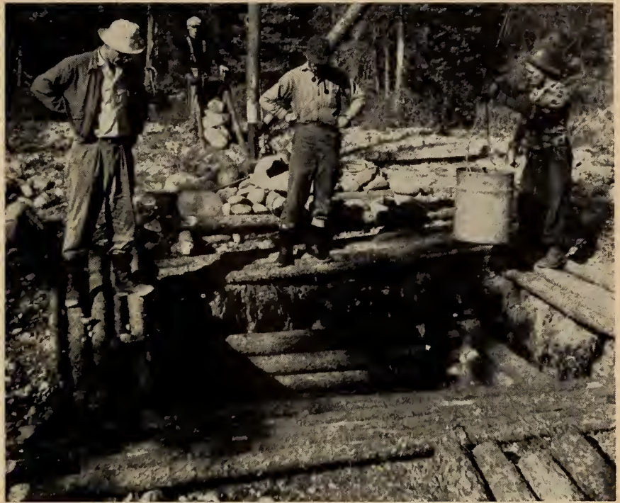
Fig. 7. The deepest test pit, 41 feet, dug in two weeks.
