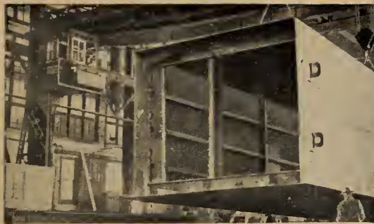
• Steel box section weighing over 40 tons for a mining company.
