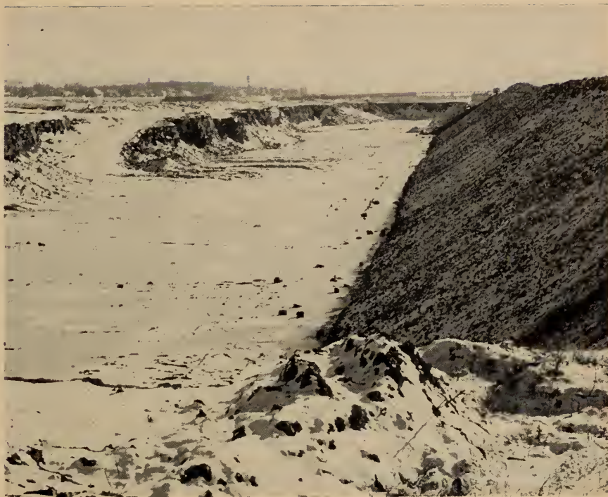
Fig. 9. Approach channel below St. Lambert lock during construction.
