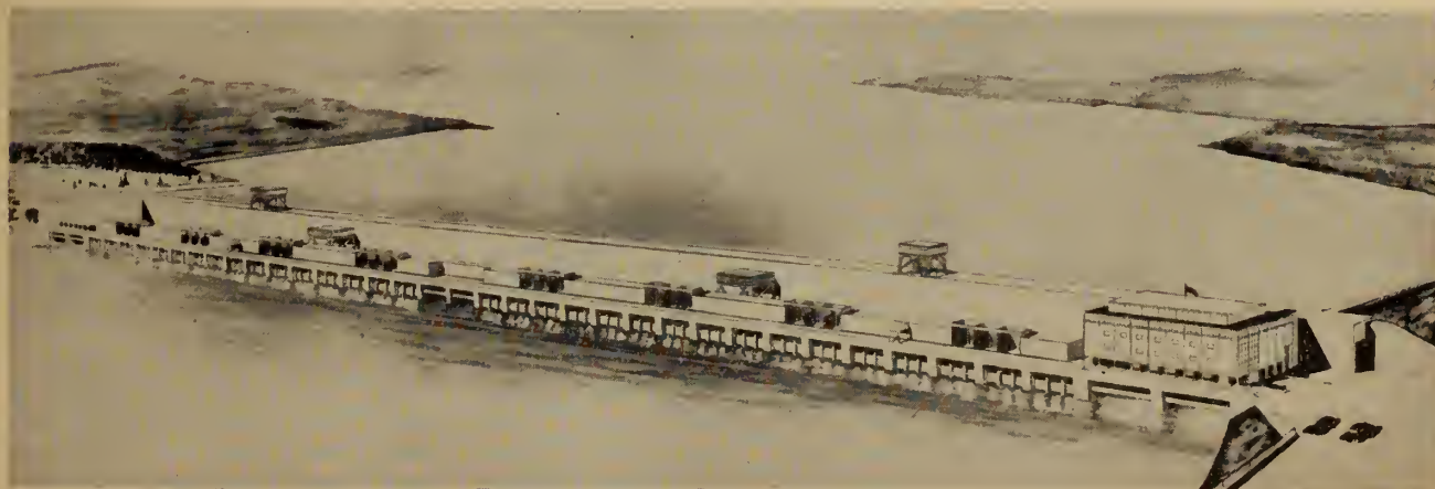
Architect's model, showing part of the Canadian section of the St. Lawrence powerhouse. The building will span some 3,300 feet between Barnhart Island and the Canadian mainland, and will be built by Ontario Hydro and the Power Authority of the State of New York.
