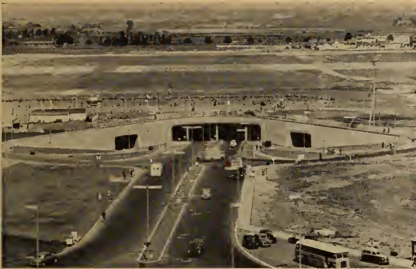
Looking north from the control tower, showing the entrance to the main tunnel connecting the central area to the Bath Road (top of Fig. 2).
