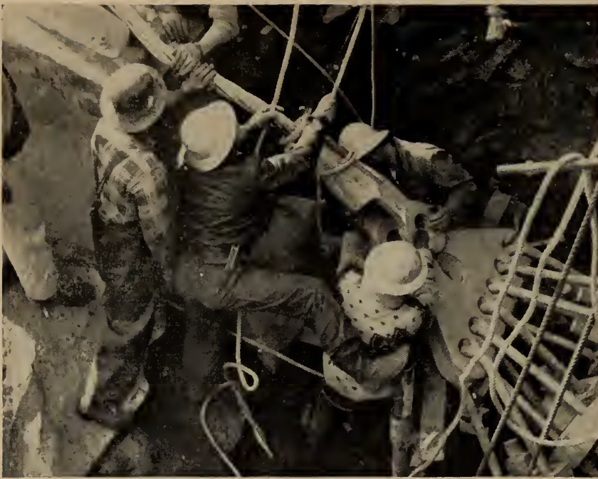
Fig. 8. Final closure at anchorage A.
