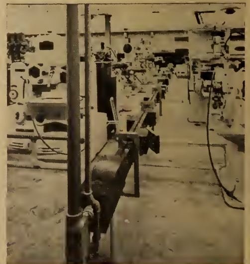
Fig. 9. Plug-in duct installations may be mounted near the ceiling (below) or at a convenient height just above the floor (right).
