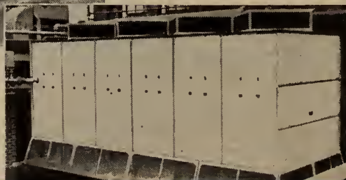
Evaporative condenser handling 330 tons of refrigeration
