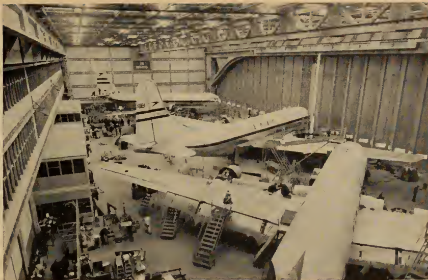
Interior view of a hangar in the B.O.A.C. hangar block.
