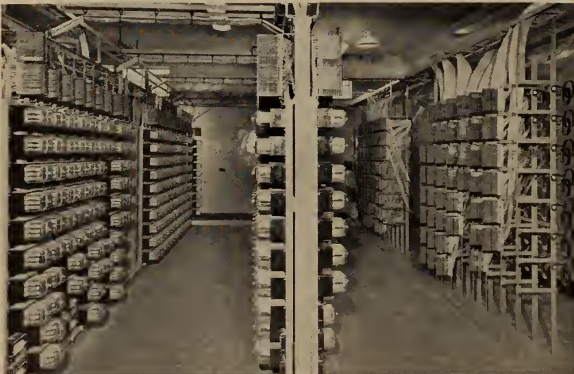
Airport lighting control equipment (apparatus room).
