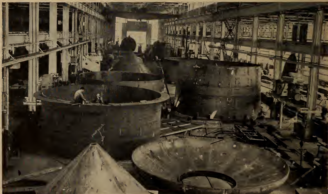
Fig. 3. Part of the plate shop during the fabrication and assembly of the 18 main sections of the catalytic cracking unit. Weights of sections ranged from 35 tons to 85 tons.
