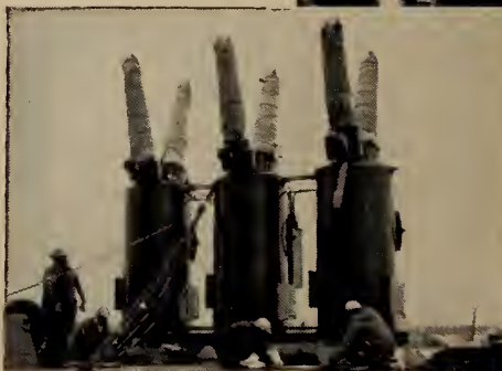
Huge Westinghouse step-up transformers like this are now being built at Westinghouse for the St. Lawrence Generating Station.
