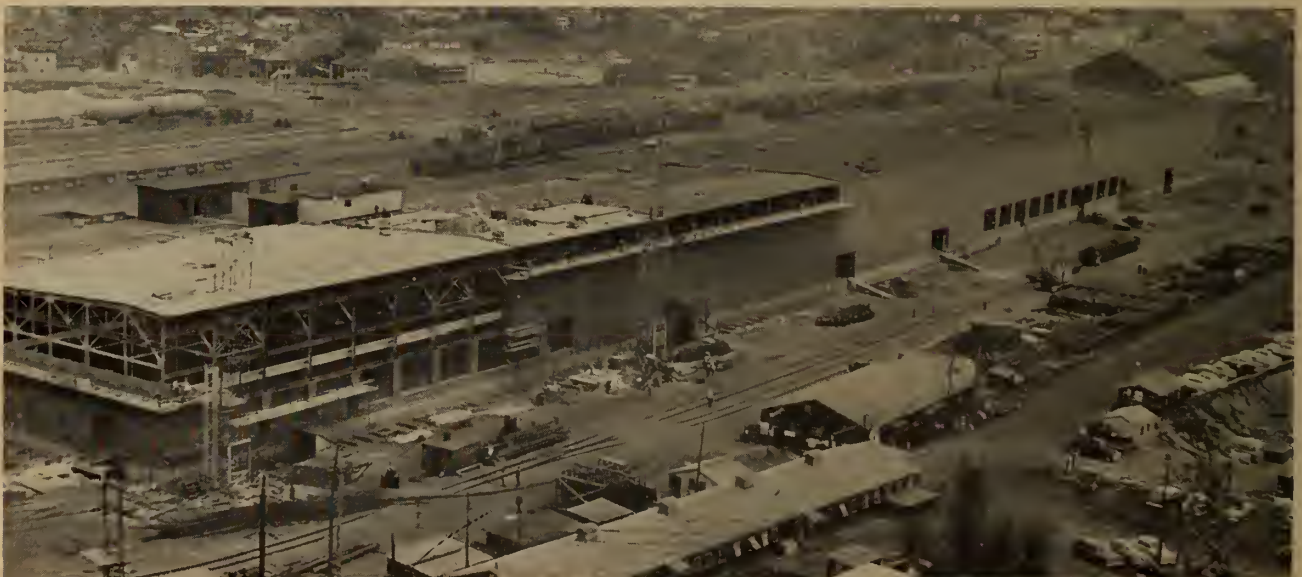
Fig. 9. General view of the new machine room nearing completion clearly shows the arrangement of the roof trusses with provision for their extension to house an additional paper machine.
