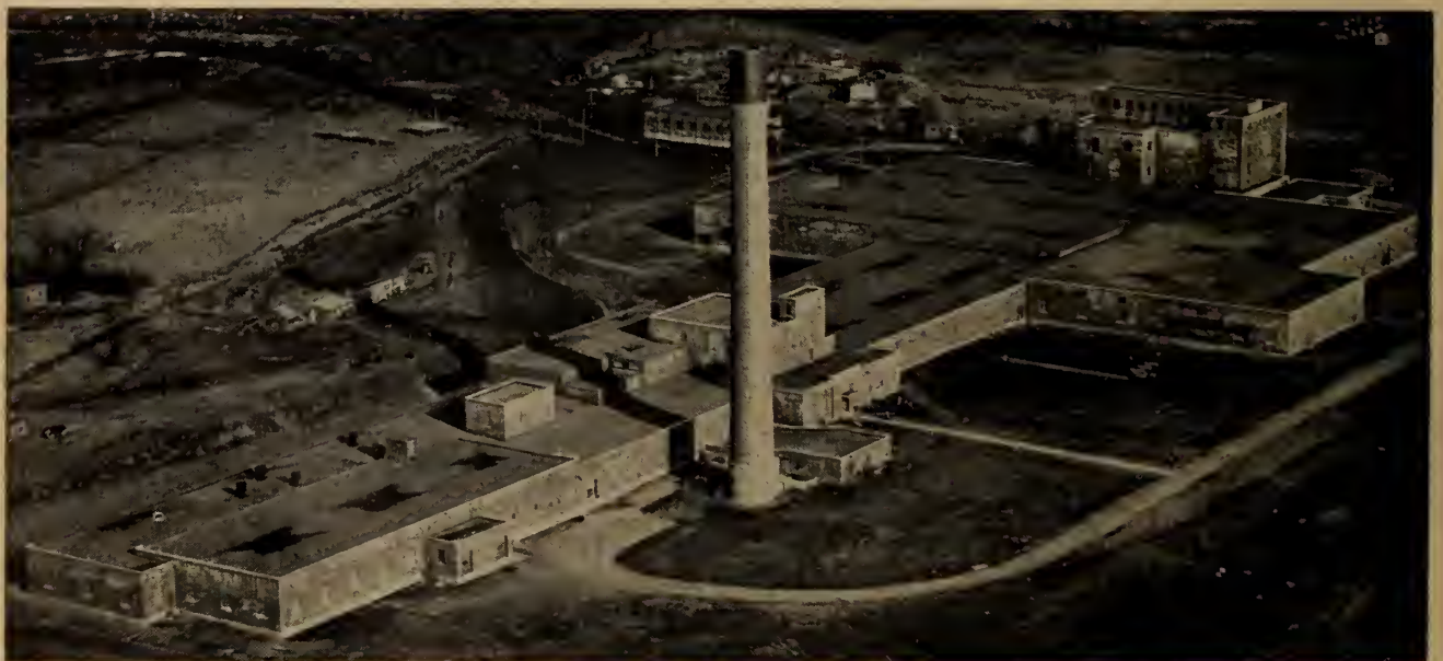
Fig. 2. Aerial view of No. 5 mill. Staple fibre plant at left, with foul air stack (15 ft. dia., 225 ft. high). Three-storey structure behind stack is the staple fibre acid preparation building. Central viscose plant adjoins, right centre, with churn house (five storeys) at far end. CS 2 storage building behind top of stack; sulphuric acid tanks at right centre.
