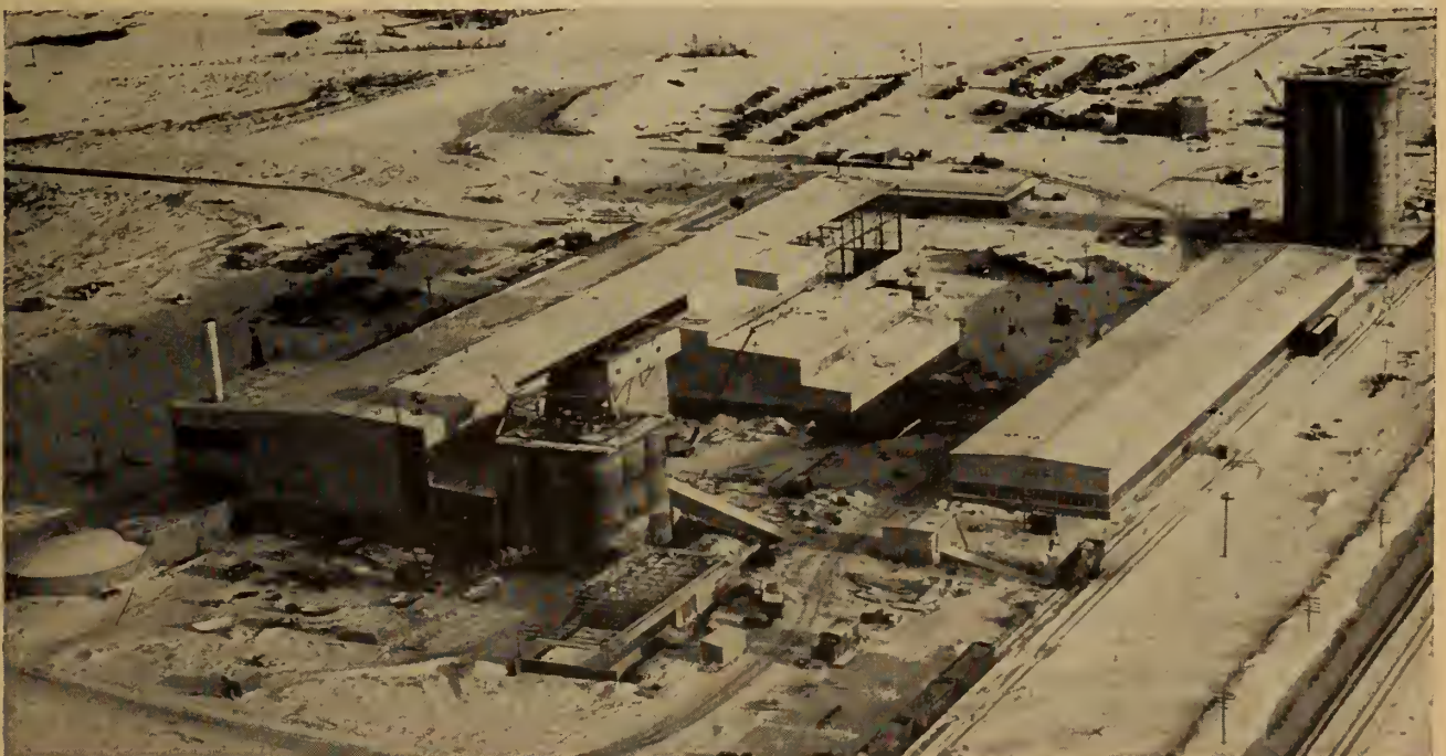
Fig. 10. Aerial view of the plant.
