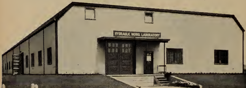
Front view of the Ontario Hydro Hydraulic Model Laboratory at Islington.
