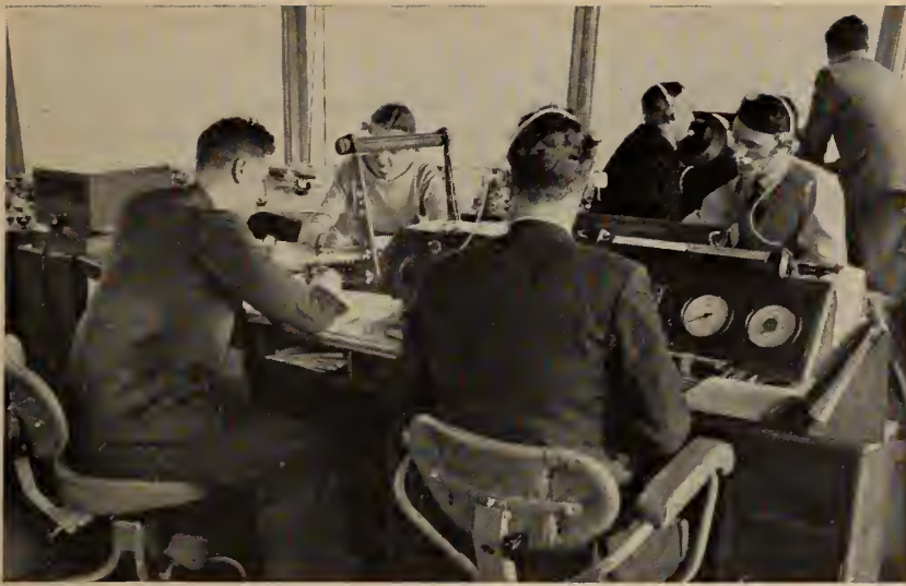
The control room on the ninth floor of the control building.
