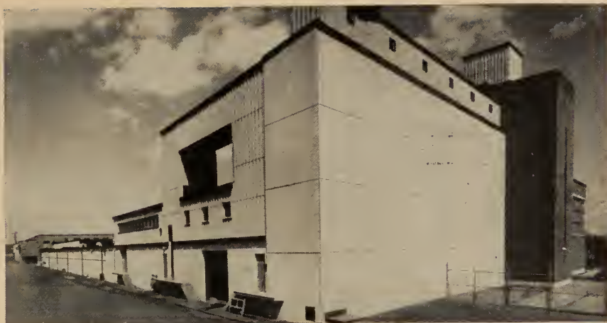
A general view of the new plant (from the right hand end of Fig. 1).
