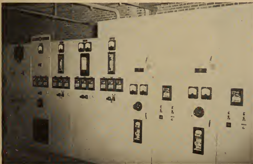
Fig. 10 (below). Main control switch-board.
