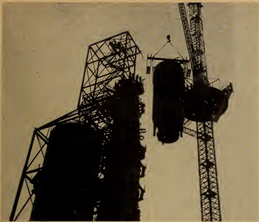
Fig. 7. The 85-ton catalyst disengager nearing the top of the cracking unit.
