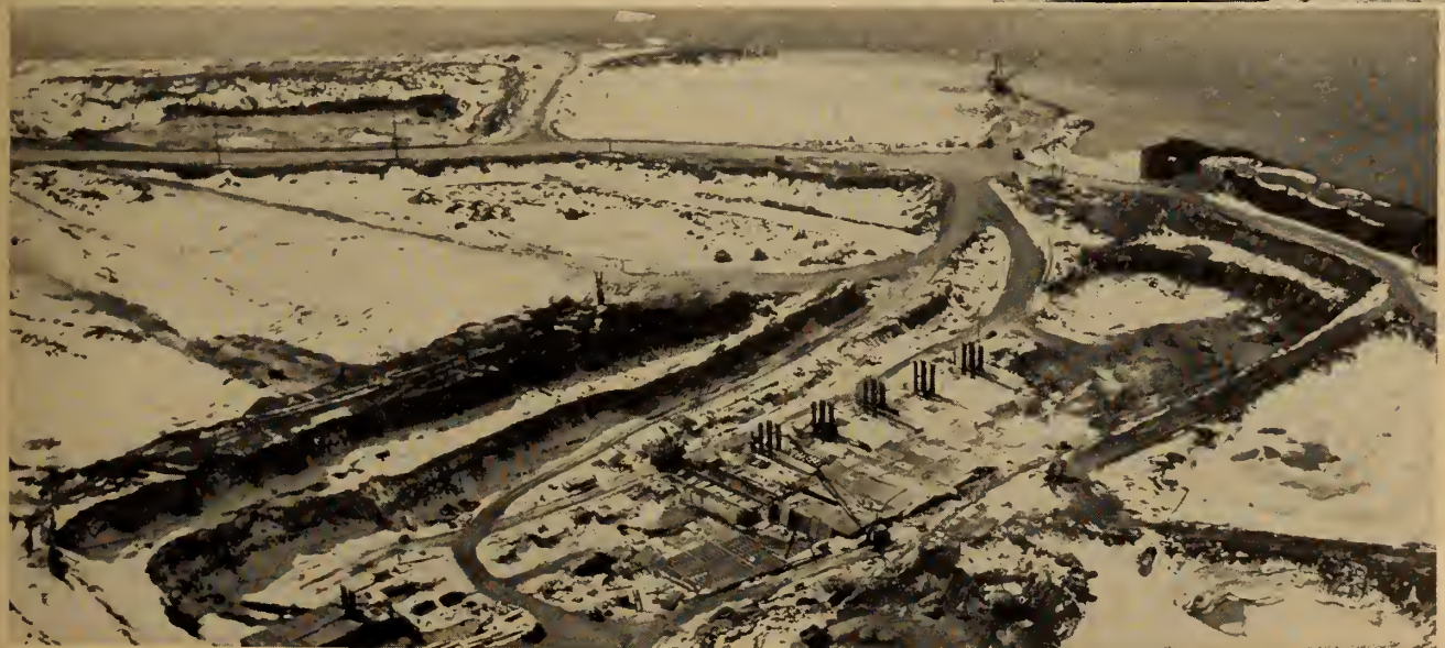
Iroquois dam. Excavation operations are in progress and concrete operations continue.
