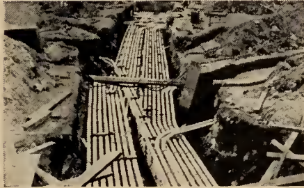
J-M TRANSITE DUCTS — Made of asbestos and cement. Transite Conduit and Korduct are inorganic and unaffected by electrolysis and corrosive soils. Long, lightweight lengths.
