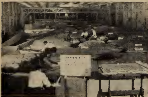
This giant model of the St. Lawrence built by Ontario Hydro measures flow problems.
