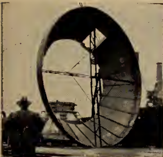
• Prefabricated sections of tank 80 ft. in diameter at the base.
