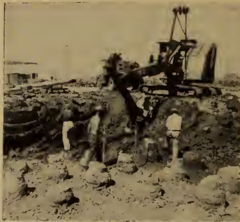
Fig. 3. Construction of the cement silos: left, excavating piles; right, sliding forms in position.
