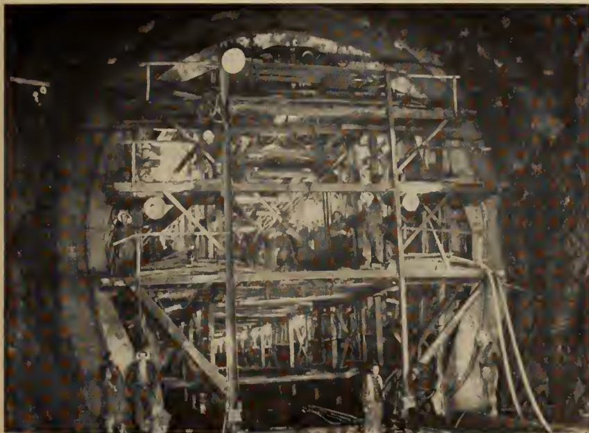
Fig. 15. Tunnel form used for concrete lining.
