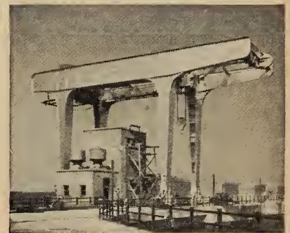
60-ton headworks gantry crane
