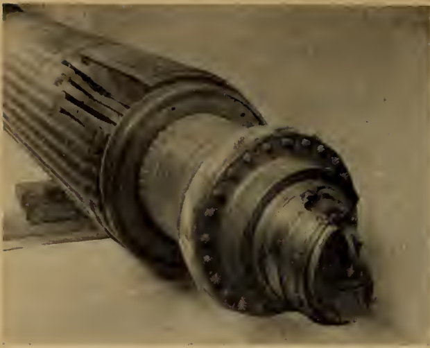
Fig. 29. Final condition of rotor.
