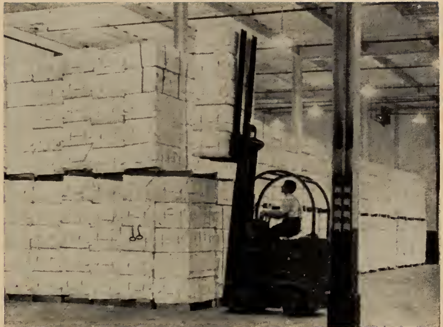
Fig. 6. Stacking 500-lb. bales of wood pulp in the pulp storage room of the central viscose plant. Battery-operated high-lift fork trucks are used.
