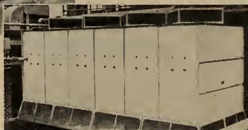
Evaporative condenser handling 330 tons of refrigeration
