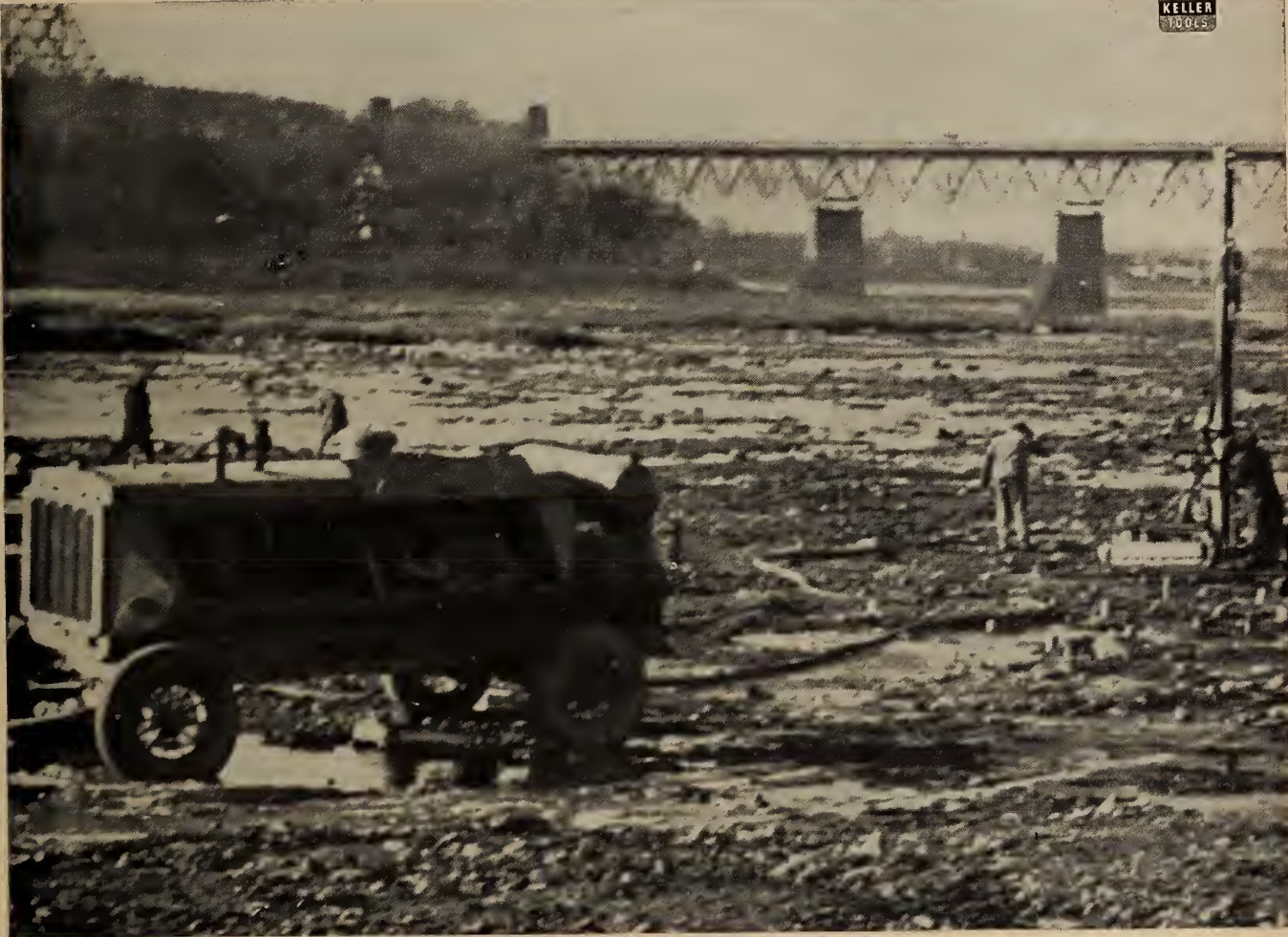
A Gardner-Denver portable compressor and Air Trac® drill making the first blast holes in the drained St. Lawrence River bottom.
