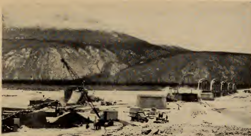
Donjek bridging project on the Northwest Highway System.
