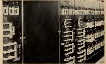
J-M ASBESTOS EBONY — A permanent high-dielectric panel board material. Won't rust, rot, shrink or buckle. Available in sheet form or in pre-fabricated shapes to order.
