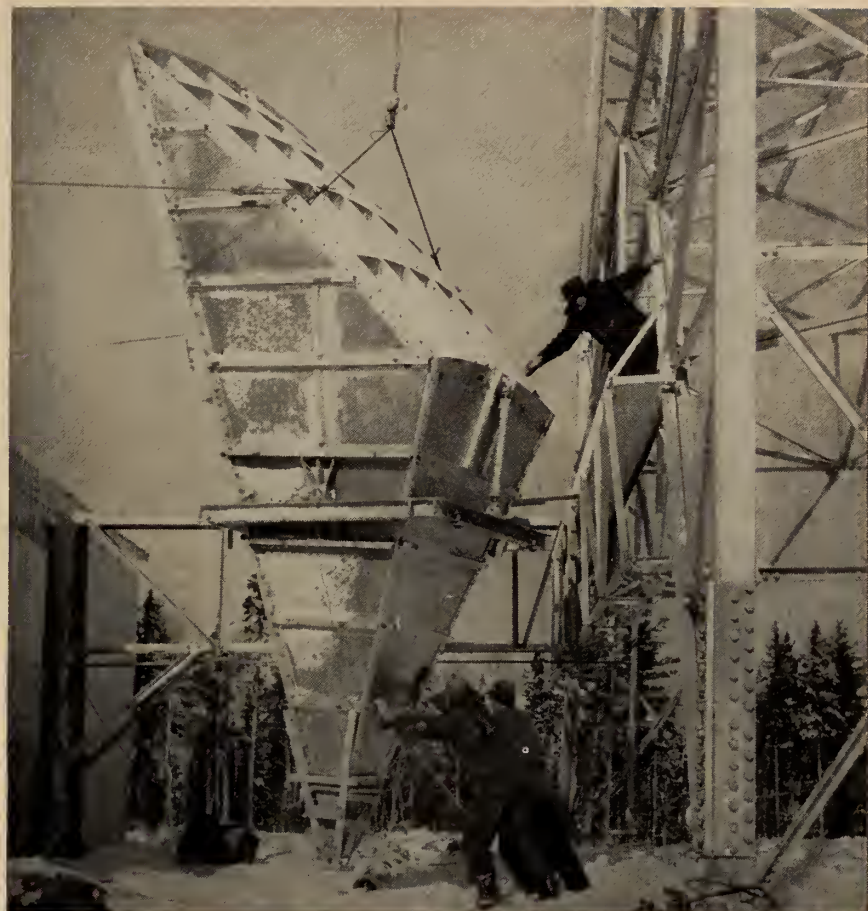
Fig. 5. Preparing to install the horn reflector antenna.
