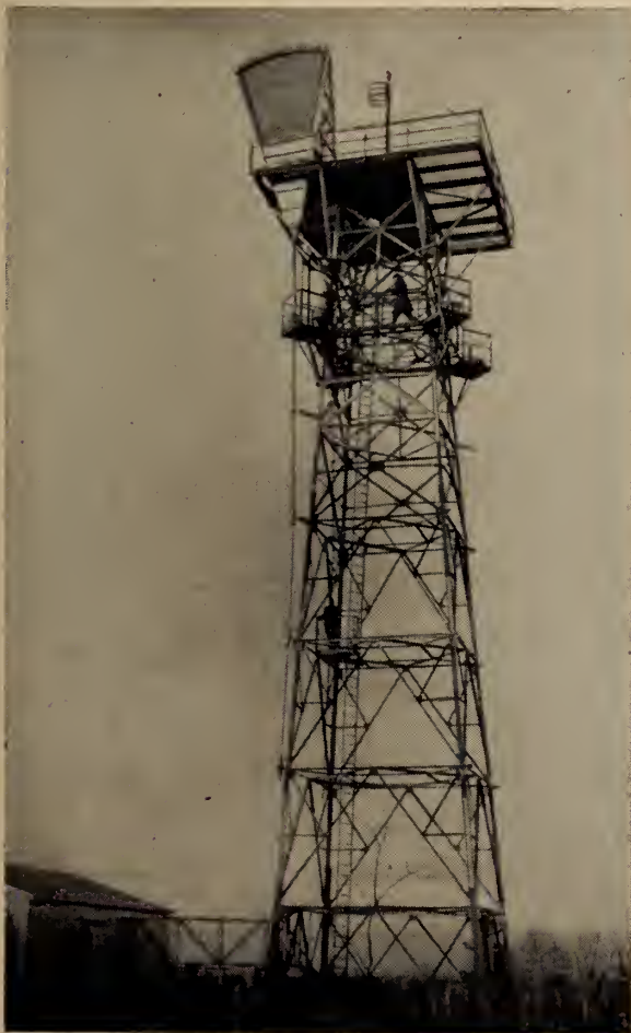
Fig. 12. View of part of the completed repeater station building and the associated tower at New Liskeard.
