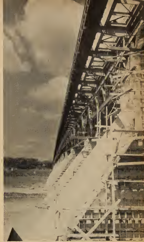
Piers of the Jacques Cartier Bridge are being enlarged.
