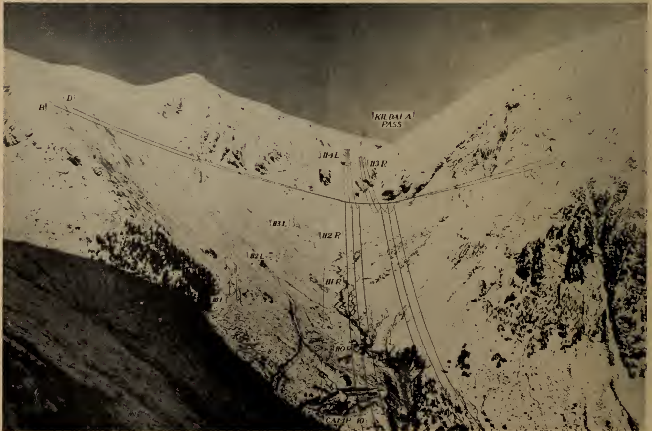
Fig. 1. A retouched panoramic view of the cross suspension system from Twin Peaks with Kildala Pass in centre background.
