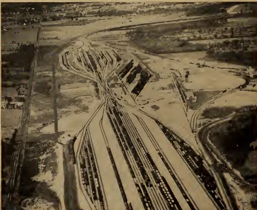
One aspect that may concern the engineer is the construction of all types of switch yards and improvement of existing facilities. (Photo: Canadian Pacific Railway)
