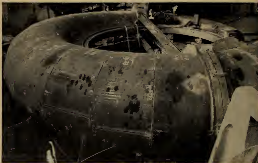
Fig. 13. Fabricated scroll case of 175,000 b.h.p. high head reaction turbine.
