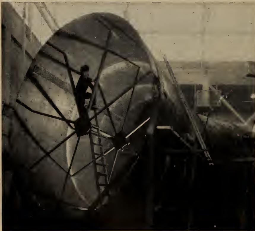
Fig. 8. Shop assembly of Niagara scroll case.
