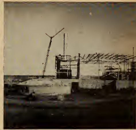
Fig. 2. Kiln dust cyclone collector (left); kiln chimney and slurry storage basin (right).
