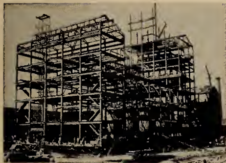
The new Hiram Walker & Sons Ltd. Distillery Building in Windsor, Ontario, uses approximately 30,000 Stelco High-Strength Bolts.
