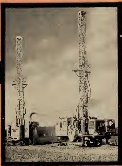
JOY 58-BH CHAMPION BLAST HOLE DRILL For primary blast hole drilling on deep cuts, outperforms churn drills five-to-one.
