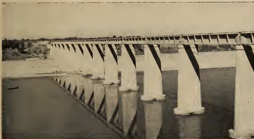
The Mahi Bridge, India, nearing completion.
