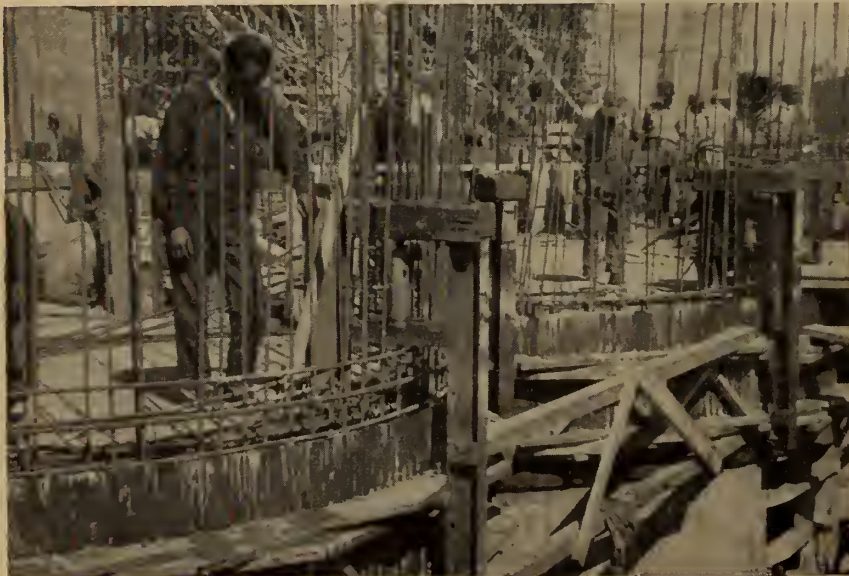
Fig. 6. Construction of the slurry silos with sliding forms.
