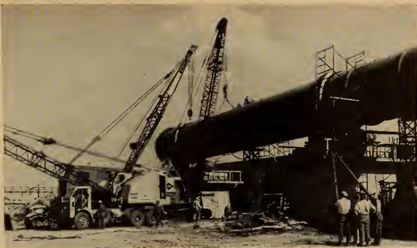
Fig. 5. Lifting a section of the kiln, at the east end.
