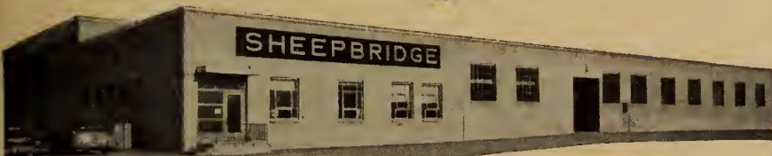
The new Sheepbridge plant at Guelph, Ontario.
