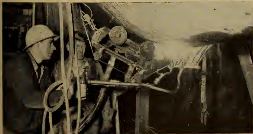
Fig. 45. Low temperature stress relieving of field weld.
