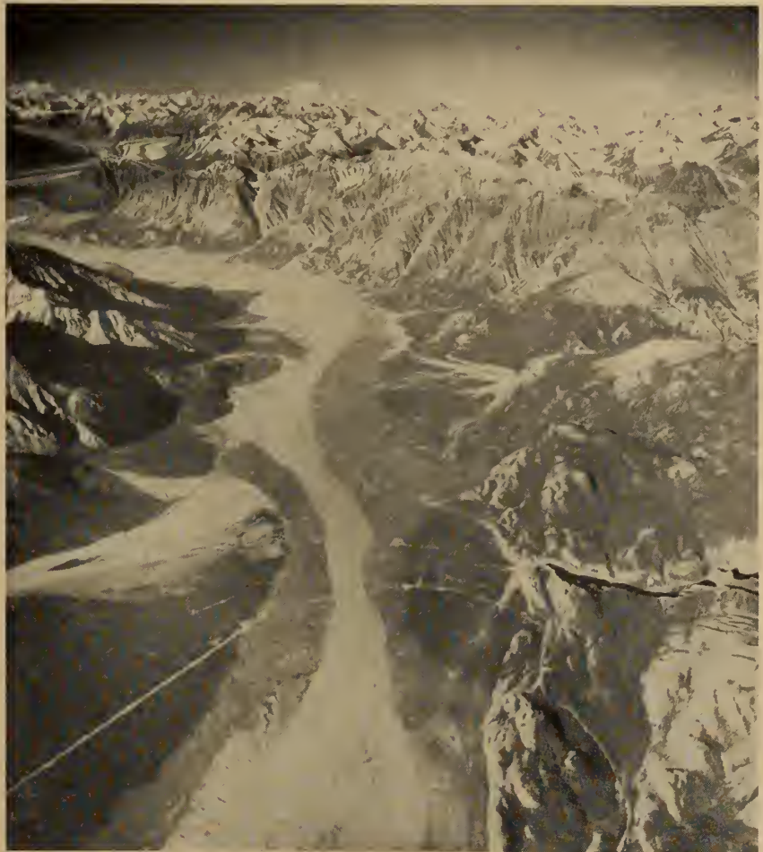
Fig. 1. Slims River, Mile 1059, is one of the typical glacier-fed streams crossed by the Alaska Highway. The crossing in the foreground is part of the pioneer road and the existing crossing is located three miles downstream. Identifiable in the background are mountains of the St. Elias Range including Mount Logan (El. 19,850 ft.) to the right, Mount Vancouver (El. 15,700 ft.) just left of the center, and Mount Hubbard (El. 14,950 ft.) to the extreme left.
