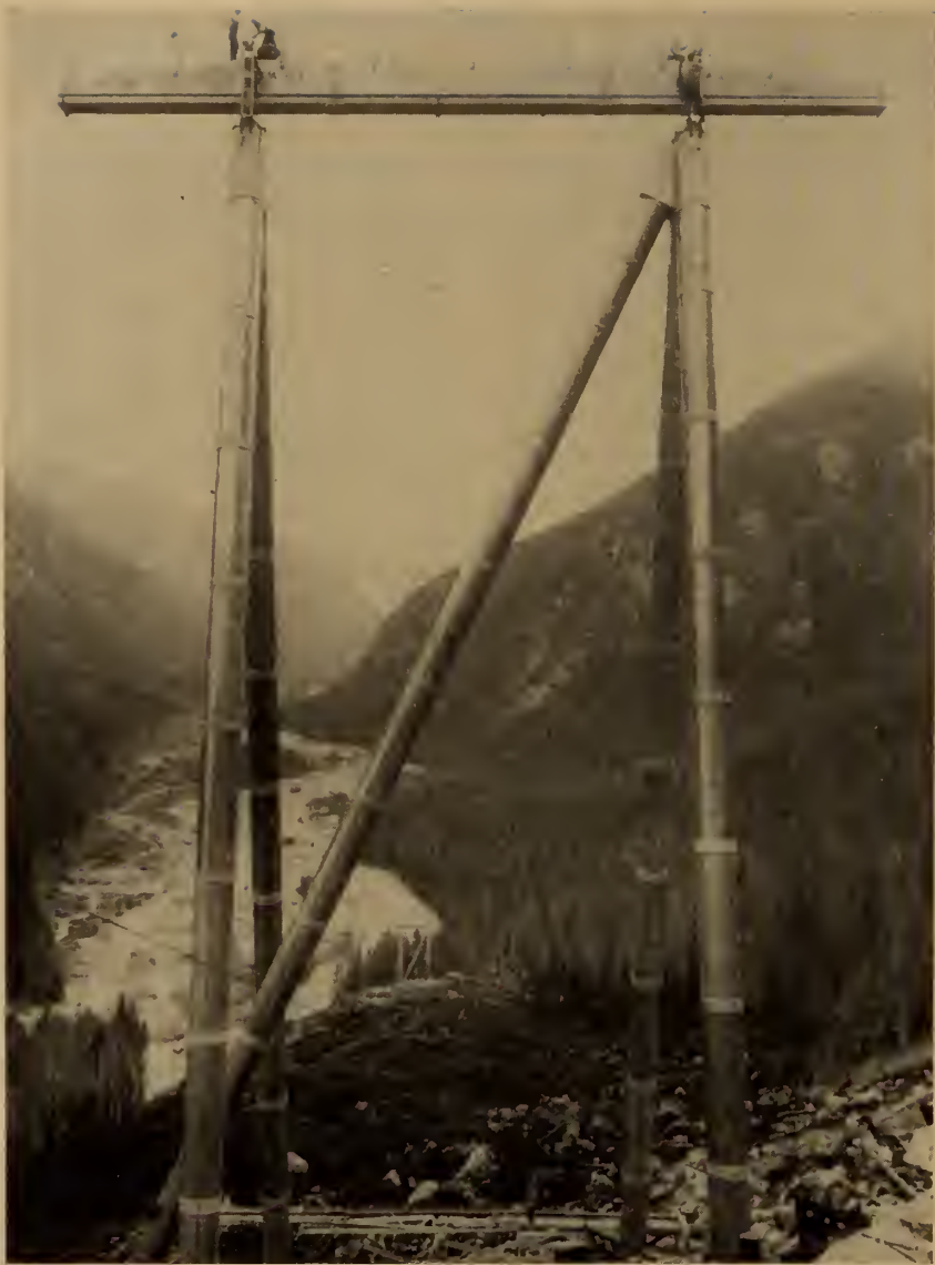
Fig. 60. Erection of aluminum tower.
