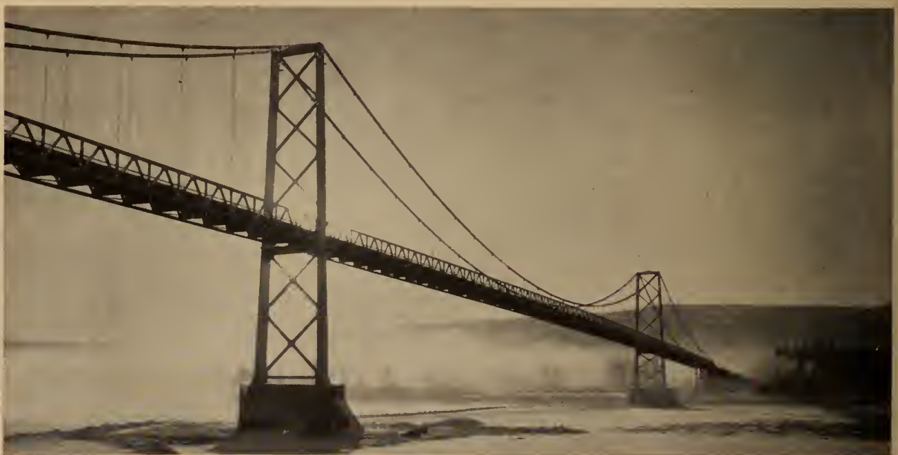
Fig. 5. The Peace River bridge at Mile 35, with an overall length of 2,267 feet, the centre span being 930 feet.
