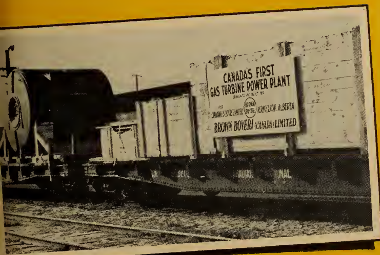
CANADA'S FIRST GAS TURBINE POWER PLANT—enroute for erection at Canadian Utilities Ltd. plant, Vermillion, Alberta.
