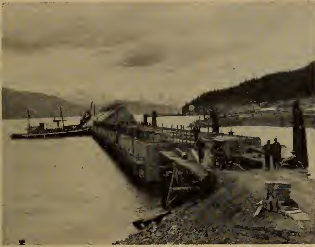
Fig. 84. (Left)—The caissons in place and the third being careened into place.
