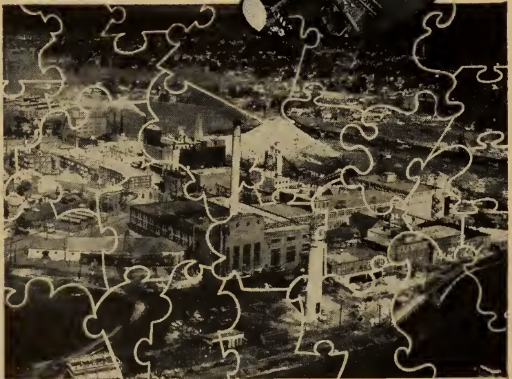
Howard Smith Paper Mills, Cornwall, Ontario, housing Canada's largest fine paper machine, installed by Provincial Engineering Ltd.
