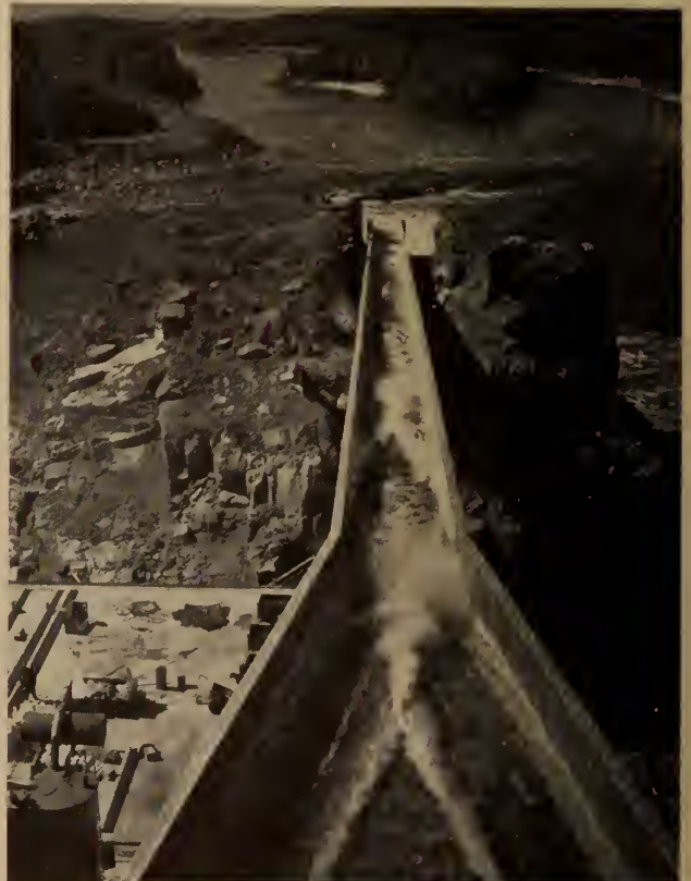
Fig. 10. Prototype flow in Peribonka No. 1 log chute.
