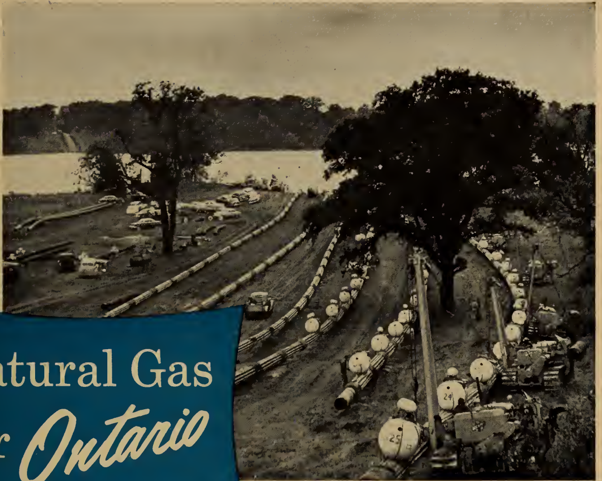
Preparing for dual crossing of Niagara River
