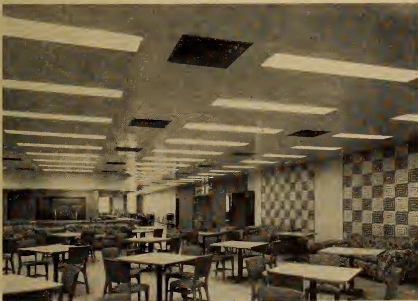
Fig. 12. Finished ceiling system of cafeteria in Manufacturers Life Building.
