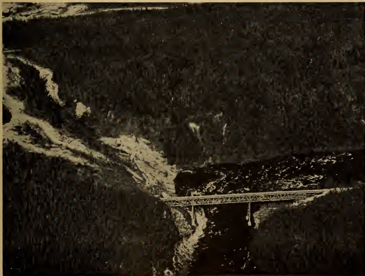
Moisie River Bridge at Mile 12 (Rodrigrey).
