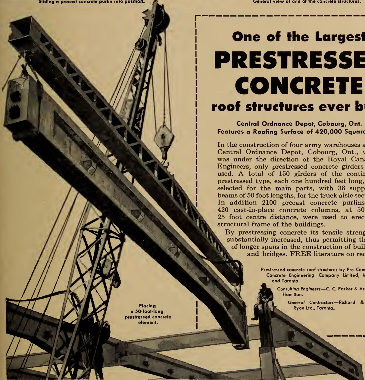
Sliding a precast concrete purlin into position.
