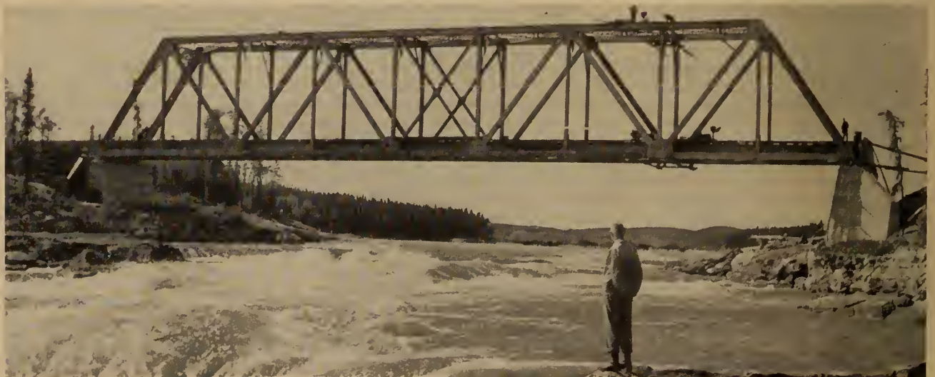
Fig. 2. 201 ft. 4 in. through truss crossing north channel of Churchill River.
