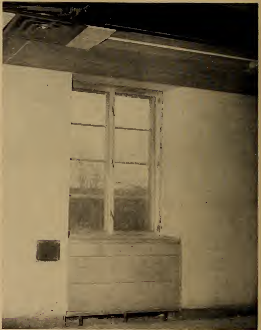
Fig. 9. Typical window installation in Manufacturers Life Building.
