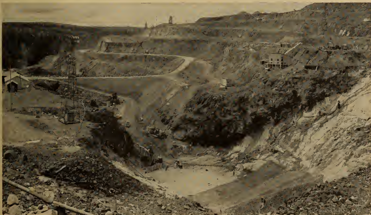
Fig. 5. Damsite before placing of core material was started, looking upstream.
