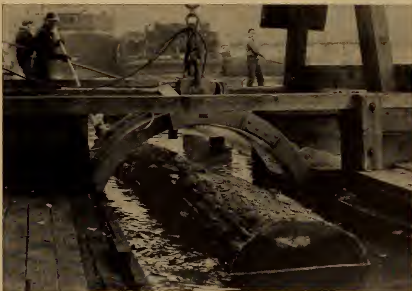
Fig. 2. A log passing through coil of metal detector.
