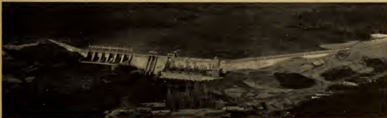
Fig. 17. Chute-à-la-Savane, looking north. Left to right: west wingwall, sluice gates, regulating gates, log chute, headblock and powerhouse, east wingwall. The aluminum switching station is in the foreground.
