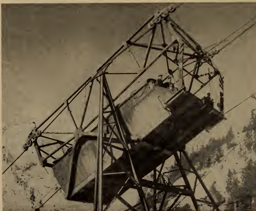
Fig. 40. The 25-ton tramway carried men and cargo from Kemano Camp 5 to the camps at the 1,600 and 2,600 foot elevation.
