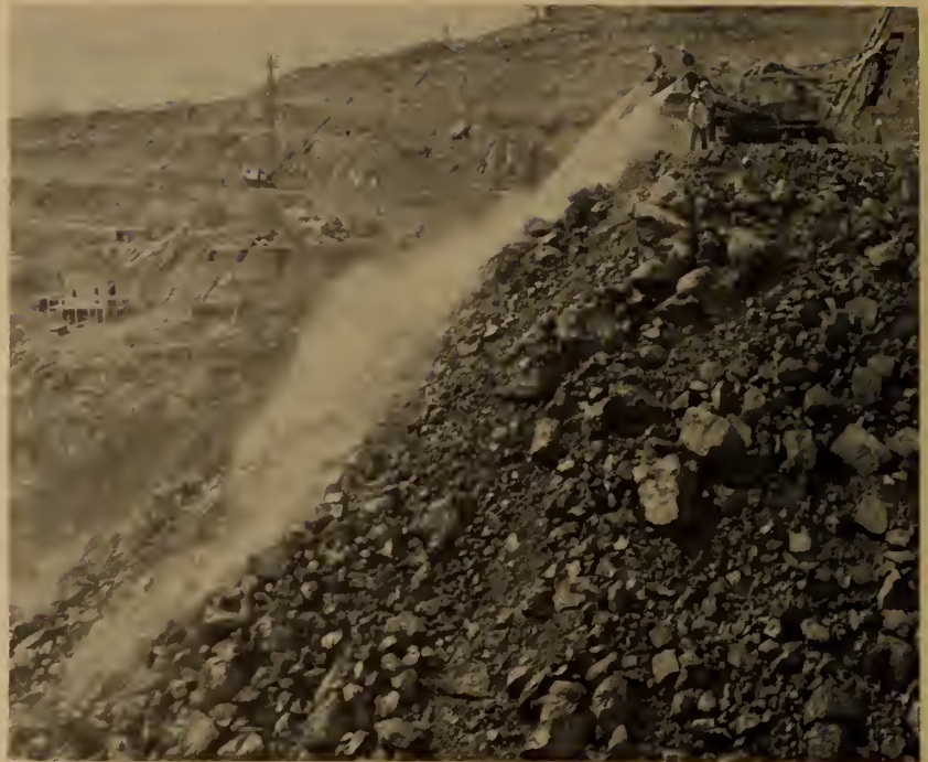
Fig. 9. Sluicing dumped rock fill.
