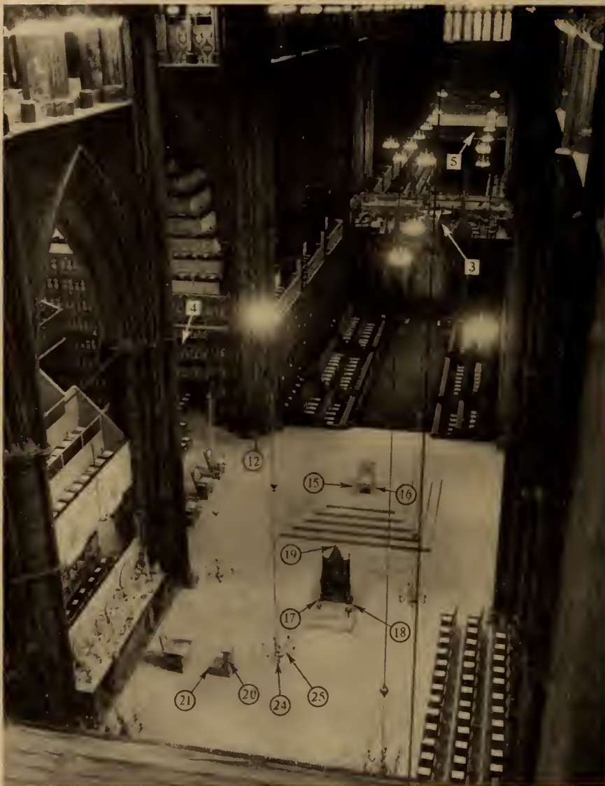
Fig. 4. View of Westminster Abbey from the triforium, near No. 2 camera position, showing some of the camera and microphone points and part of the special lighting.
