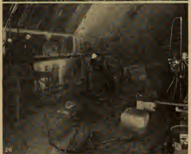
Fig. 23. The upper half of the pilot tunnel that was "raised" as the first step in excavating the inclined penstock.
