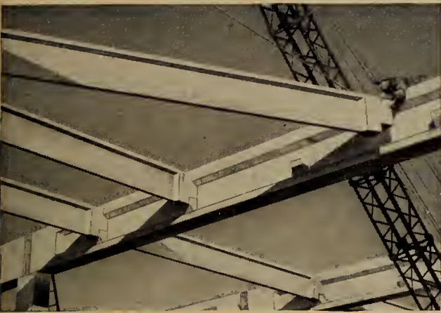
Sliding a precast concrete purlin into position.
