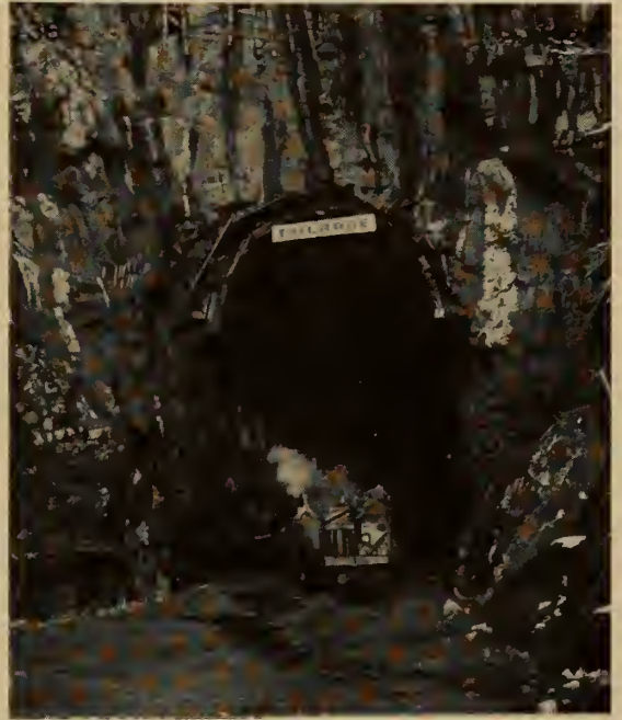
Fig. 34. Weak rock and tailrace branch intersections were protected by concrete. (Top Left)
