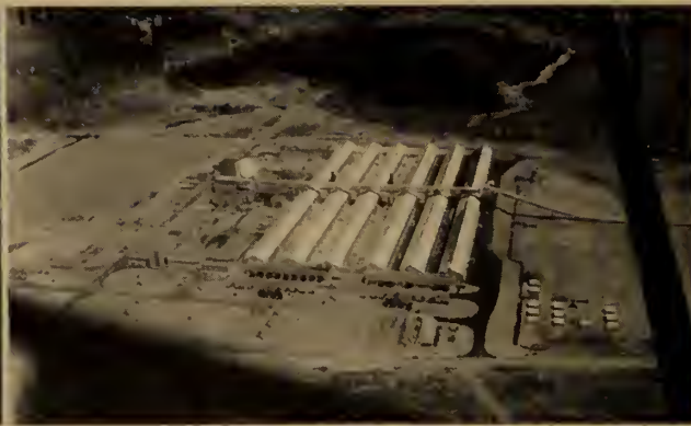
Fig. 121. Aerial view of smelter, showing conveyor gallery crossing potrooms to the carbon paste plant at left.
