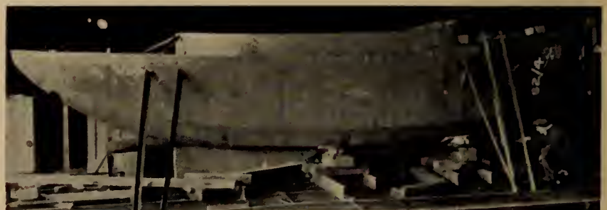
Fig. 4. Welded 28-foot double-chine towing launch; lifting weight, 4 tons.
