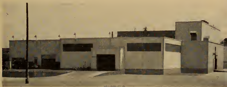
Extension of No-Co-Rode plant, Cornwall, Ont., built of "SIPOREX"
