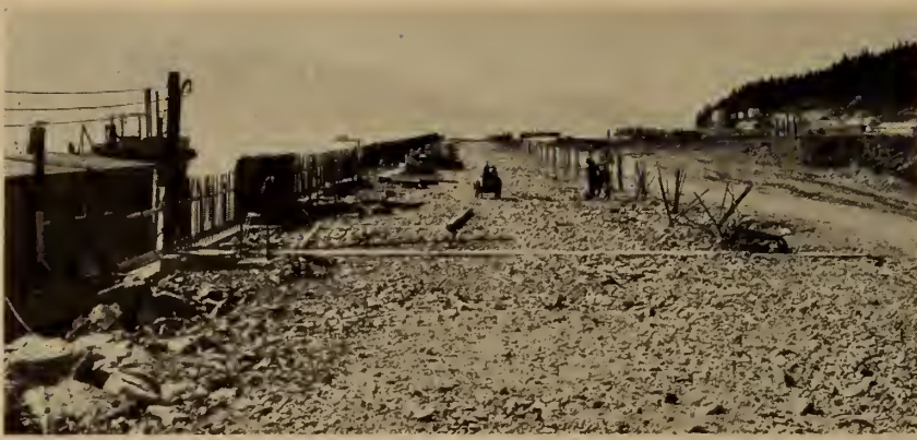
Fig. 87. Looking south along wharf, backfill completed.
