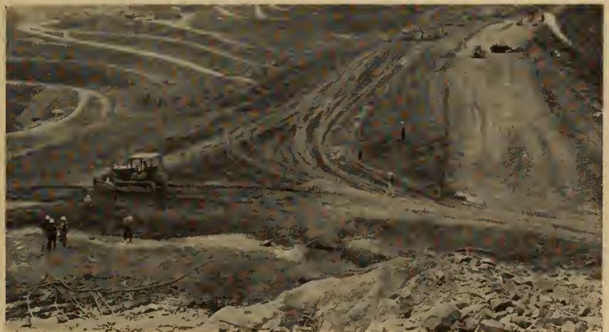
Fig. 10. Placing of core and downstream filters.
