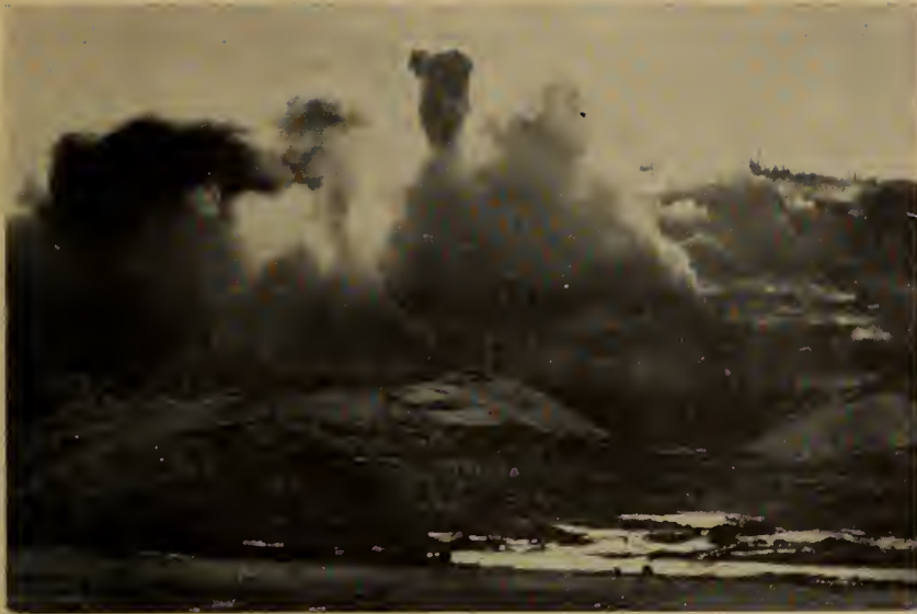
Fig. 7. Coyote hole blast in quarry.
