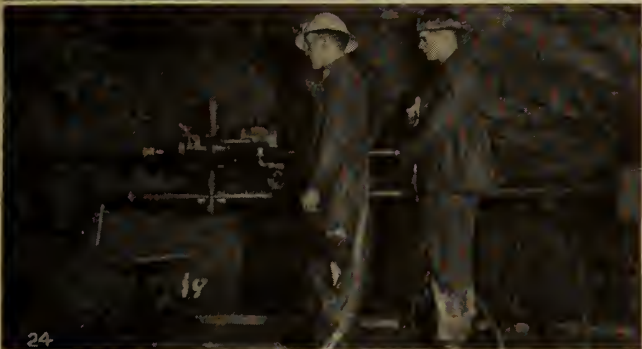
Fig. 22. Timbers hung from "bull horn" steel bars carry the walkway and skip for serving the pilot tunnel of the inclined shaft.
