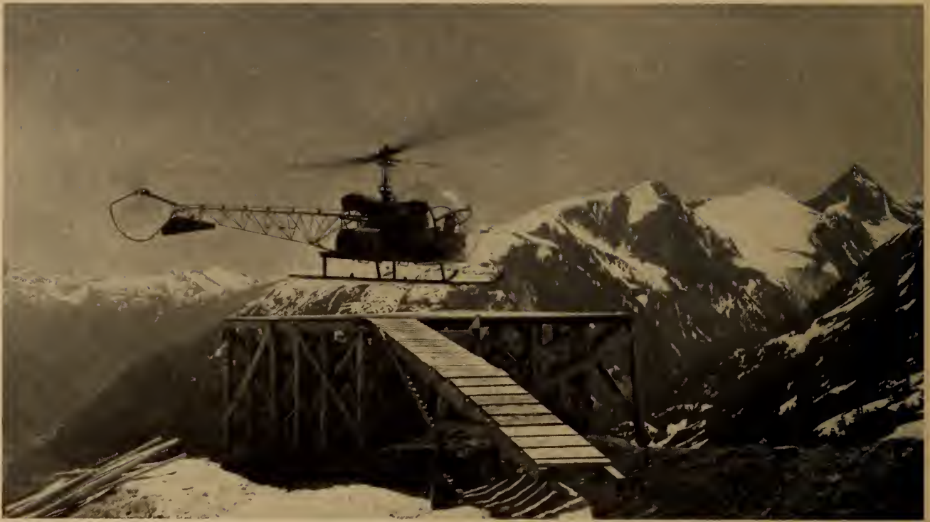
Fig. 54. Helicopter landing platform.
