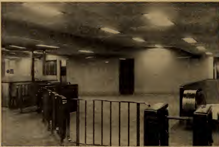
Fig. 2. Lighting of a typical control area.
