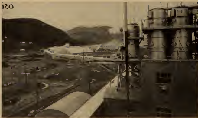
Fig. 120. Plant conveyor system as seen from Kangaroo crane. Smelter plant in background, storage building in center, and part of pneumatic unloading plant in foreground.
