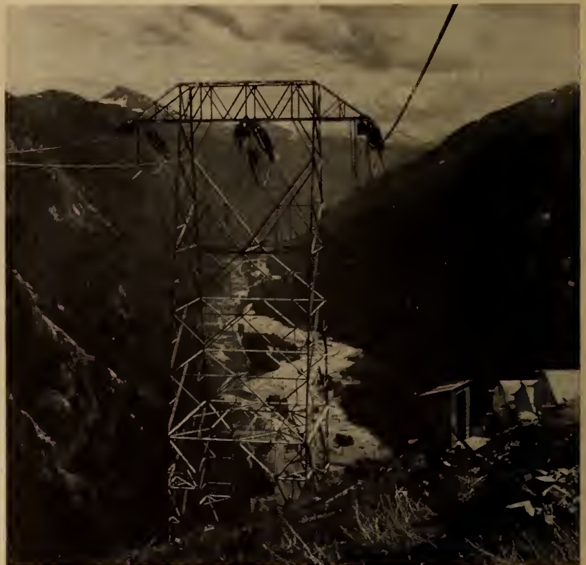
Fig. 58. Stringing operations on single circuit strain tower. Kemano valley in background.
