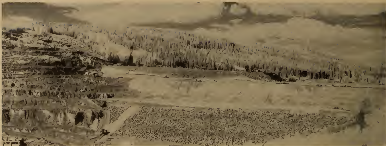
Fig. 11. Dam approaching full height.
