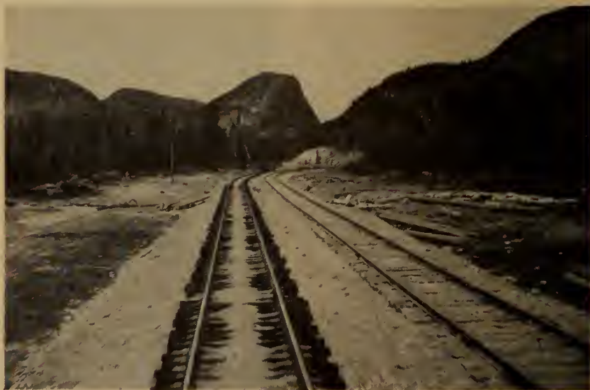
Finished track; rock ballast to be placed later.
