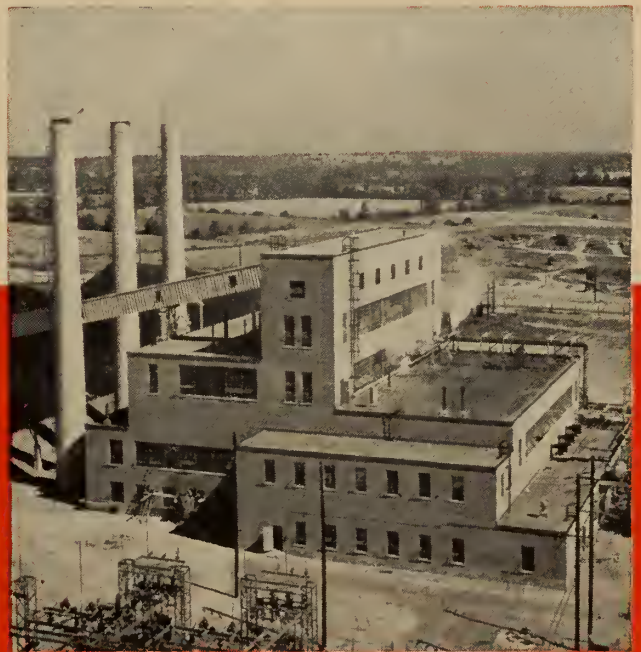
View of power house.
