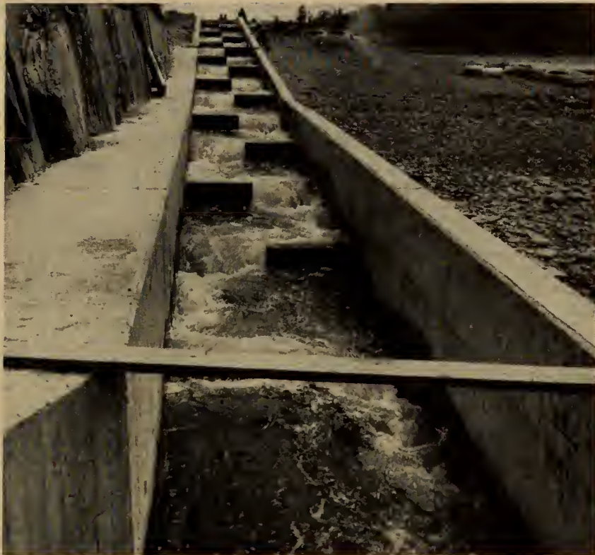
Fig. 4. Tobique Fishway. Lower leg from No. 1 entrance looking upstream.
