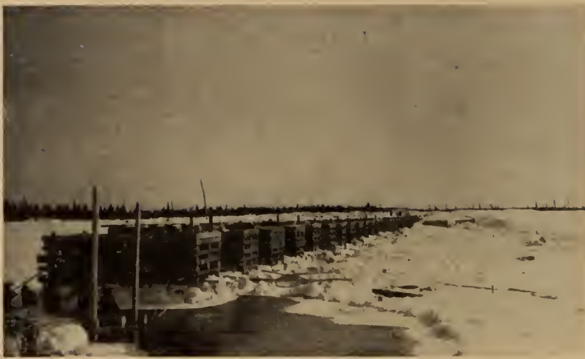
Winter construction of the coffer-dams.
