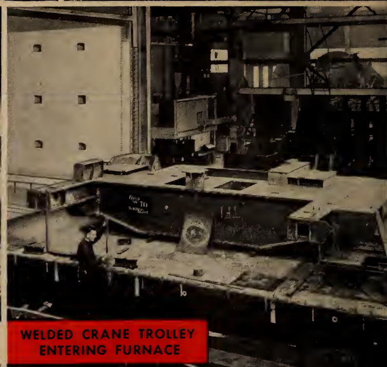
STRESS RELIEVING FURNACE
