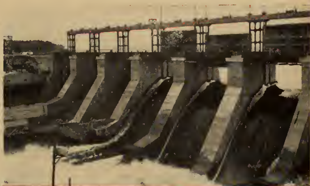
Peribonka No. 1 Spillway—located at Chute du Diable, Quebec. Owner: The Aluminum Company of Canada, Ltd.; Engineers and Contractor same as Peribonka No. 1 Powerhouse.
