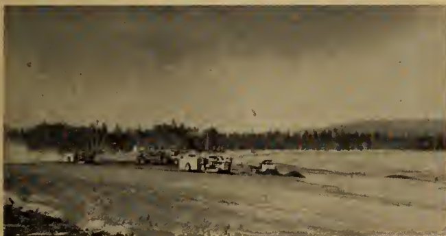
Fig. 96. (Above) Placing operations for compacted gravel fill.
