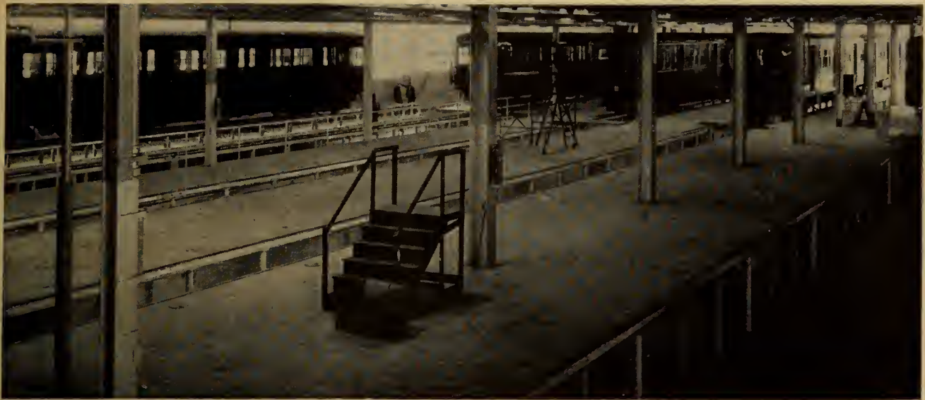
Fig. 3. An interior view of the Davisville Shop.
