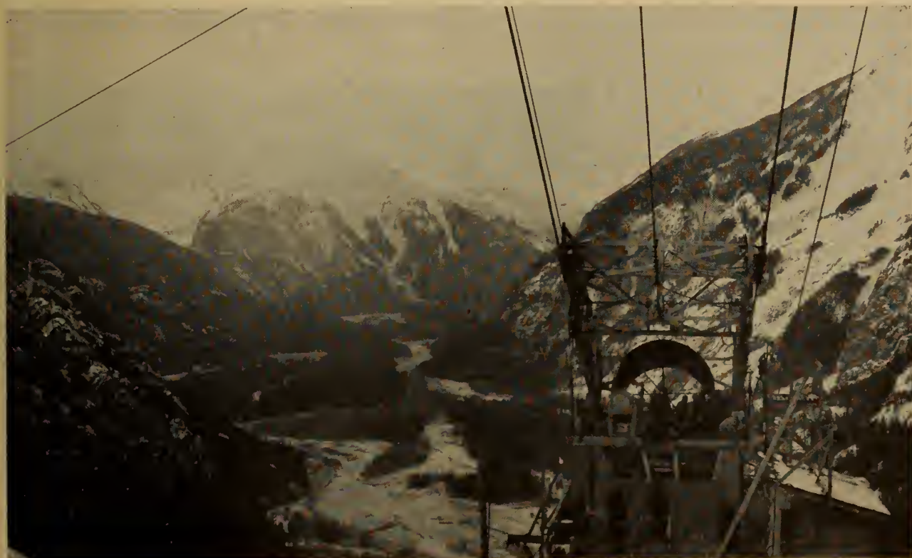
Fig. 42. Lifting penstock liner section by cableway from Kemano valley to El. 2600.
