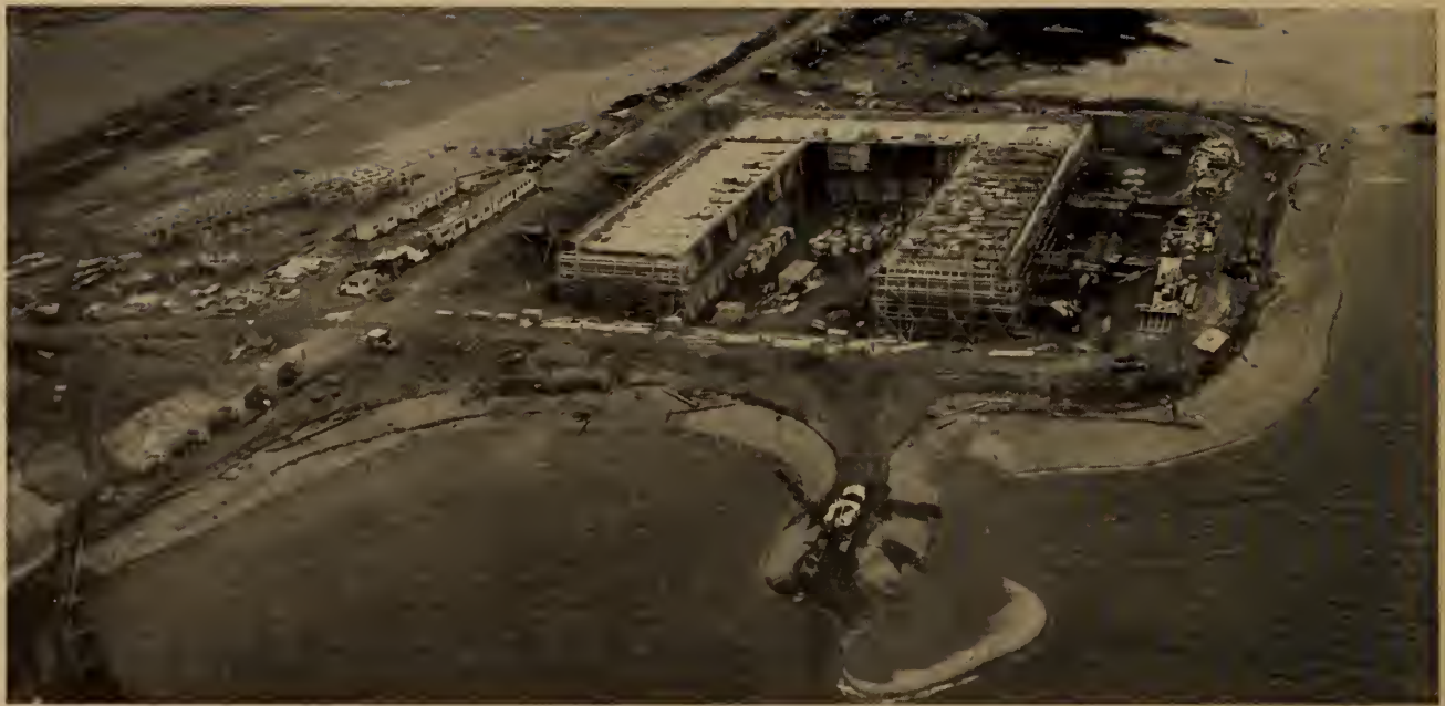
Fig. 79. The three caissons in the graving basin.
