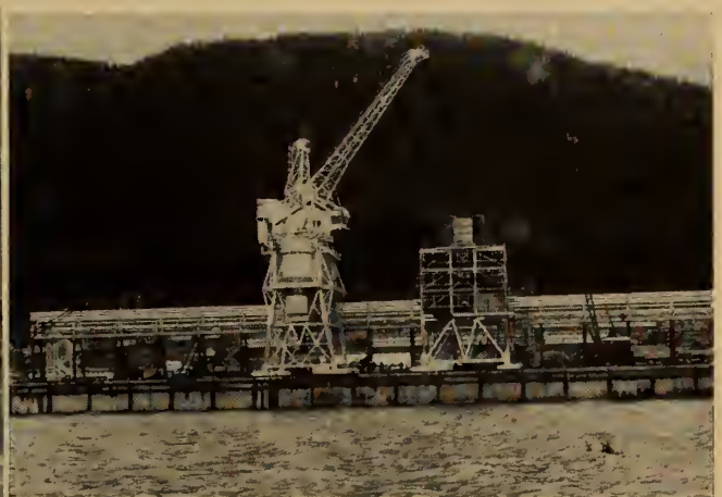
Fig. 119. Kangaroo crane—shown helping in assembly of pneumatic unloading plant.
