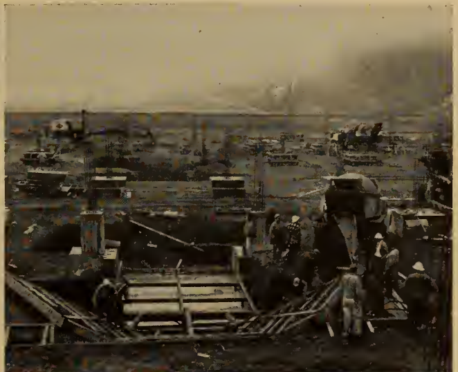
Fig. 96. (Above) Placing operations for compacted gravel fill.
