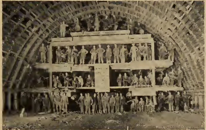
Record Breaking Heading Crew, Niagara River Hydro-Electric Development.
