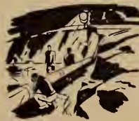
F-M Portable Electric Plants for operating tools and flood lighting
