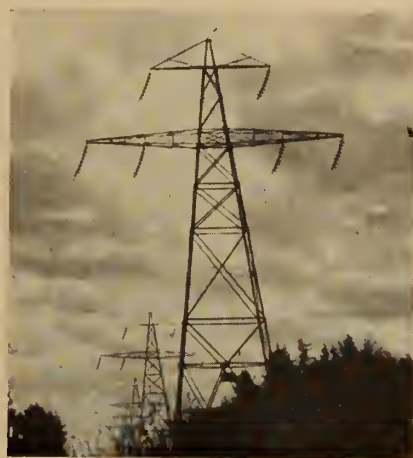
Fig. 5. Conductors swing in the wind.
