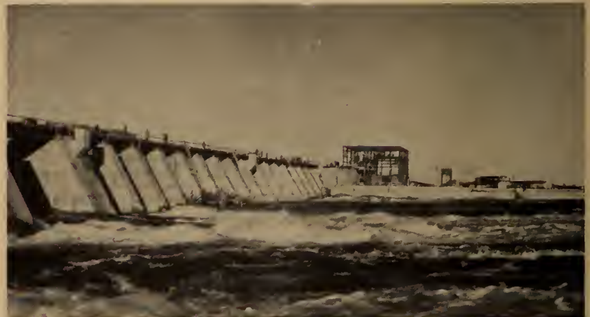
Downstream, the powerhouse in the background.
