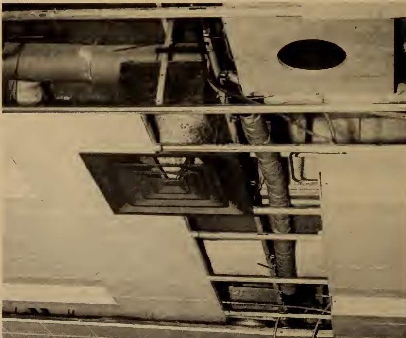
Fig. 10. Portion of partially completed ceiling in Manufacturers Life Building.
