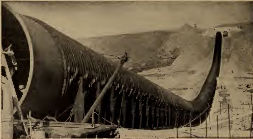
The above view shows our thirteen foot inside diameter continuous Wood Stave Pipe installed as a syphon between irrigation ditches on either side of a coulee in the St. Mary's River Irrigation Development. Ease of installation and long life were major reasons for this installation.
