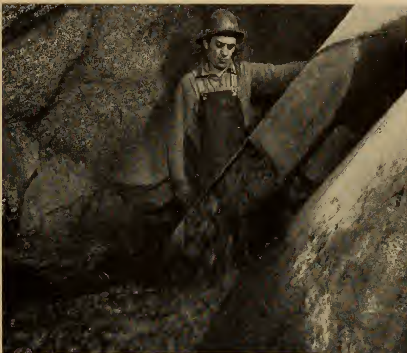
Fig. 46. Placing coarse aggregate outside liner.
