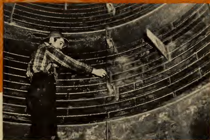
This new fractionating tower at Imperial Oil's Ioco Refinery is lined with Monel strip to resist corrosion present. Monel's strength, toughness and ease of fabrication were necessary, too, for this application.
