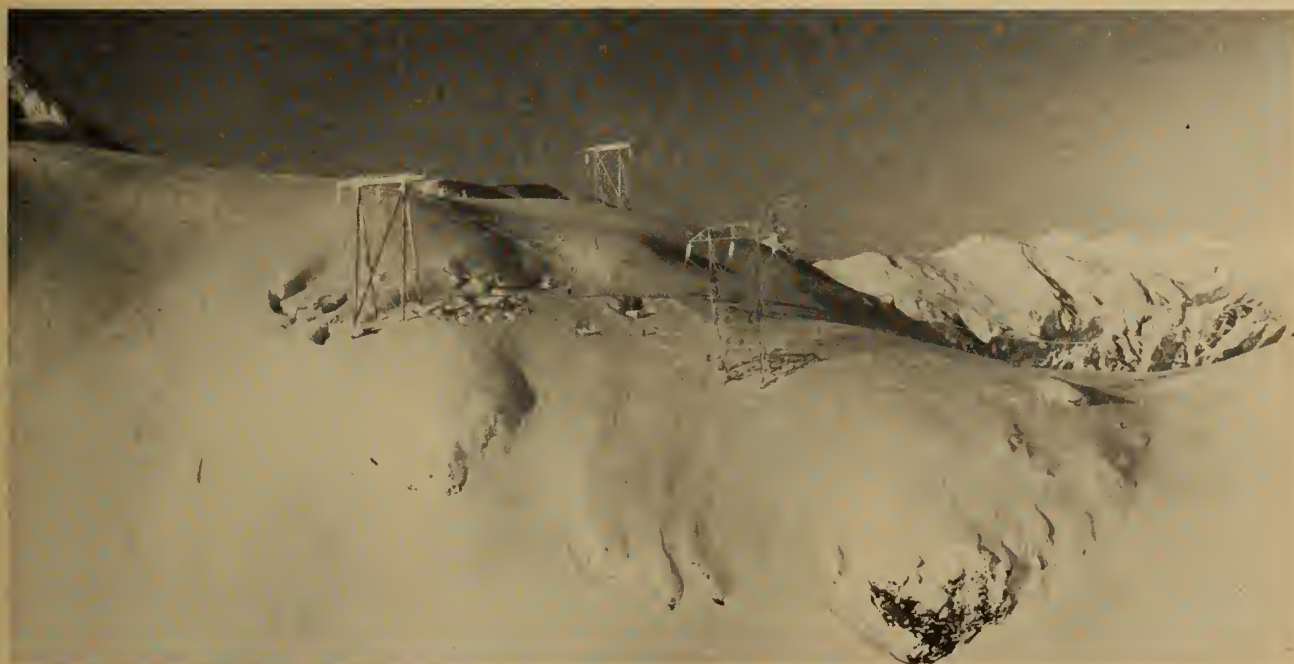
Fig. 59. Kildala Pass in winter, before completion of stringing operations on left line.
