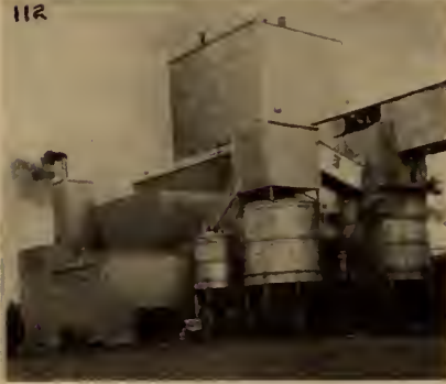
Fig. 111. Potroom buildings under construction showing progress of concrete, structural steel and aluminum cladding.
