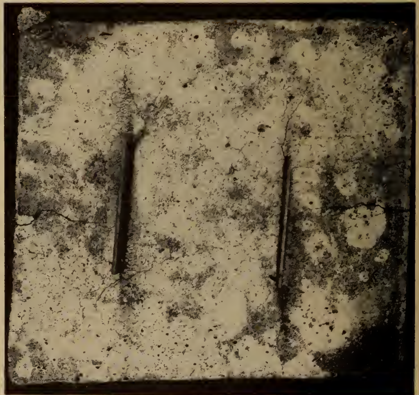
Fig. 4. A typical cracked block. St. Mary's Portland cement block 1:3:0 mix.
