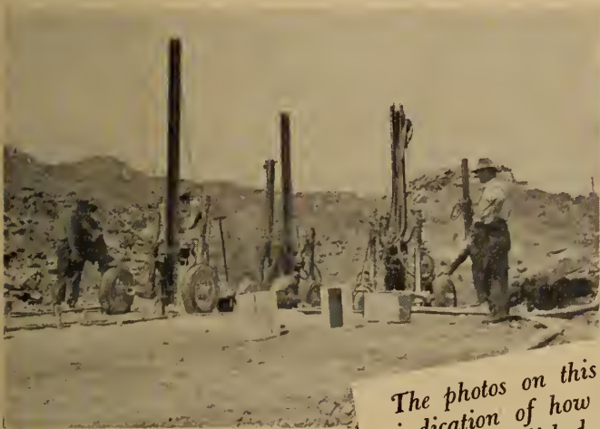
Wagon-mounted Drifter-drills on the canal section of the project. Similar drills cut an access road down the steep side of the Niagara Gorge to facilitate construction of the Generating Station.
