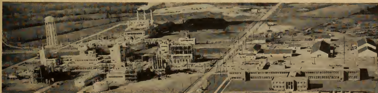
Fig. 1. Aerial view of the plant.
