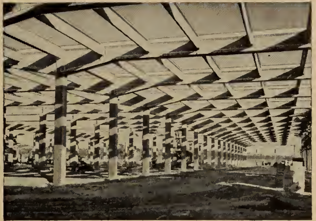
General view of one of the concrete structures.
