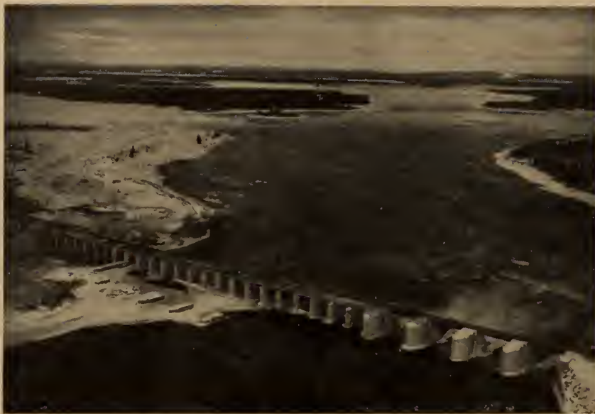
Upstream view of the site.
