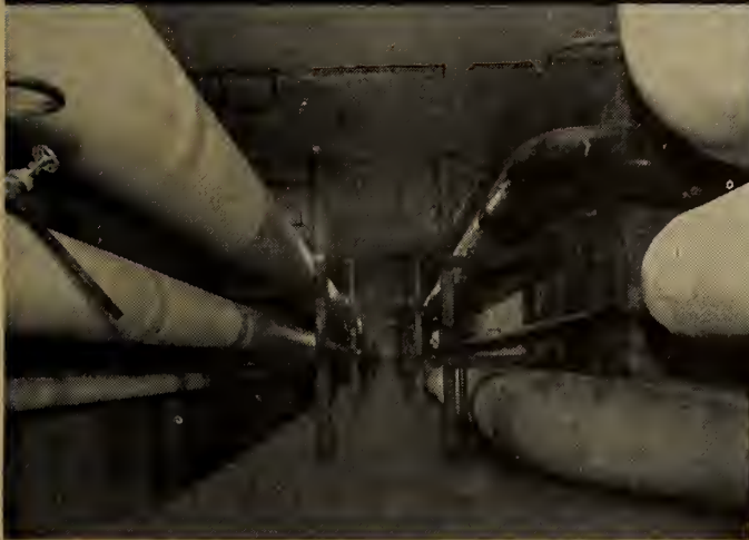
(Above) A partial view of the 1700 foot underground tunnel which houses mains carrying steam and water from power house to assembly plant.
