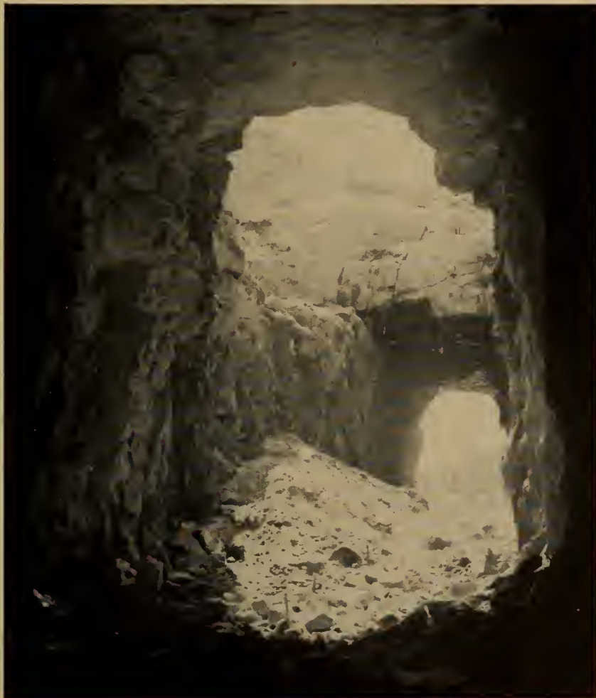
Break through at south portal of tunnel at Mile 12.
