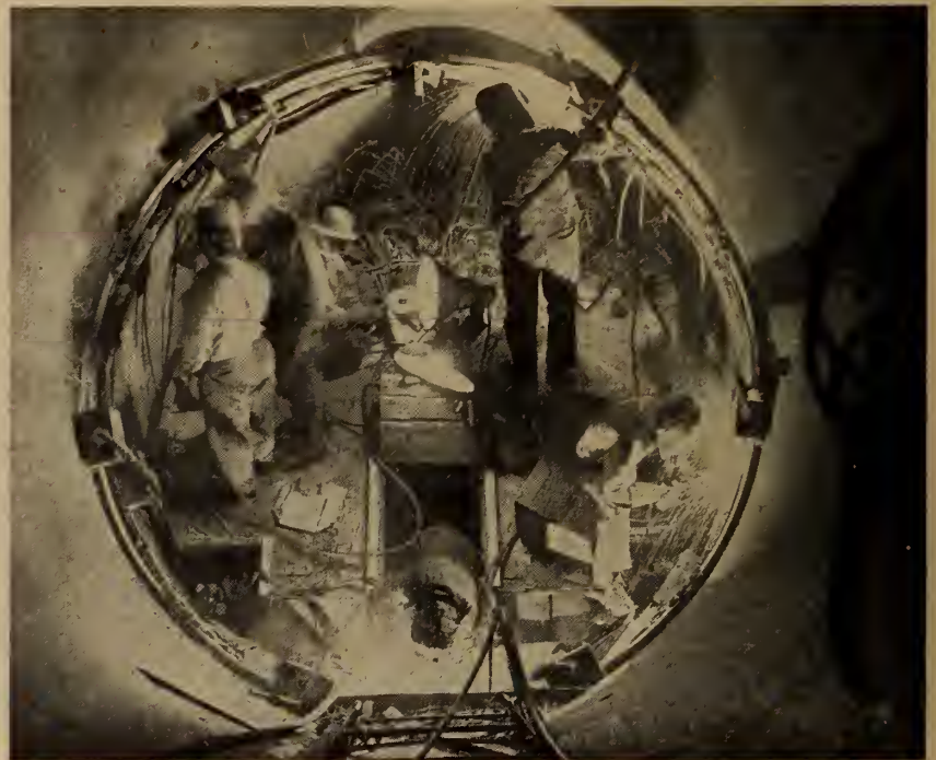
Fig. 44. Welding circumferential joint in liner plate.
