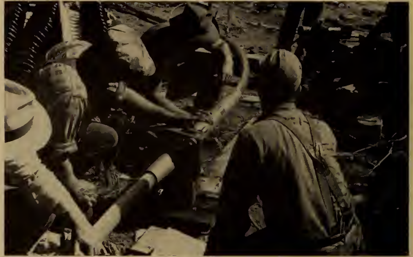
Fig. 57. Top: Compressing joint in "Emu" conductor.
