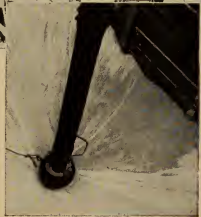
Sinker nozzle in operation at Kitimat.
