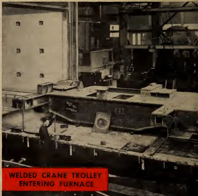
STRESS RELIEVING FURNACE
