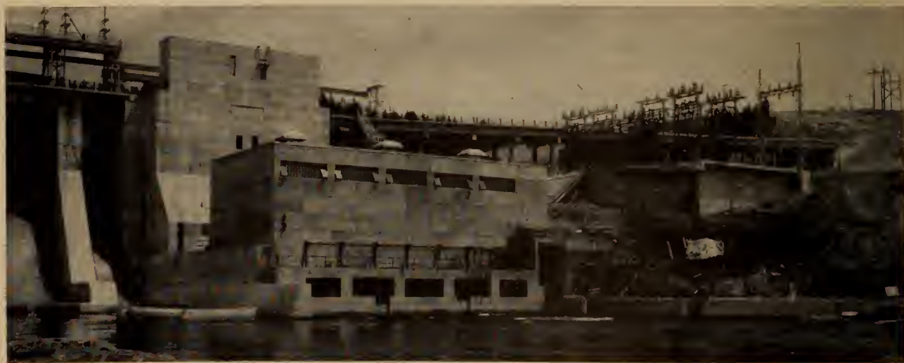
Fig. 3. Tobique Narrows powerhouse, showing four entrances to fishway from the tailrace.
