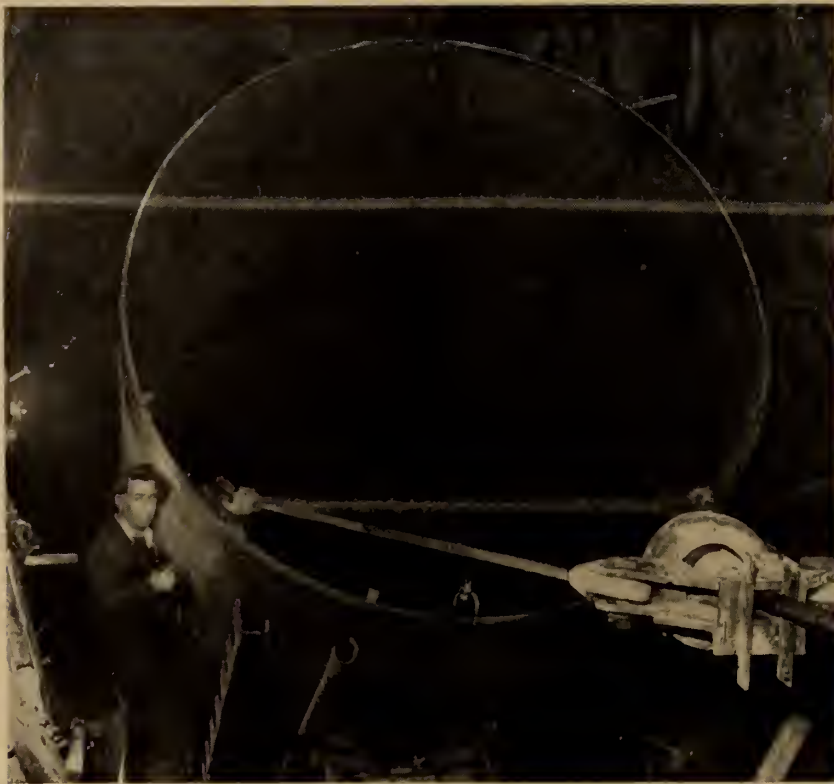
Fig. 43. Lowering liner section down penstock raise.
