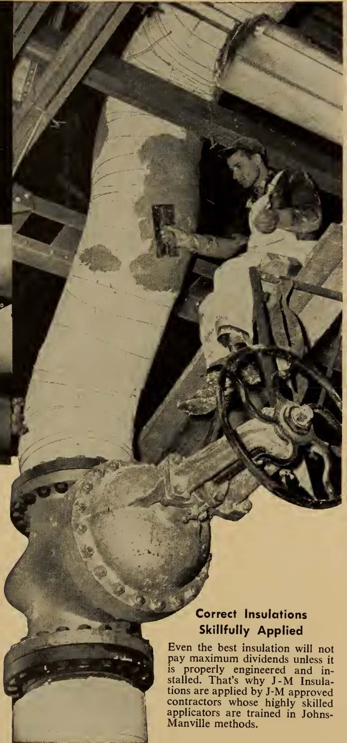
(Above) A partial view of the 1700 foot underground tunnel which houses mains carrying steam and water from power house to assembly plant.
