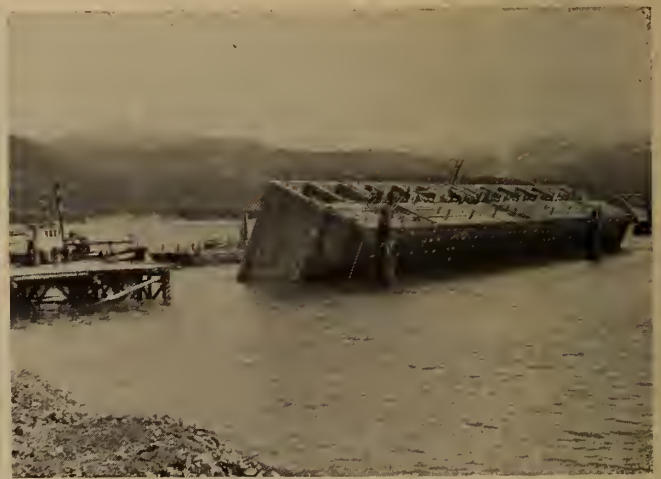
Fig. 83. The first caisson moored to its dolphins and partly careened.
