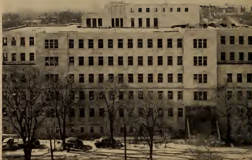
Fig. 3. The building nearing completion.
