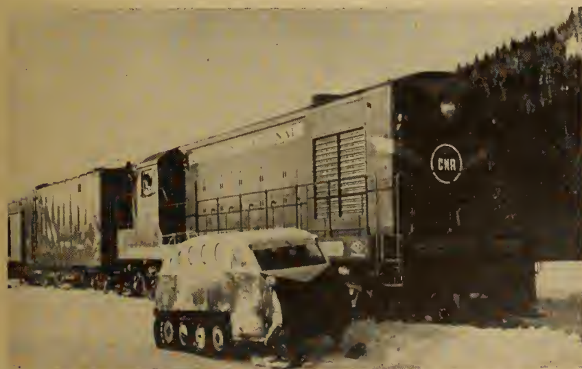
Fig. 3. Diesel road switcher, 1,200 hp.
