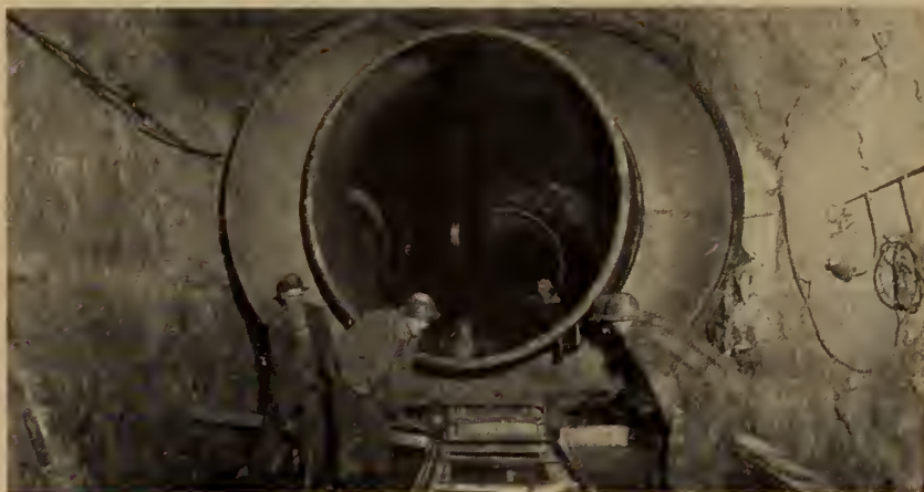
Fig. 49. Wye No. 2 looking downstream through 7 ft. 9 in. inlet.
