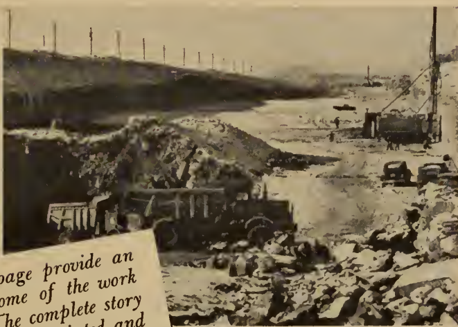
Huge Quarrymasters were used in drilling the 70 foot deep canal. This picture shows a drill at each side of the canal putting down line holes to obtain a solid vertical face.
