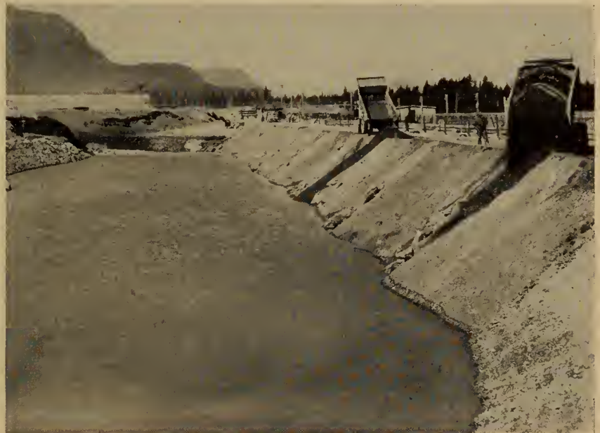
Fig. 86. Placing the sand filter blanket behind the caissons.
