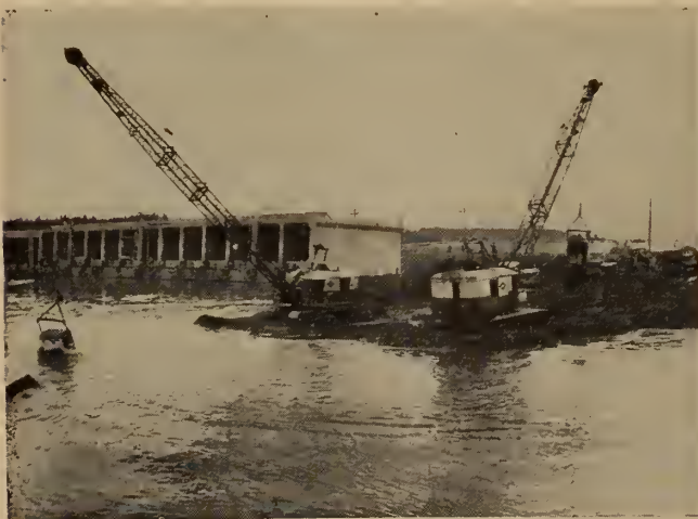
Fig. 82. The dikes breached and the caissons floating on their sides.
