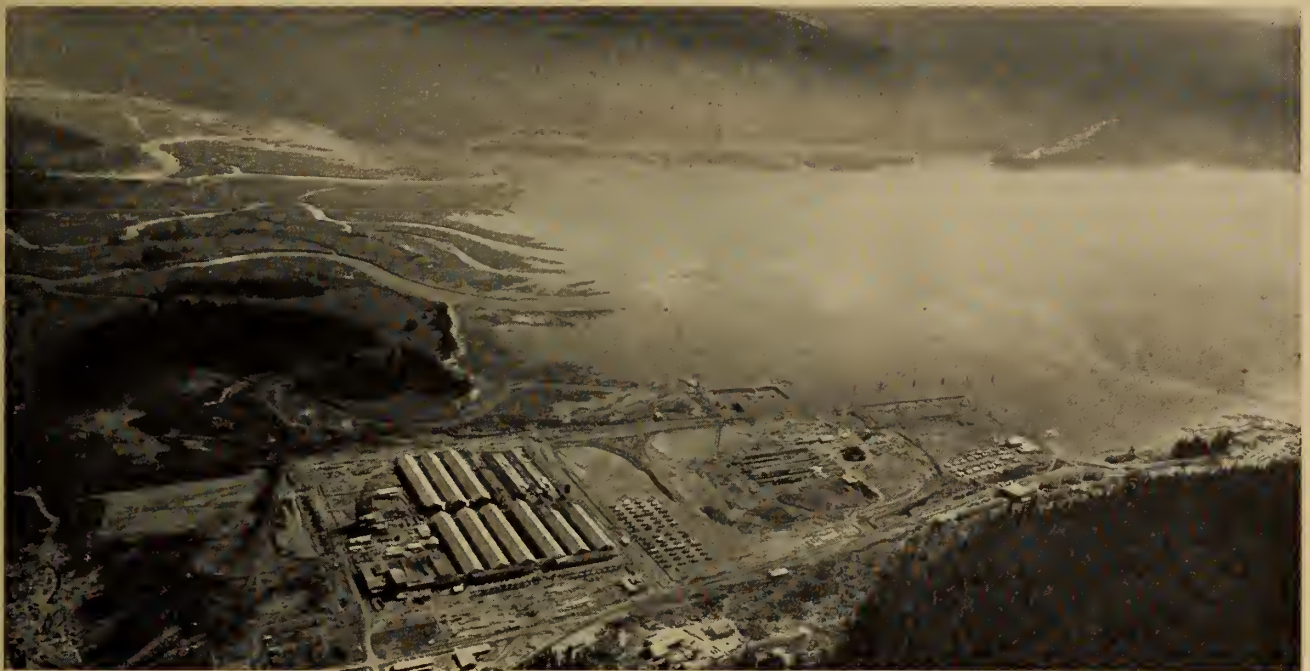
Fig. 88. Aerial view showing completed wharf at right center with line of dolphins beyond.
