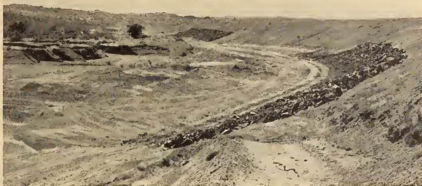
Fig. 6. Riprapping Dike No. 1.
