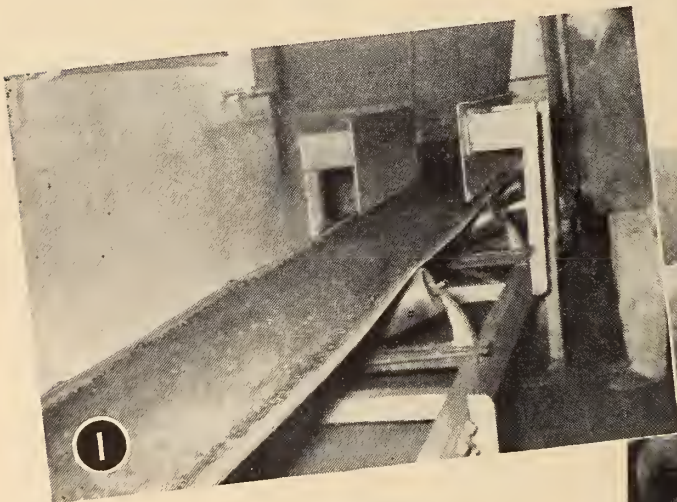
1. 24" Dominion "Giant", 312' long, is coal conveyor transfer belt carrying fuel to powerhouse.
