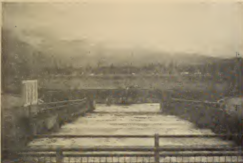
Fig. 2. One of the Bonneville Dam Fishways looking downstream.
