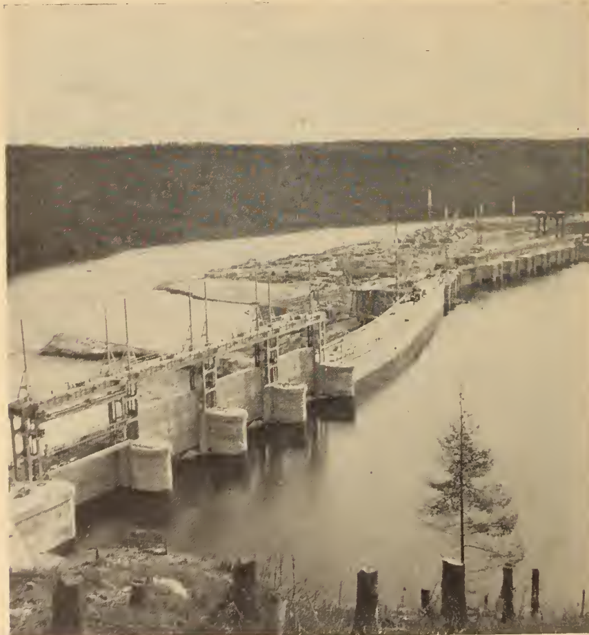
Fig. 5. View from the east bank showing, in the foreground, the sluice section, centre, the main dam and, background, the regulating gates and intake section. The length from shore to shore is 1,500 ft.
