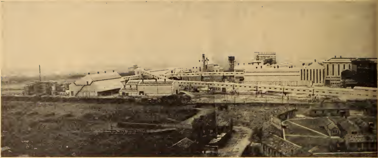
Fig. 1. On this and the facing page is a panoramic view of a fertilizer factory adjacent to Immingham Dock, Lincolnshire. Raw materials enter at the right via quayside grabbing cranes, reception hoppers and the conveyor in the lower elevated gallery. The finished product is exported to ship by conveyor in the upper elevated gallery.
