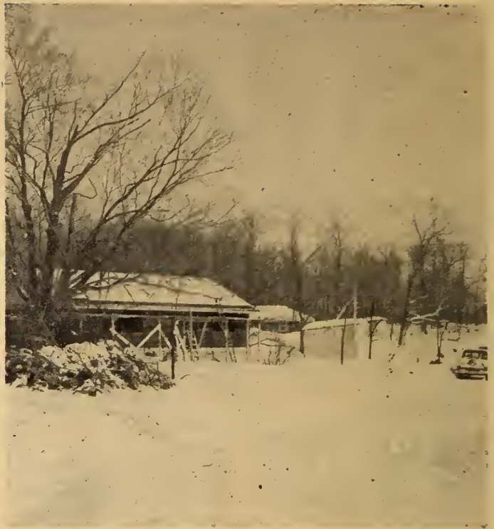
Photos above and below are views of the Fairhaven project.
