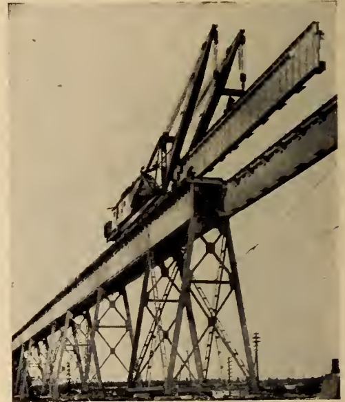
Port Arthur ore dock approach
