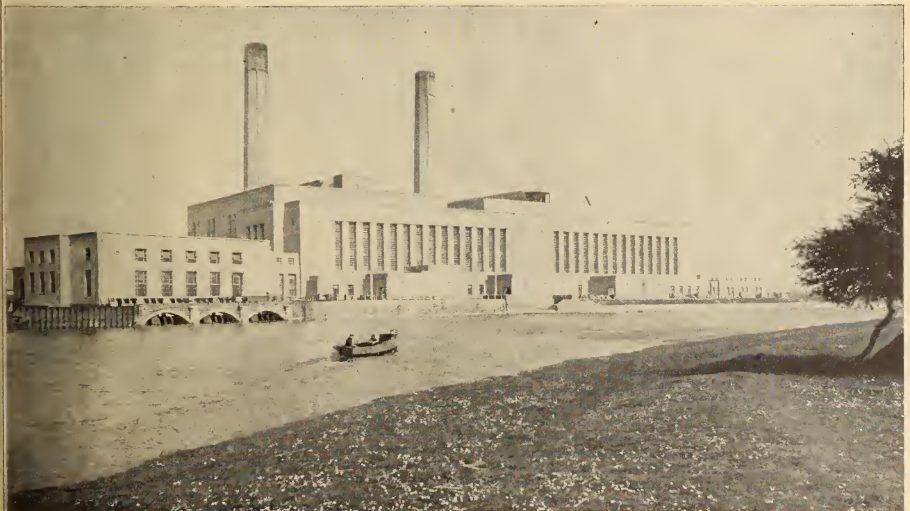
Fig. 2. Staythorpe Generating Station. Exterior view from across the river.
