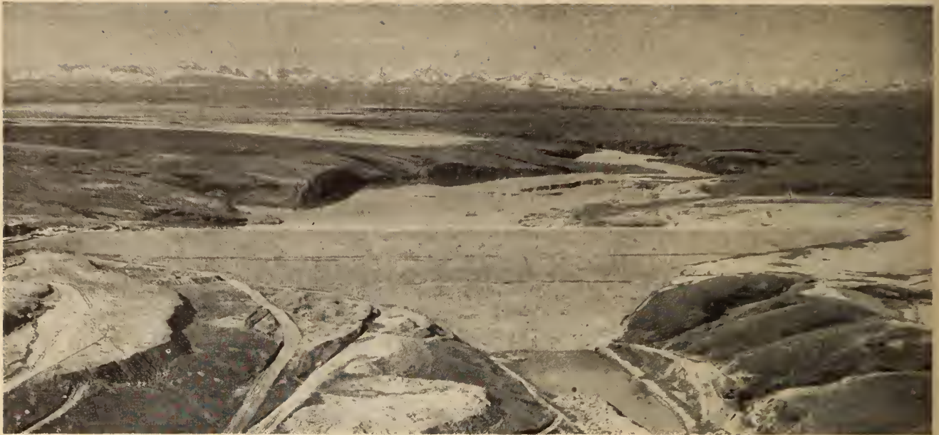
Fig. 1. Aerial photo of St. Mary Dam, looking west. Reservoir and mountains in background.
