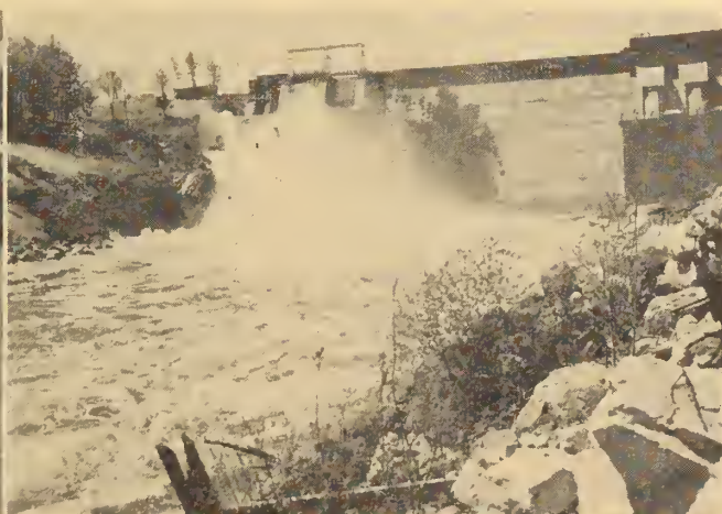
Fig. 11. View showing energy dissipation with 16,000 cubic feet per second discharge from right gate.
