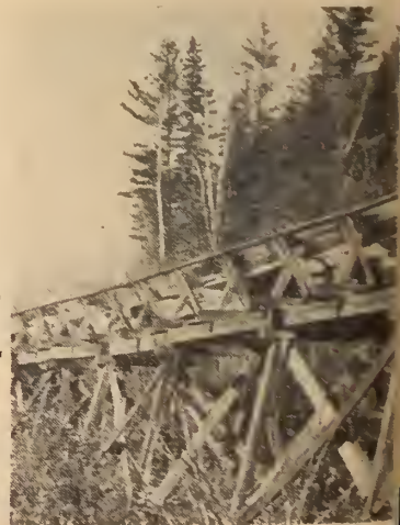
FLUME.—Saguenay district. 14-year-old Osmose-treated section required no maintenance. Untreated section replaced after 8 years.
