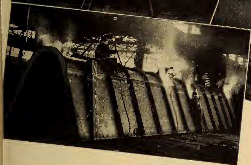
Log Chute for Hydro Power Dam at Des Joachims 1000 ft. long (50 ft. sections) 240 tons
