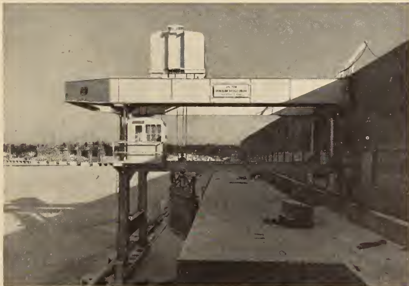
The photograph shows a 25-ton electric gantry crane on the headworks of the Des Joachims development of The Hydro-Electric Power Commission of Ontario. It is used for handling trash racks, emergency stop logs and head gates, and incorporates an auxiliary high-speed hoist for lifting the trash rack cleaners.
