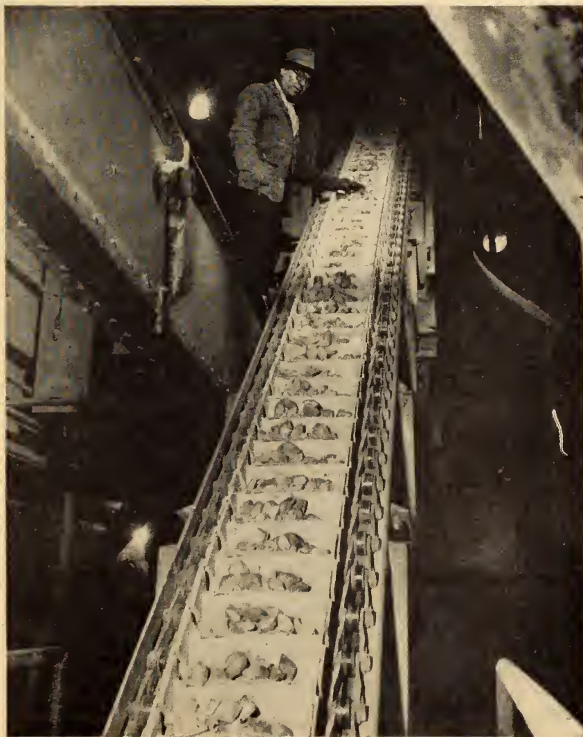
Fig. 2. Moist lime hydrate briquettes being conveyed to dryer.
