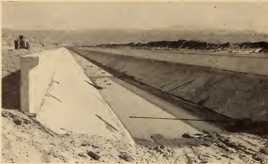
Fig 2 (above). Wasteway No. 1 Outlet.
