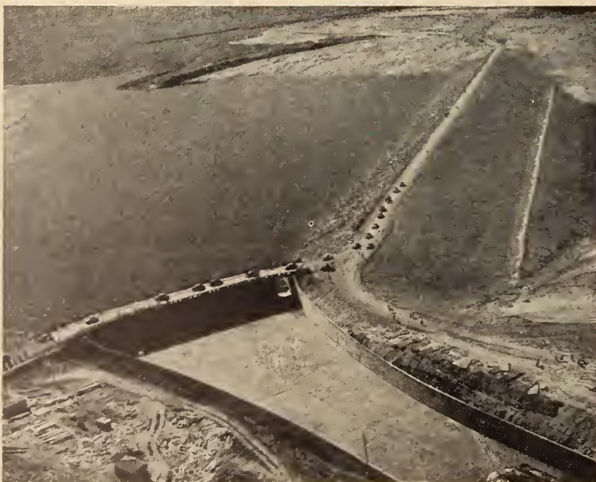
Fig. 3. St. Mary Dam and spillway.
