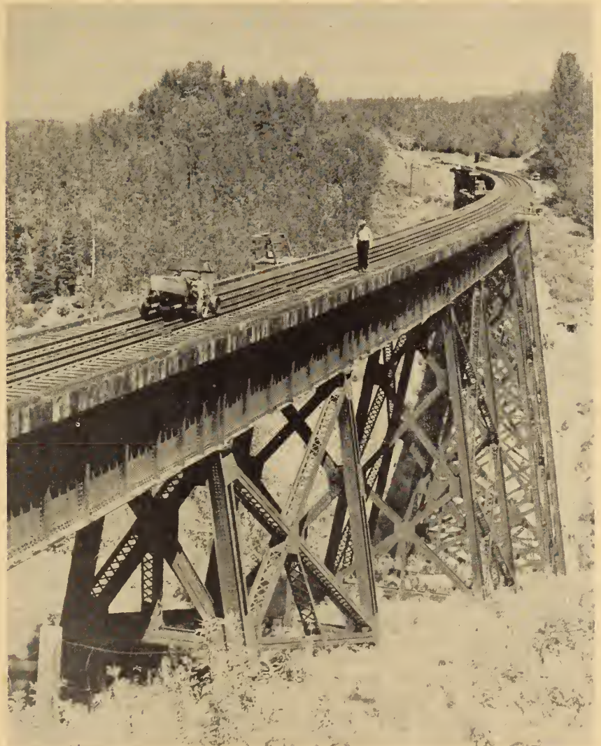
Fig. 4. Railway trestle on the Prince Rupert line near Smithers, B.C.
