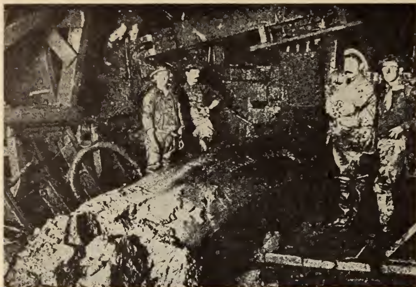
Fig. 11. Tunnel driven in river silt. Silt flowing through bottom door.
