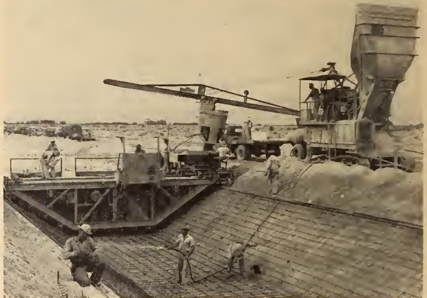
Fig. 3 (below). Concreting Wasteway No. 1 Channel.
