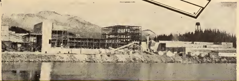
EARLY CONSTRUCTION VIEW.
