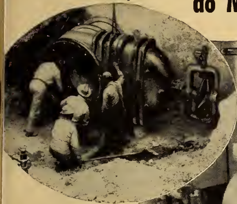
(Above) New Supply Line from reservoir of large city, showing installation of Crane 48-inch Gate Valves, bevel gear operated.
