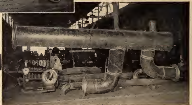
8" assembly including 76½XR gate valve with ¾" by-pass.
