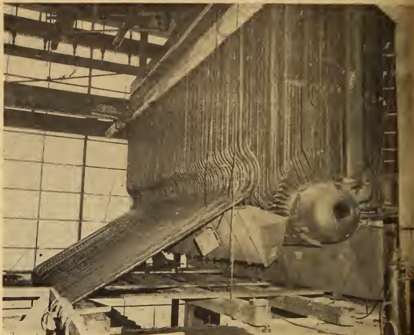
Fig. 7. Steam generator tubing at the J. Clark Keith Generating Station, Windsor.
