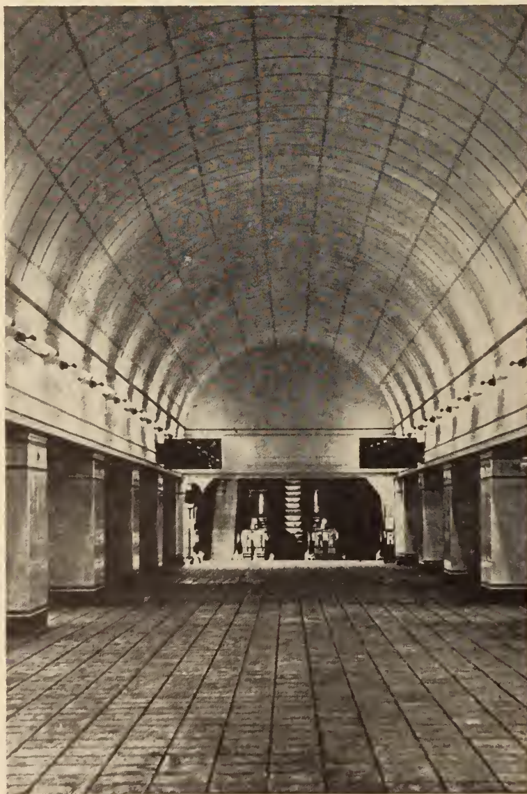
Fig. 17. London underground railway. Gants Hill Station.
