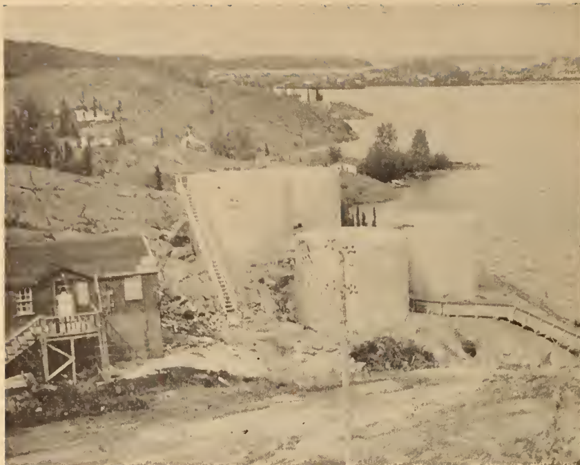
Fig. 4. Fuel oil tanks at the intake pump house.
