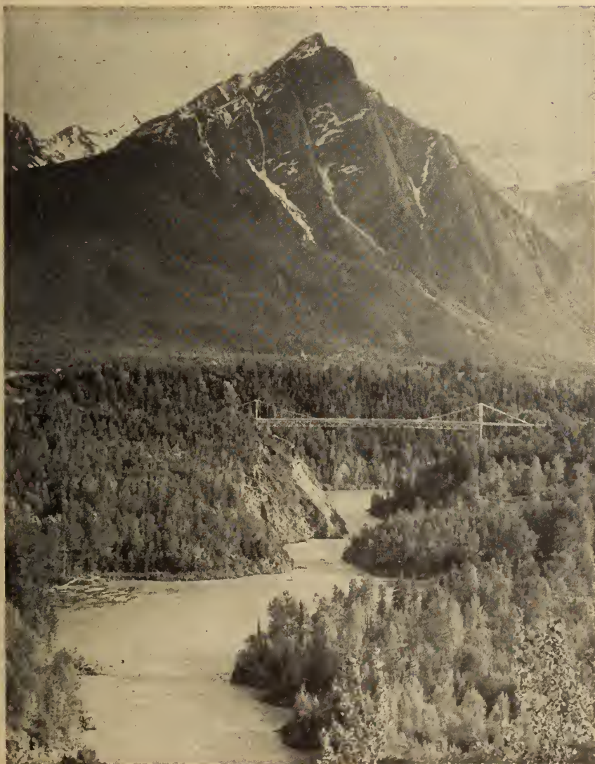
Fig. 2. Prince Rupert Communications. Highway bridge over Bulkley at Hazelton.
