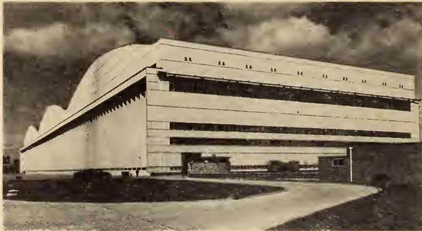
Fig. 1. View of the Brabazon hangar from the south-east.
