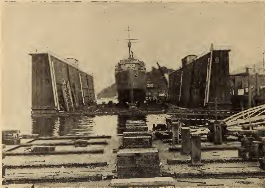
Fig. 5. Newly constructed naval vessel in Prince Rupert drydock during the Second World War.
