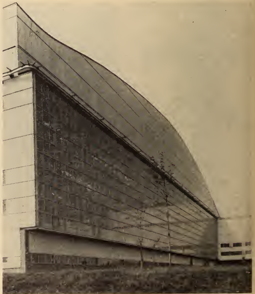
Fig. 2. The all-glass rear wall of one of the hangar bays. Total glass area of rear walls is some 50,000 sq. ft.
