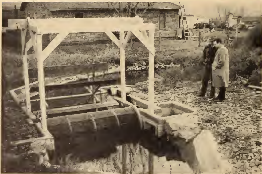
Fig. 4 (top). Hell's Gate Fishways under construction, Fraser River, B.C.
