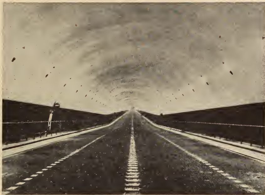
Fig. 6. View of completed vehicular tunnel 44 ft. 6 in. internal diameter.
