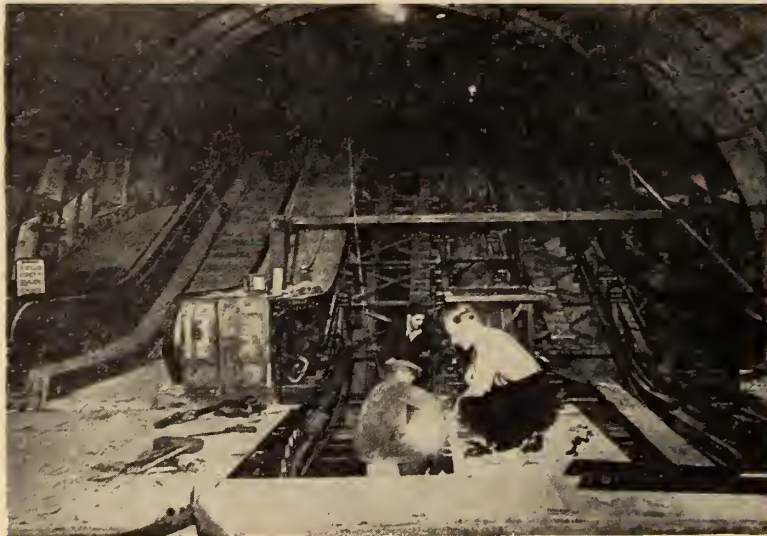
Fig. 14. London underground railway escalator tunnel showing escalator in course of construction.
