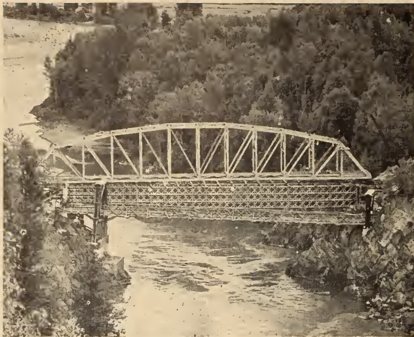
Fig. 6. The completed structure, with the Bailey still in position, and with the original highway bridge in the foreground.
