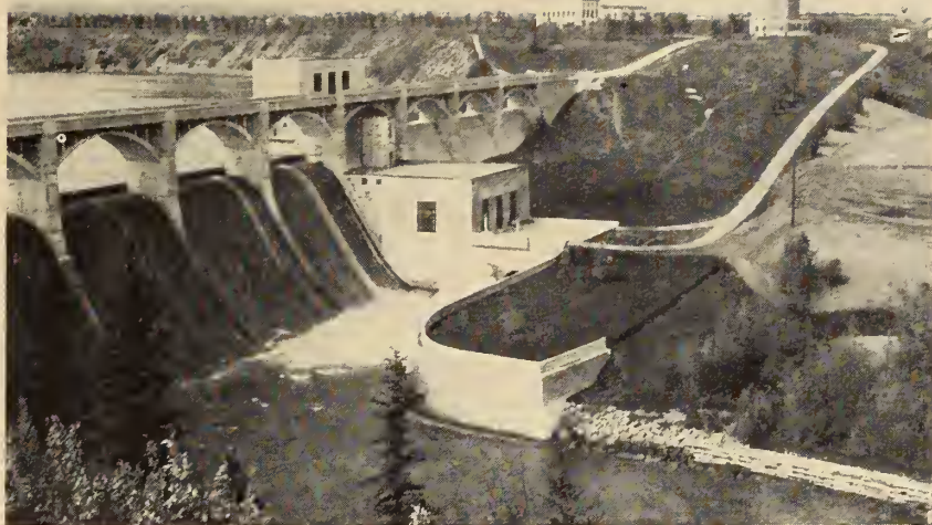
Fig. 2. Glenmore dam, Calgary, Alta.
