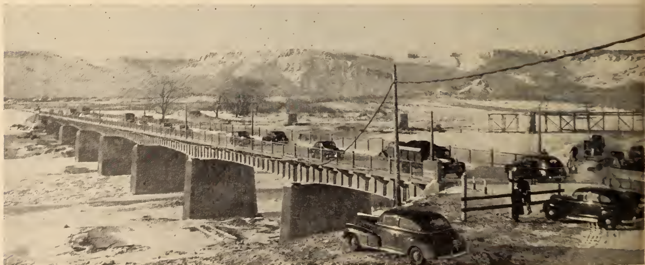
Fig. 1. New bridge at Lethbridge, Alta.
