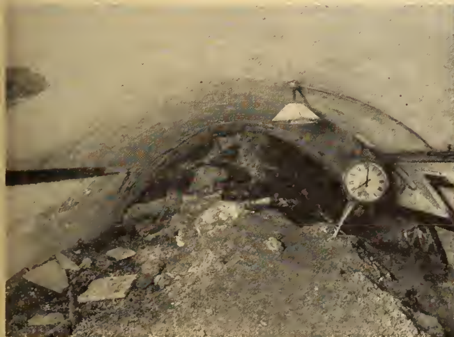
Figs. 3 and 4. (Left). Debris in Balham tube station under bomb crater. (Right). Repairs to brickwork of Euston Square — Kings Cross tunnel after bomb damage.
