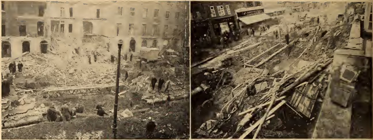
Figs. 1 and 2. Bomb damage at Cliveden Place (left) and South Harrow (right) in London. Note damaged sewers, water and gas mains, and electric utility lines.
