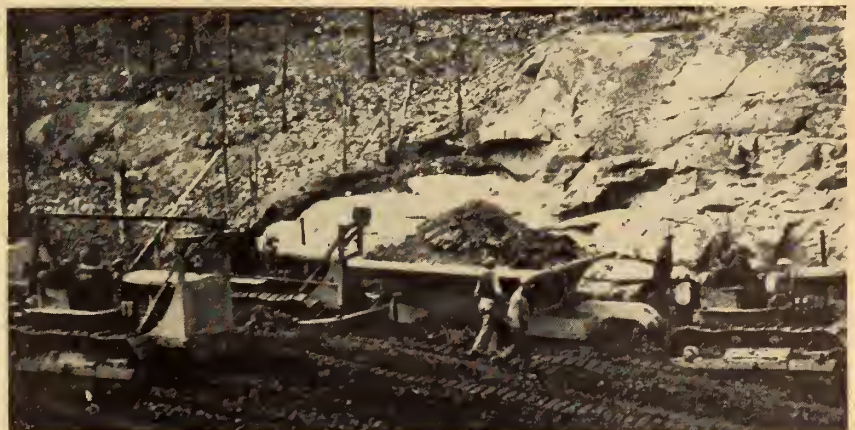
Fig. 4. Placing rolled fill in north channel.
