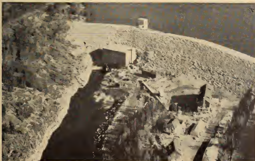
Fig. 8. General view of completed project.
