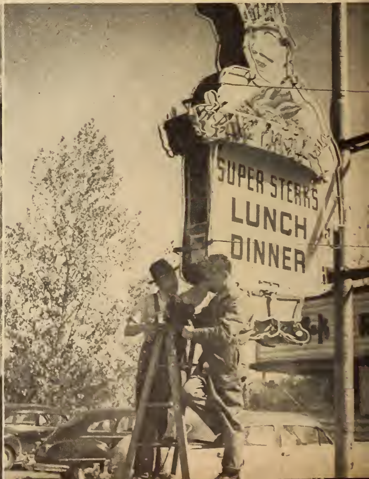
Fig. 8. Transformers on Neon signs are among the many types of frequency-sensitive equipment that must be converted for 60-cycle operation.
