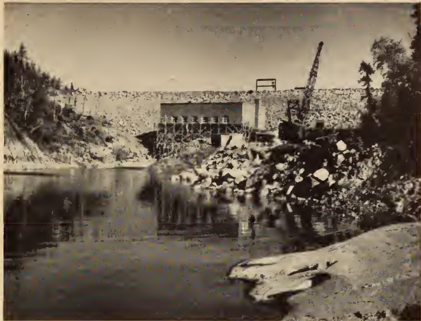
Fig. 7. General view from tailrace showing completed dam and power house.
