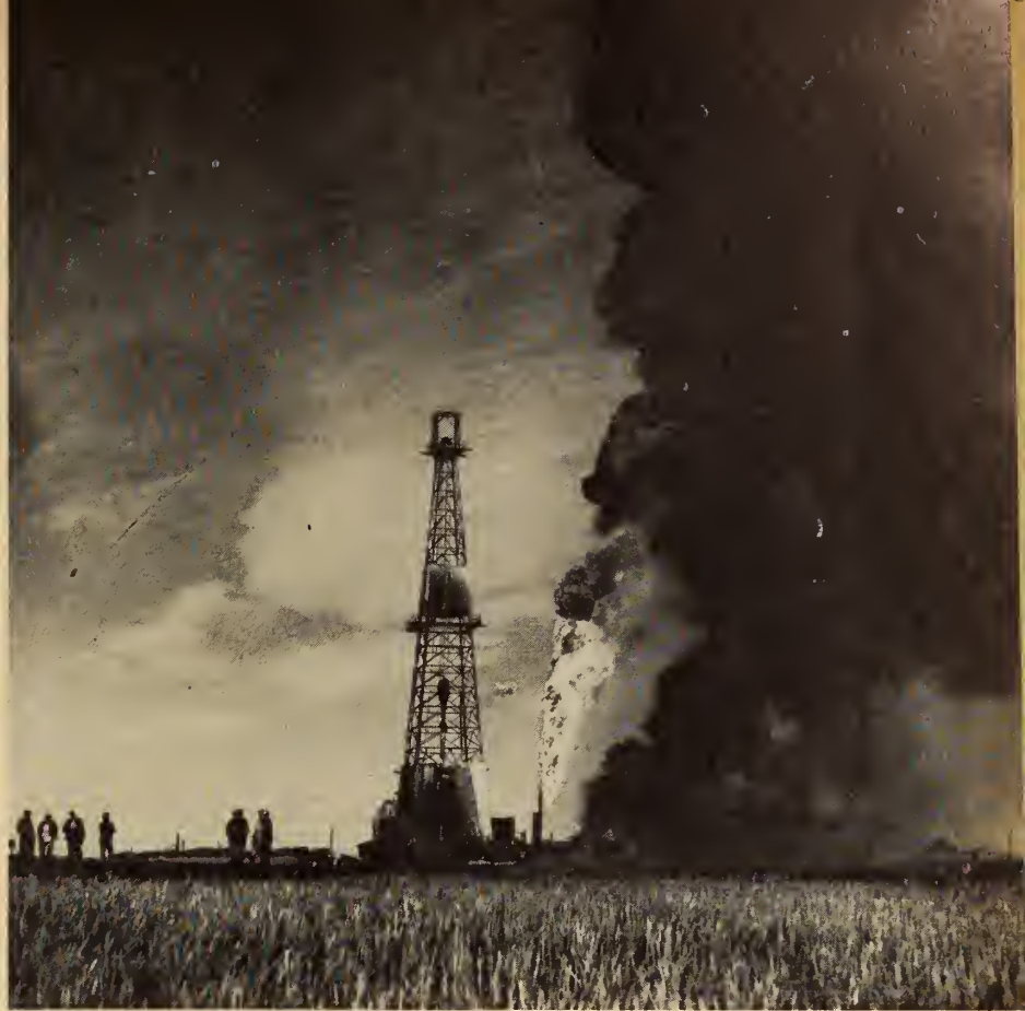
Fig. 3. Great columns of smoke and flame roar out of the flare pit at Imperial Schoepp No. 1 during the brief time it took to clear the hole of mud following its kick-in to production.
