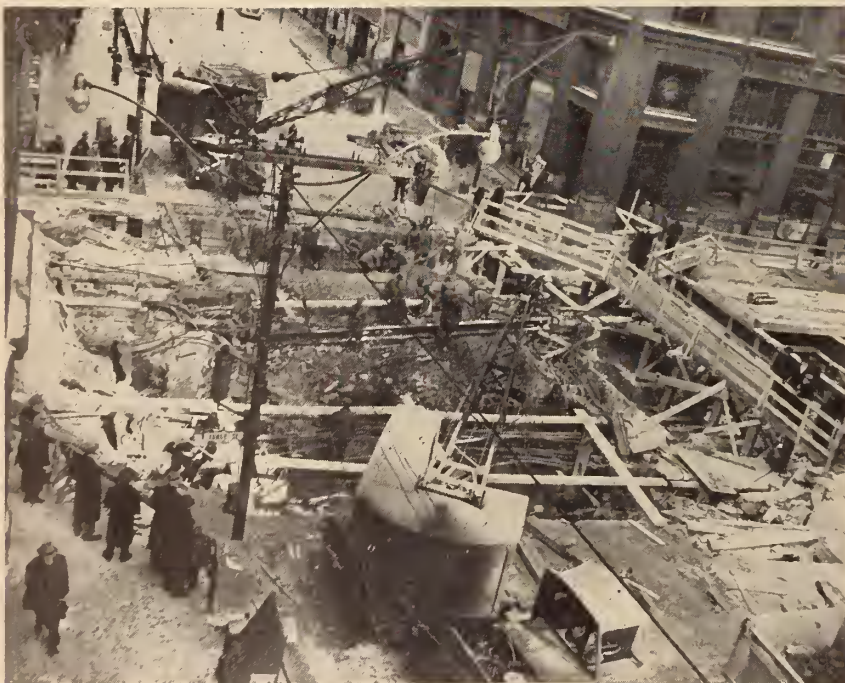
Fig. 1. Top lift excavation intersection King and Yonge Streets showing exposed utilities.
