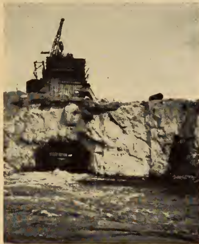
Fig. 3. Downstream end of tunnels, at future site of power house.
