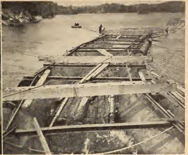
Fig. 3. View of flume from downstream end.
