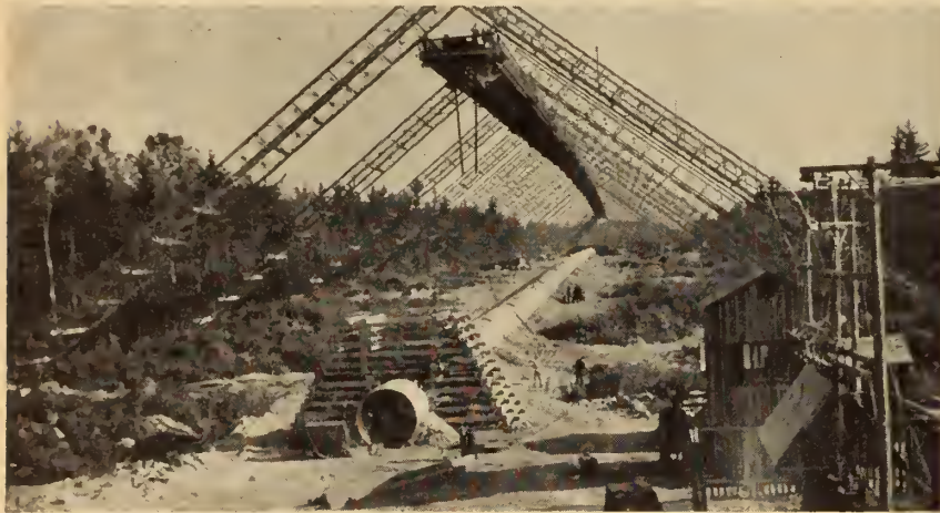
Fig. 7. Above: Bailey bridge application for concrete aggregate conveyor supports.
