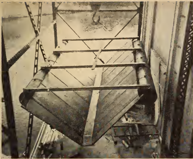
Fig. 2. Assembled 33-ft. flume section ready for launching.
