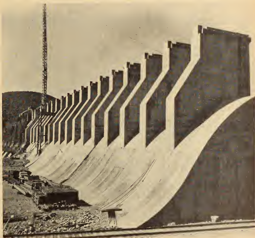
Fig. 12. La Cave Development — Close-up of rollway section topped with 16-foot stoplog sluices.
