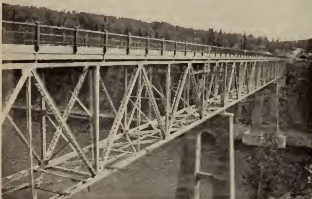
Fig. 1. View of completed bridge looking south, showing trusses, deck and railings.
