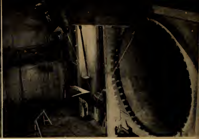
Fig. 3. The Hermann Göring wind tunnel (A.3) at L.F.A., showing nozzle and wing model in place.
