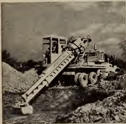
(Left, top) — Residential and industrial foundations are excavated with sheer, vertical sides and floored to perfect grade, eliminating the expense of extra hand operations.
