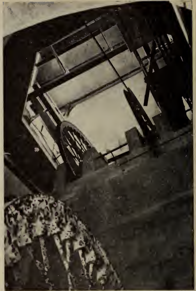
Fig. 7. Interior of headframe.
