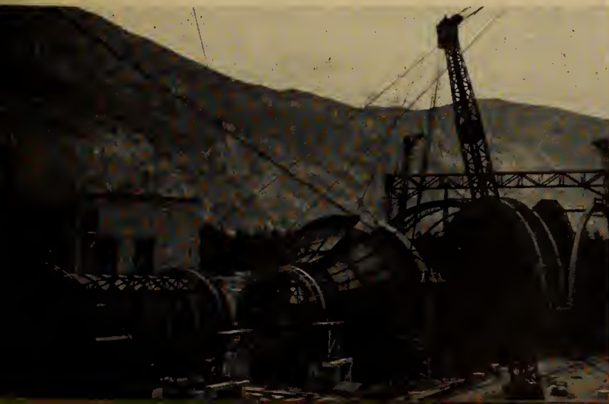
Fig. 14. (below) 100,000 hp wind tunnel of the L.F.M., in the Ötztal Alps, with direct water power drive.
