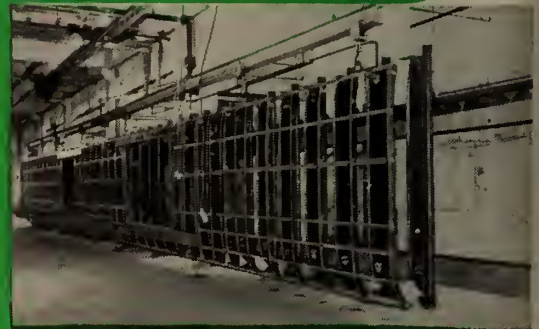
Side frame assembly after straightening, prior to final side assembly.
