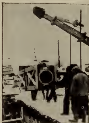
Assembly of pipe and coupling being removed from the line for laboratory tests.
