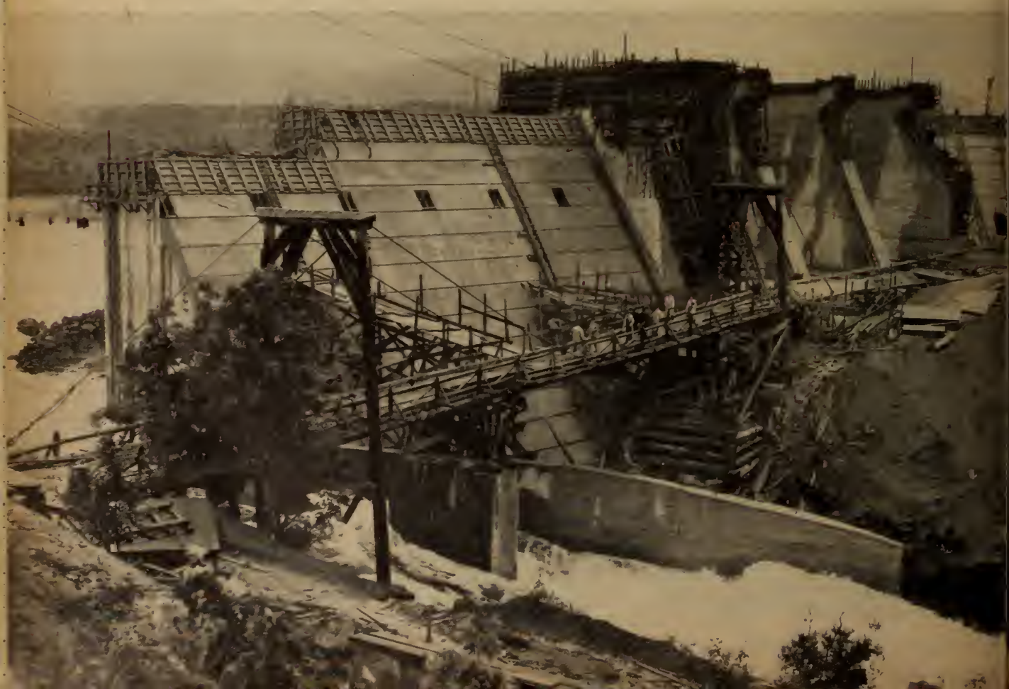
View of main dam. Irene Pool in background. Old B.C. Forest Service Bridge in foreground.
