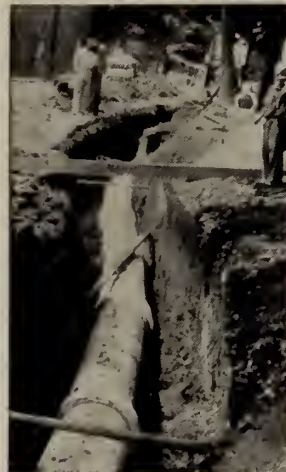
DEFLECTIONS up to 5° of each joint are possible with the Simplex Coupling. This permits laying the pipe around curves or obstructions as shown by the installation above.
