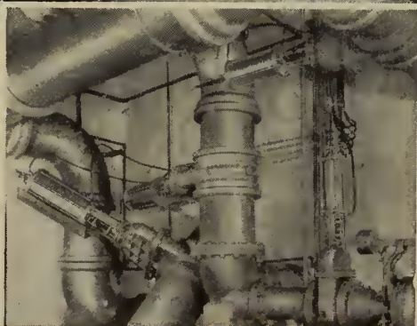
8" CRANE No. 465½ Iron body cylinder-operated gate valve.
