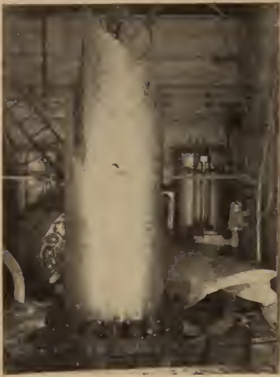
Fig. 3. Photograph of fractured portion of the column.
