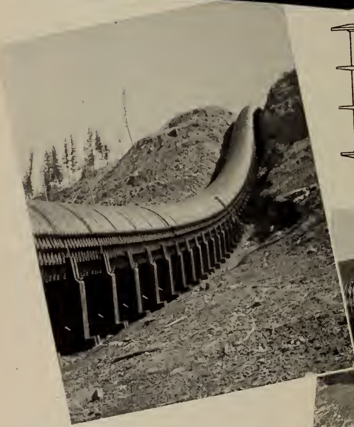
Two views of the ten-foot Creasoted Continuous Wood Stave Pipe, installed for the Calgary Power Company Limited at Banff, Alberta. Pacific Metal Butt Joints (Patented) were used for connecting stave-ends.
