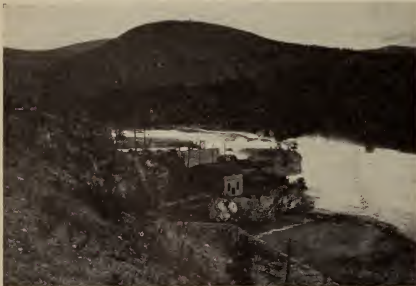
Fig. 5. The original No. 1 Plant, the first hydro-electric plant on the Kootenay River, was built by the West Kootenay Power and Light Company in 1897-98 and was designed to develop 4,000 hp. In the background is Lower Bonnington Falls. This plant was replaced in 1925 with a new plant of 60,000 hp. capacity.
