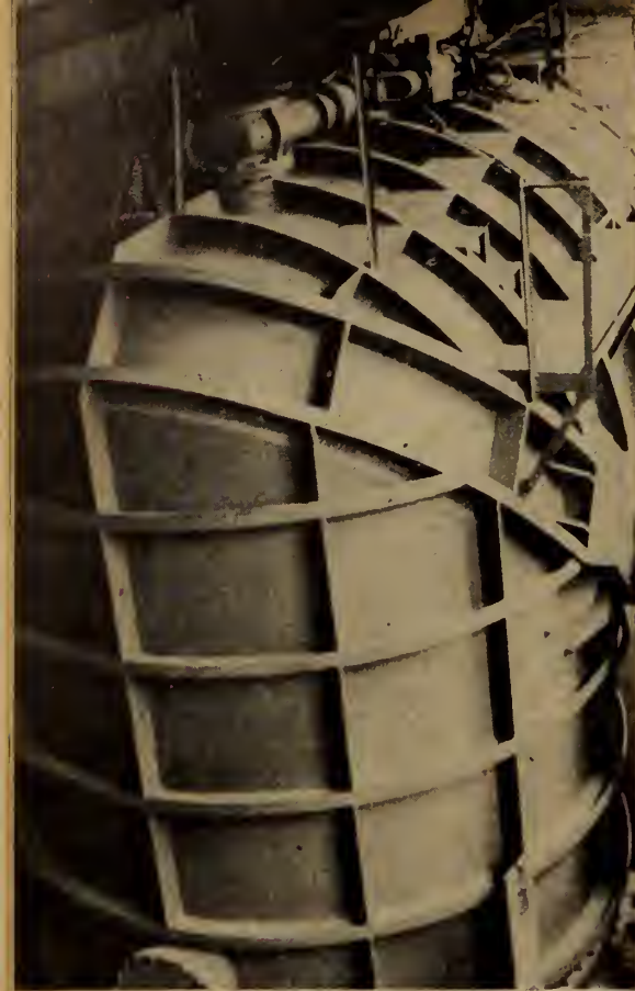
Fig. 9 (left) Construction detail of supersonic wind tunnel A.9b at L.F.A.
