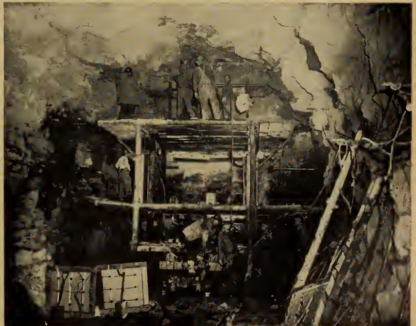
Fig. 6. Drilling jumbo, diversion tunnel, St. Mary Dam.
