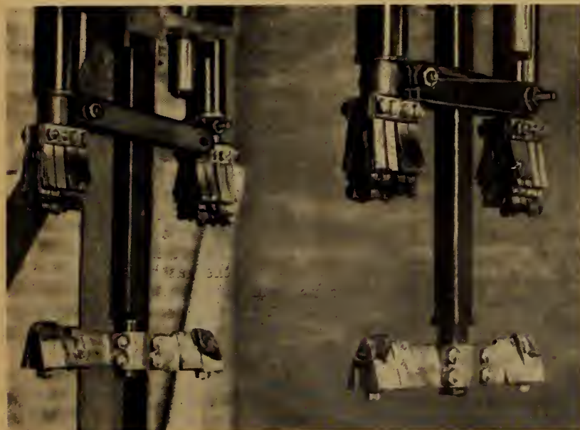
Fig. 8. High power testing demonstrates the necessity of adequate bracing.
