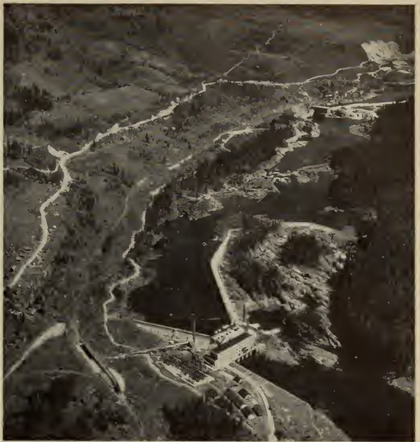
Fig. 6. Aerial view of No. 3 Plant of the West Kootenay Power and Light Company, showing in the background the new No. 1 Plant. Note the rugged mountainous country through which the Kootenay River flows on its way from the Kootenay Lake to the Columbia River.
