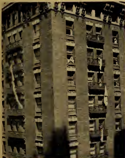
(above) Hotel fire.
