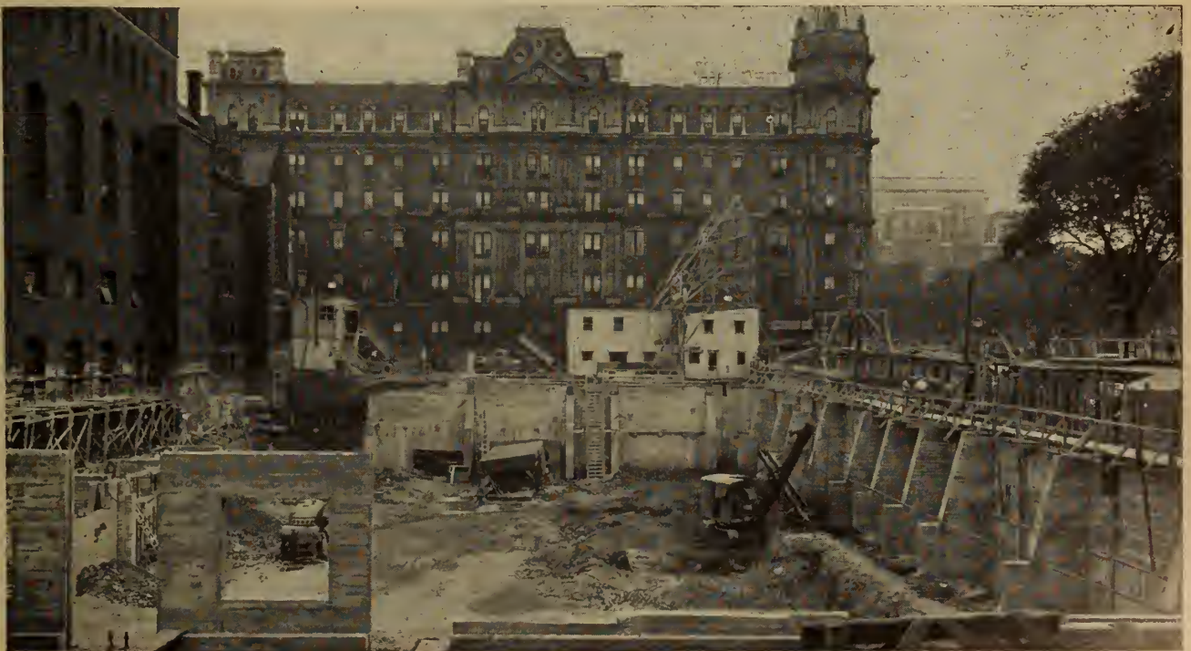
Retaining wall and buttresses. August 2, 1946.
