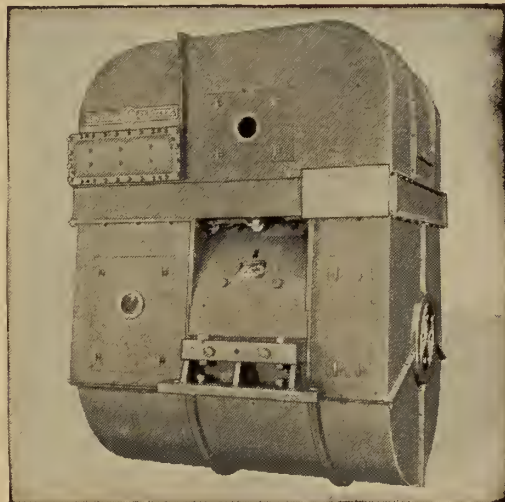
One of the eight G-E main generator sets each of which is rated 1050 kw—325 volt and is driven by a 12 cylinder diesel engine.
