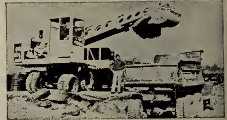
(Left, top) — Residential and industrial foundations are excavated with sheer, vertical sides and floored to perfect grade, eliminating the expense of extra hand operations.
