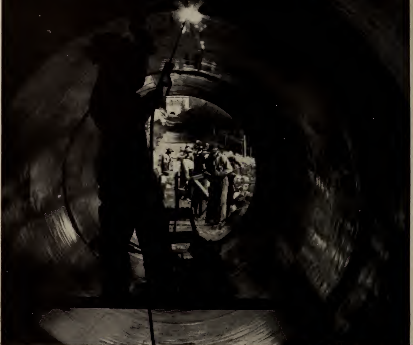
7½ foot diameter intake pipe, Seymour Falls to Vancouver
