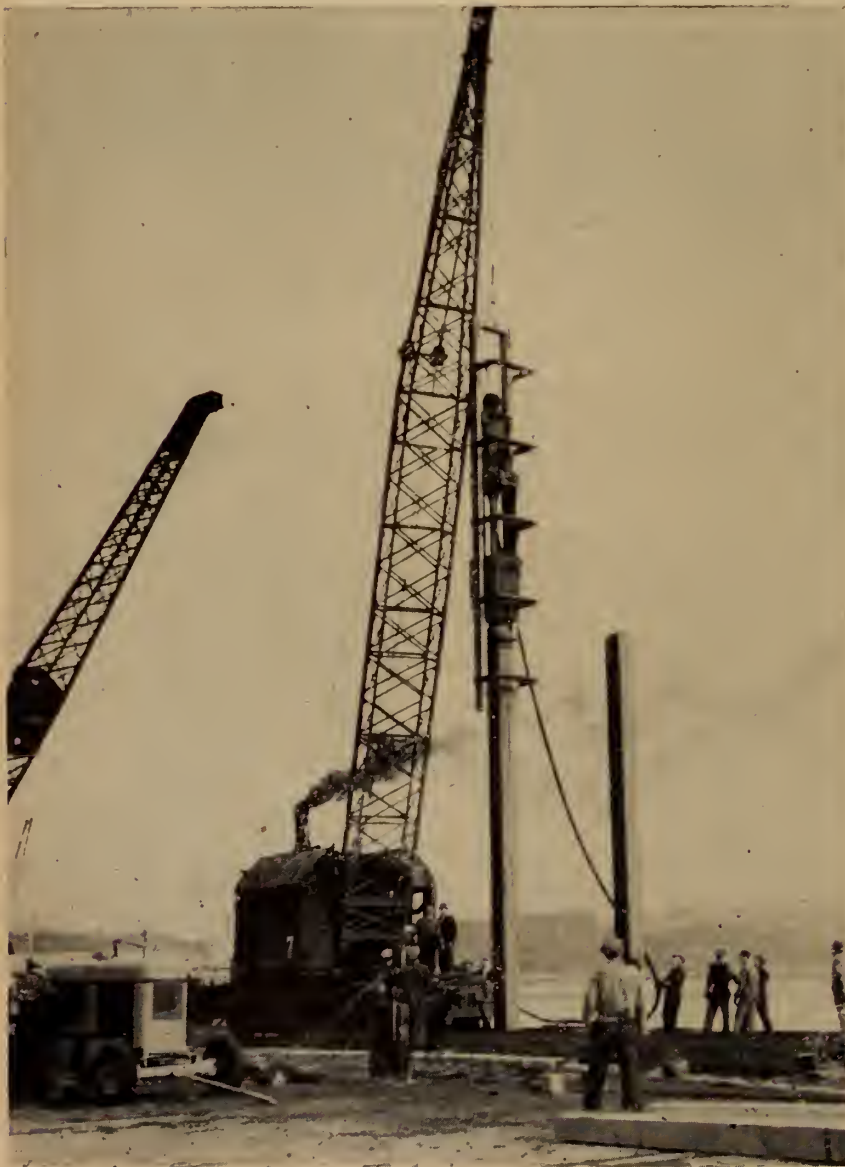
Fig. 1—View during driving of test piles, showing driving equipment, etc.
