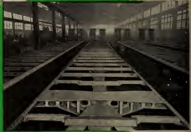
Underframe of all-welded steel car in position prior to assembly of side sheet assemblies.
