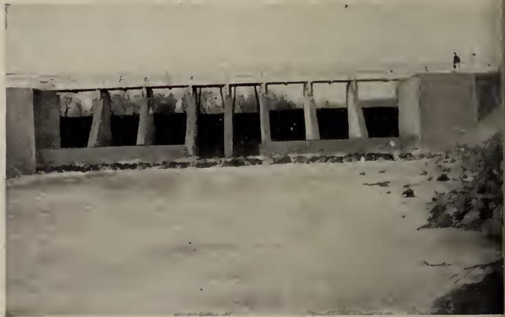
Looking upstream at Craven Dam on Qu'Appelle River, Saskatchewan. Bird Construction Company, Contractor. P.F.R.A.
