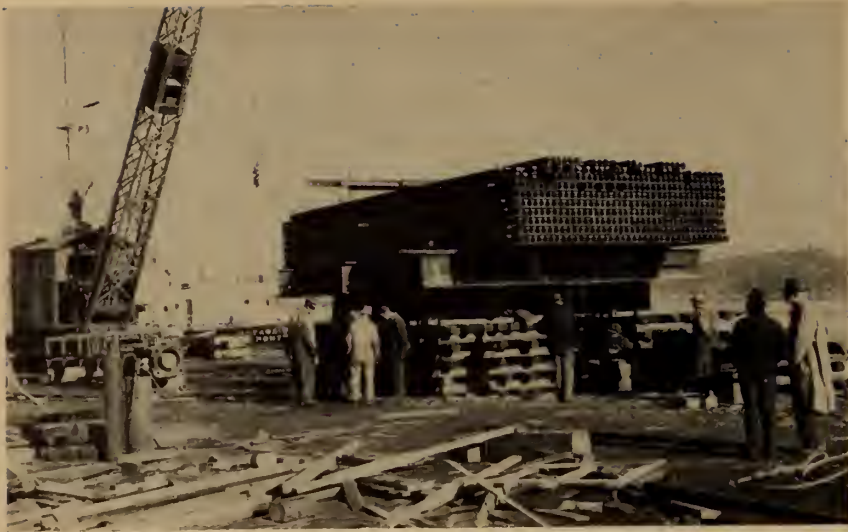
Fig. 5—View of static test load and supporting grillage.
