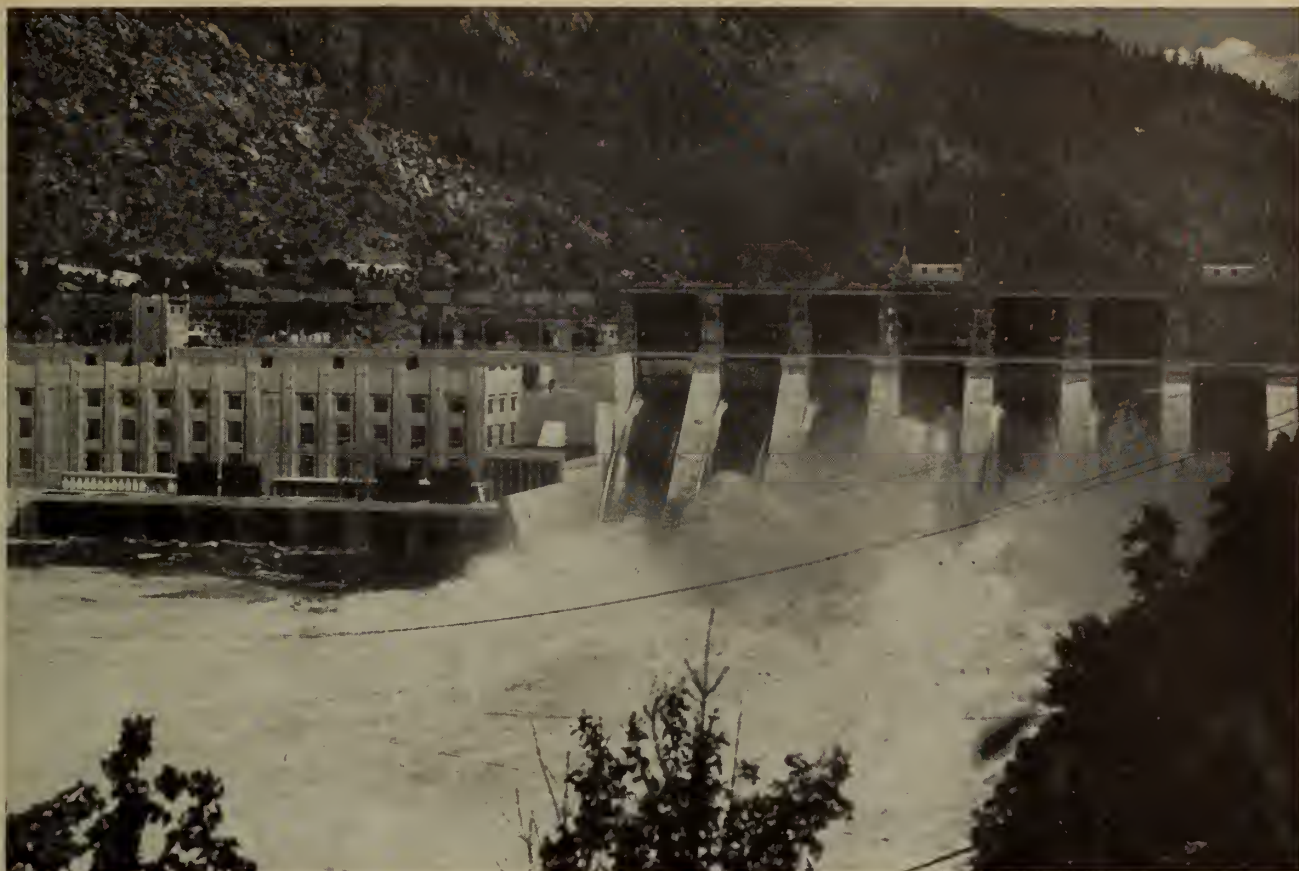
Fig. 8. No. 5 Plant, the most recently completed hydro-electric plant on the Kootenay River, is at Brilliant, B.C. Its ultimate capacity will be 148,000 hp. Cominco photo.
