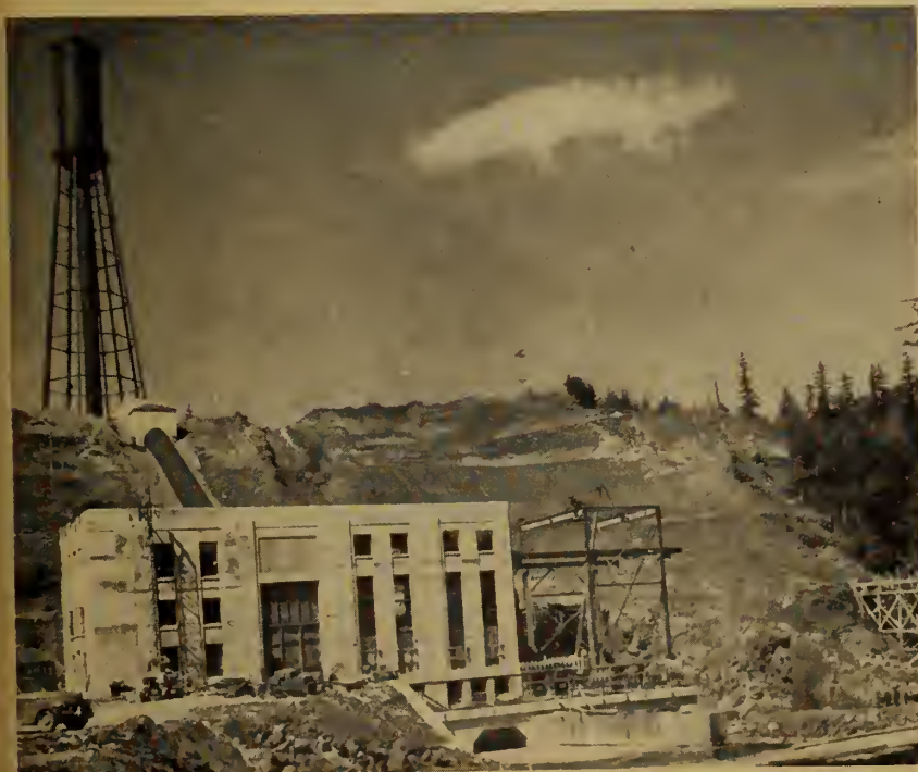
Powerhouse, penstock and surge tank.
