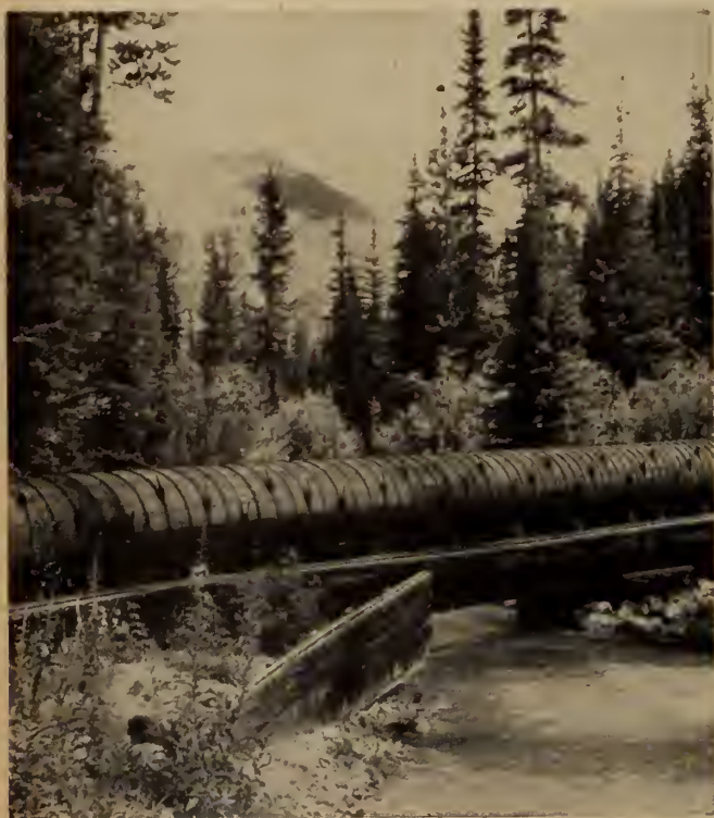
Three foot diameter wood pipe used for Hydro Electric Development, installed by us in Selkirk Range.
