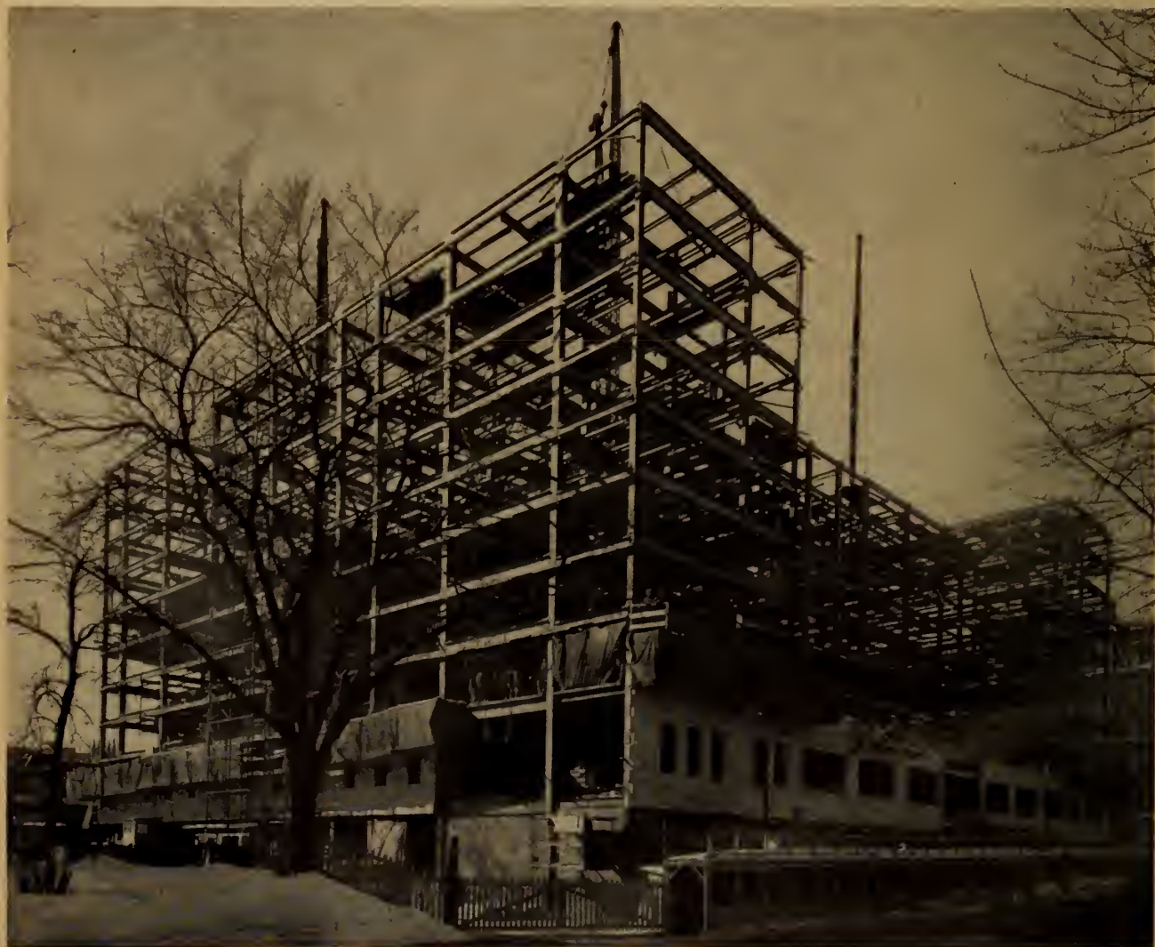
Below —Progress of structural steel at February 18, 1947.
