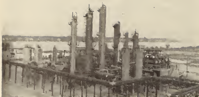
Fig. 3—Light ends fractionating unit.
