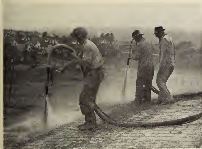
Fig. 4—Shooting gunite on dome roof.
