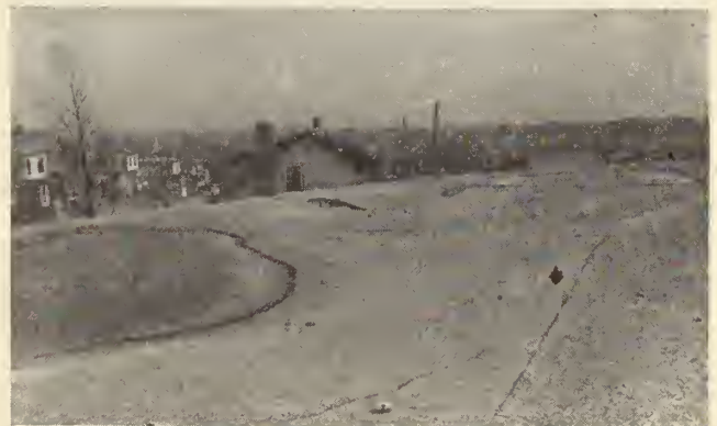
Fig. 1—Old roof showing failures in slab.
