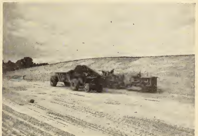
Fig. 1—Grading a deep cut with elevating grader on new Toronto-Barrie highway.
