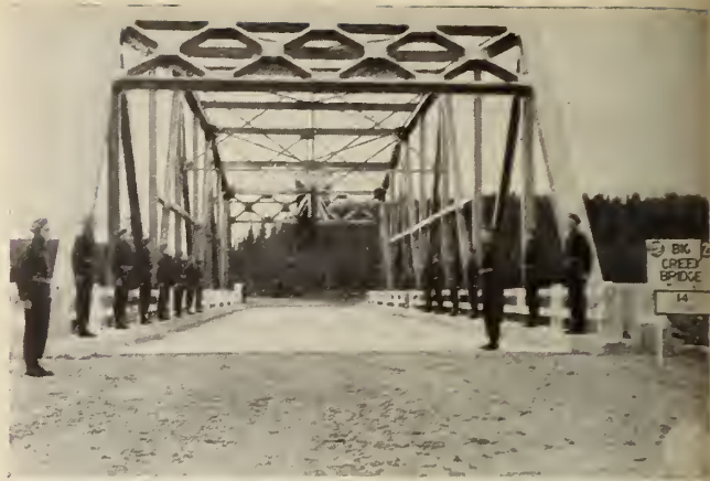
The guard of honor from No. 1 Road Maintenance Coy., R.C.E., at the opening of the Big Creek Bridge.
