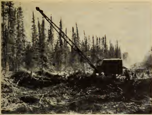
Fig. 4—Grubbing with a dragline on the new Red Lake highway, summer 1946.
