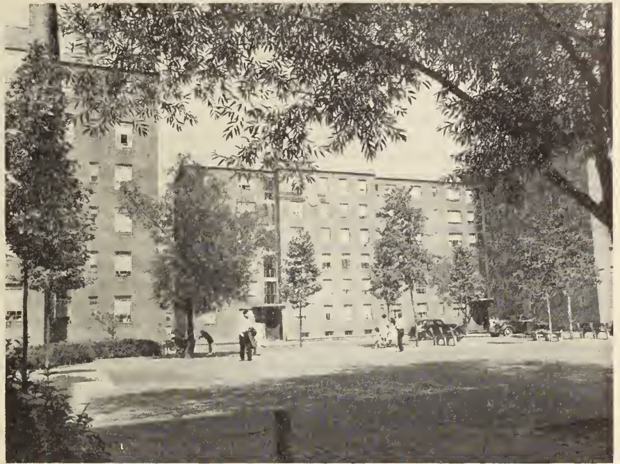
East River Houses. Notice the open parapets in place of solid masonry. This project showed a record low construction cost of $2,980 per apartment, for modern fireproof construction with all conveniences. Eighty per cent of the site is open space.
