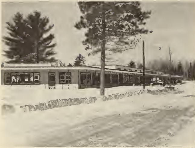
Fig. 7—Shopping centre at Deep River Village.
