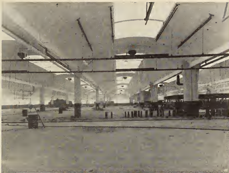
Fig. 5—Interior view of the Engineering Shops Building at Wright Field, Ohio.
