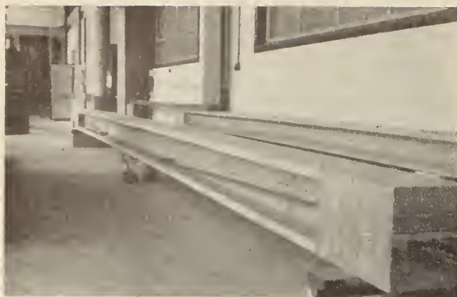
Fig. 5—Prestressed concrete beam cast in the University of Ghent laboratory.
