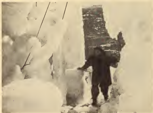
Fig. 5—Ice accumulation can make a \frac{1}{8} in. dia. cable grow to 6 in.
