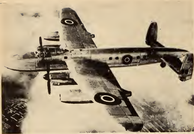
Fig. 12. Flight testing of jet engines—an Avro Lancasterian flying on two Nene engines in the outboard positions. (The inboard Rolls Royce Merlins are stopped and their propellers feathered.)
