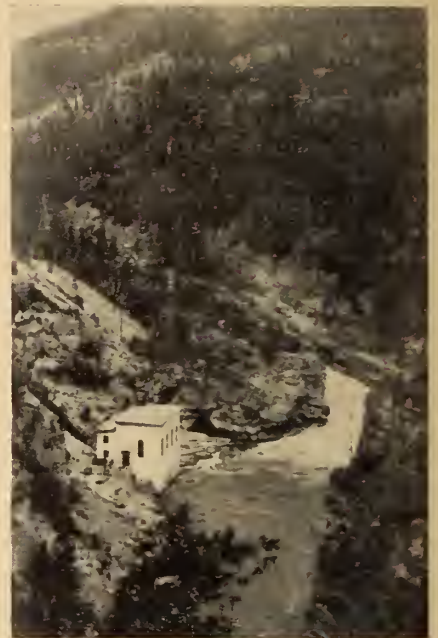
Above: Elk River, showing the Elko power plant of the East Kootenay Power Company.
