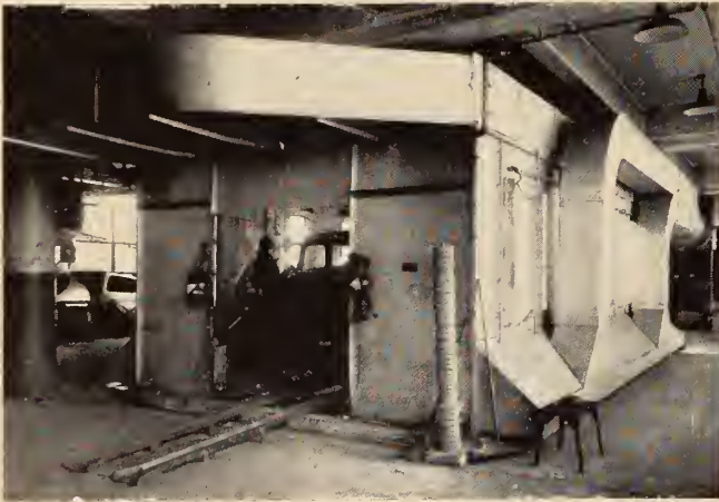
Fig. 7. Supply-exhaust booth for grinding on automobile body solder. Note worker with air-supply hood. See items D-1 and F-2 in classification, page 592. Courtesy R. C. Mahon Company, Detroit.
