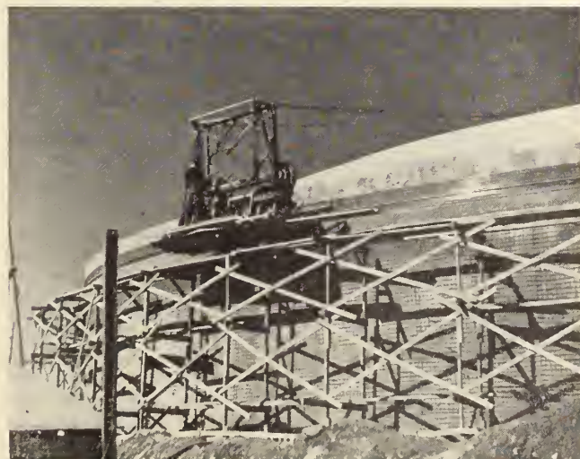
Fig. 5—Wire winding dome roof ring.
