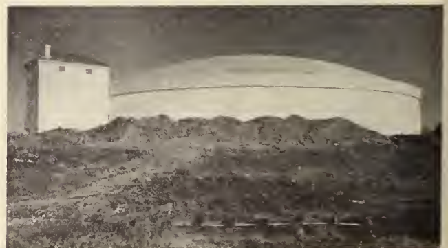
Fig. 6—Completed reconstruction before backfilling and grading.
