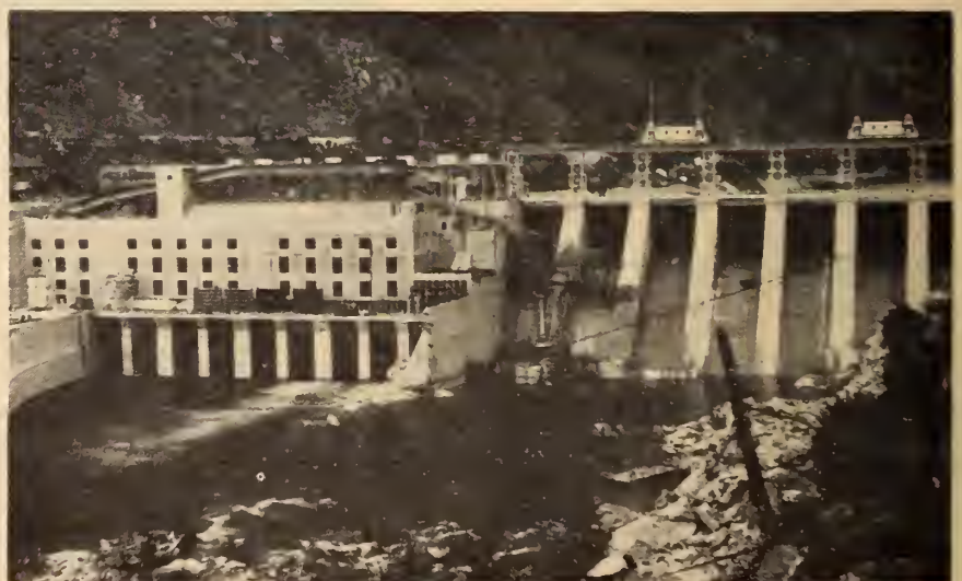
Right: West Kootenay Power and Light Company Limited No. 5 on the Kootenay River at Brilliant, about one mile above the Columbia River, where two generating units with rated capacity of 34,000 hp., when operating under 85-foot head, are installed. The power house is designed to hold four such units.
