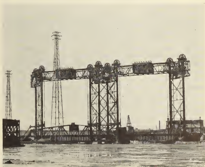
Fig. 5—Side elevation of bridge looking from the south.
