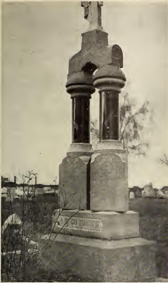
Fig. 7.—Rotation effect on monument. This rotation in a monument in a graveyard beside Rivière Ouelle church was caused by the earthquake of 1925. This is typical of rotations in epicentral regions where the soil is deep. This one happened to be contra-clockwise. Most of the rotations on the south shore caused by this earthquake were in this sense, the ones on the north shore turning clockwise as a rule. (This rule was exactly reversed in the case of the Cornwall-Massena earthquake of 1944.) Practically every stone in every graveyard in the epicentral region was either rotated or overthrown.
