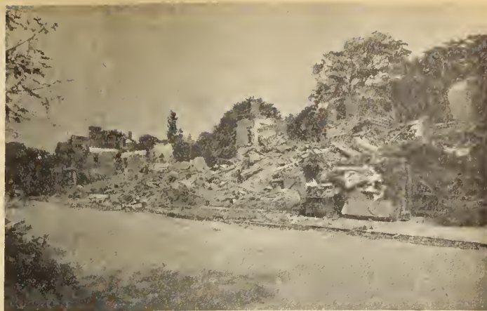
Fig. 6—Extent of damage caused by the incident of a flying bomb.
