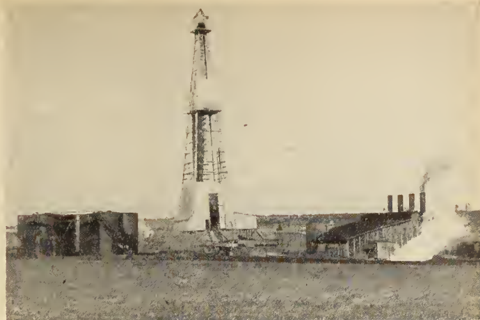
Rotary equipment operated by the Sun Oil Company near Amherst, N.S.
