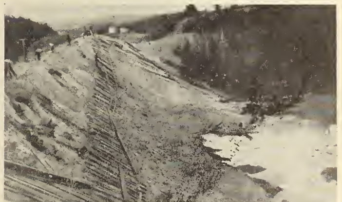
Fig. 8.—The Parent, Que., slide. This slide occurred on the railway near Parent, Que., at the time of the Timiskaming earthquake of November 1, 1935. It is more than 200 miles away from the epicentre.
