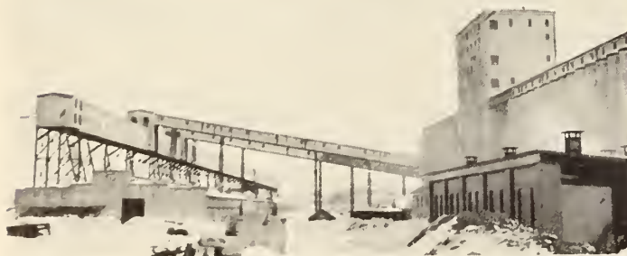
Fig. 3—Grain loading equipment on the banks of the St. Charles River at Quebec. This structure stands on deep, made ground. It is very top-heavy. At the time of the earthquake of 1925, the heavy superstructure of the distribution sheds (1,000 ft. long) swayed outward toward the river, but did not fall. The effect on the lower ends of the outer steel struts is shown in Figs. 4 and 5.
