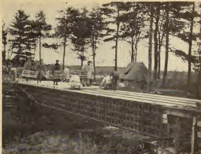
Fig. 9—Timber decking being placed on four fifty-foot bridge assemblies.
