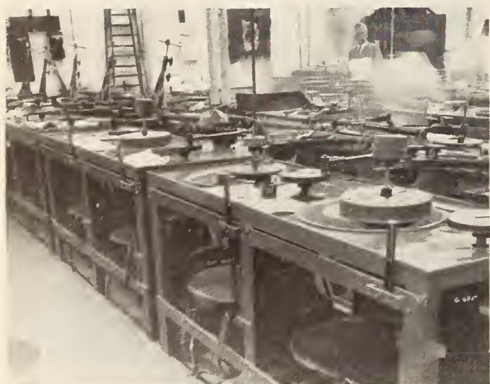
Fig. 18—A row of planar polishing machines with plaster blocks.
