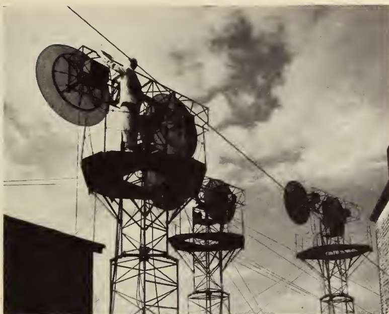
Fig. 4—Searchlight antenna used with AN/TRC-6 microwave pulse modulated radio relay system.
