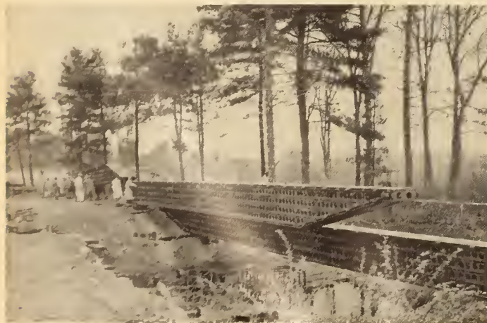
Fig. 1—Launching of bridge by cantilever method.
