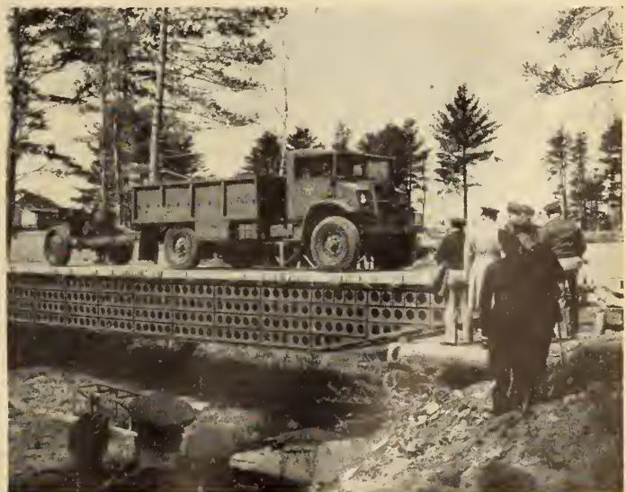
Fig. 10—Fully loaded three-ton truck weighing 16,000 lb. towing a 3,100 lb. gun. Total live load of 19,000 lb.
