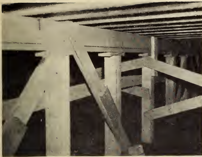
Fig. 7—Shimming under warehouse floor.
