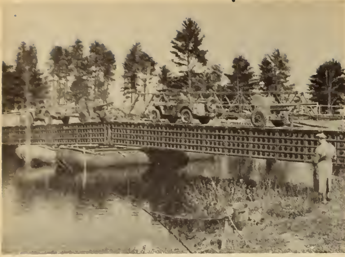
Fig. 11—Long spans supported on pontoons.
