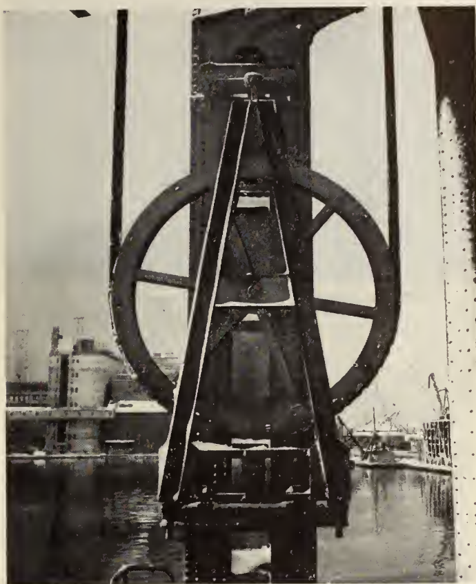
Fig. 9—Wheel to restrict the swing of counterbalancing chains. The weight of this wheel is carried by the chain. Wheel supports are carried on bridge post in such a way as to permit unrestricted vertical motion of wheel due to variegations in length of chain.
