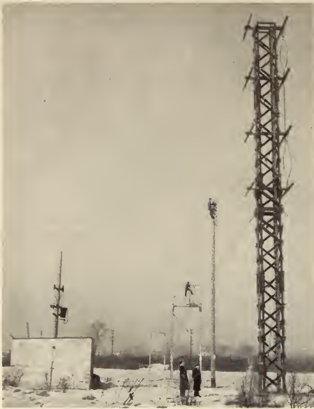
Fig. 2—Experimental antenna station, Lachine, Que., used to check characteristics of VHF antenna structures for telephone relay station used on East Coast defence system.
