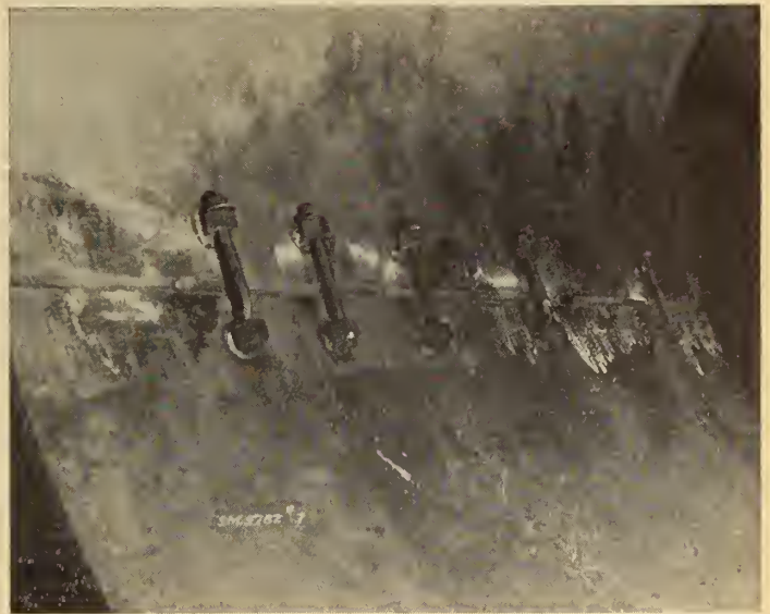
Fig. 2—Preparation of longitudinal seam, showing draw bolts and tack welds.
