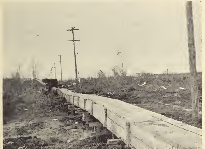
Fig. 8—Alignment of utility line after one cycle of freezing and thawing.
