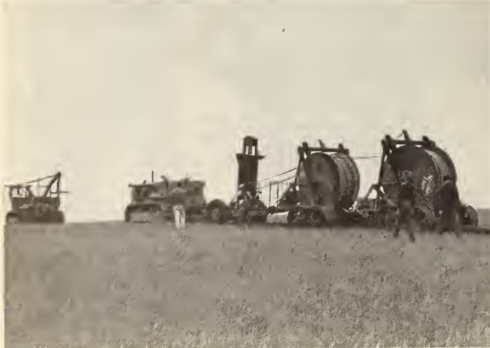
Fig. 2 Skyline view of plough train underway.
