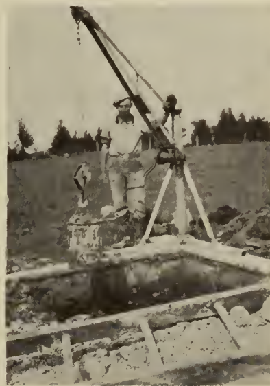
Fig. 4—Digging test pits for borrow area exploration.
