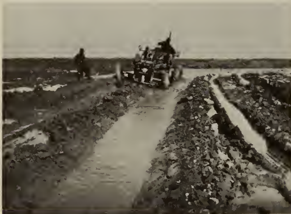
Fig. 8—Airport Drainage—Using Blade Grader for “V” Ditch.
