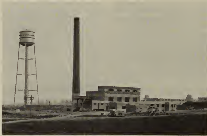
Power Plant of the Ontario Mental Hospital, St. Thomas, Ont.
