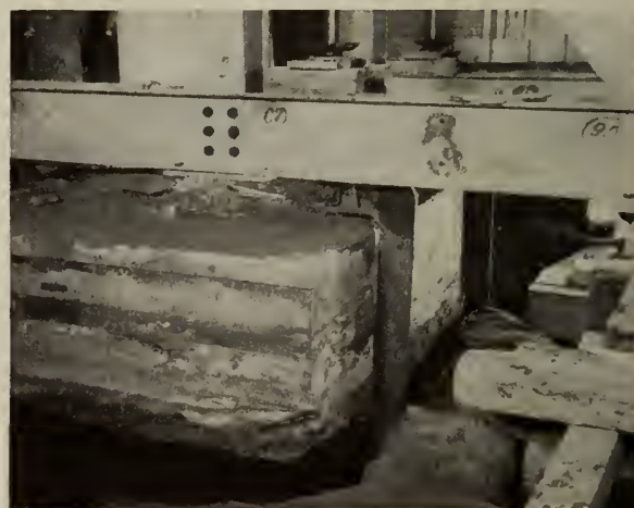
Fig. 6—Footing block suspended by hooks, excavation complete ready for lowering.
