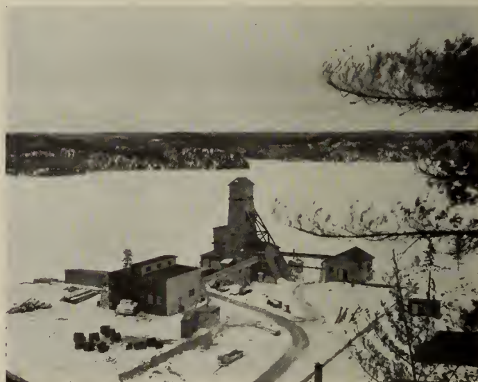
Fig. 6—Surface plant at Middle Arm.
