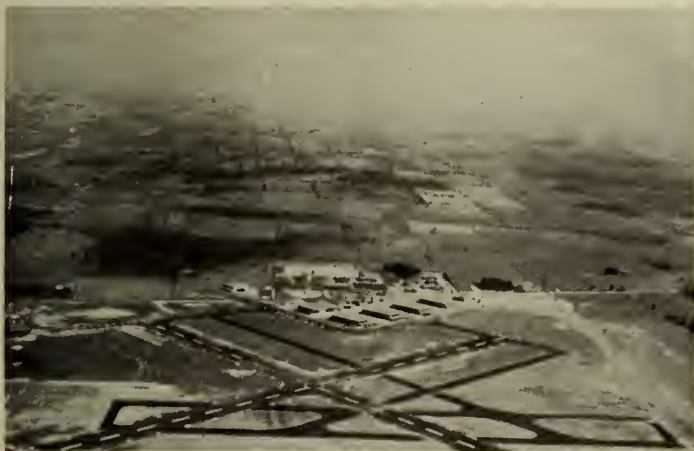
Fig. 2—Ottawa Airport Modified to Service Flying Training School.
