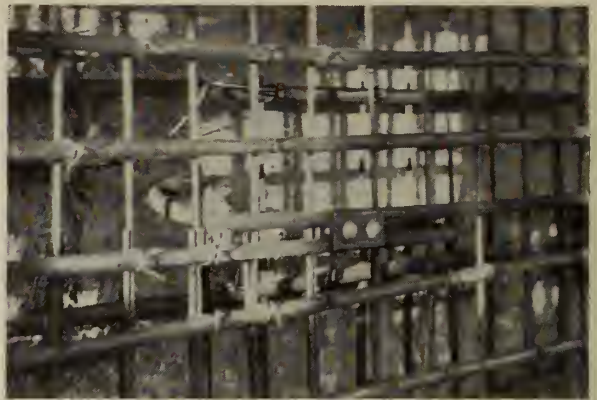
Bolted clamps in place.
