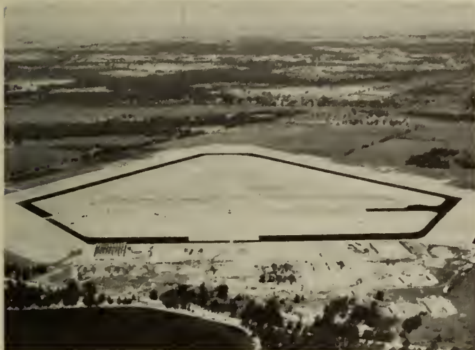
Fig. 6—Collins' Bay (Kingston)—Main Aerodrome for Service Flying Training School.
