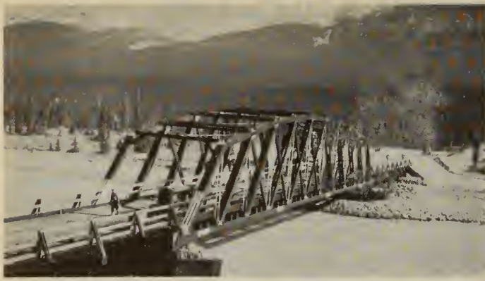
Fig. 3—Bow string treated truss, North Saskatchewan River.
