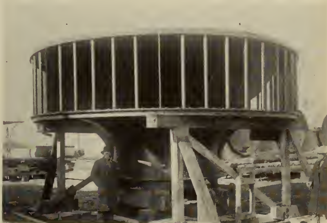
Fig. 3—Inlet to Intake (20 ft. diameter), Victoria Park.
