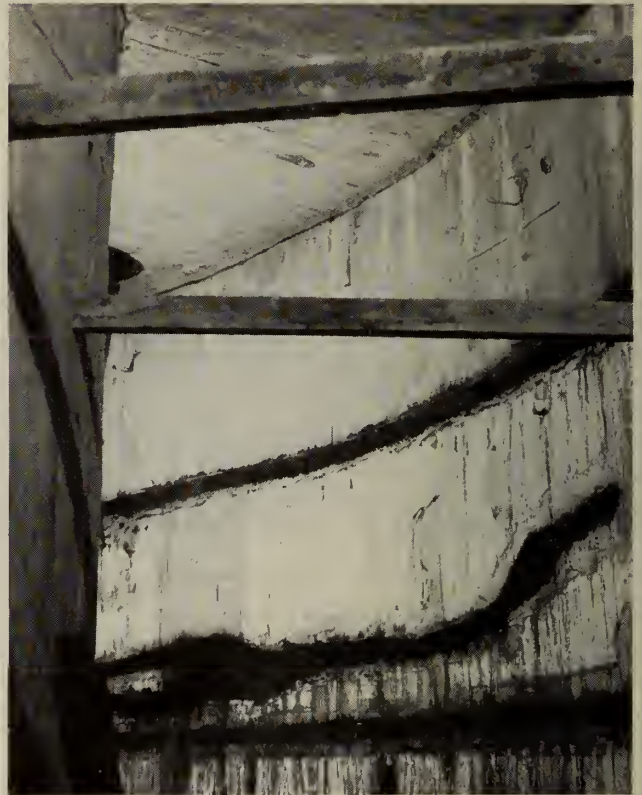
Fig. 5—Sealed horizontal joints in reinforced concrete scroll case.
