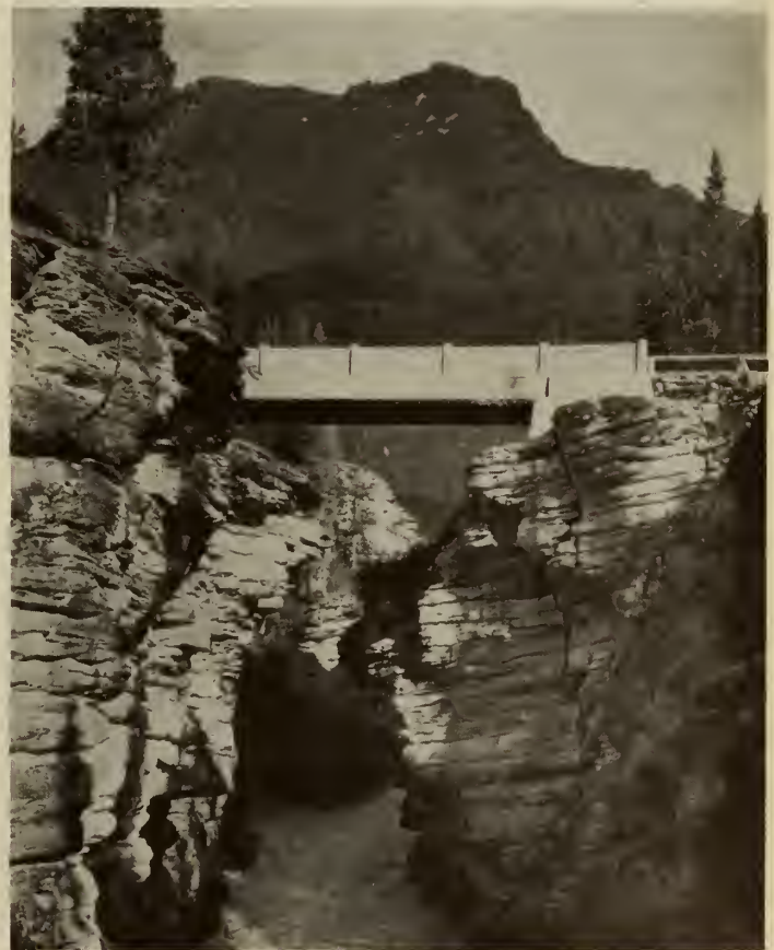
Fig. 2—Typical concrete girder bridge, Athabaska River.
