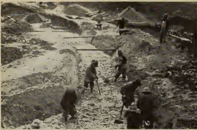
Fig. 6—Building Choquetanga Dam.
