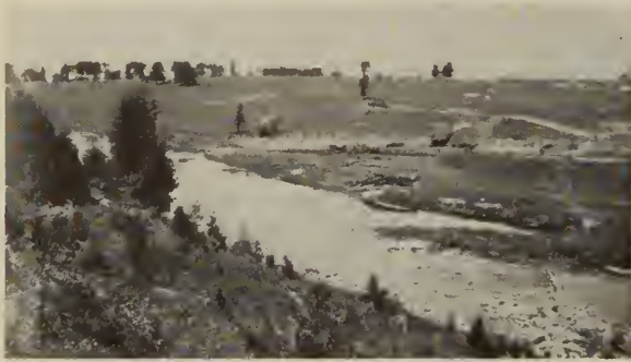
Fig. 2—General view from east abutment at commencement of work, June 1939.
