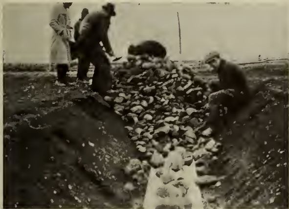
Fig. 9—Stone Filled "V" Ditch.
