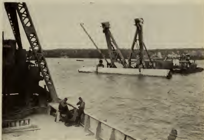
Fig. 2—Placing Intake Pipe—Victoria Park Intake.
