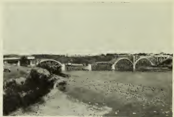
Fig. 14—Progress at August 10th, 1932.
