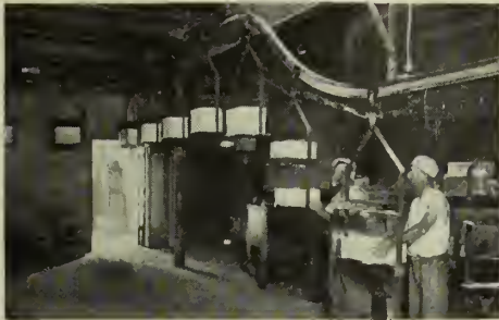
Jeffrey Trolley Conveyor handling Saggers.
