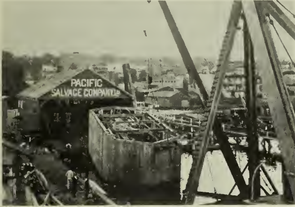
Fig. 27—Caisson 1B stuck on Ways at Launching, at Point of Sliding Off.
