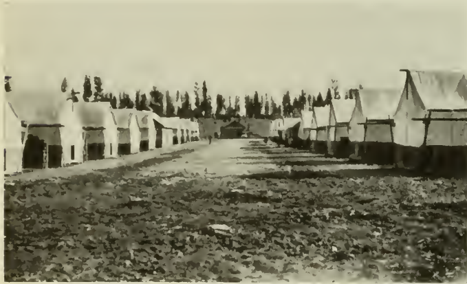
Fig. 1—Frame and Canvas Camp Buildings, Kimberley-Wasa Highway, B.C.
