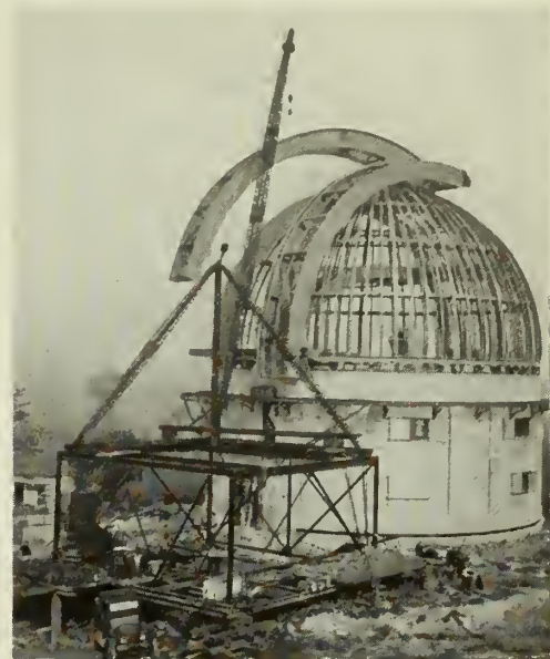
Fig. 15—Building with Dome Partially Erected.
