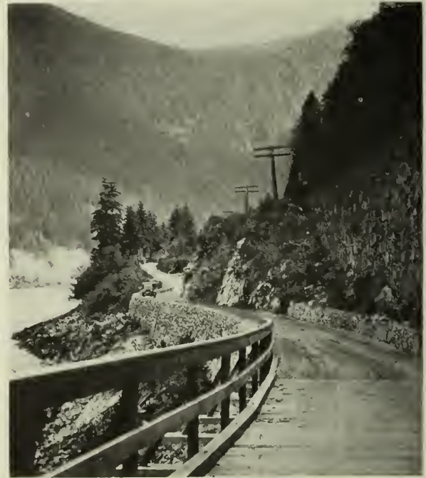
Fig. 6—Cariboo Highway, Fraser River Section.
