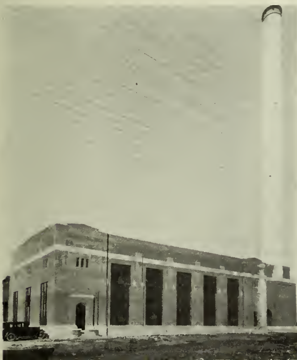
Fig. 1—Wall Street Steam Station.
