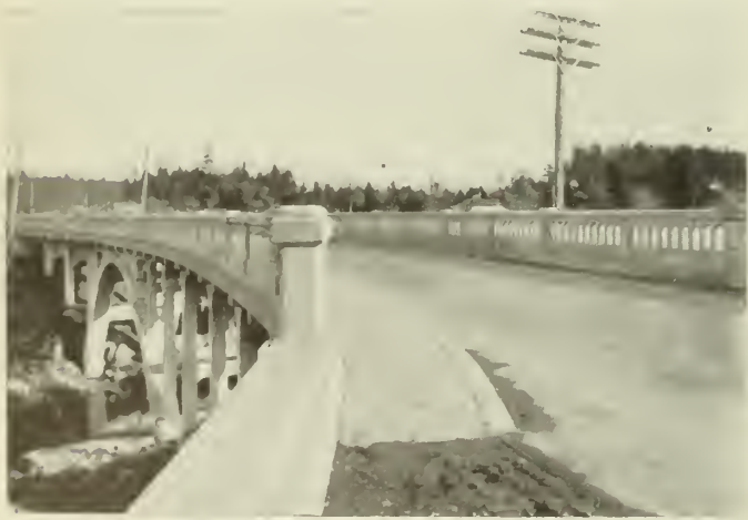
Fig. 12—Parsons Bridge on Island Highway, Victoria, B.C.
