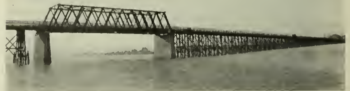
Fig. 9—Fraser Avenue Bridge over North Arm of Fraser River.
