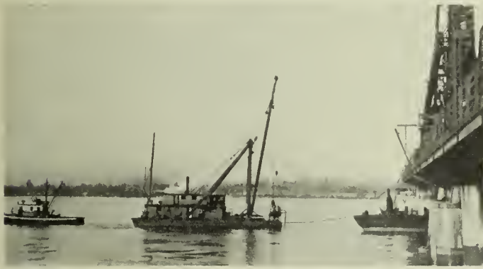
Fig. 21—Placing 30-ton Anchor for 2B, October 11th, 1933.
