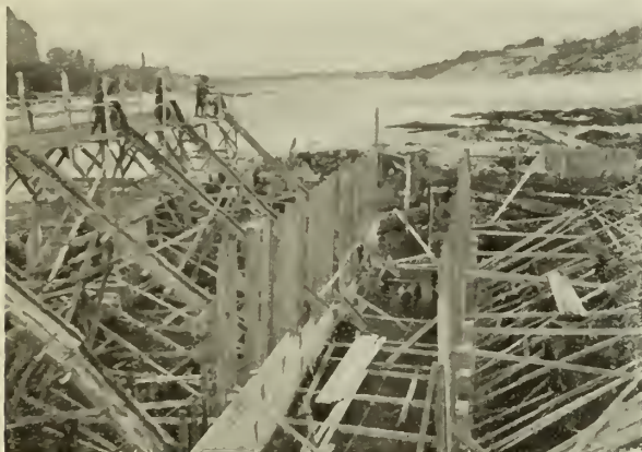
Fig. 12—Forming and Pouring, Pier 3, February 26th, 1932.
