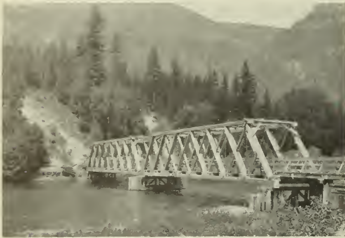
Fig. 8—Bridge over Slocan River at Vallican.
