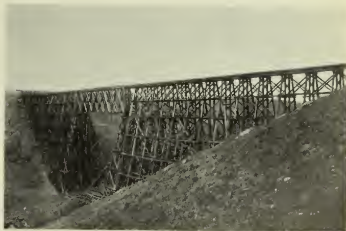
Fig. 2—Structure over Creek Adjoining the St. Mary's River.
