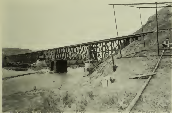
Fig. 1—St. Mary's River Crossing.
