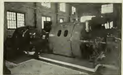
At Noranda. Westinghouse 2800 H.P. Motor, 550 V., 750 r.p.m., driving blower supplying air for converters.
