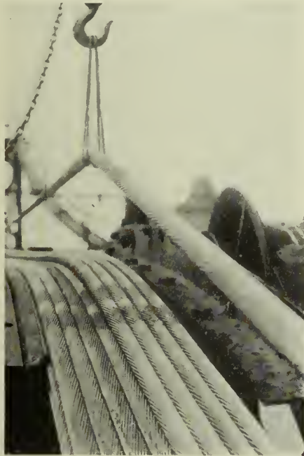
Fig. 4—Right and Left Lay Rope Strands in Adjacent Layers—Maysville Bridge.
