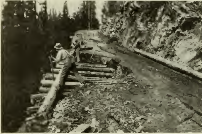
Fig. 7—Cribwork, Big Bend Highway, North of Revelstoke, B.C.
