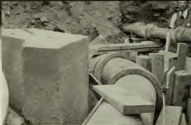
Anchorage used at bend in line.
