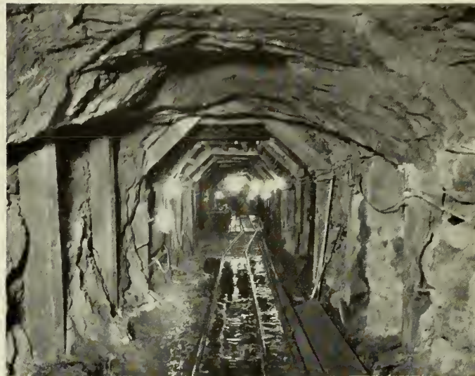
Fig. 5—Tunnel, showing Invert, Permanent Rails, Timbered Section and Gunite on Sidewalls.
