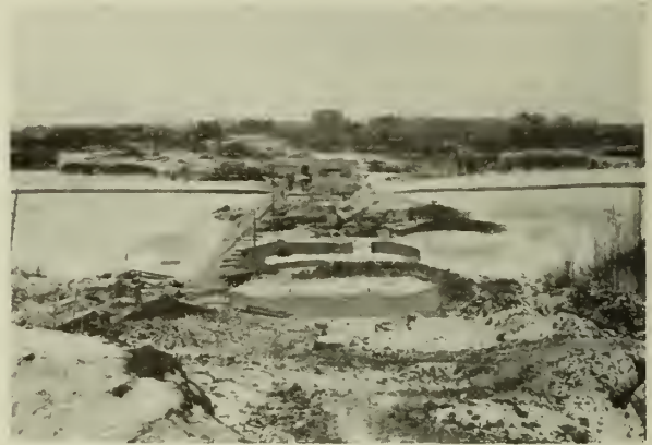
Fig. 10—Work in Progress, February 19th, 1932.
