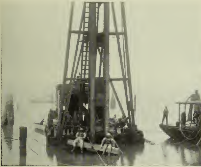
Fig. 17—Pile Driver ready to lower Bent Cap.
