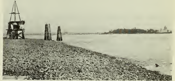
Fig. 3—Drilling Hole No. 53, Calamity Light in Background.
