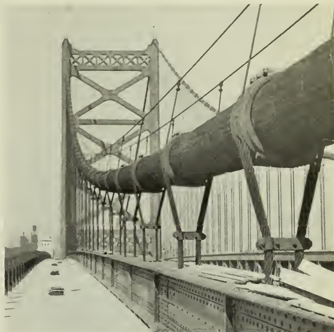
Fig. 2—Type (a) Main Cable as Compacted into Cylindrical Shape—Philadelphia Bridge.
