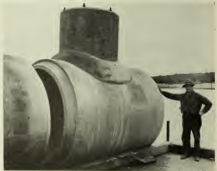
Fig. 20—T-Pipe with Manhole.
