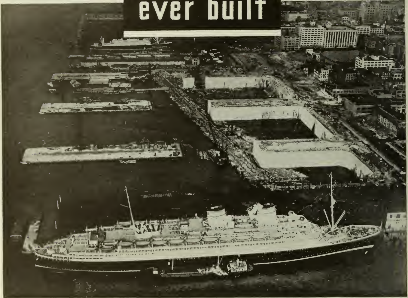
Contractor: Allen N. Spooner and Son, Inc.; Consulting Engineer: H. A. Sloane.
