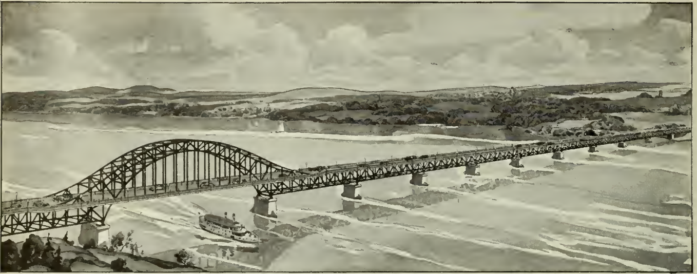
●New steel highway bridge now being constructed over the St. Lawrence River, between Ville LaSalle and Caughnawaga, just west of Montreal. Length 2919 feet, Roadway 27 feet wide.
