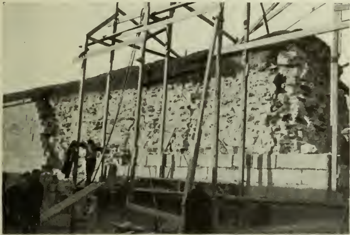
Fig. 9—Repairing Citadel Walls, Quebec, Que.
