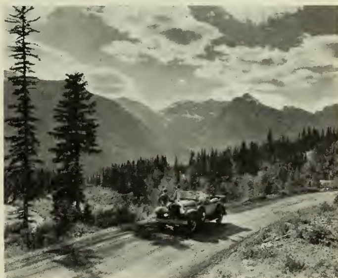
Fig. 2—Trans-Canada Highway in Banff National Park. Massive Range in Background.
