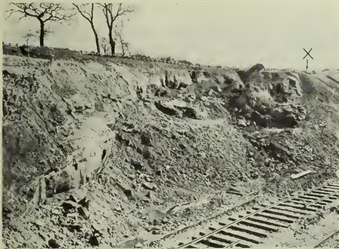
Fig. 6—L.M. and S. Railway, England. Combination of Trough Slips as under X and Hanging Wall Slips.
