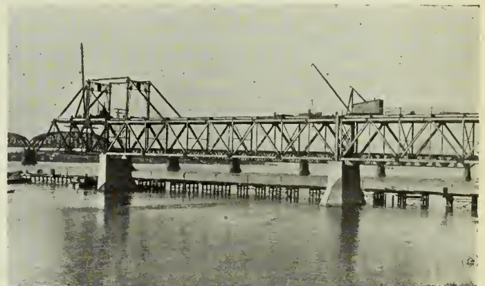
Fig. 9—Saddle Fully Erected.
