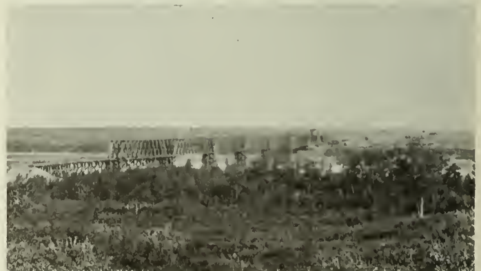
Fig. 22—First Bridge across the Saskatchewan at Saskatoon.
