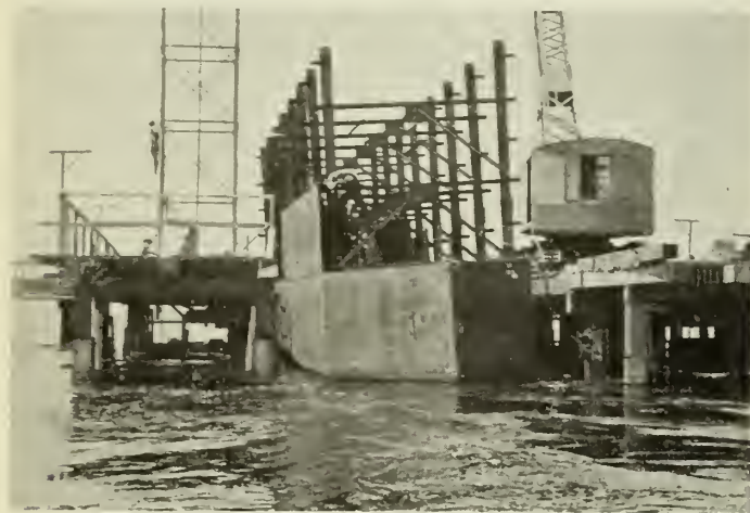
Fig. 6—Erecting Caisson Steel.
