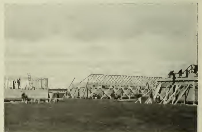
Fig. 3—Hut Construction, Dundurn, Sask.
