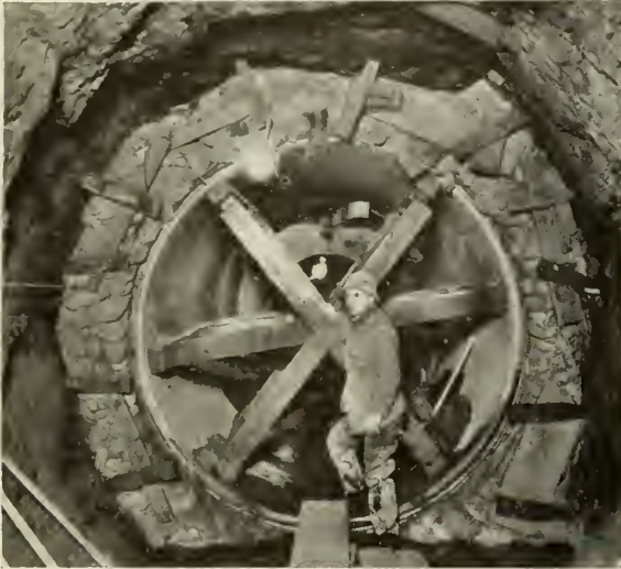
Fig. 10—Bulkhead in Place and Concrete Setting.
