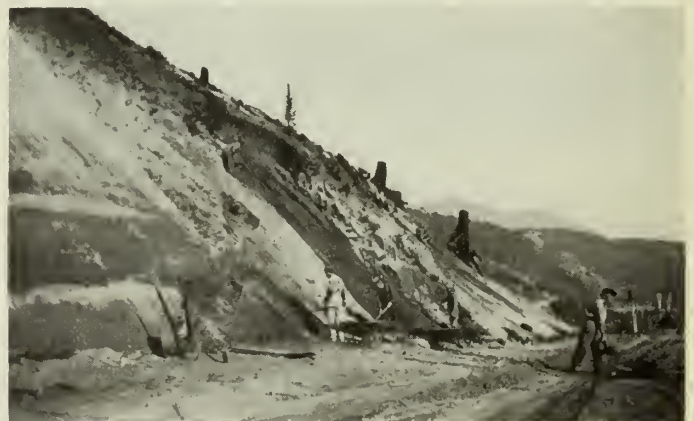
Fig. 6—Highway Construction near Tadanac, B.C.
