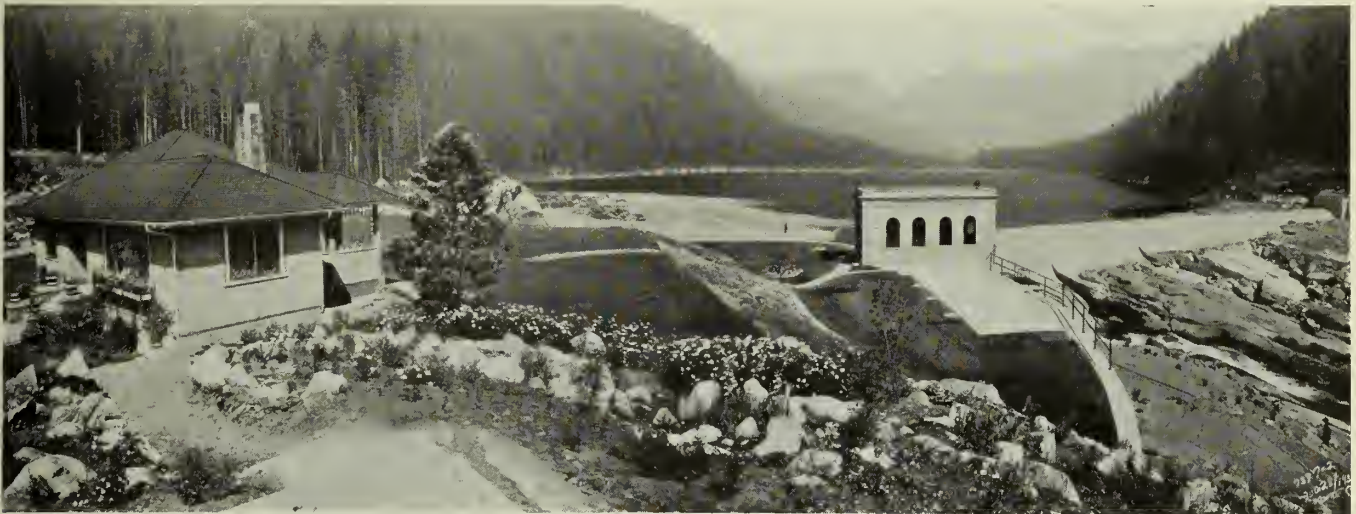
Seymour Falls Water Intake, Vancouver, B.C.
