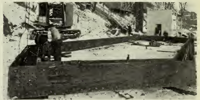
Fig. 5—Cutting Edge, Caisson No. 3.
