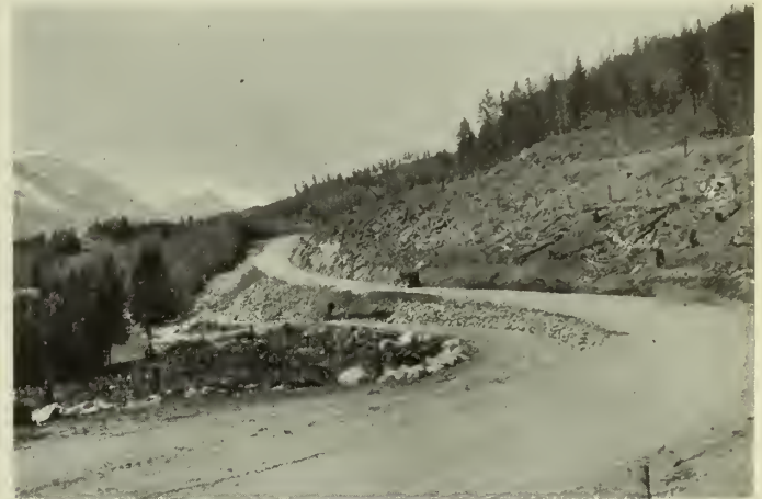
Fig. 7—Diversion of New Denver-Rosebery Road.
