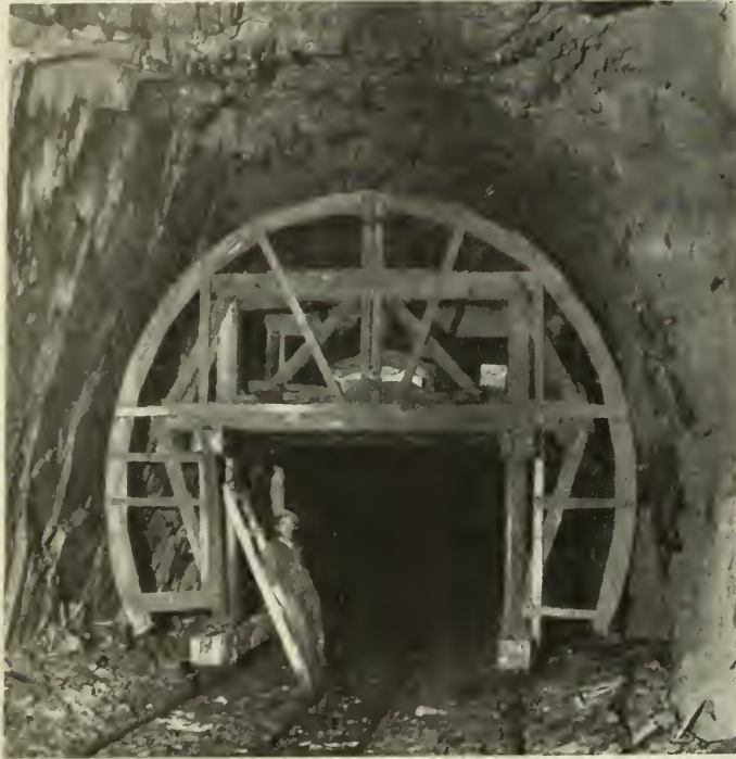
Fig. 5 -Tunnel Running along Strike.
