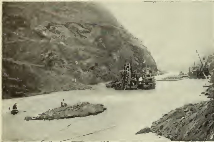
Fig. 1—Gaillard Cut, Culebra, Panama Canal.
