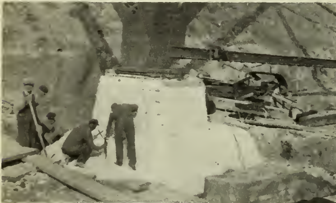
Fig. 7—Cutting away Top of Old Pedestal.
