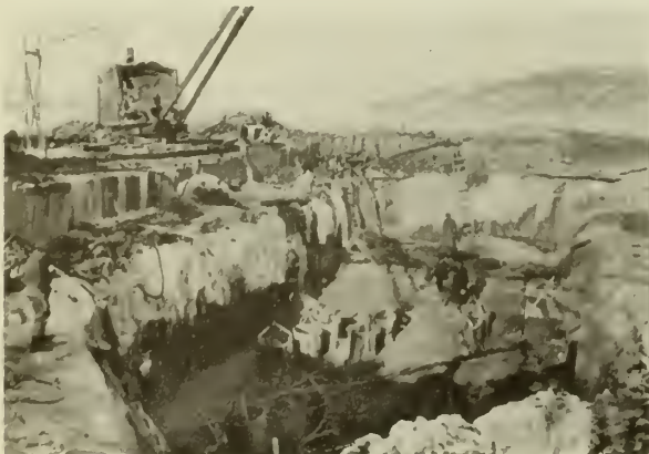
Fig. 9—Excavation for Pier 5, March 10th, 1932.
