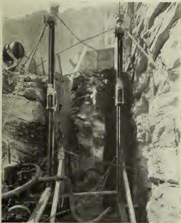
Fig. 9—Wire Saw Rigs Set up in Calyx Drill Holes.
