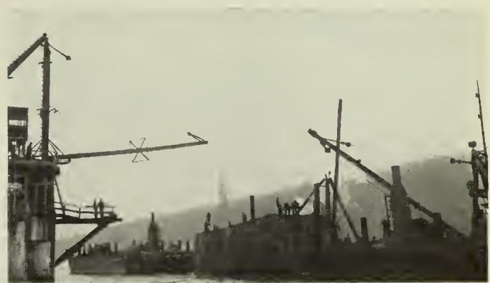
Fig. 29—Caisson 1B from northwest, November 17th, 1933.
