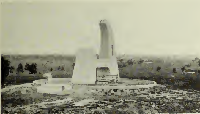
Fig. 14—View of Site from Southeast showing Piers.
