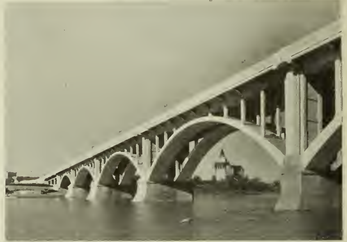
Fig. 2—Broadway Bridge Completed.
