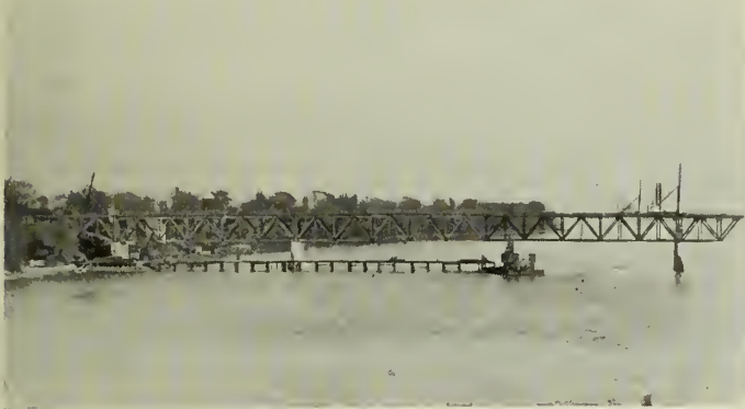
Fig. 8—First Stage of Cantilever Erection.
