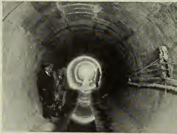
Dec. 21, 1931—Intake from Shaft South
