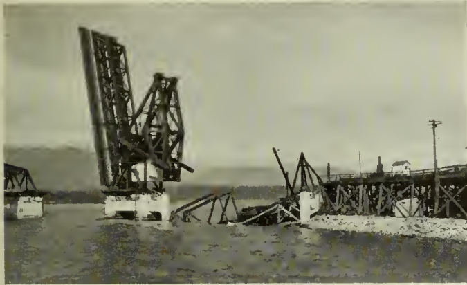
Fig. 3—Accident in April 1930, 150-foot span being cut up.
