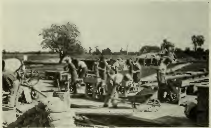
Fig. 8—Making Concrete Blocks, Air Station, Trenton, Ont.
