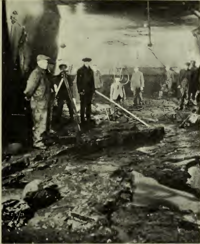
Fig. 10—Working Chamber of Caisson No. 3.
