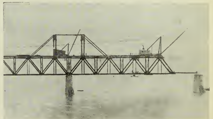
Fig. 10—Second Stage of Cantilever Erection with Saddle Functioning.
