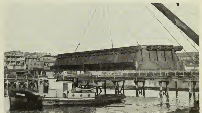
Fig. 24—Steel Assembly being Landed from Scows.
