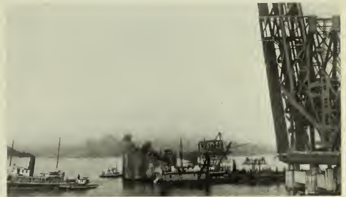
Fig. 23—Caisson 2B—October 12th, 1933. Taken from Roadway.
