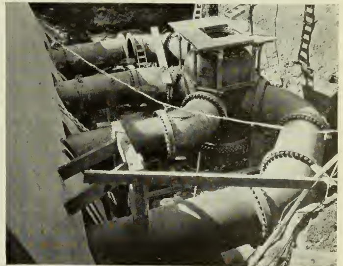
Fig. 13—Pipes Between South Shaft Cap and Valve Chamber.
