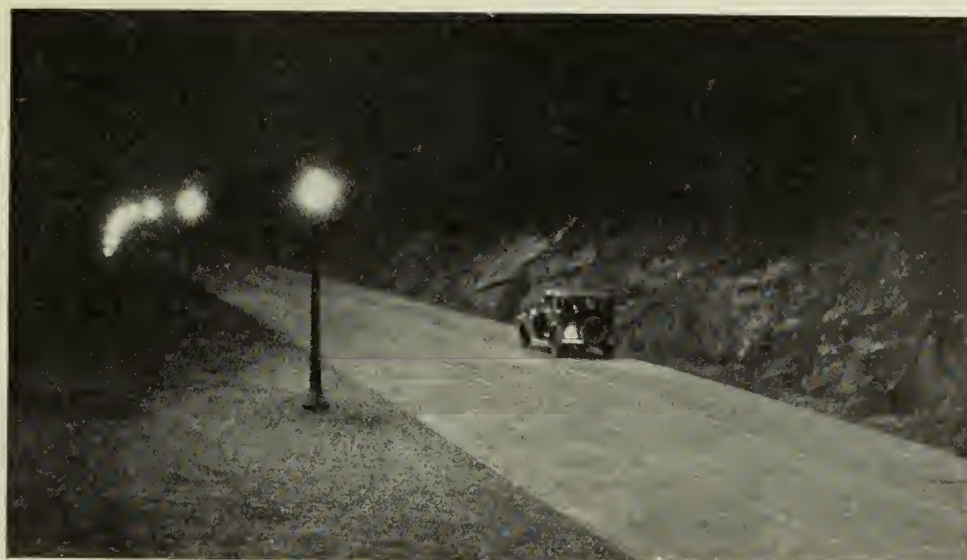
Fig. 4—Highway Lighting with Sodium Vapour Lamps.
