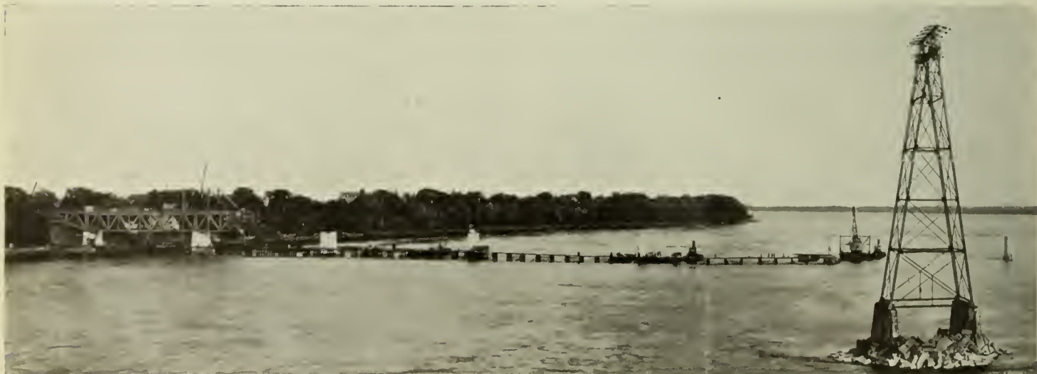
Fig. 1—General View Downstream of Bridge under Construction.
