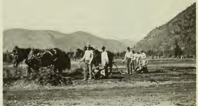
Fig. 10—Grading Landing Field, Salmo, B.C.
