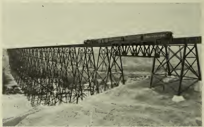
Fig. 4—Lethbridge Viaduct from North West.
