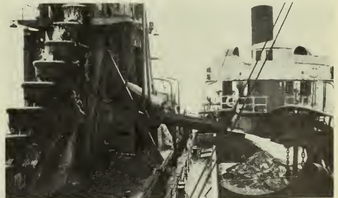
Fig. 5—Broken Rock Being Deposited in Hopper.
