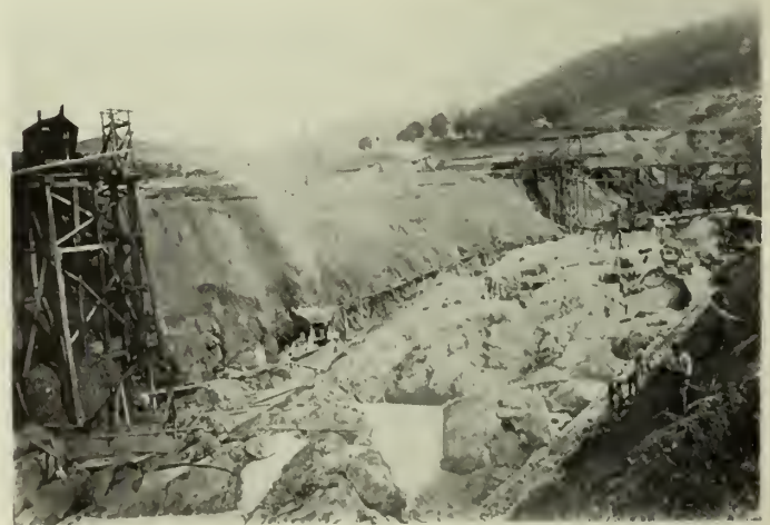
Fig. 3—Vyrnwy Dam showing Exposed Foundation Bed of Glaciated Rock.
