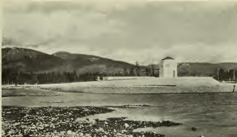
Access House, North Shaft.
