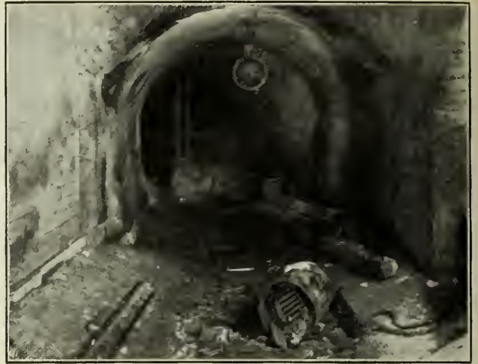
Figure No. 8.—Interior of Sewer, Looking Westwards, from Junction Chamber, Station 0+00.
