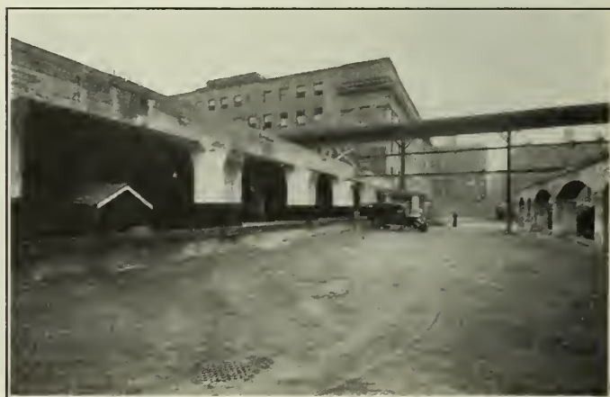
Figure No. 10.—Post Office Teamway before Erection of the Steel Spans which Carry the Overhead Tracks.
