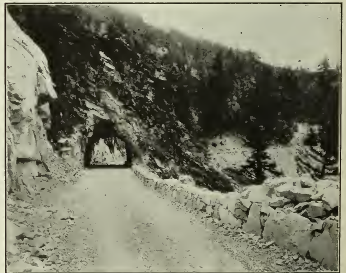
Figure No. 6.—Tunnels 19 miles North of Yale.
