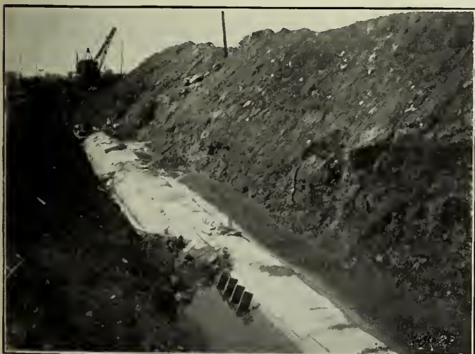
Figure No. 11.—General View of Works from Station 41 + 30, Looking Eastwards.
