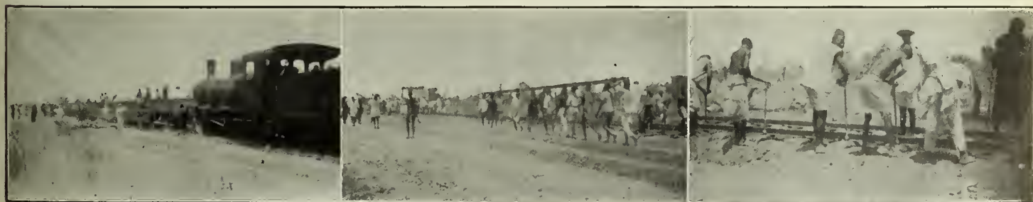
Railway Construction Work in Nigeria.
