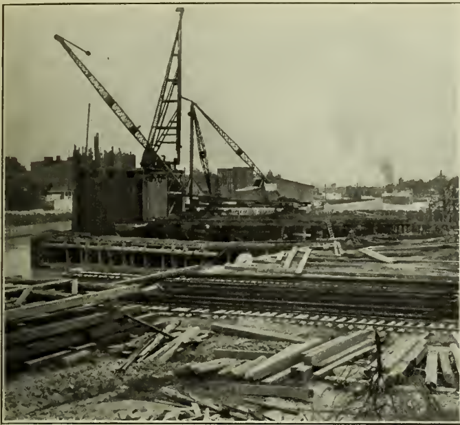
Figure No. 9.—Cofferdam Under Construction Looking South, June, 1926.
