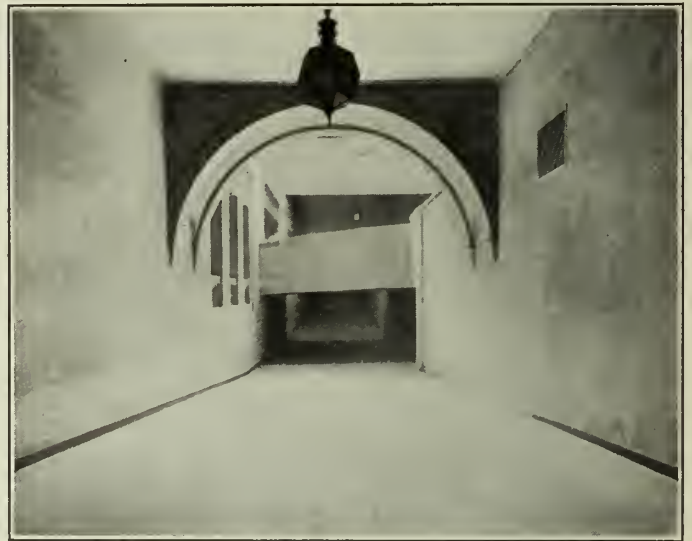
Figure No. 13.—View showing Junction of East and West Exit Passages under the Bridge Carrying the Ramped Passage Connecting Ticket Concourse (El.22) with Train Waiting Room (El.15.5).
