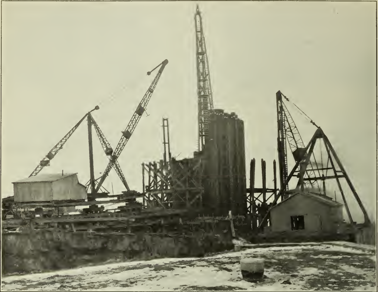
Figure No. 8.—Driving Cell Piling after Preassembly, February, 1926.
