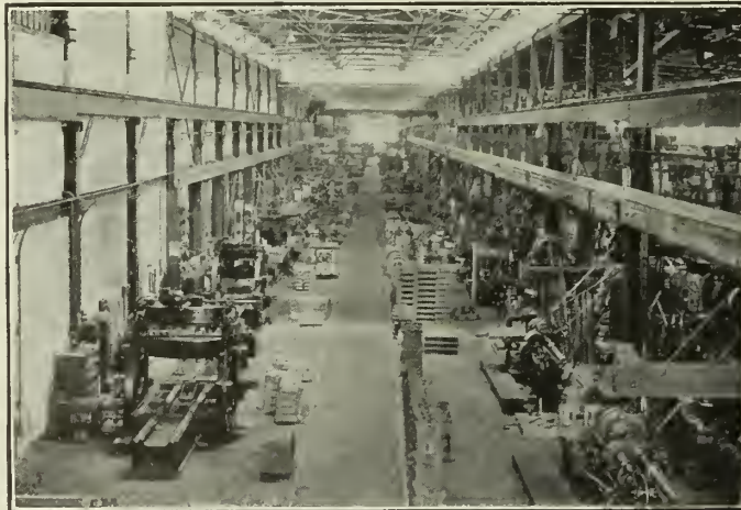
Machine Shop of One of the Manufacturing Plants to be Visited.
