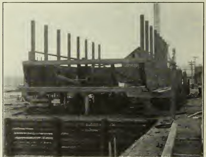
Figure No. 2.—Creosoted Scow under Construction—Timbers Framed before Treatment.
