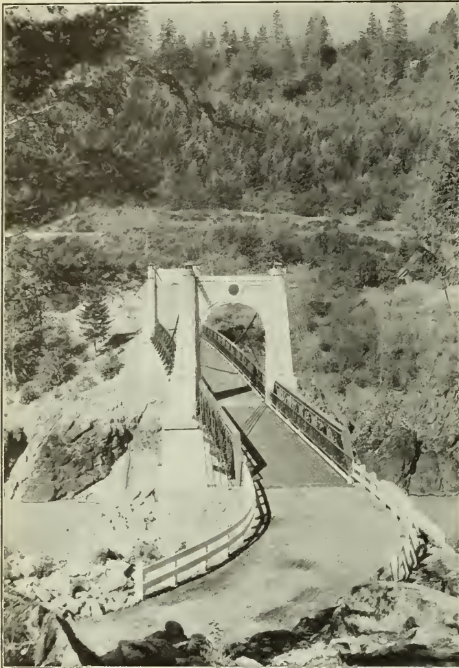
Figure No. 5.—Alexandra Bridge, Yale District.
