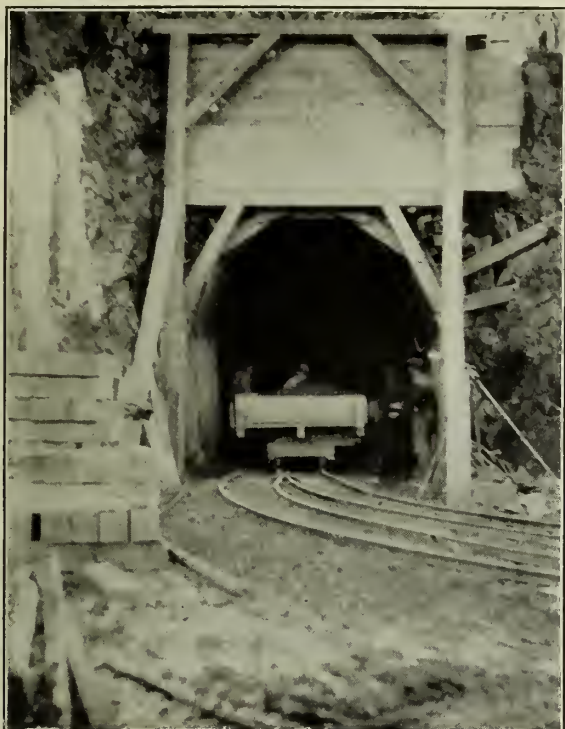
Figure No. 14.—Bridge River Tunnel Seton Portal.
