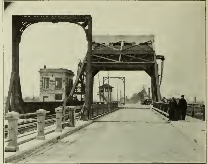
Figure No. 16.—Bridge No. 1—Front View Bridge Closed.
