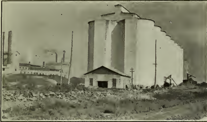
Plant of Canada Cement Company, Lakefield, Ont.
