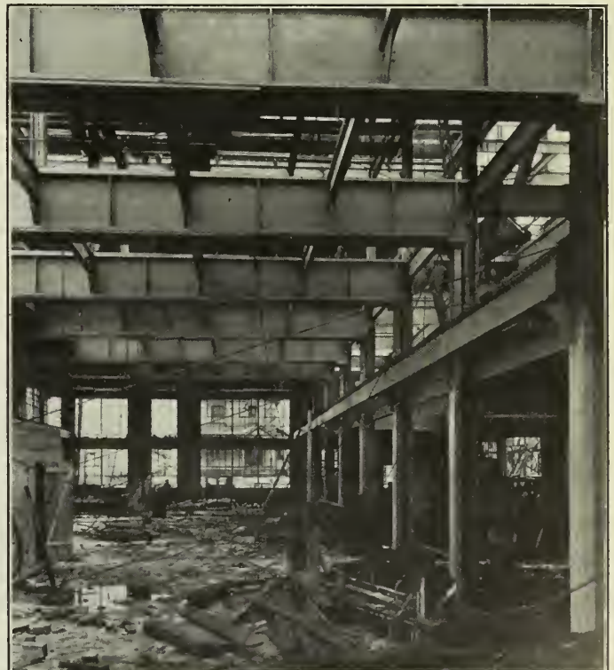
Figure No. 7.—View of the Plate Girders of the Sharon Building.
