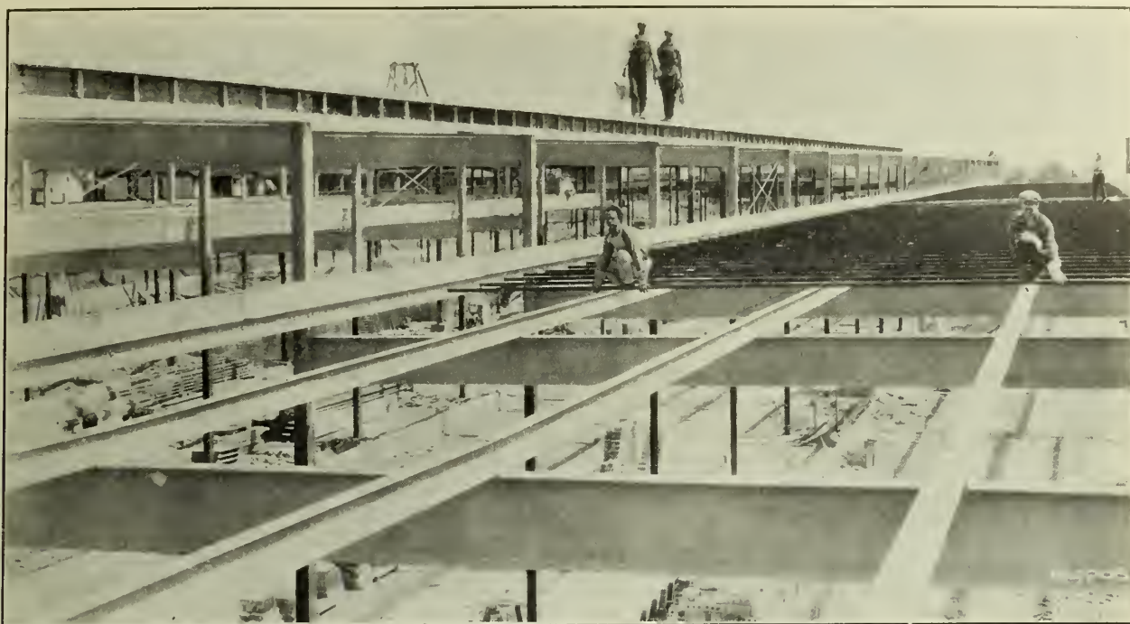
Figure No. 10.—Welded Steel-work of Building at Derry, Pa.
