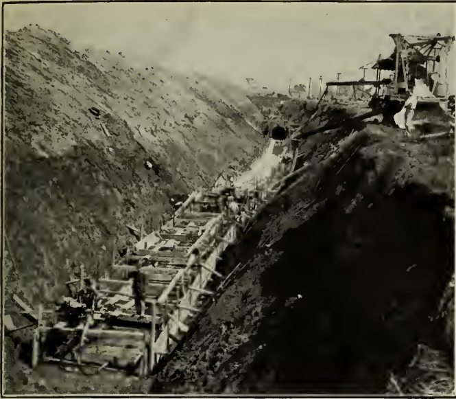
Figure No. 10.—General View of Works from Station 15 + 00, Looking Westwards.
