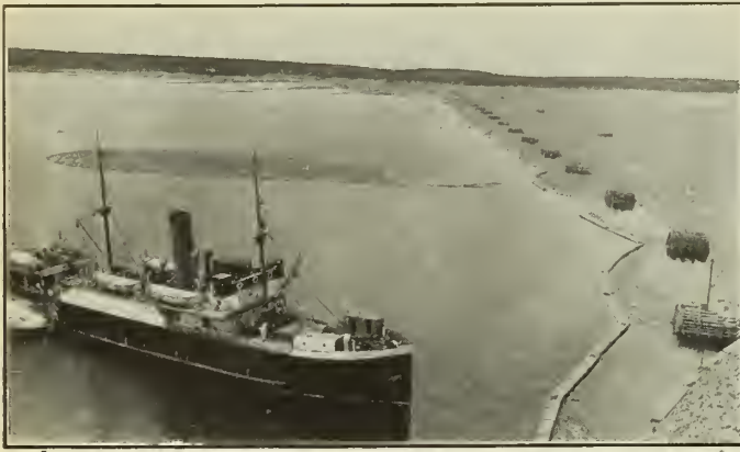
Figure No. 2a.—View from Loading Plant Looking Across Ellis Bay.
