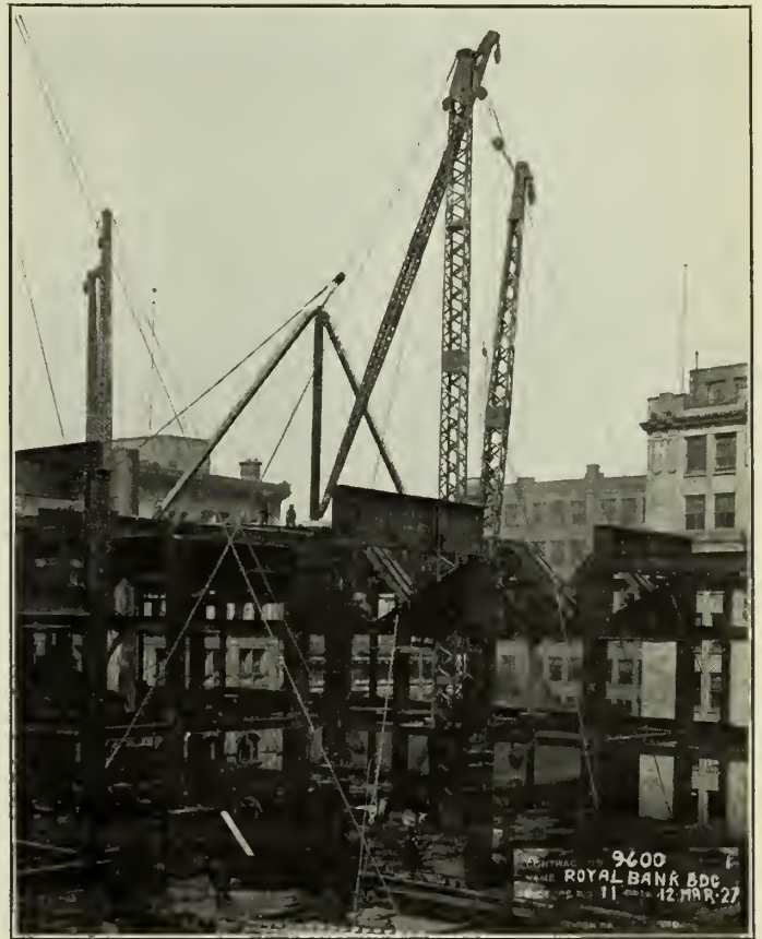
Figure No. 17.—Progress of Steel Erection, March 12th, 1927.
