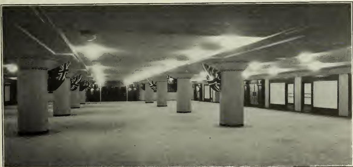
Figure No. 15.—Portion of Train Waiting Room after Completion.
