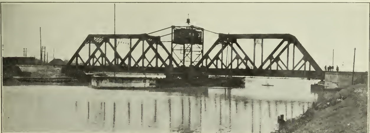
Figure No. 1.—Bridge No. 15.—Side View of Bridge Closed.
