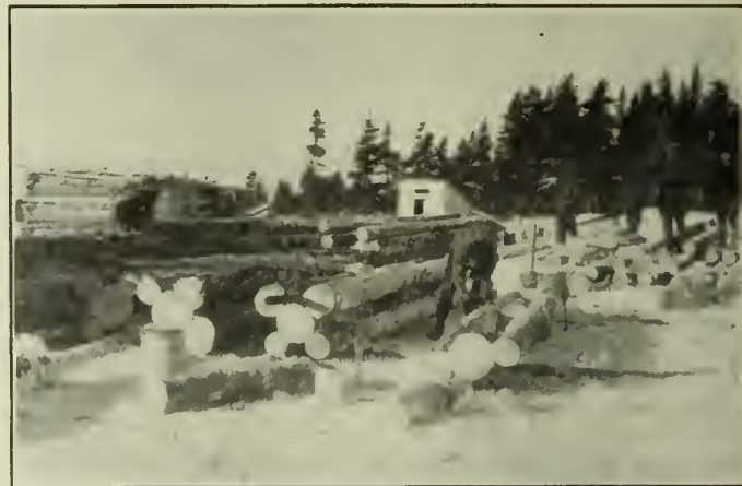
Figure No. 9.—Construction of Four-Piece Towing Boom.
