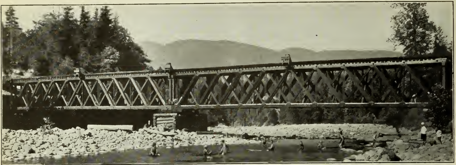
Figure No. 4.—Creosoted Deck—Howe Truss Railroad Bridge, Vancouver, B.C. All chords and web members were framed and then creosoted.
