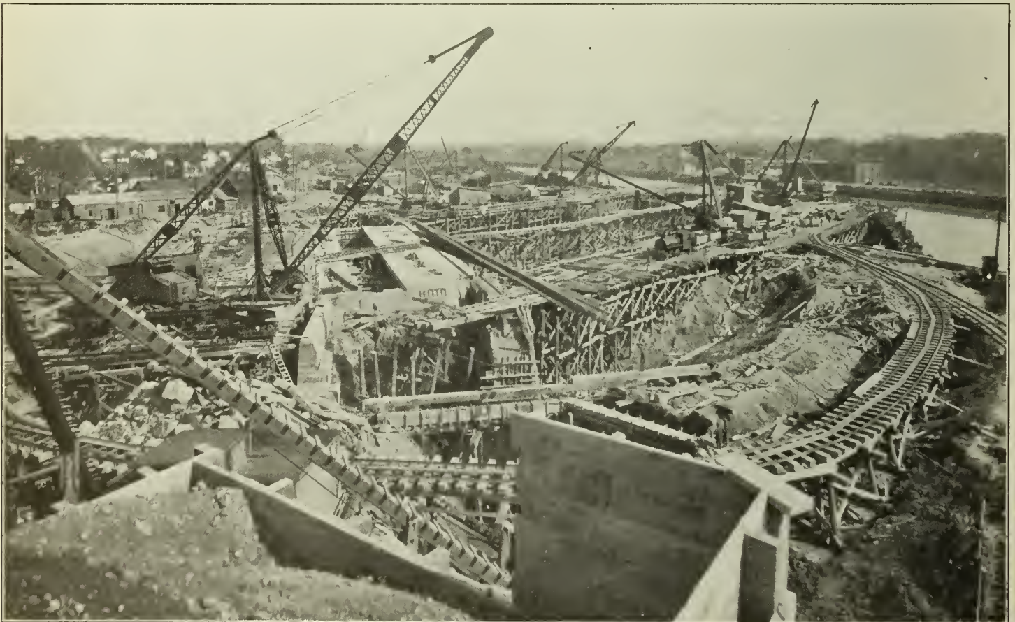
Figure No. 4.—General View of Works Looking Northeast, October, 1927.
