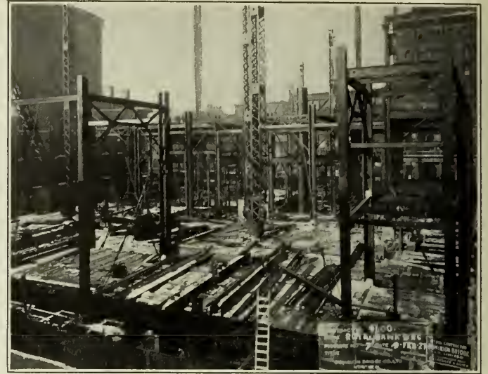
Figure No. 14.—Progress of Steel Erection February 9th, 1927.
