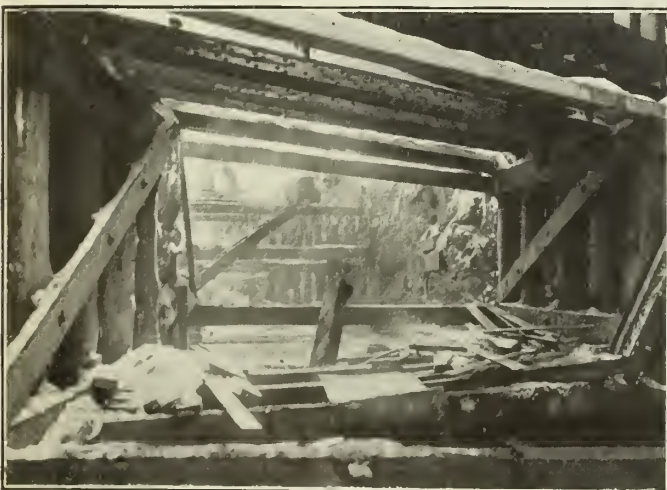
Figure No. 7.—View of Bracing under Canadian National Railway Tracks.
