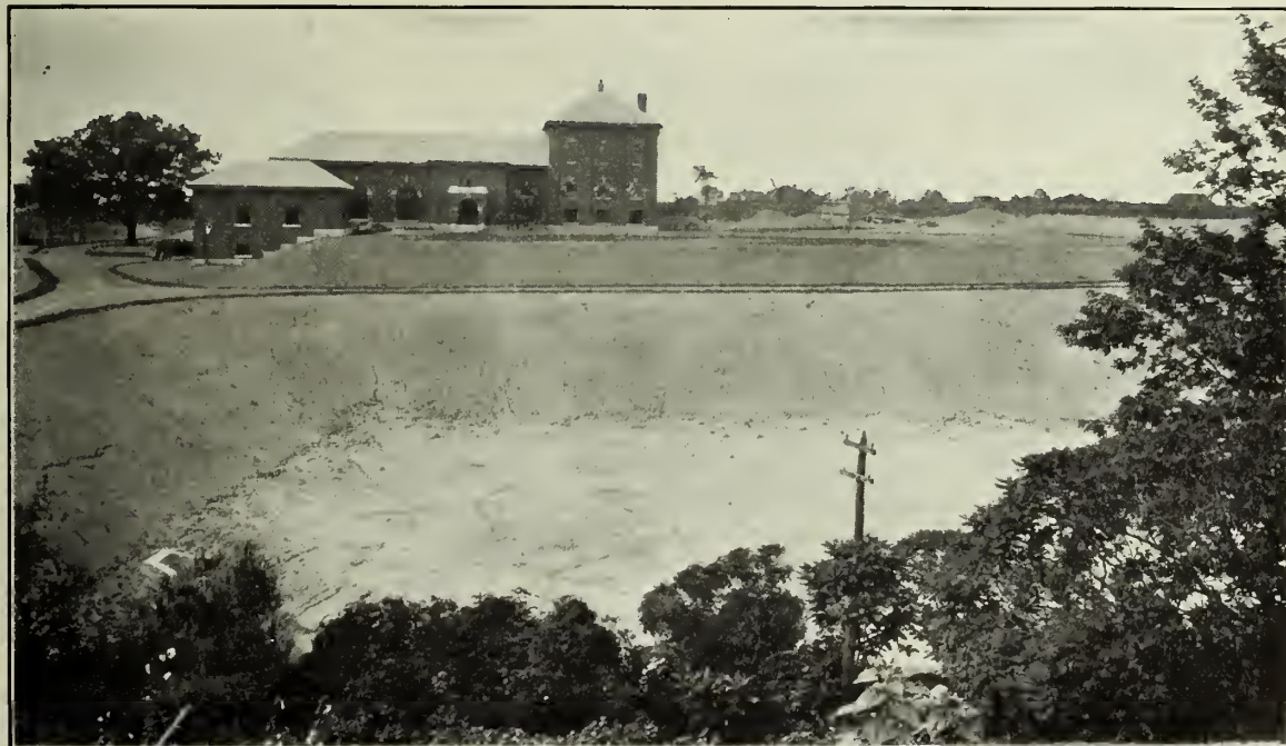
St. Catharines Water Works Filtration Plant.
