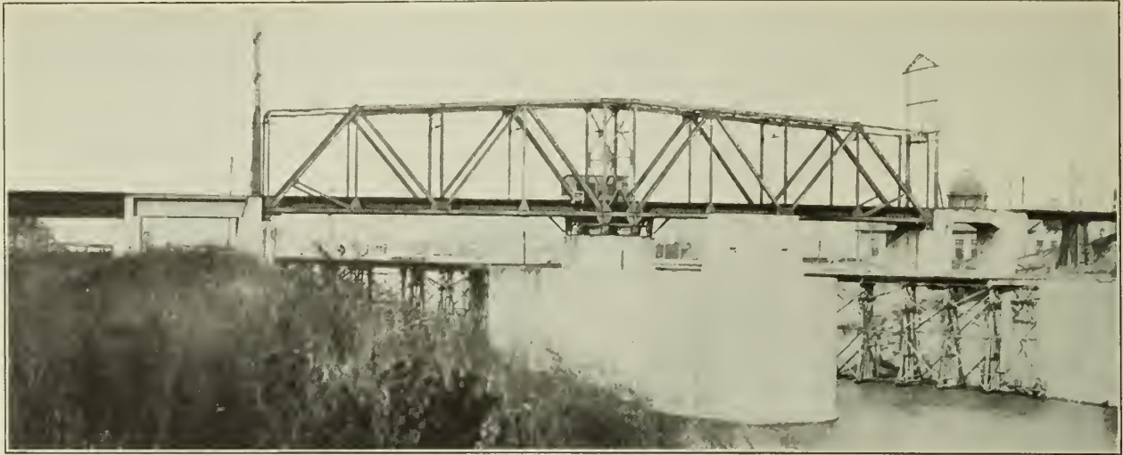
Figure No. 4.—Bridge No. 8.—Side View of Bridge Closed.
