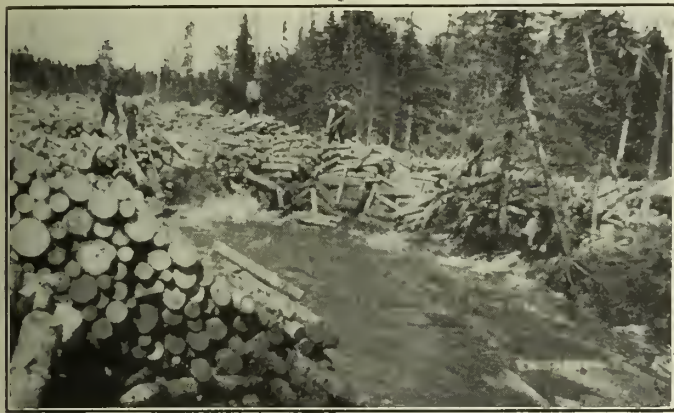
Figure No. 5.—Commencement of Drive on Canard River.
