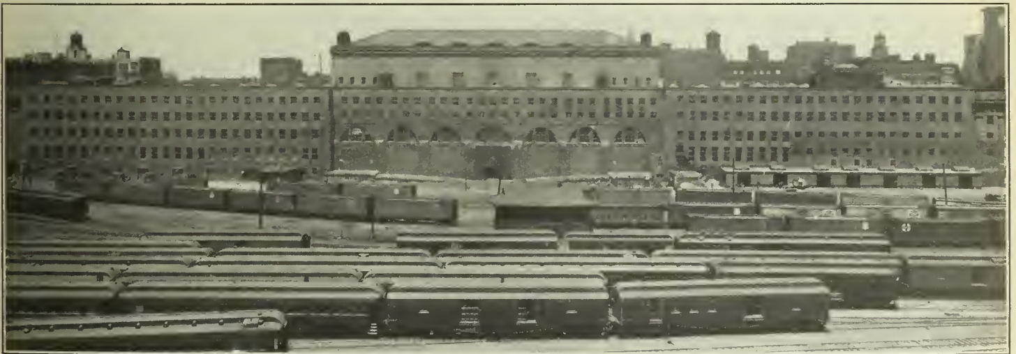
Figure No. 1.—View Looking North showing Rear of Station Building and a Portion of the Site before Construction.
