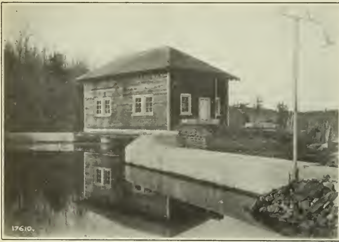
Figure No. 18.—Concrete Eight Years Old that Was Designed to Have Low Porosity but which Tested only about 1,500 pounds per Square Inch at Twenty-eight days.
