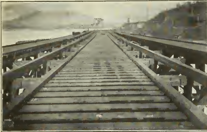
Figure No. 1.—Pre-framed and Creosoted Railway Trestle Approach to Alberta Wheat Pool Elevator, Vancouver, B.C.
