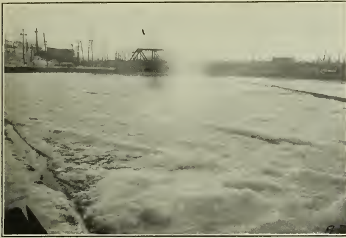
Figure No. 6.—Severe Ice Conditions in Forebay, Shawinigan Falls.
