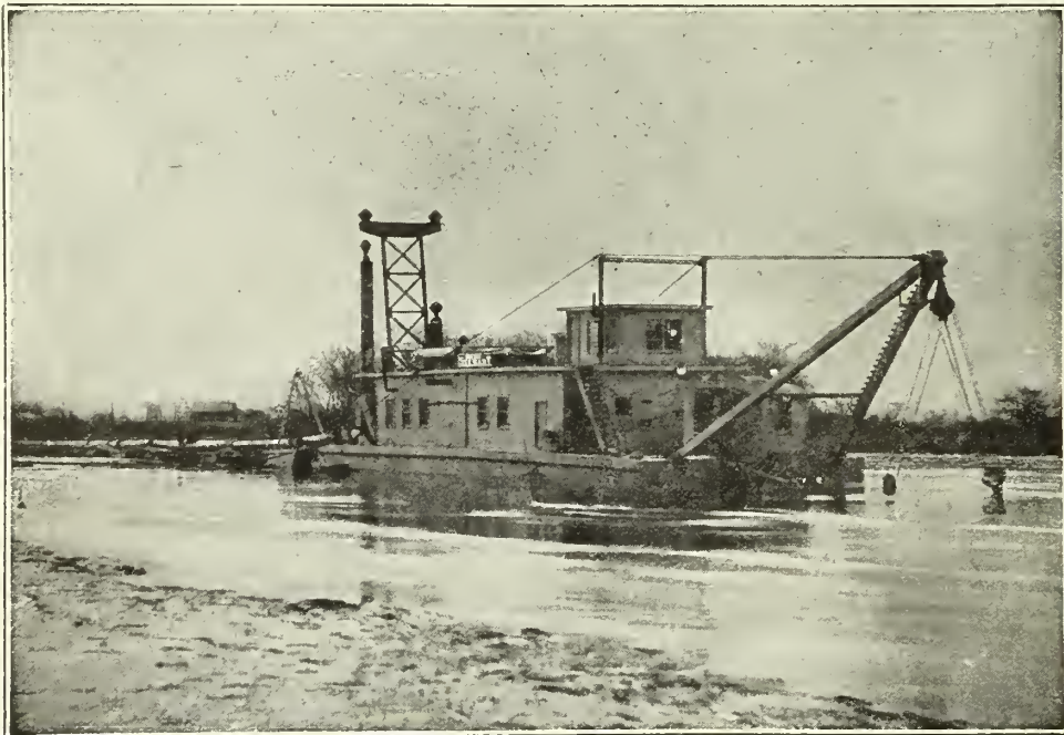
Electric Dredge on Queenston-Chippawa Power Development
