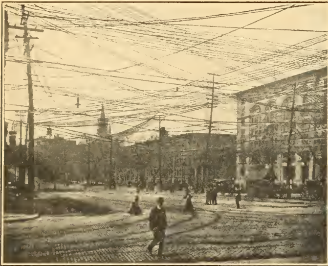
Figure No. 1.—Victoria Square, Corner of St. James and McGill Streets before removal of overhead wires.
