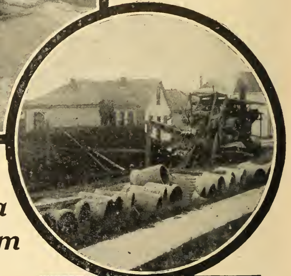
Concrete Sewer Hamilton, Ont.
