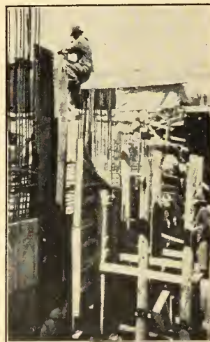
Figure No. 10.—Erecting Bedded Parts before pouring the Mass Concrete.
