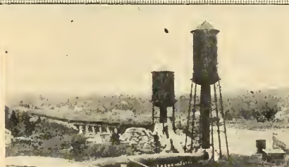
Power protects need surge tanks and penstocks that are fabricated and erected to the highest standards.
