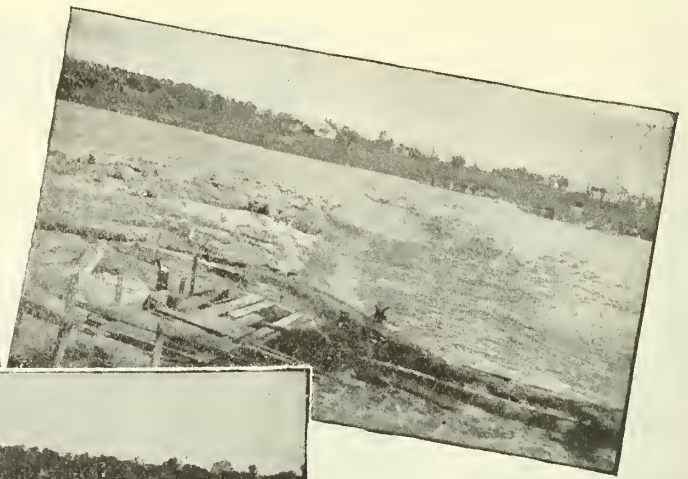
Old Caledonia Dam before Concrete reconstruction commenced.
