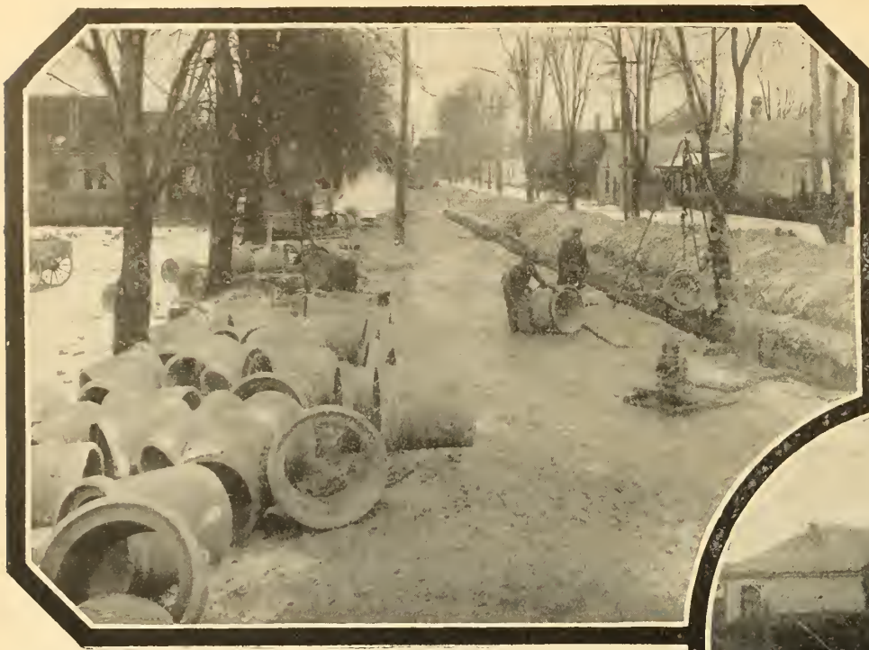
Concrete Sewer London, Ont.
