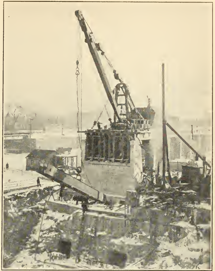
View during erection of Niagara Arch Bridge.
