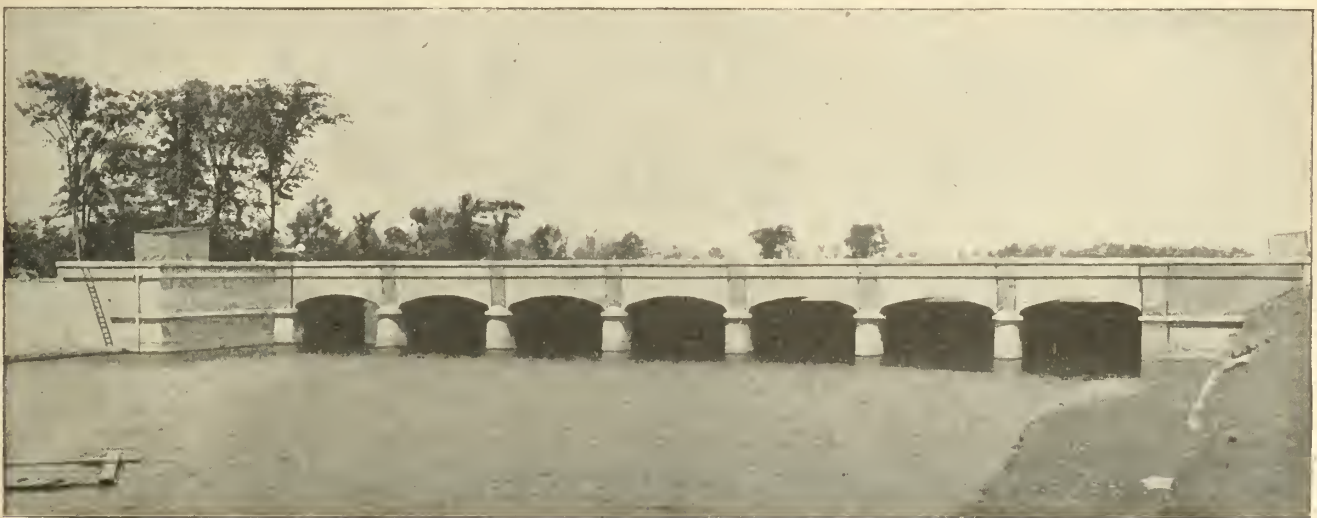
Figure No. 2.—Crawford Bridge and Control Dam dividing Montreal Aqueduct into two sections.
