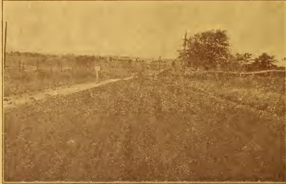
Barrie-Bradford Provincial Highway at Fennell's Corners after using Imperial Gravel Dust Layer on the fine, loose gravel roadway. (In circle) Dust clouds before treatment.
