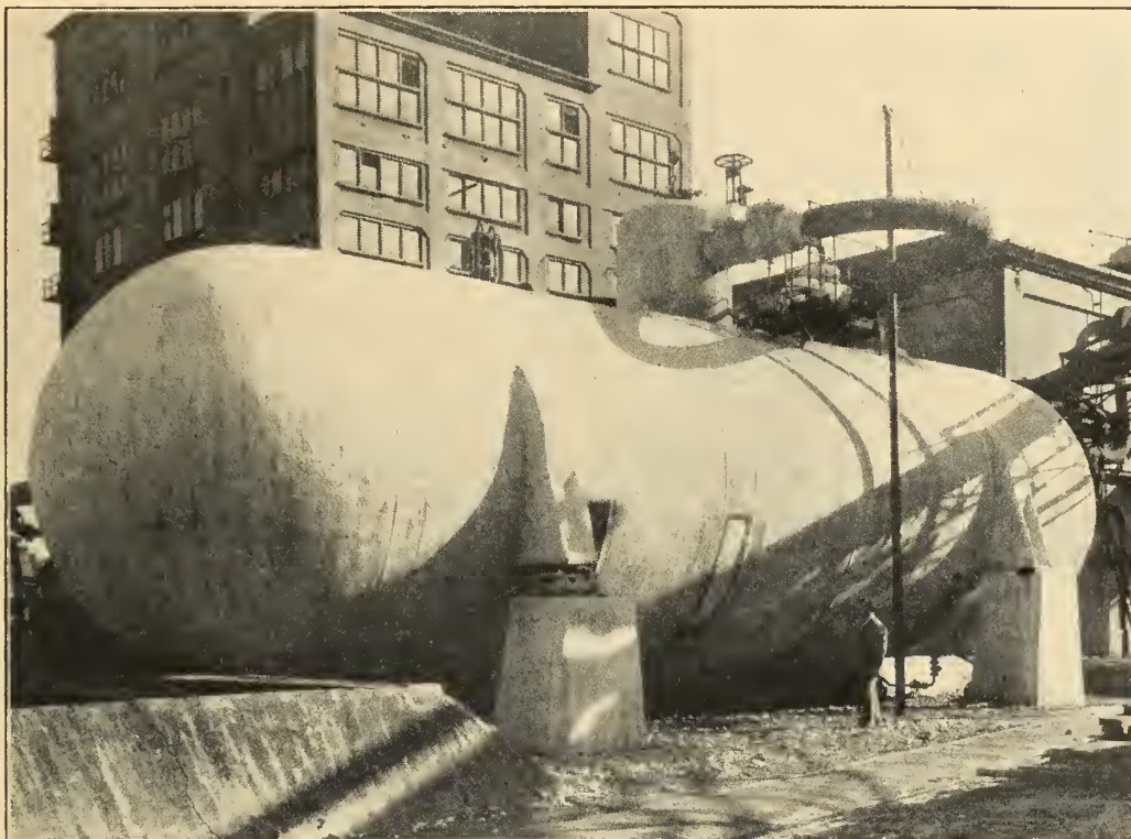
Installation in a Pulp and Paper mill. Accumulator approx. 60 ft. long and 16 ft. in dia. — 11,300 cu. ft. storing 43,000 lbs. of steam. Accumulators have been built large enough to store 80,000 lbs. and small enough to store 180 lbs. of steam.
