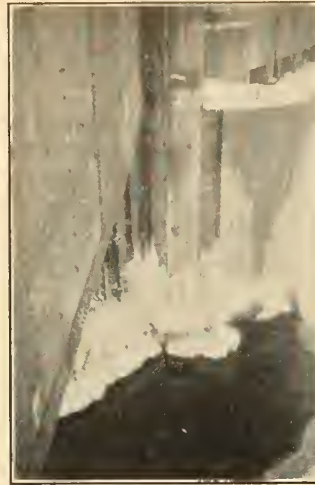
Figure No. 18.—Ice formed on the Roller Path, and Guides under open Sluice Gate.
