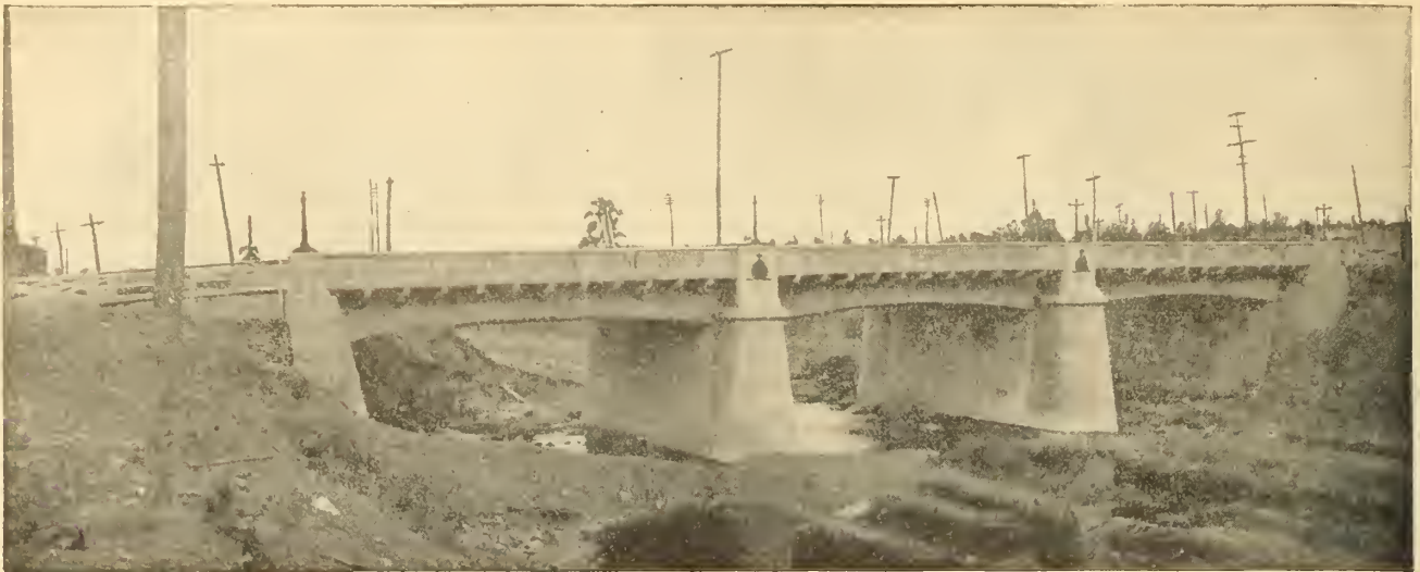
Figure No. 3.—Church Street Bridge over Montreal Aqueduct.
