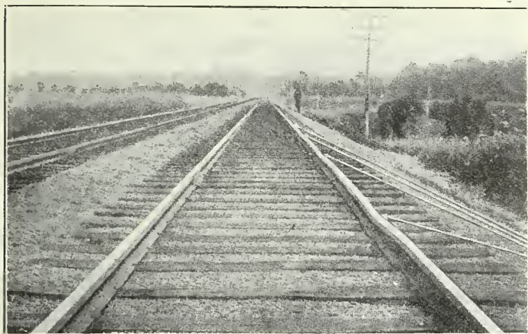
Section of 80-lb. rail bent from the effect of over counter-balance of locomotive at high speed, demonstrating the extreme toughness of the steel.
