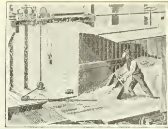
Figure No. 18.—Power operated car shovels.
