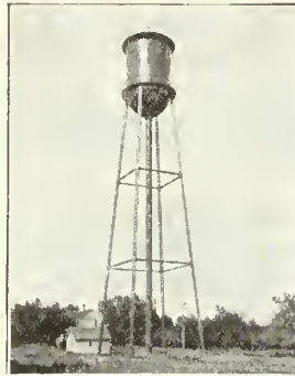
Above is an elevated tank of hemispherical-bottom type, used by municipalities for water supply. At the right is an 80,000 barrel oil tank
