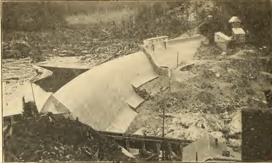
Ocean Falls Dam.
