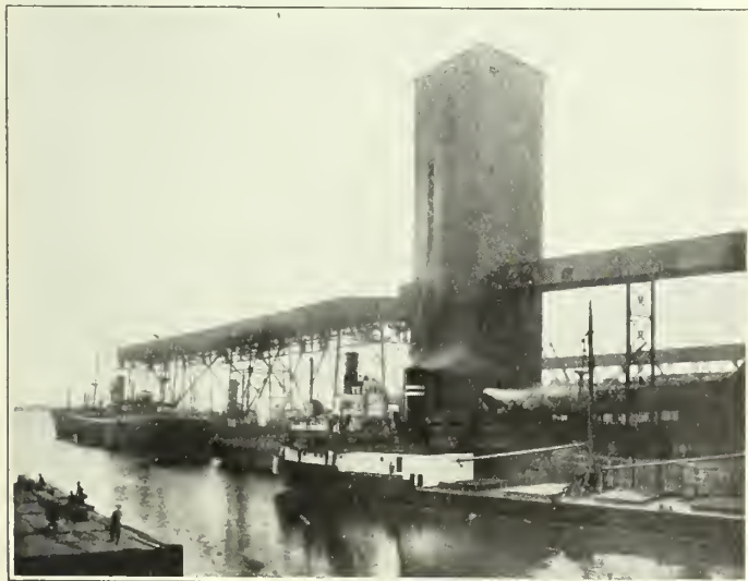
Figure No. 10.—Harbour Commissioners of Montreal, jetty gallery, Elevator No. 2.
