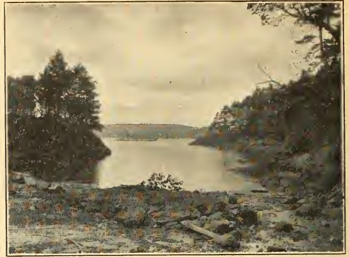
Figure No. 2.—Site of New Esquimalt Drydock at Skinner's Cove before Construction Operations — 1921.
