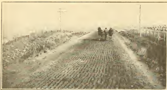
Figure No. 6.—Incorporating Bitumen into Dirt Road Surface.
