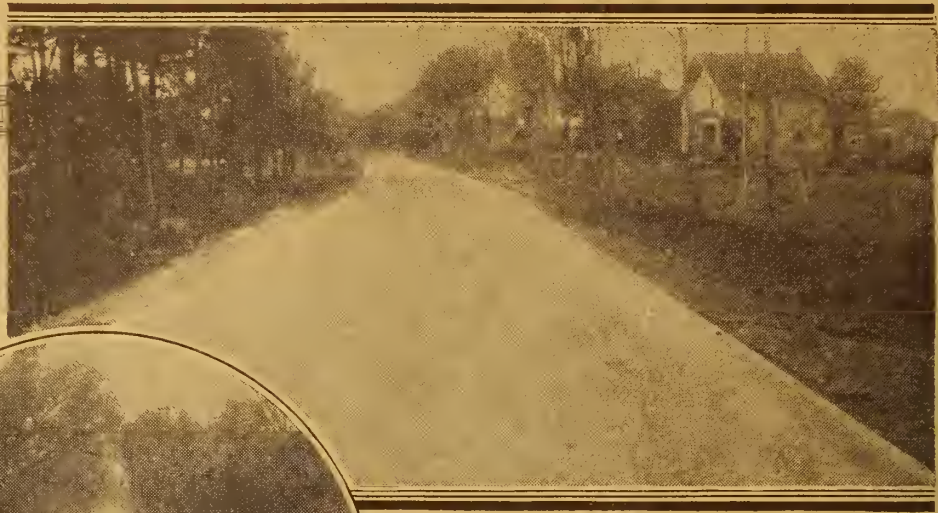
Two views on the Kingston Road Provincial Highway between Oshawa and Bowmanville. Hot-Mix Asphalt laid in 1924 by Johnson Bros. Limited, for the Department of Public Highways of Ontario.
