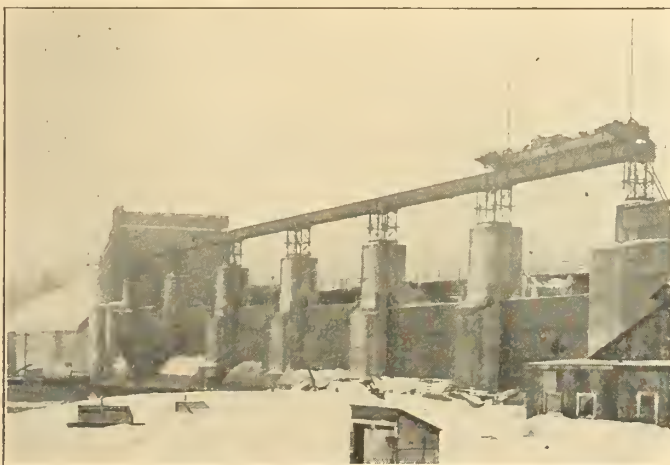
Figure No. 15.—Sluice Gates in Dam with Bridge and Travelling Type of Screw Hoist.
