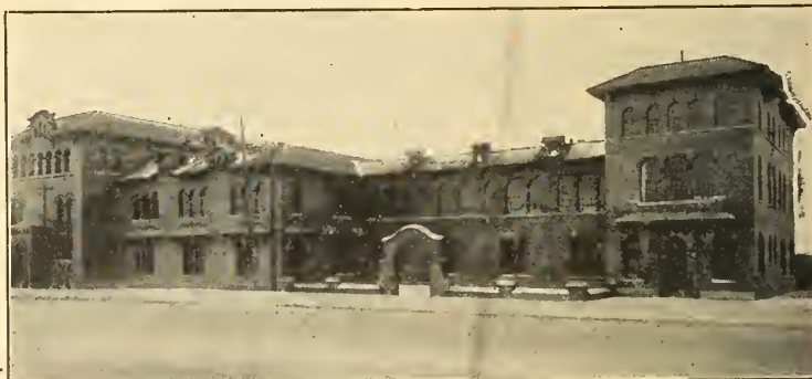
Pumping Station, Montreal Filtration Plant. HARD-N-TYTE used on all concrete floors.
