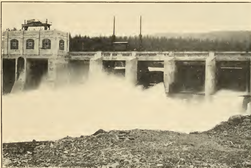
Blind Slough Dam.
