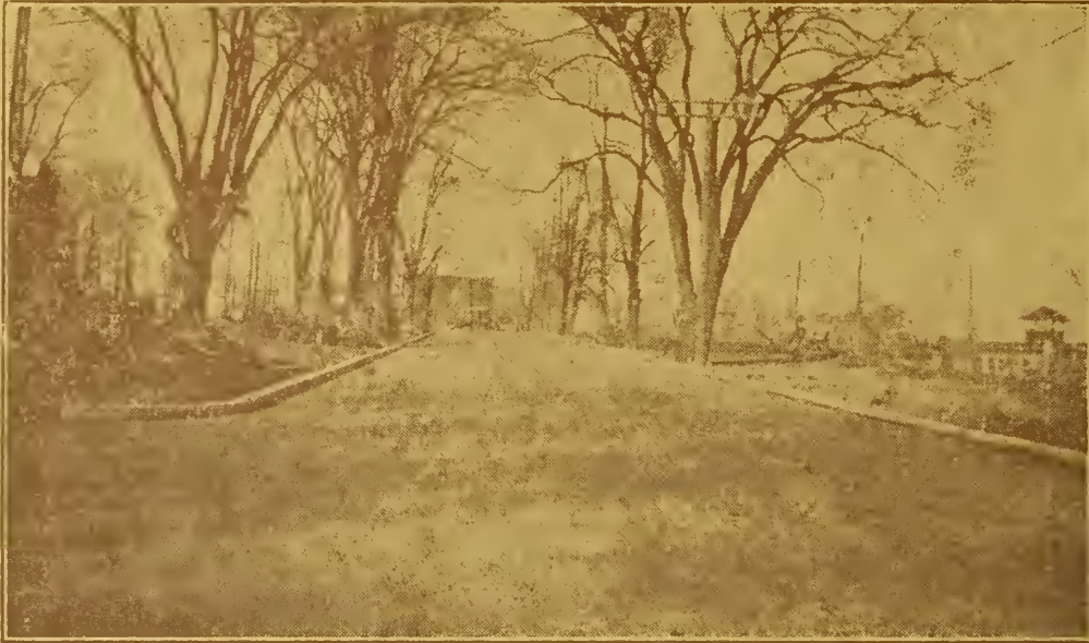
Asphalt pavement (Amiesite) on River Road, Verdun, P. Q.
