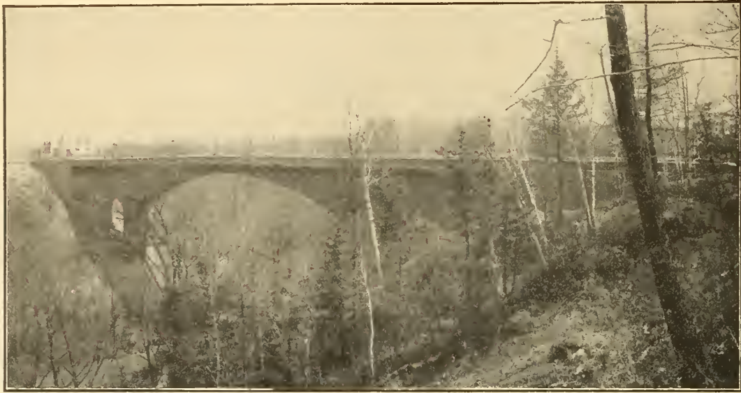
The Governor's Bridge spanning the Belt Line Ravine, Rosedale, Toronto. Centre span, 200 feet. Height above Ravine, 88 feet. Length of bridge structure, 480 feet. Width, 28 feet 4 inches.
