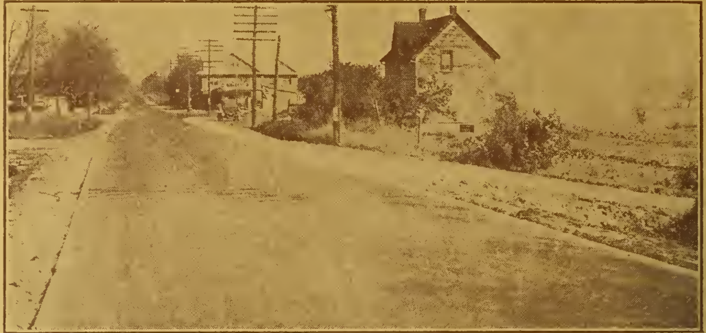
Two views on the Dundas Highway near Islington. Both photographs were taken near the turn leading to the new Bloor St. viaduct over the Humber River.
