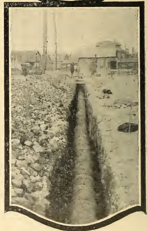
Concrete Sewer Guelph, Ont.
