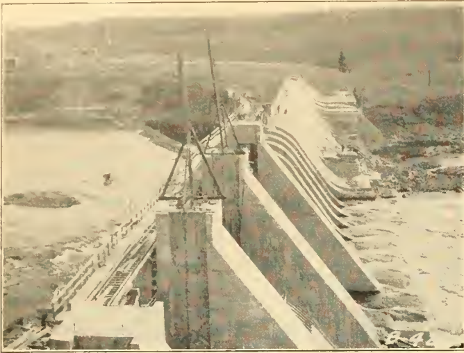
Figure No. 9.—Sluice Gate Piers showing Voids left for Bedded Parts.
