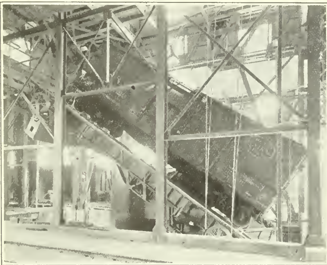
Figure No. 22.—“Metcalf” Car Dumper in operation showing end tilt.
