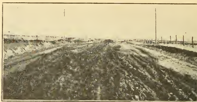
Figure No. 7.—Dirt Road after Heavy Rain — Experimental Strip in Background.
