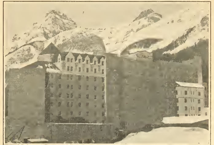
Figure No. 3. — Lake Louise Hotel — Showing Hoarding Partially Removed.
