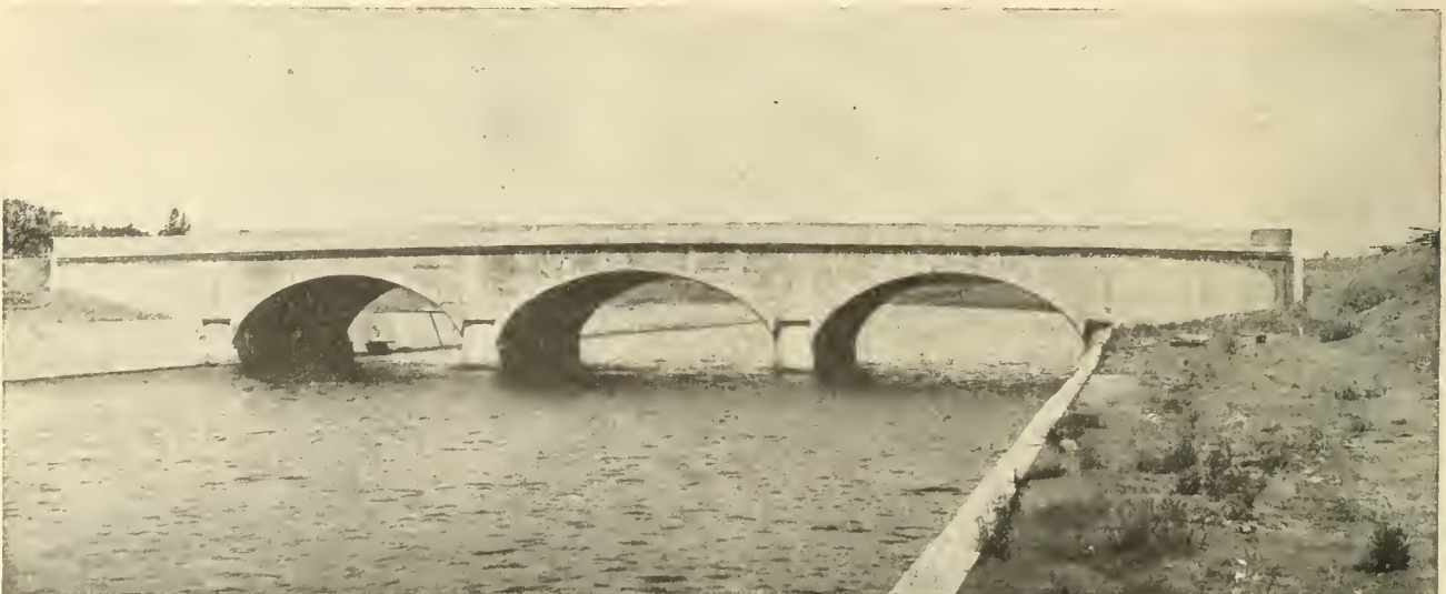
Figure No. 1.—Latour Bridge over Montreal Aqueduct.
