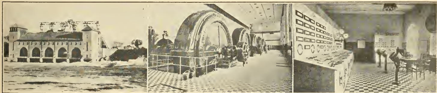
Exterior View of Power House.
