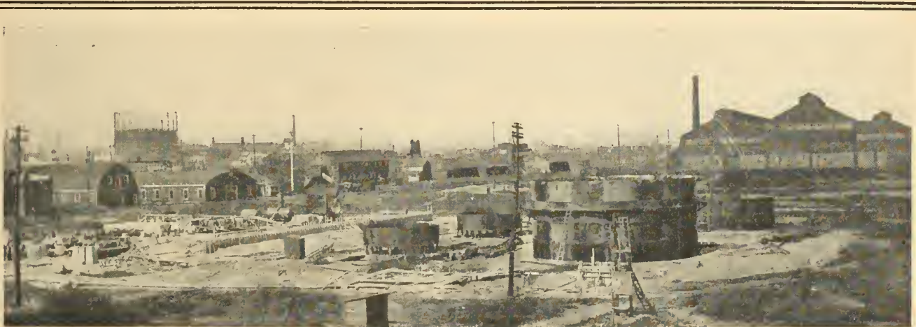
At McColl Bros. New Refinery
