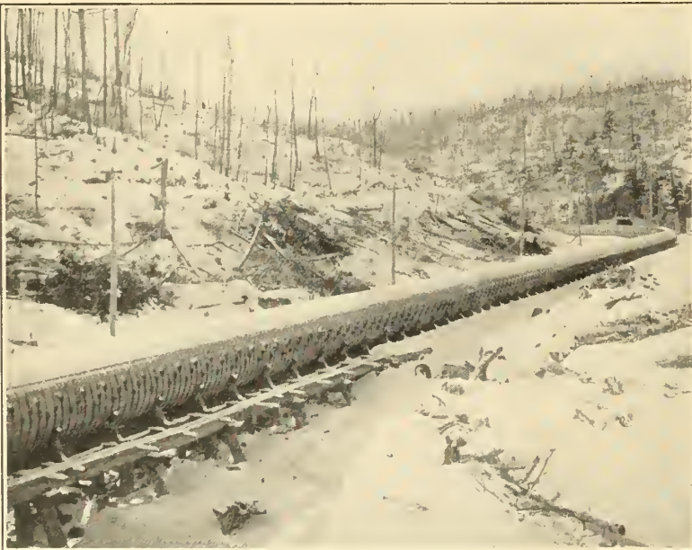
AVON RIVER PIPE LINE
