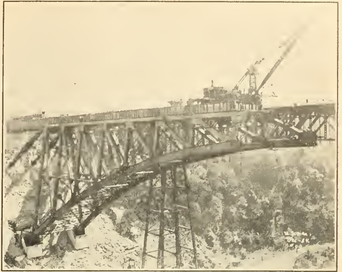
Erection of New Niagara Arch Bridge.
