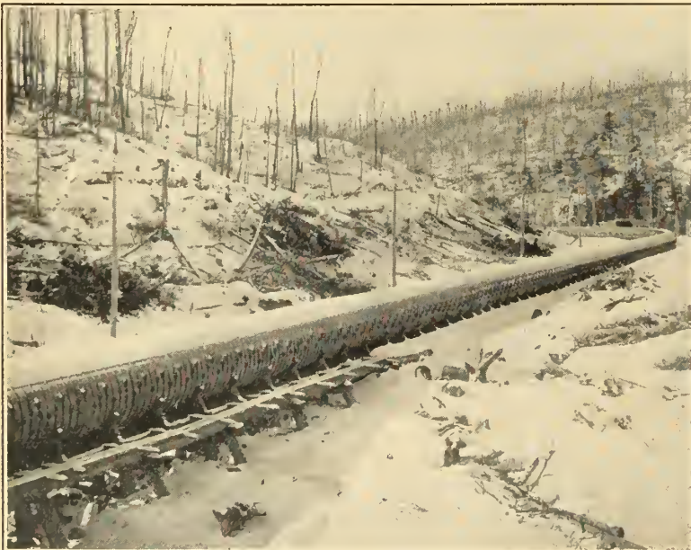
AVON RIVER PIPE LINE
