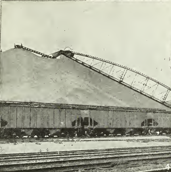
4—Showing how a single Barber-Greene Conveyor has enabled the D. L. & W. Coal Co. to increase their storage 75,000 tons. It will handle at least 25 cars a day.
