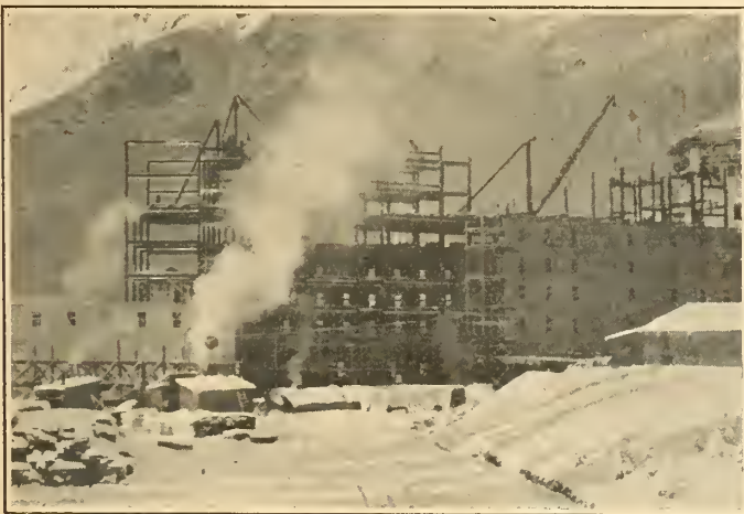
Figure No. 2. — Lake Louise Hotel — Erection of Steel Work and Hoarding.
