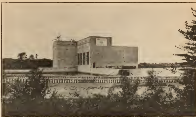
Drummondville Development on the St. François River, Quebec, of the Southern Canada Power Company — 7,500 h.p.
