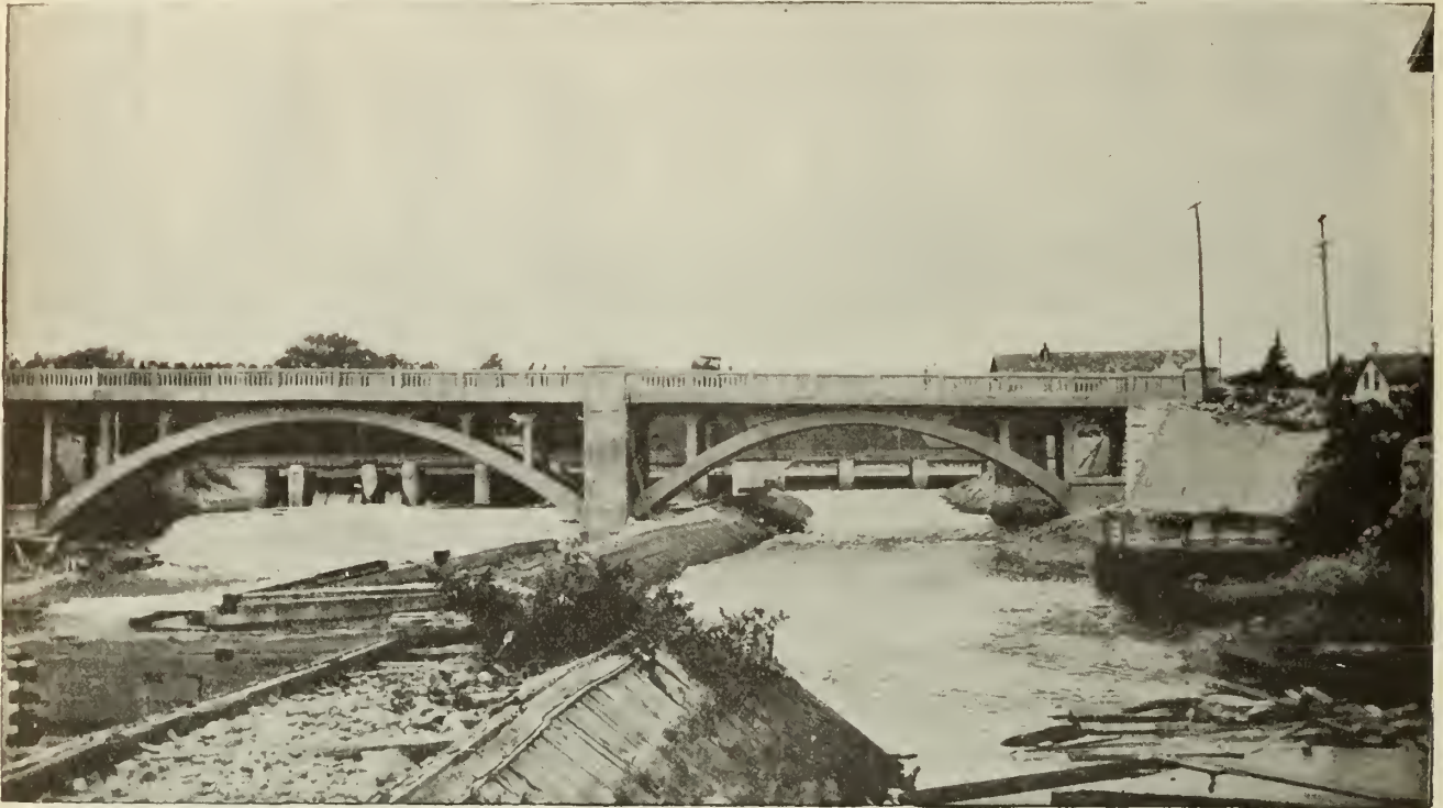
Attractive new concrete bridge spanning the Otonabee River at Lakefield, Ont. This bridge was built in two sections supported by two shore piers and a pier at the center of the river. The deck is of concrete beam and slab construction. One unusual feature of the Lakefield Bridge is that it forms part of a hill and is built at a grade, the west end being considerably higher than the east end.
