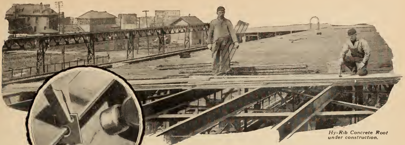
Method of attaching Hy-Rib to structural steel by means of Truscon Plate Clip.
