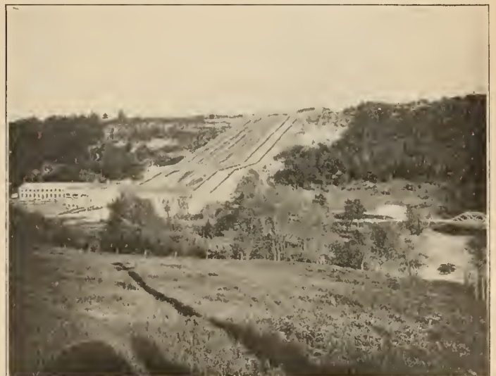
De Cew Falls Development on a diversion from the Welland Canal, of the Dominion Power Transmission Company — 45,000 h.p.
