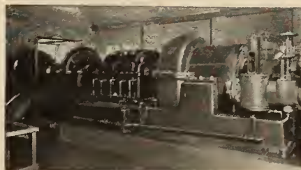
Geared Turbine Driven Centrifugal Pump 30,000,000 gal. per day, 225 ft. head
