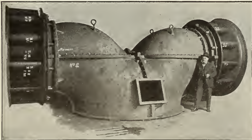
56" Type F Turbine, Centre Discharge
