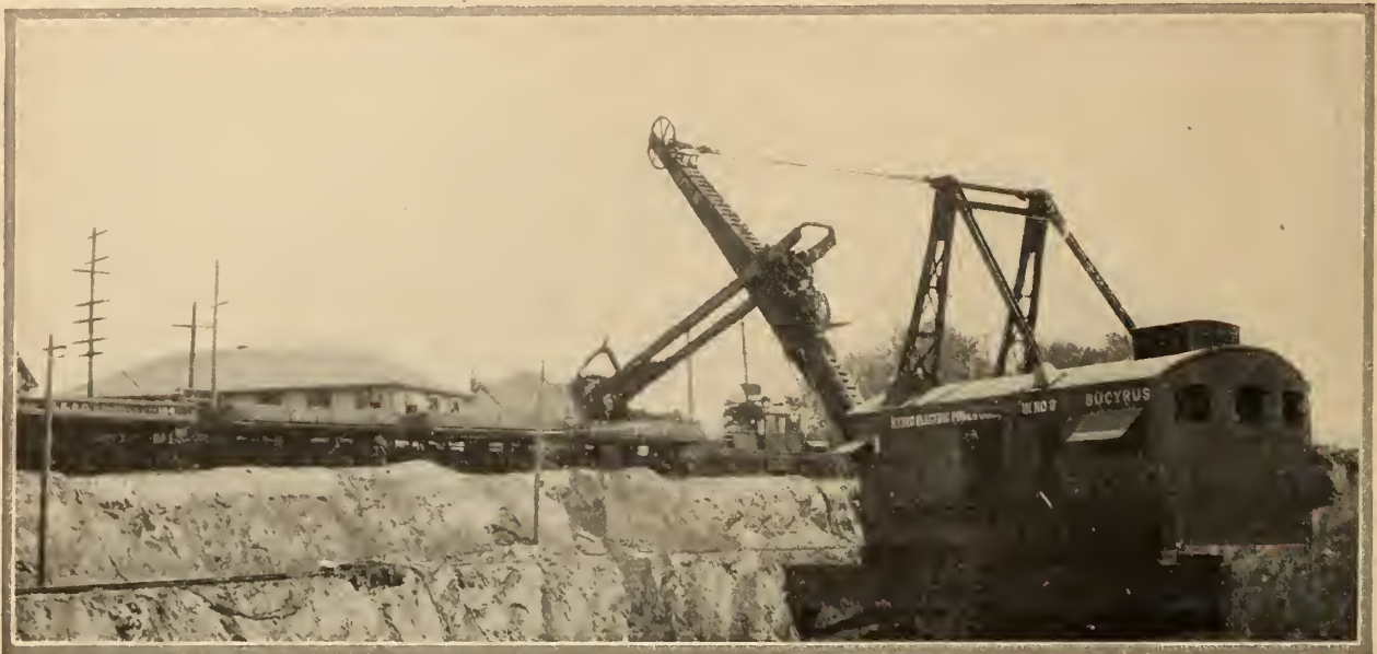
The Electric shovel loading Western automatic air dump cars, Niagara Falls, Ontario.
