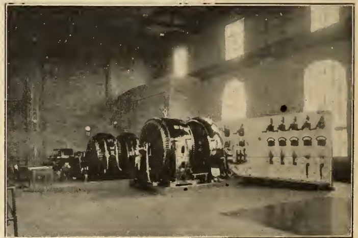
Plate No. 13, — Interior View of Modern Substation — Montreal.
