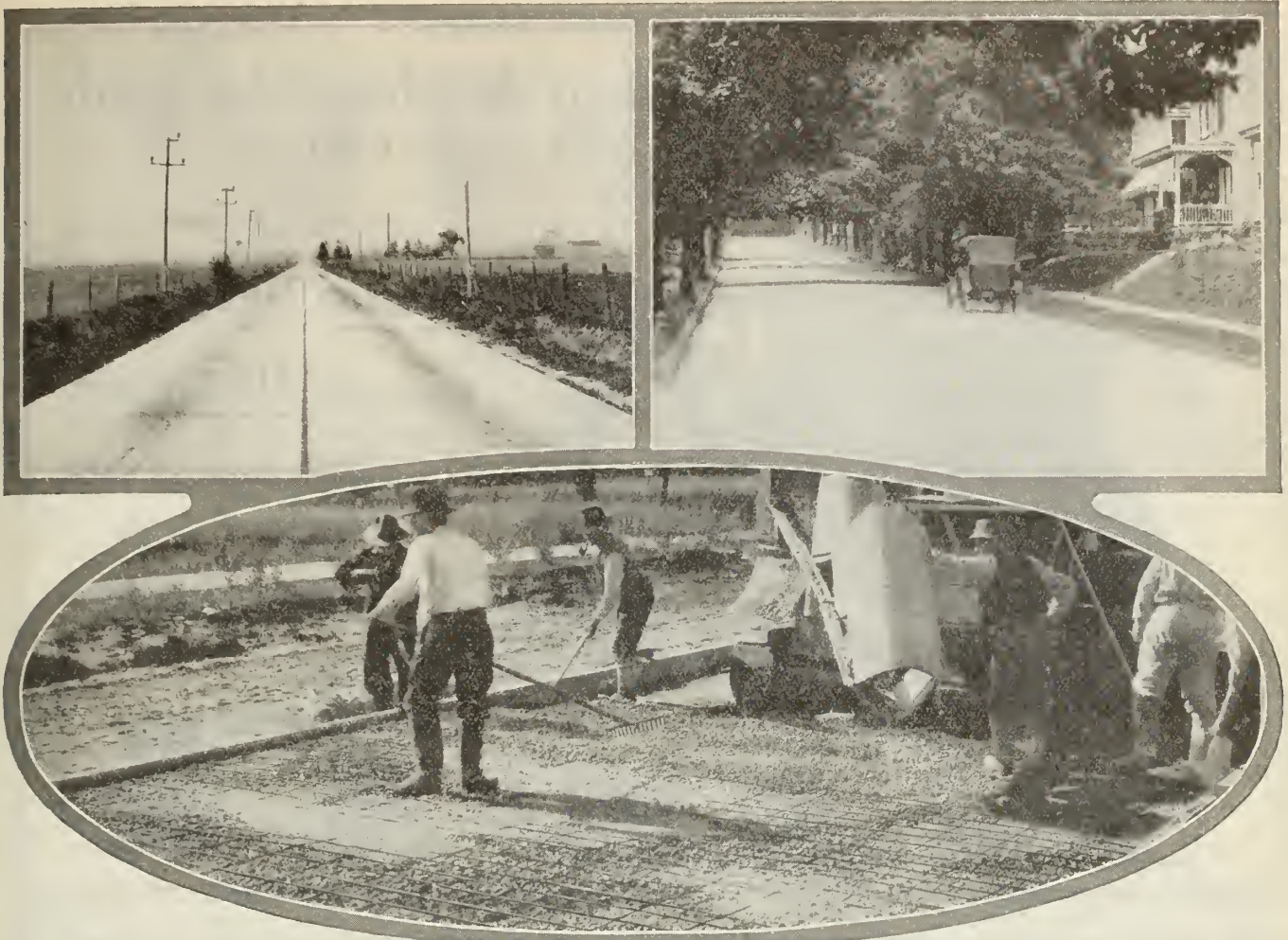
Upper left—Highway showing use of Truscon Dowel Contraction Joints and Wire Mesh. Upper right—Street view in residential section showing reinforced concrete road. Lower—Truscon Wire Mesh is the ideal reinforcement for concrete roads.
