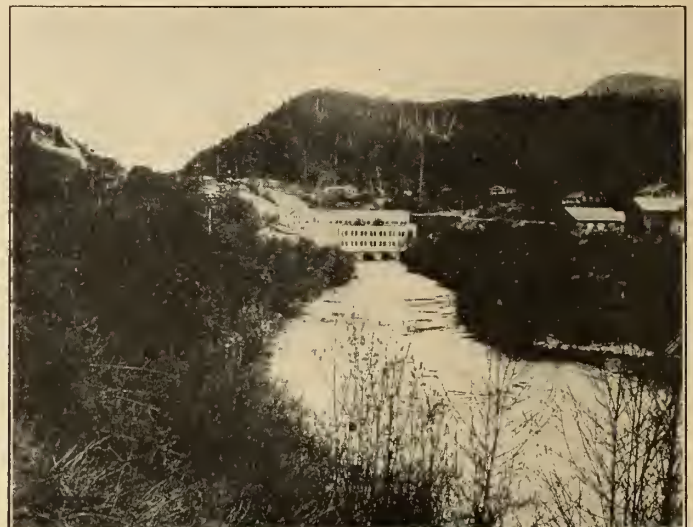
Stave Falls Development on the Stave River, of the British Columbia Electric Railway Company — 52,000 h.p.
