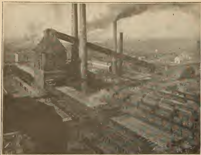
A section of Besco Coke Oven By-Product Plant
