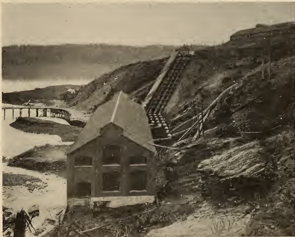
Plate No. 1.—Hydro-Electric Development of Granby Consolidated Mining, Smelting and Power Company at Anyox, British Columbia, 13,400 horse power.
