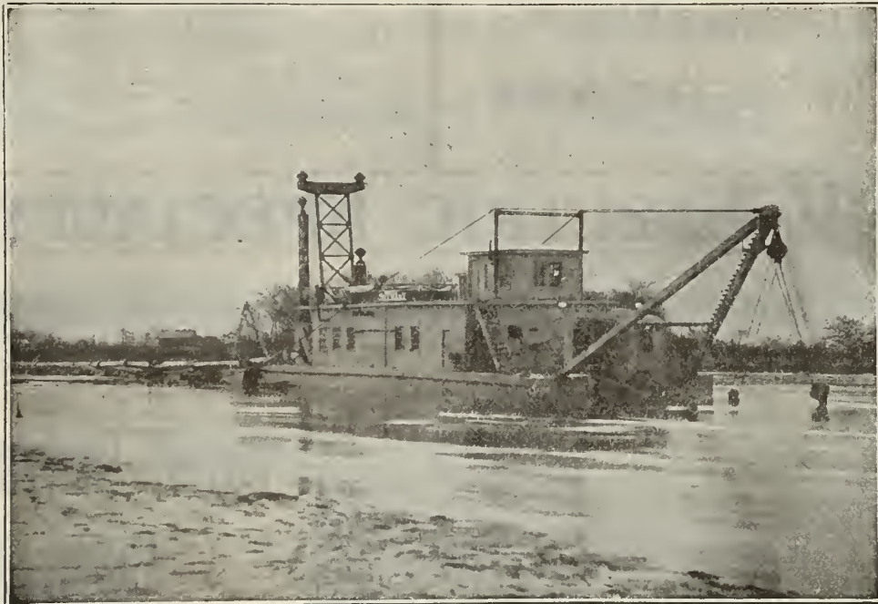
Electric Dredge on Queenston-Chippawa Power Development
