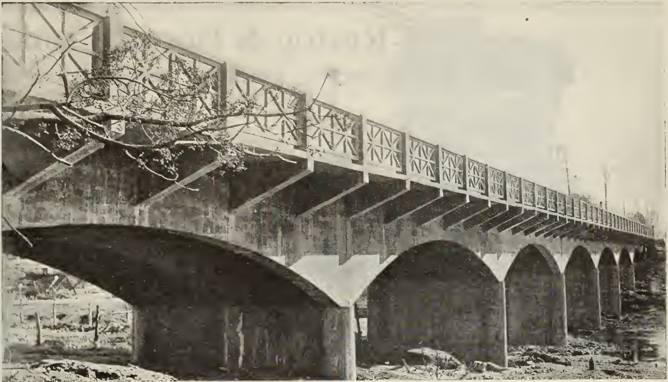
Reinforced Concrete Viaduct 385 ft. long Truscon Reinforcing Steel used throughout.
