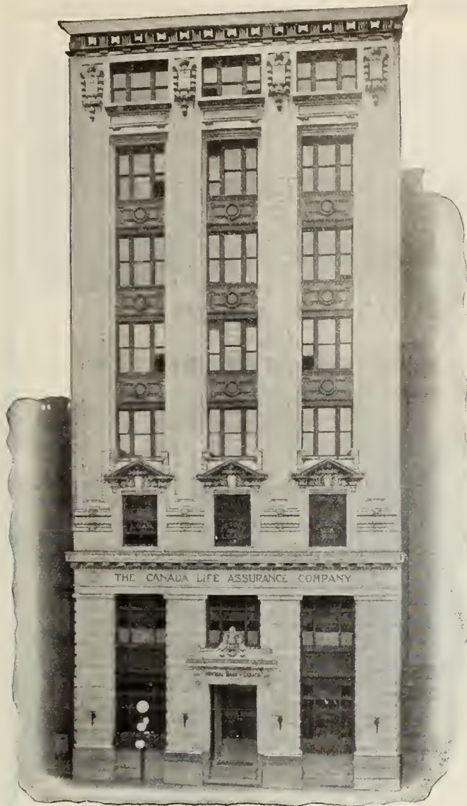
THE CANADA LIFE ASSURANCE BLDG. VANCOUVER.
