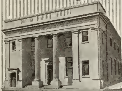
Barrett Specification 20-Year Bonded Roof on Merchants' Bank of Canada. Arch.: H. R. Little, Montreal, Que. Con't: Carter, Halls, Aldinger, Regina. Roofer: Hastings & Willoughby, Regina.
