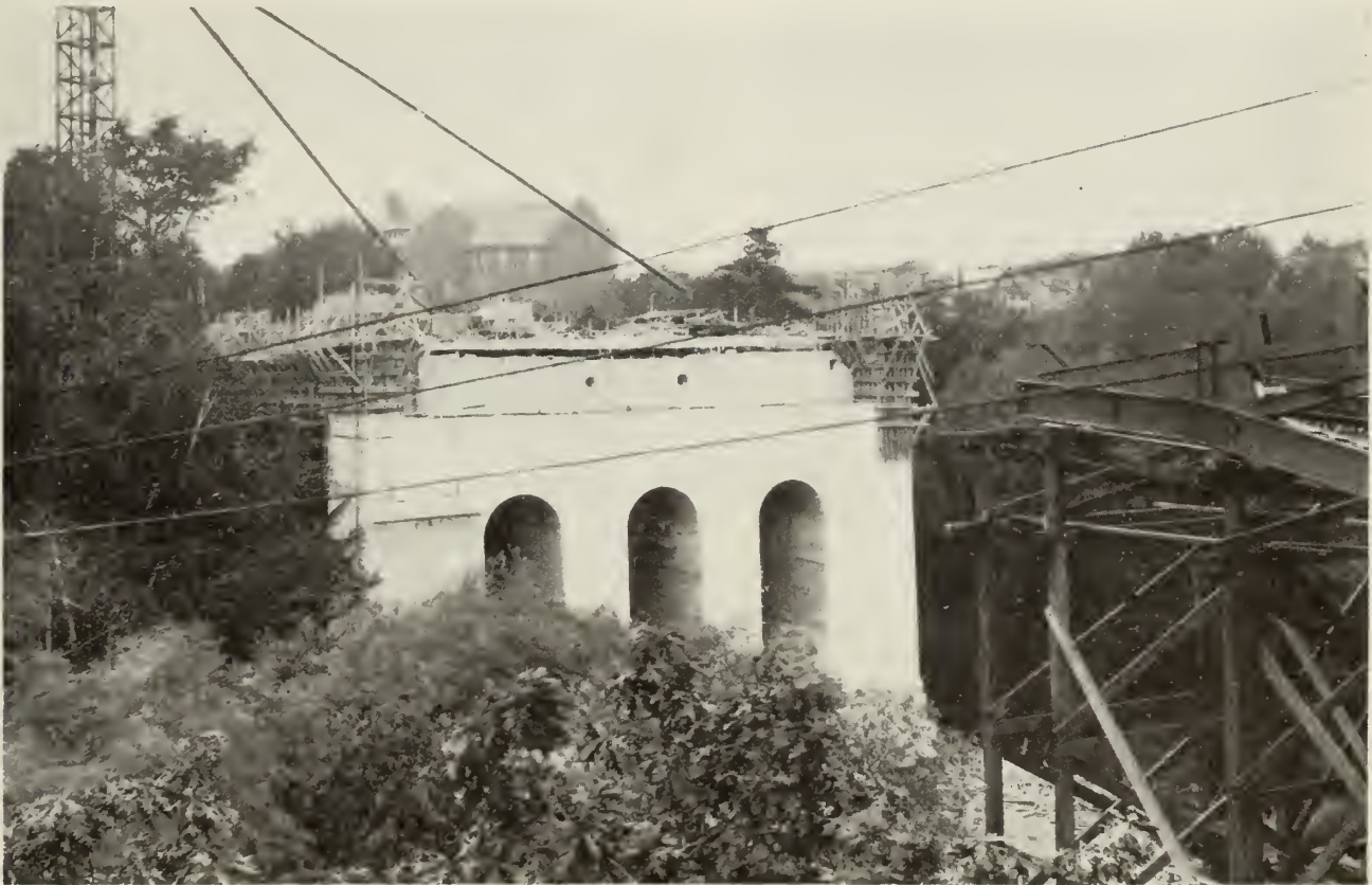
New St. Clair Avenue Bridge over Ravine, Toronto, Ont.
