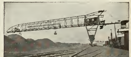
COAL HANDLING BRIDGE
