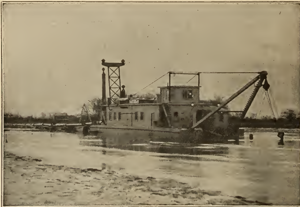
Electric Dredge on Queenston-Chippawa Power Development
