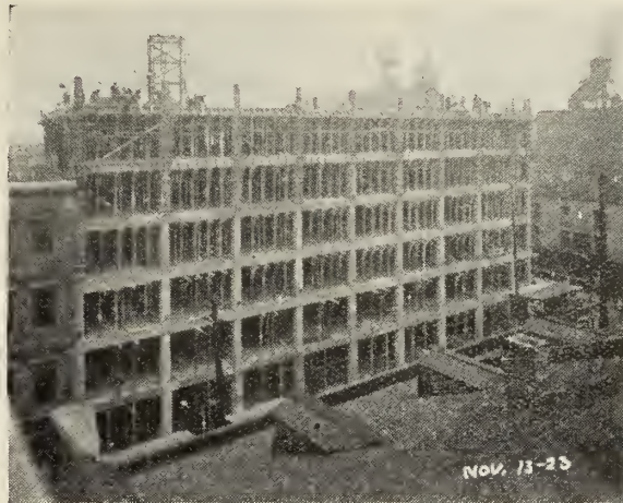
Lister Building 138 ft. x 100 ft., Six Storeys, Hamilton, Ont.
