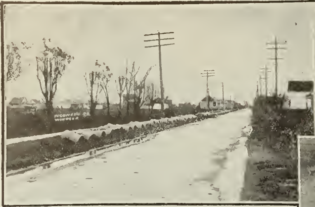
The upper illustration shows Concrete Pipe for a combined Sewer at Windsor, Ont., the lower shows a 12" sanitary sewer being laid with Concrete Pipe at Guelph, Ont.
