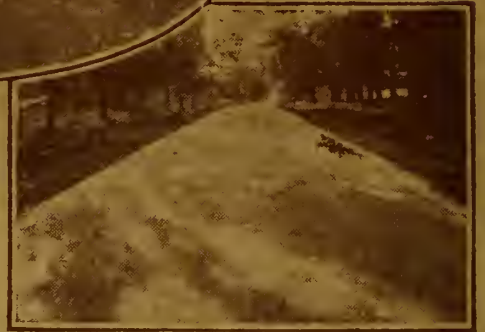
Left — A fine stretch of highway. Top — Showing the "Black Base" foundation. Right — Near Allanburg.
