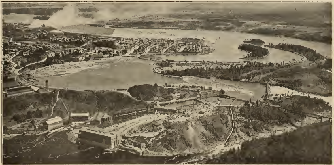
Shawinigan Falls Development on the St. Maurice River, Quebec, of the Shawinigan Water & Power Company — 191,500 h.p.
