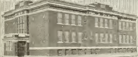
Barrett Specification 20-Year Bonded Roof on Kitchener School. Arch.: J. H. Puntin. Con't: Wilson & Wilson. Roofer: Hastings & Willoughby. All of Regina.
