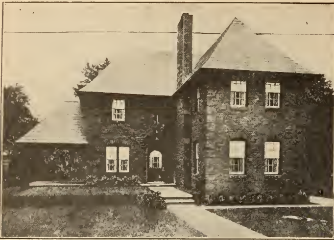
Plate No. 5. — Two Storey Residence Electrically Lighted and Equipped for Electric Service.
