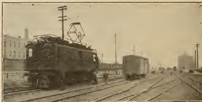
Plate No. 1,—Montreal Harbour Electrification, Catenary 2,400-V., D.C.
