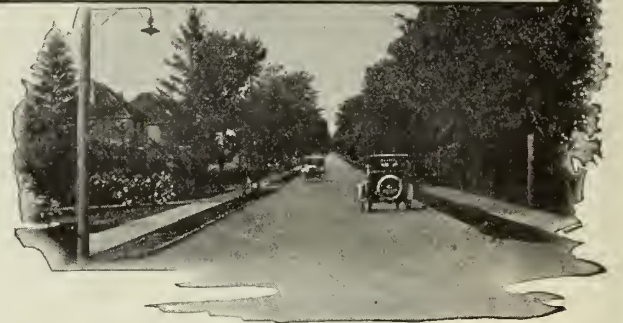
Avondale Avenue, Stratford, Ont. Tarvia-built 1919. Modern, firm, smooth, frost- and thaw-proof pavement.
