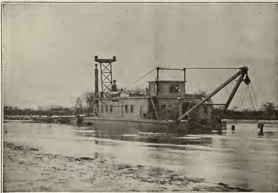
Electric Dredge on Queenston-Chippawa Power Development
