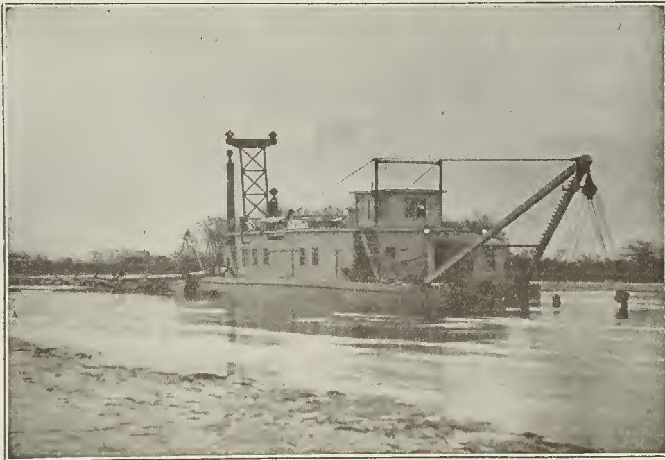
Electric Dredge on Queenston-Chippawa Power Development
