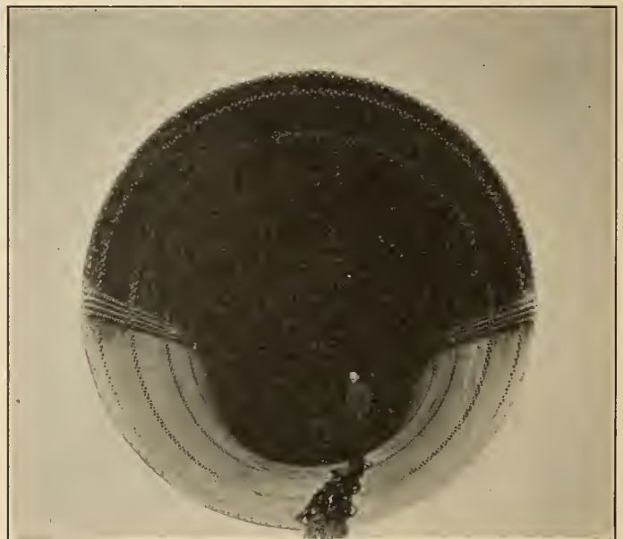
Plate No. C-25.—Penstock with Welded Joints.
