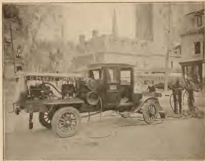
Plate No. 3,—Portable Compressor operating Paving Breaker.
