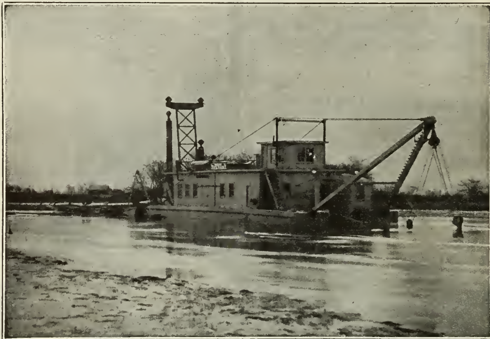
Electric Dredge on Queenston-Chippawa Power Development
