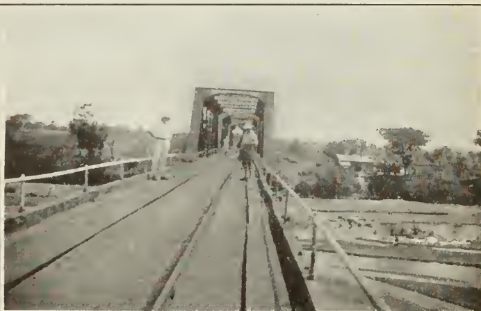
Kaduna Bridge on Main Line Lagos to Kano, March 1924.
