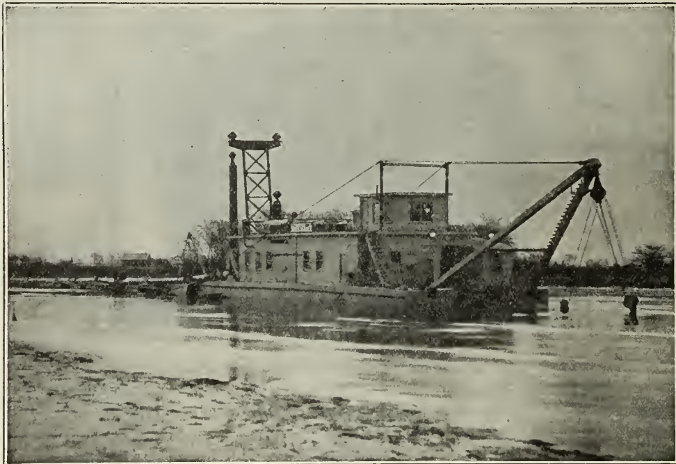
Electric Dredge on Queenston-Chippawa Power Development
