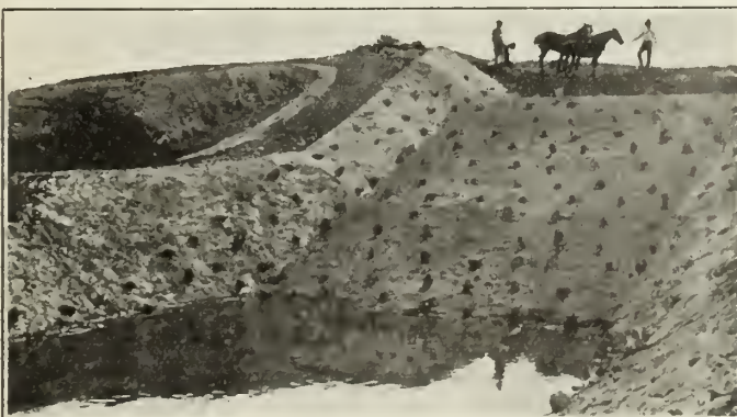
Fig. No. 5. Rock Drop 7A, Secondary A Canal near Strathmore, Alta.
