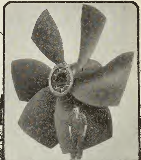
PROPELLOR TYPE RUNNER THROAT DIAMETER 15ft 9 1/2 in
