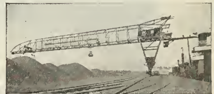
COAL HANDLING BRIDGE
