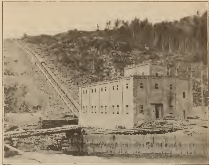
Plate No. 6.—Hydro-Electric Development of the Northern Ontario Light and Power Company, Limited, on the Matabitchouan River, Ontario, supplying power to the Cobalt Silver Mines, 11,000 horse power.
