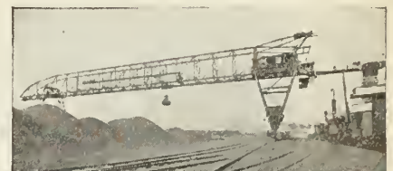
COAL HANDLING BRIDGE
