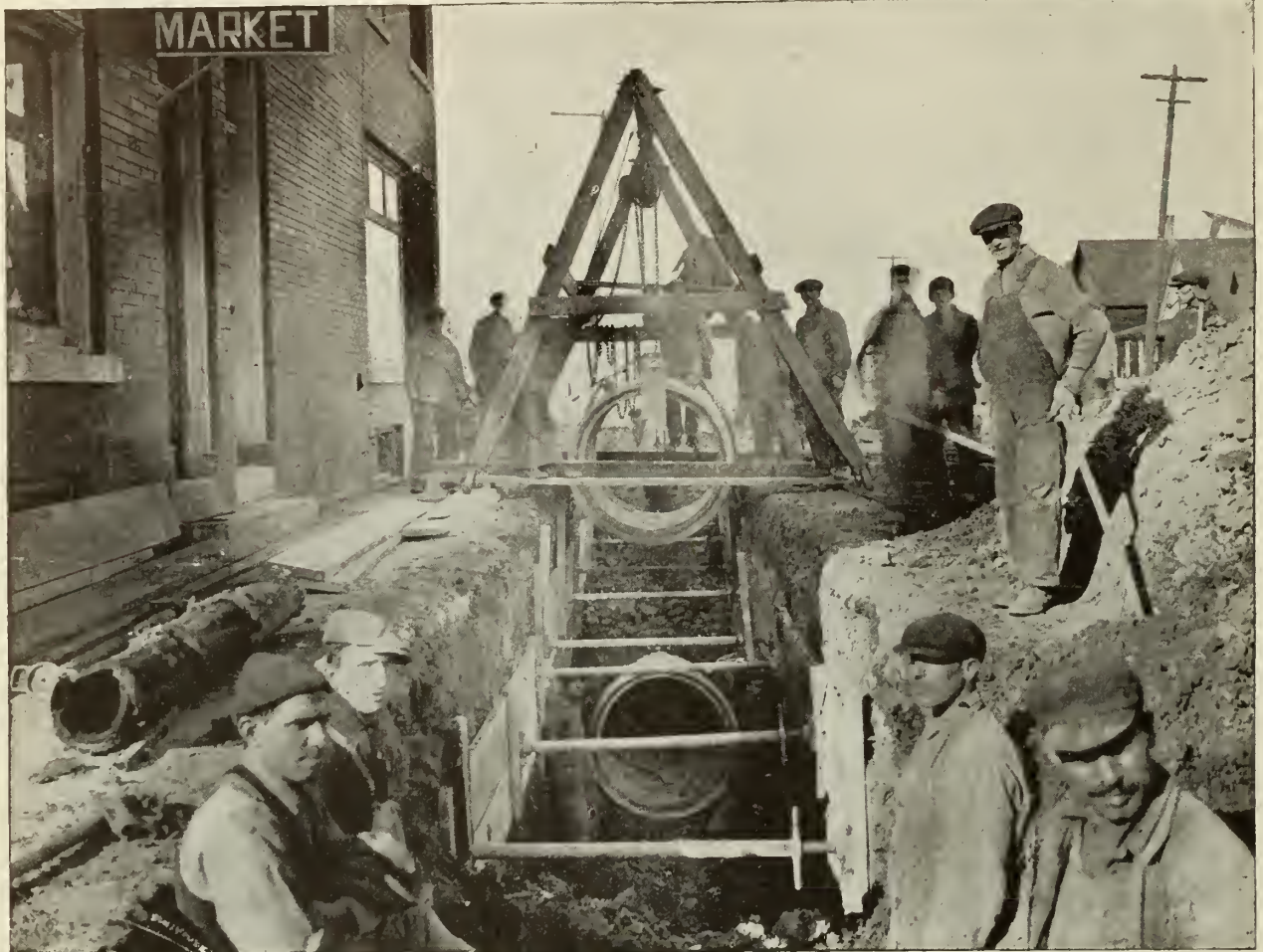
Laying Concrete Lock Joint Sewer Pipe, Ford, Ont.
