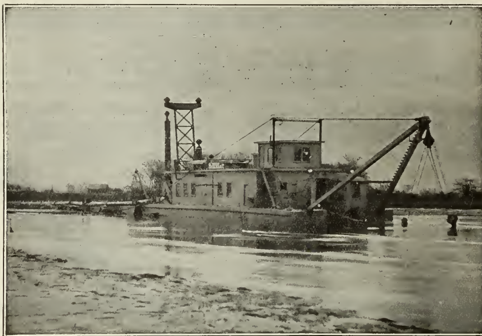
Electric Dredge on Queenston-Chippawa Power Development
