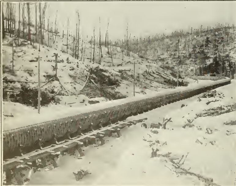
AVON RIVER PIPE LINE
