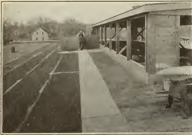
Figure No. 3.—Using 10,680 sq. ft. of Celotex for Roof Insulation.
