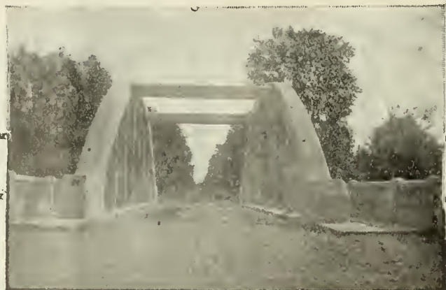
End view of Concrete Bridge at Cronsberry
