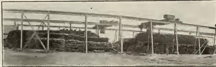
Thousands of tons of Rails awaiting their turn to be reborn to new usefulness through the heating furnace and mill.
