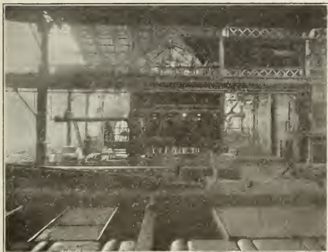
Figure No. 6.—Discharging end of Bloom Re-heating Furnace for Rail Mill.
