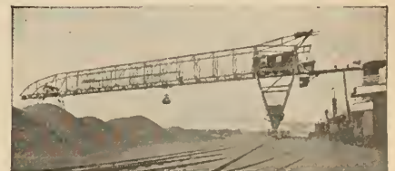
COAL HANDLING BRIDGE
