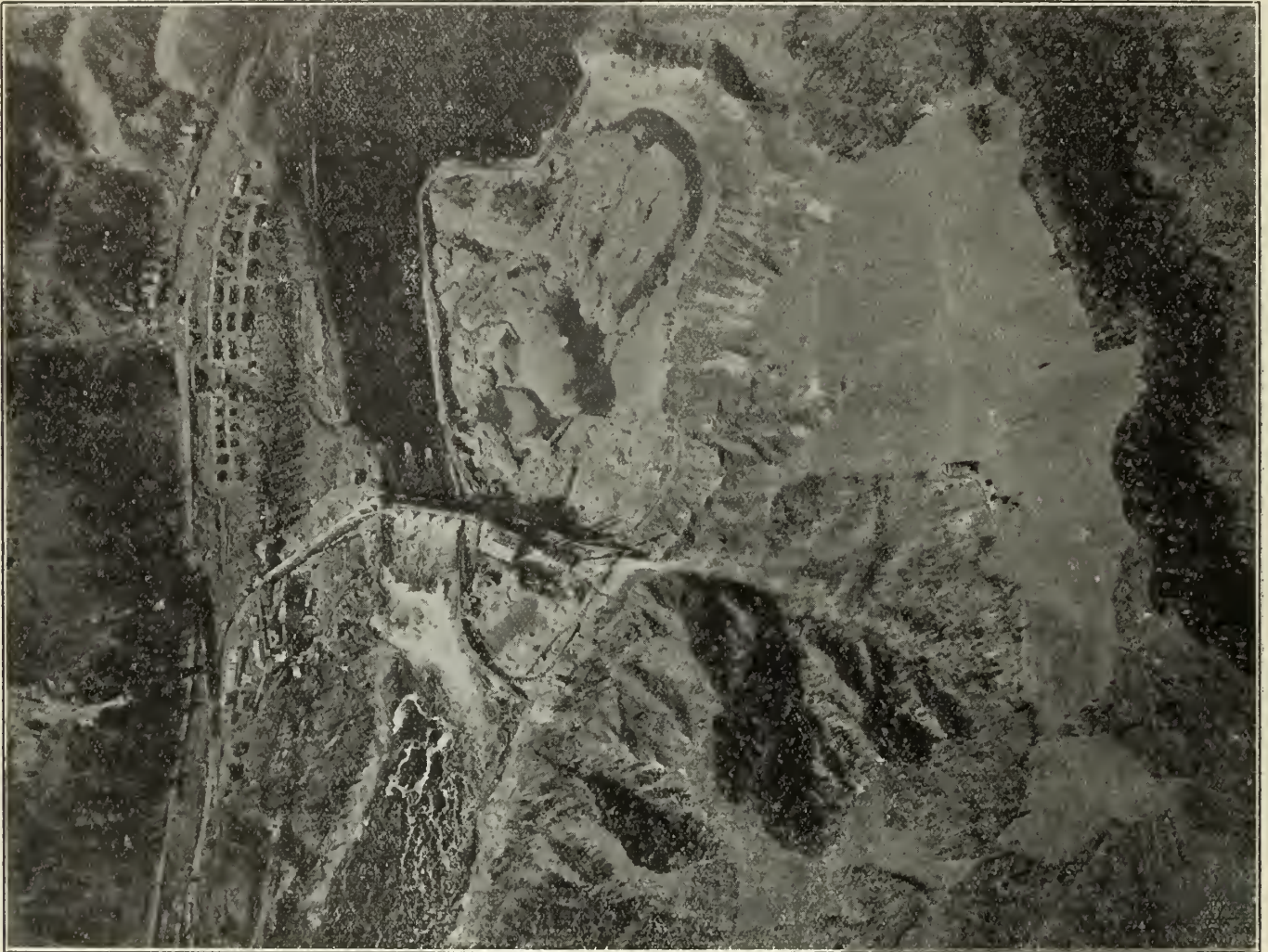
Fig. No. 3. Aerial photograph of LaGabelle, St. Maurice River. Progress of St. Maurice Power Company's development; dam, power house, coffer dam and temporary village.
