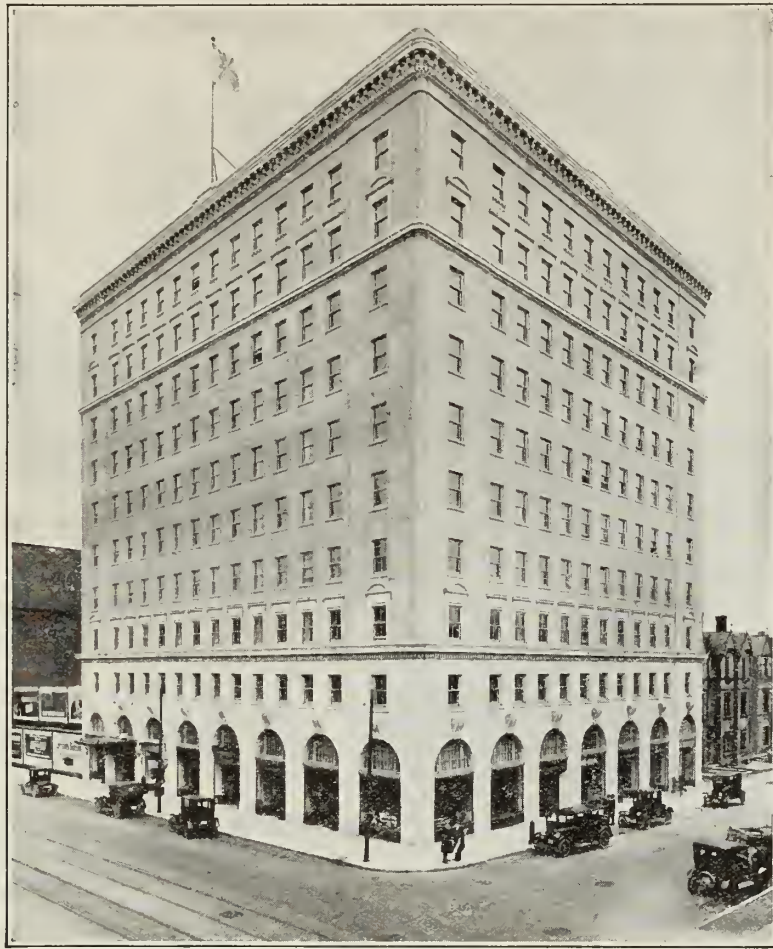
THE KEEFER BUILDING, MONTREAL
