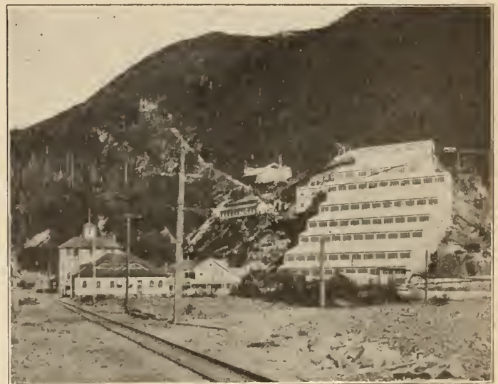
Plate No. 3.—Hydro-Electric Power Station and Concentrating Mill of Britannia Mining and Smelting Company, Limited, Britannia Beach, British Columbia, 15,000 horse power.
