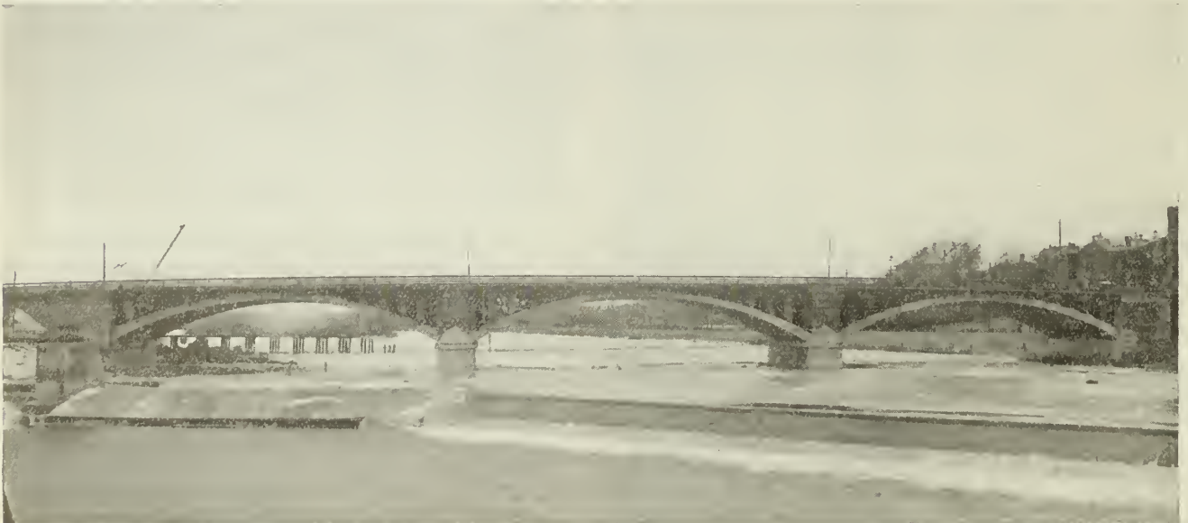
Lorne Bridge, Brantford, Ont., as it appeared on January 12th, 1924.
