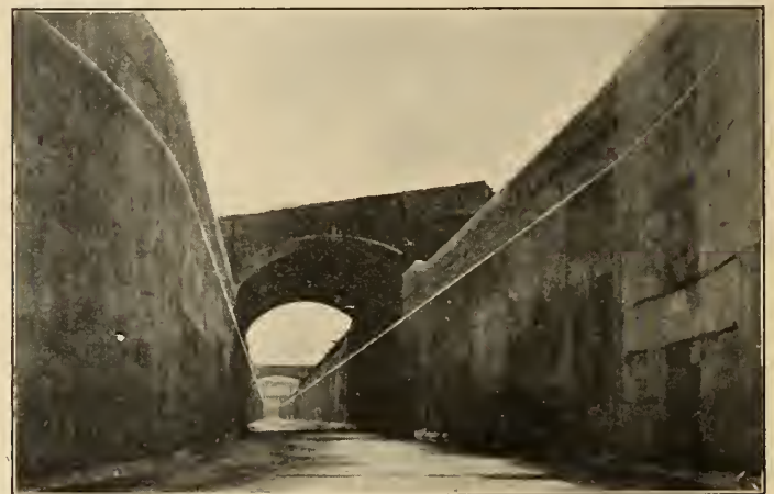
Plate No. C-8.—Concrete-lined Power Canal. Mean Water indicated by White Line.
