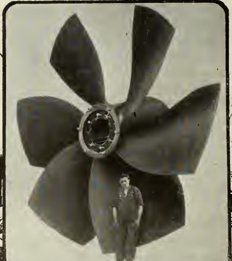
PROPELLOR TYPE RUNNER THROAT DIAMETER 15Ft 9 1/2 IN
