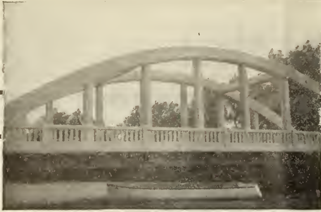
Side view of Concrete Bridge at Cronsberry
