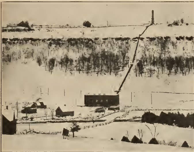
Eugenia Falls Development on the Beaver River, Ontario, of the Hydro-Electric Power Commission of Ontario, 8,500 h.p.
