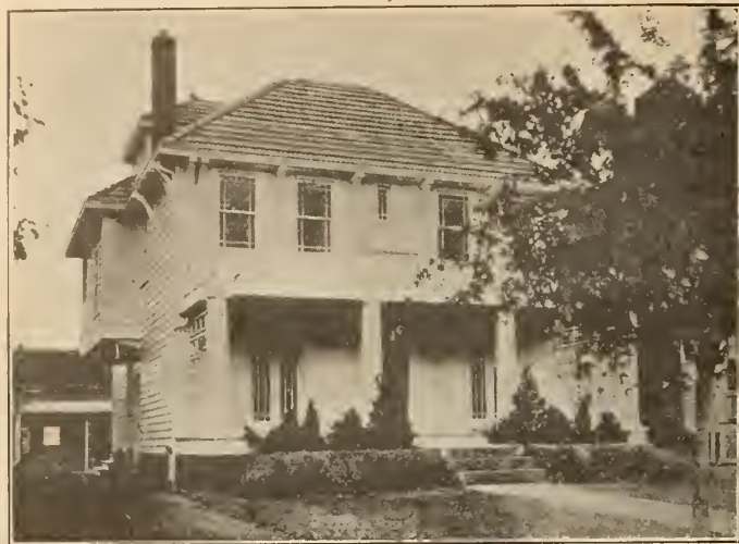
Plate No. 1.—Two Storey Residence Electrically Lighted and equipped for Electric Service.
