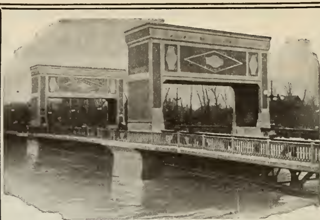
STRAUSS VERTICAL OVERHEAD COUNTERWEIGHT BASCULE. COUNTERWEIGHTS CONCEALED OSBORNE ST. BRIDGE, WINNIPEG.
