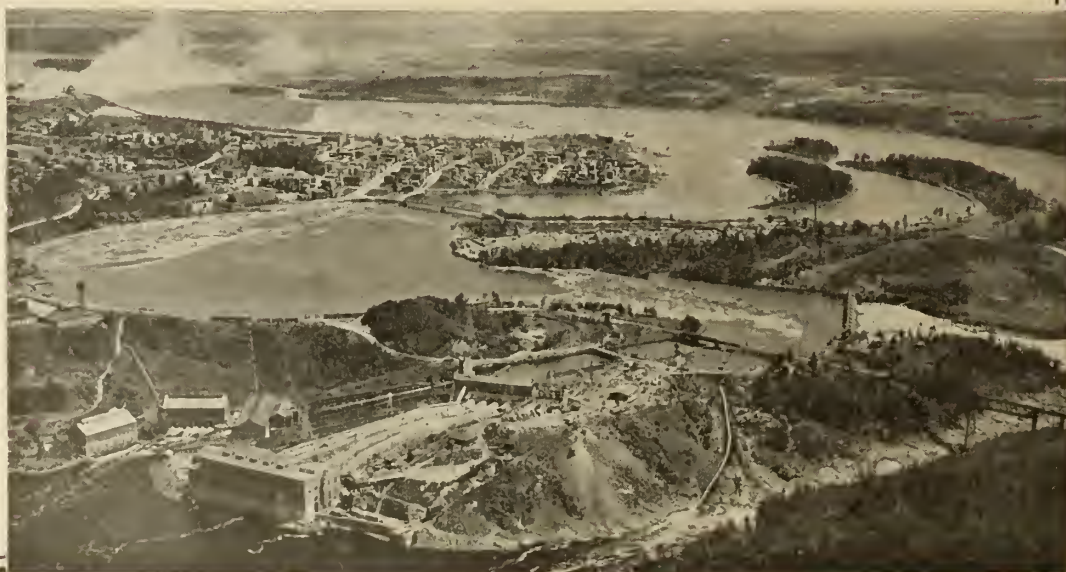
Aeroplane view of Power Plants at Shawinigan Falls, Que.
