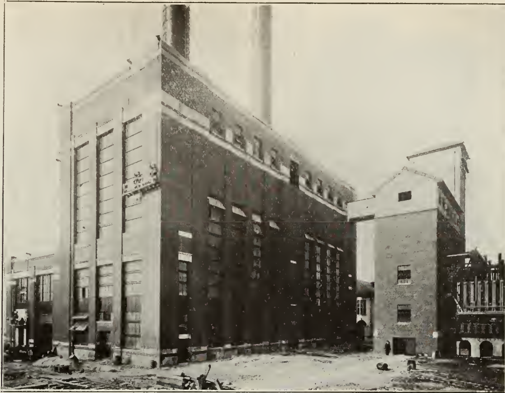
Ford Power House, Ford, Ontario. Truscon Steel Windows used throughout.
