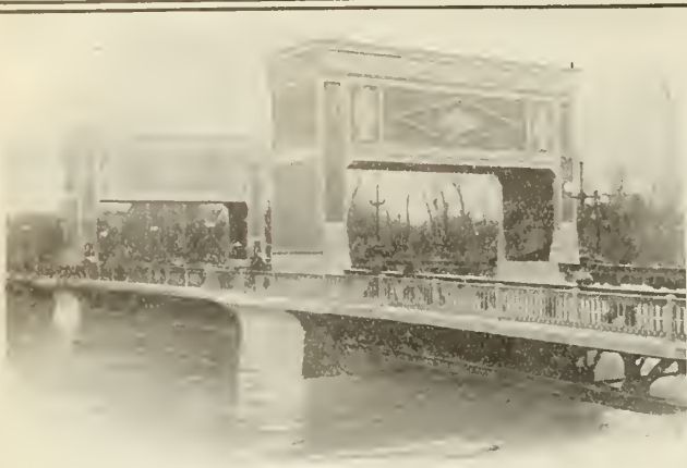
STRAUSS VERTICAL OVERHEAD COUNTERWEIGHT BASCULE. COUNTERWEIGHTS CONCEALED OSBORNE ST. BRIDGE, WINNIPEG.
