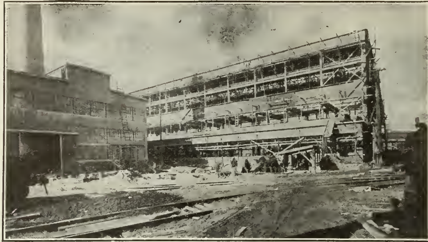
Work done and photograph furnished by Traylor-Dewey Contracting Co., Allentown, Pa.
