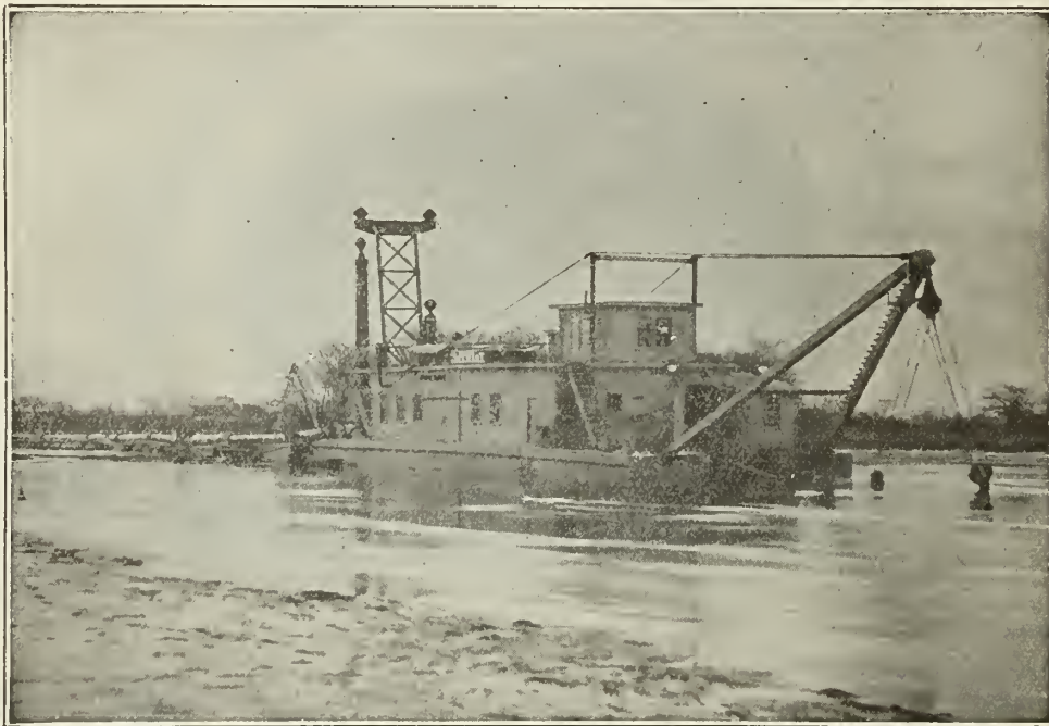
Electric Dredge on Queenston-Chippawa Power Development
