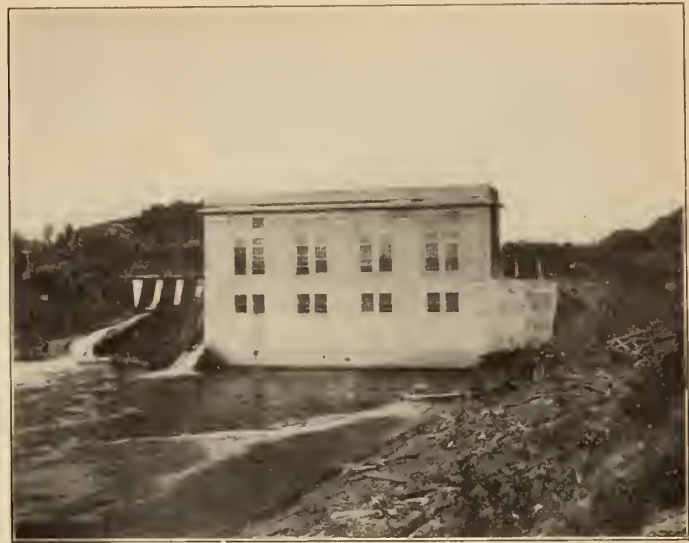
Plate No. 5.—Hydro-Electric Development of Mond Nickel Company at Nairn Falls on the Spanish River, Ontario, 4,800 horse power.
