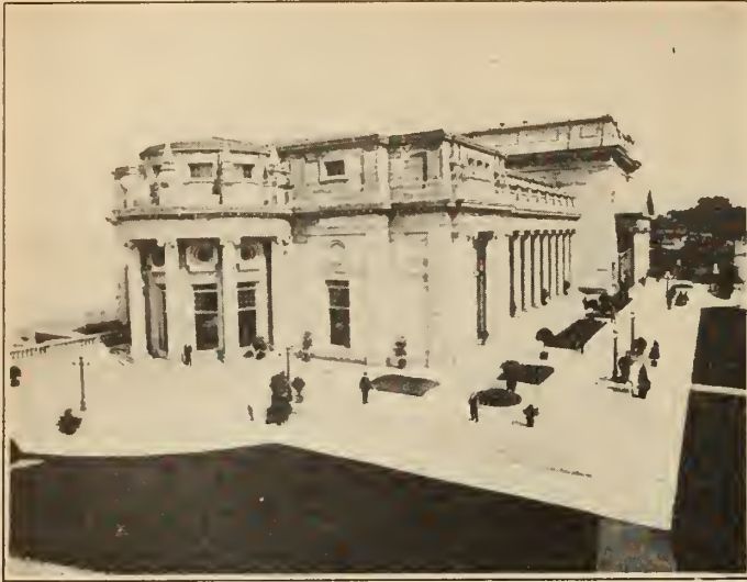
Electrical Development Company Plant of the Hydro-Electric Power Commission of Ontario at Niagara Falls — 164,000 h.p.
