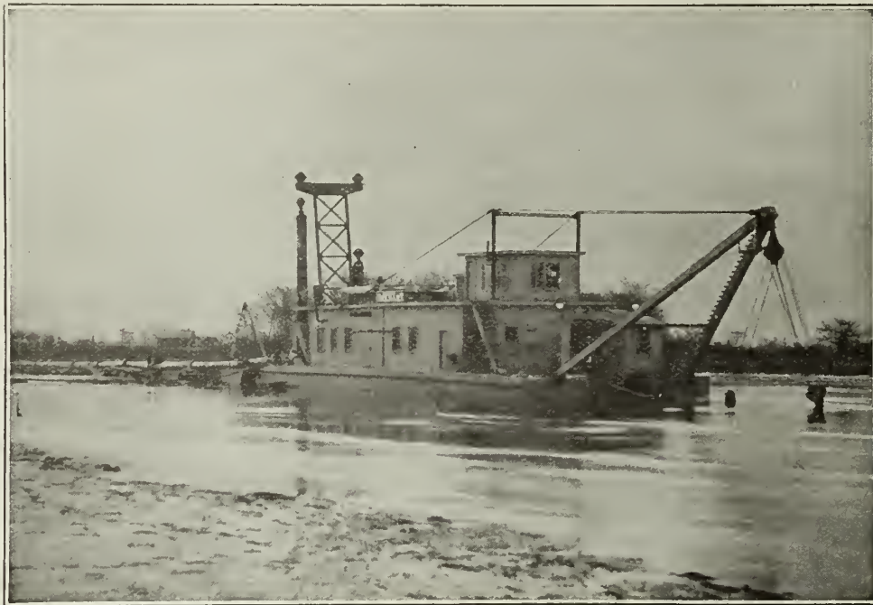
Electric Dredge on Queenston-Chippawa Power Development
