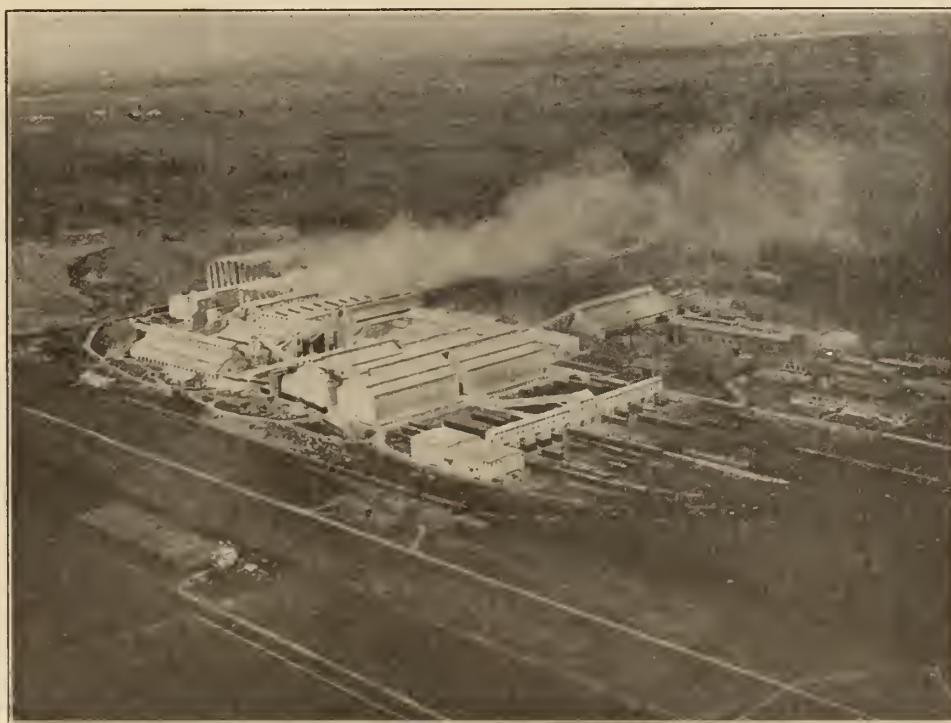
Plate No. 3.—Large Canadian Cement Mill, 10,000-barrel Capacity.
