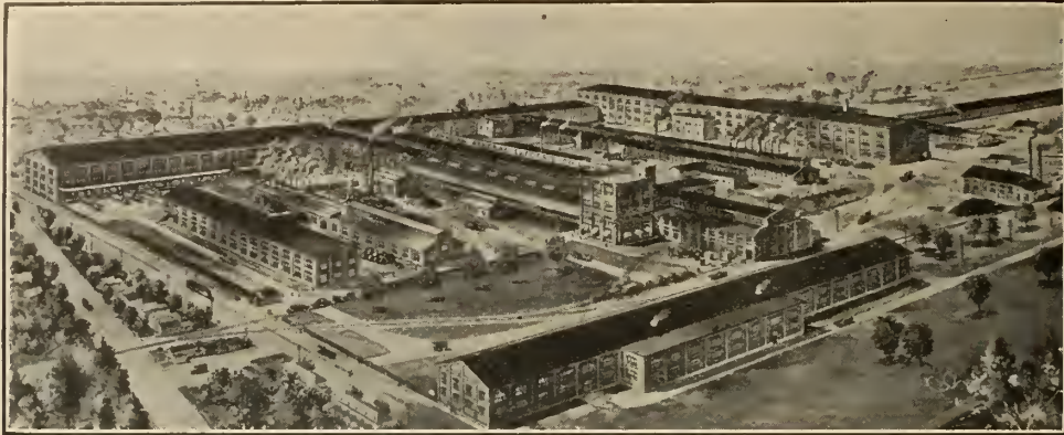
Bird's eye view of our main electrical works at Peterborough, Ont., covering 46 acres.
