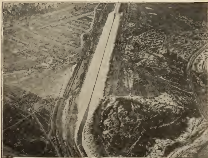
Plate No. C-10.—Aeroplane View of Trapezoidal Canal Section with Curve and Transitions.
