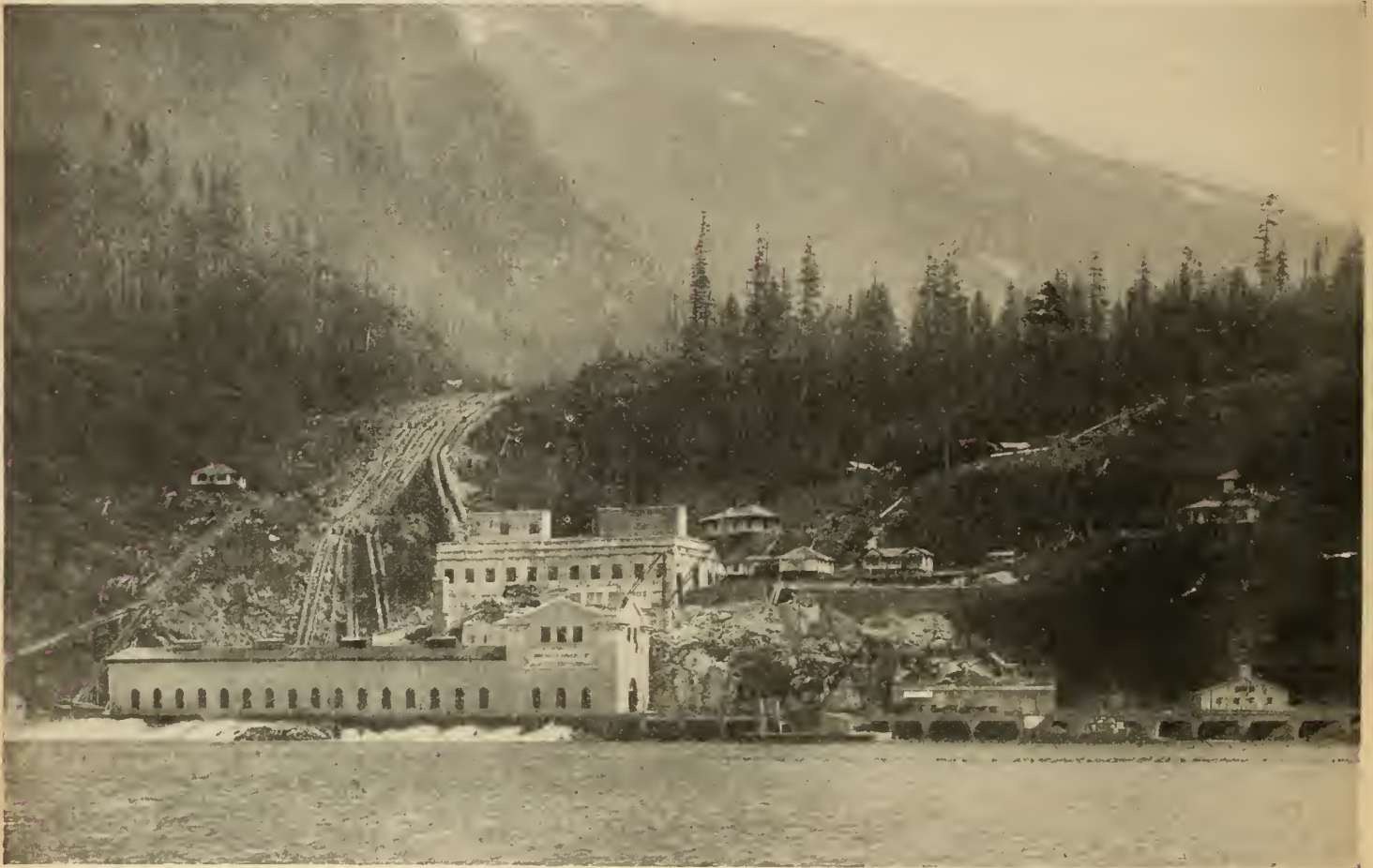
Coquitlam-Buntzen Development No. 1 of the British Columbia Electric Railway Company — 43,500 h.p.
