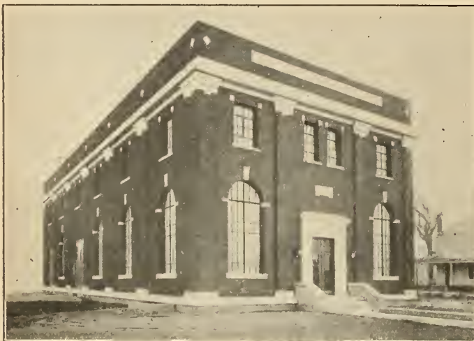
[Plate No. 12, — Modern Substation — Montreal.
