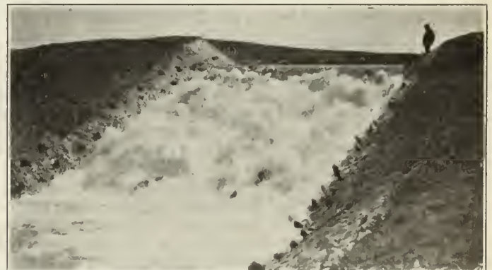
Fig. No. 7. Completed Rock Drop No. 7A, near Strathmore, Alta.
