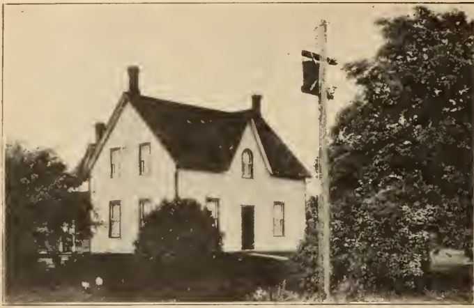
Plate No. 5a,—Rural Distribution of Power.
