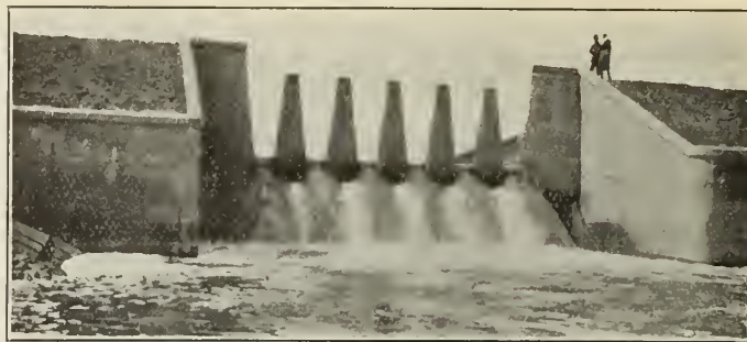
Fig. No. 4. Notch Drop No. 1, Main Canal.
