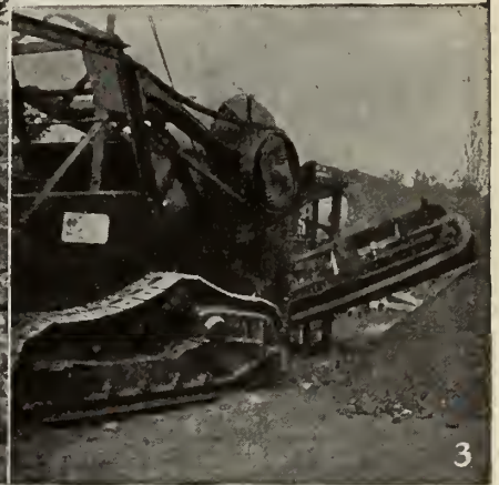
3—A close-up of the ditcher, showing discharge.
