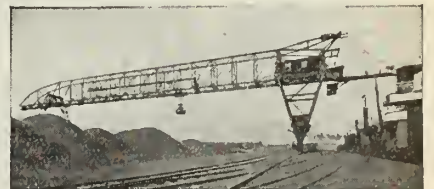
COAL HANDLING BRIDGE
