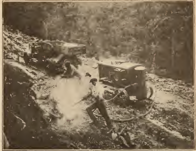
Plate No. 5.—Portable Compressor and Jackhammer Drills on Road Construction Work.
