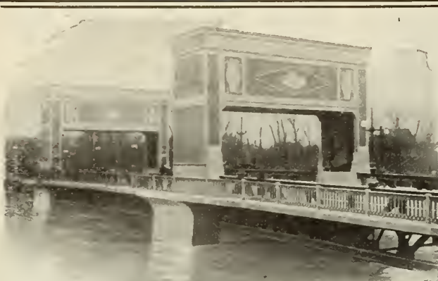
STRAUSS VERTICAL OVERHEAD COUNTERWEIGHT BASCULE. COUNTERWEIGHTS CONCEALED OSBORNE ST. BRIDGE, WINNIPEG.
