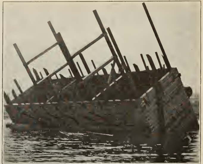
Figure No. 3.—Launching Caisson
