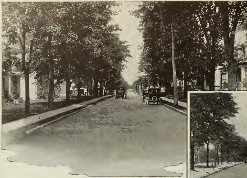
Wellington Street, Stratford, Ont., Tarvia-built 1913, in excellent condition after 11 years of traffic.
