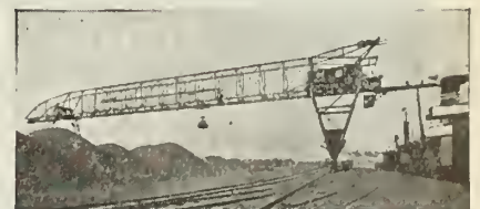
COAL HANDLING BRIDGE
