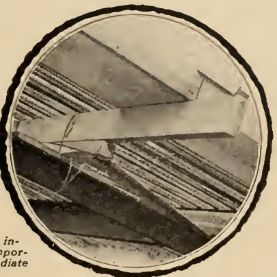
Method of installing temporary intermediate supports.
