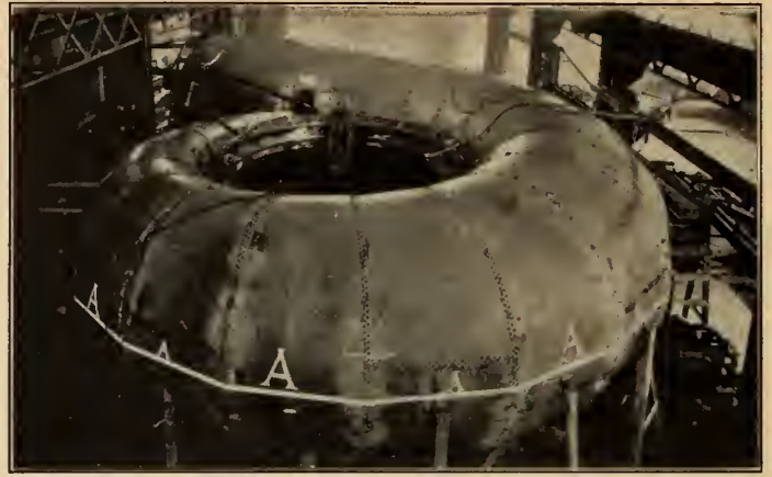
Plate No. C-36.—Steel Plate Scroll-case under Construction.
