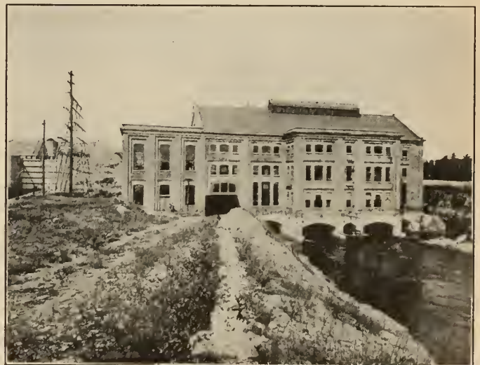
Healey Falls Development on the Trent River, of the Hydro-Electric Power Commission of Ontario — 16,800 h.p.
