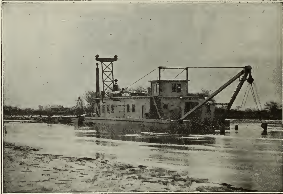
Electric Dredge on Queenston-Chippawa Power Development
