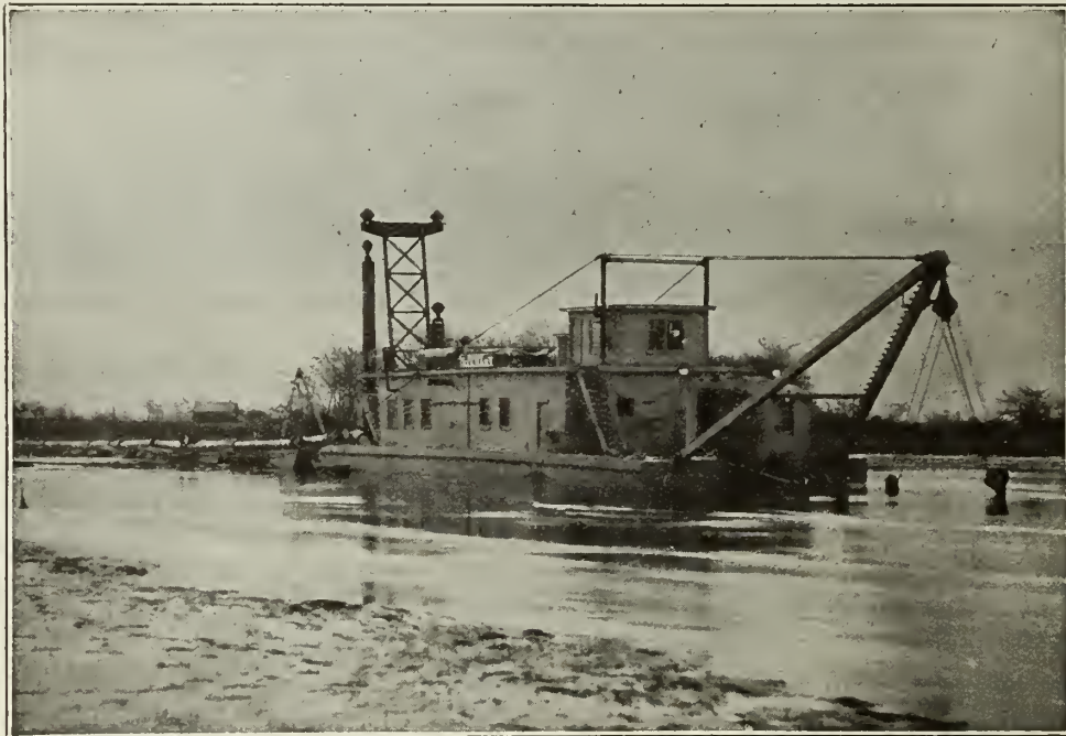
Electric Dredge on Queenston-Chippawa Power Development
