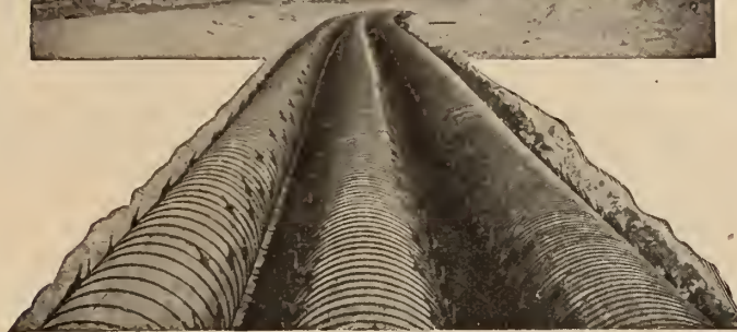
GROUP OF CONTINUOUS STAVE PIPES
